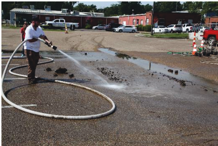
Figure 18. Washing large dirt clods off asphalt driveway.
