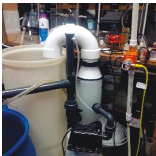
Figure 24. Picture of the foam separation skimmer.
