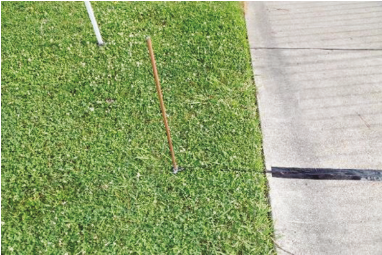
Figure 6. Generator grounding stake.
