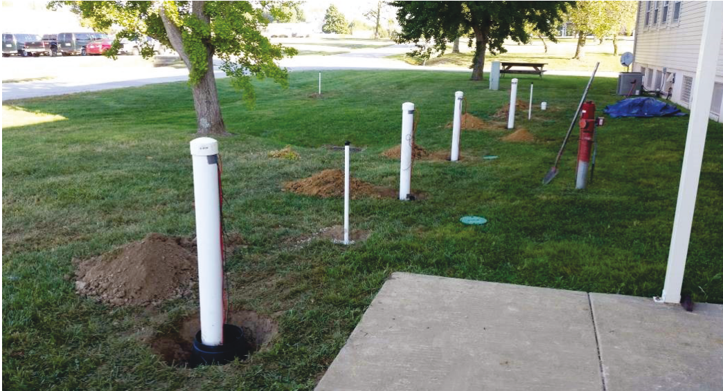
Figure 5. ISWEOD wells and piezometers during installation.
