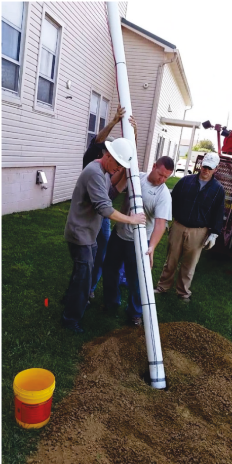
Figure 6. ISWEOD well installation on west side of building.
