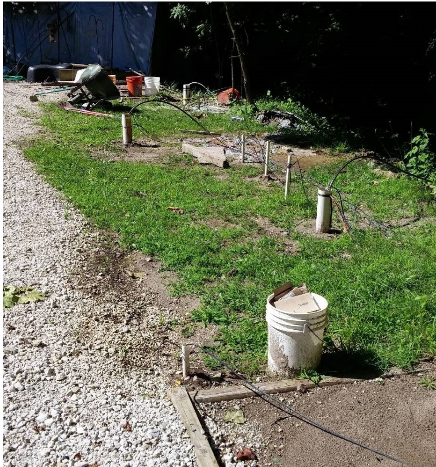
Figure A17. Photograph showing complete layout of second pilot test site. PZ-BKGRD is closest, followed (near to far) by Well 1, PZ-1, PZ-4, PZ-2, Well 2 (off line with others), PZ-3, and Well 3.
