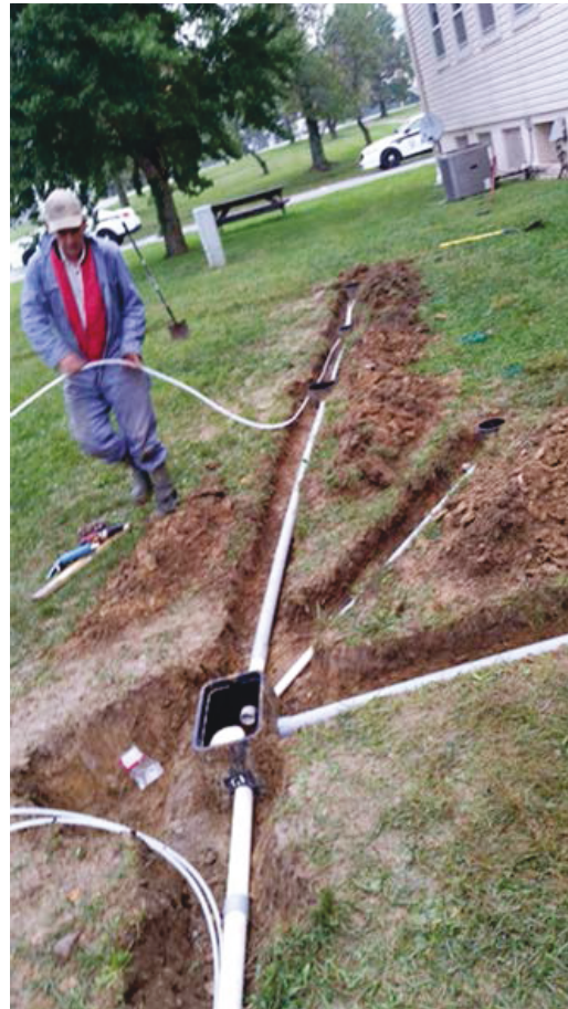
Figure 7. Vault, conduit, and drain line (tubing) installation.
