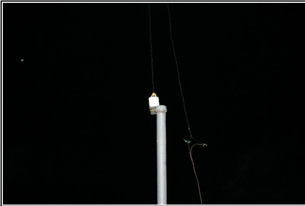
Figure 1-2. Demolition charge being aligned for detonation.
