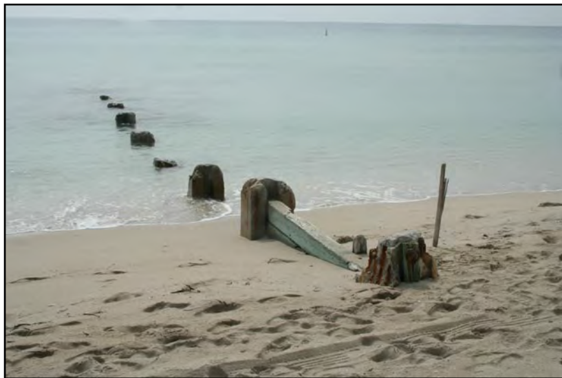
Figure 1. Beach view of exposed groin (E) on Bal Harbour Beach.
