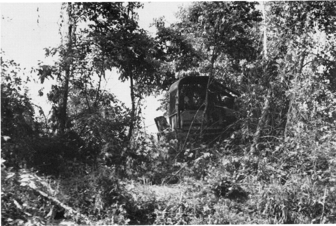
Figure 3. D-3 bulldozer used to clear the bank
