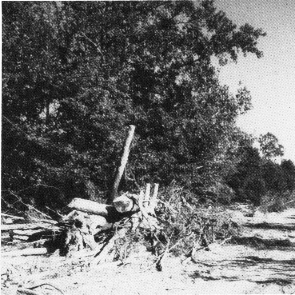
Figure 7. Access road on side of channel designed to minimize disturbance to the riparian environment. Channel is to right edge of road just outside photo
