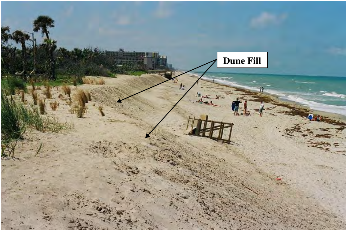
Figure A-20. Mid Reach dune fill, constructed in 2005
