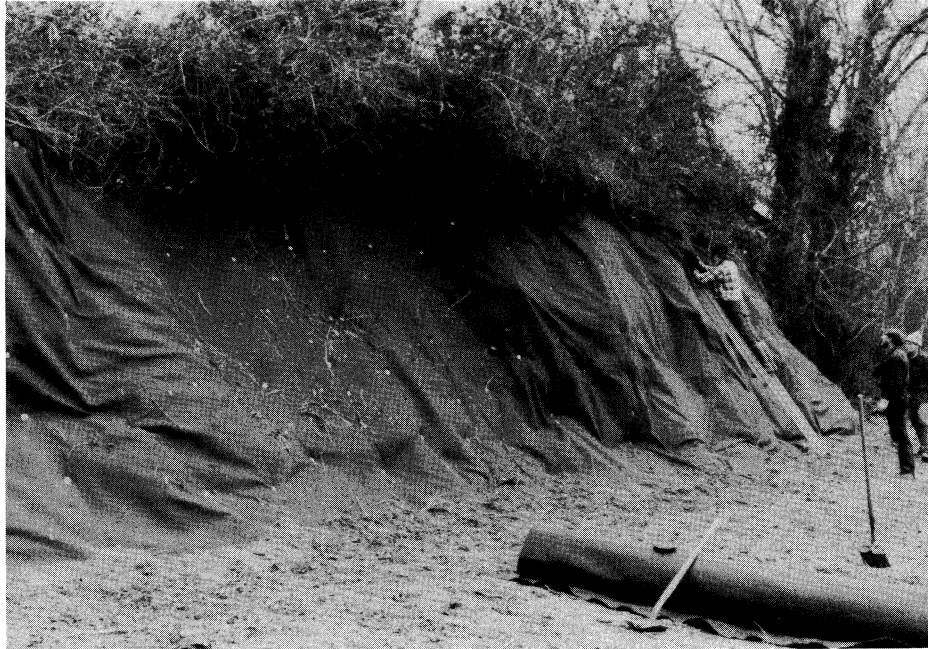
Figure 7. Filter fabric covering on Huffine Island Mound, Watts Bar Lake, Tennessee
