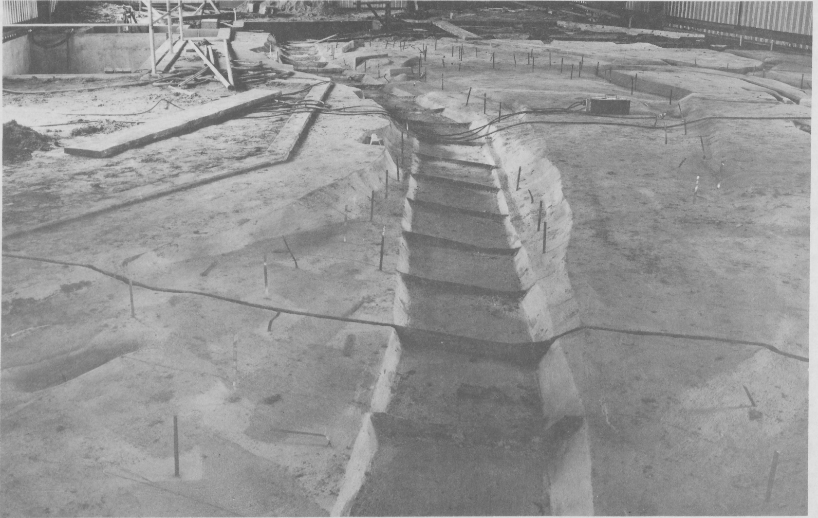
Figure 3-14. Trough for later installation of enlarged channel.
