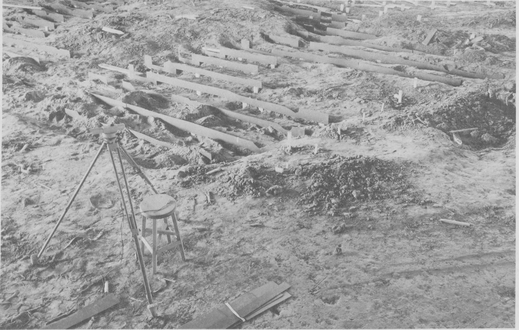
Figure 3-10. Rough-graded templates.
