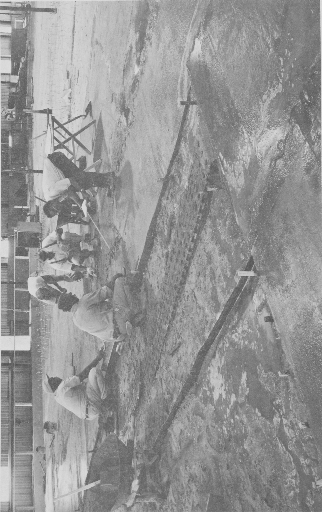
Figure 3-12. Sketching details before molding.
