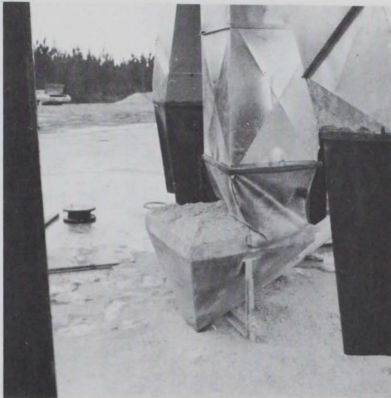
Figure 5.33 Storage hopper-feed hopper arrangement.
