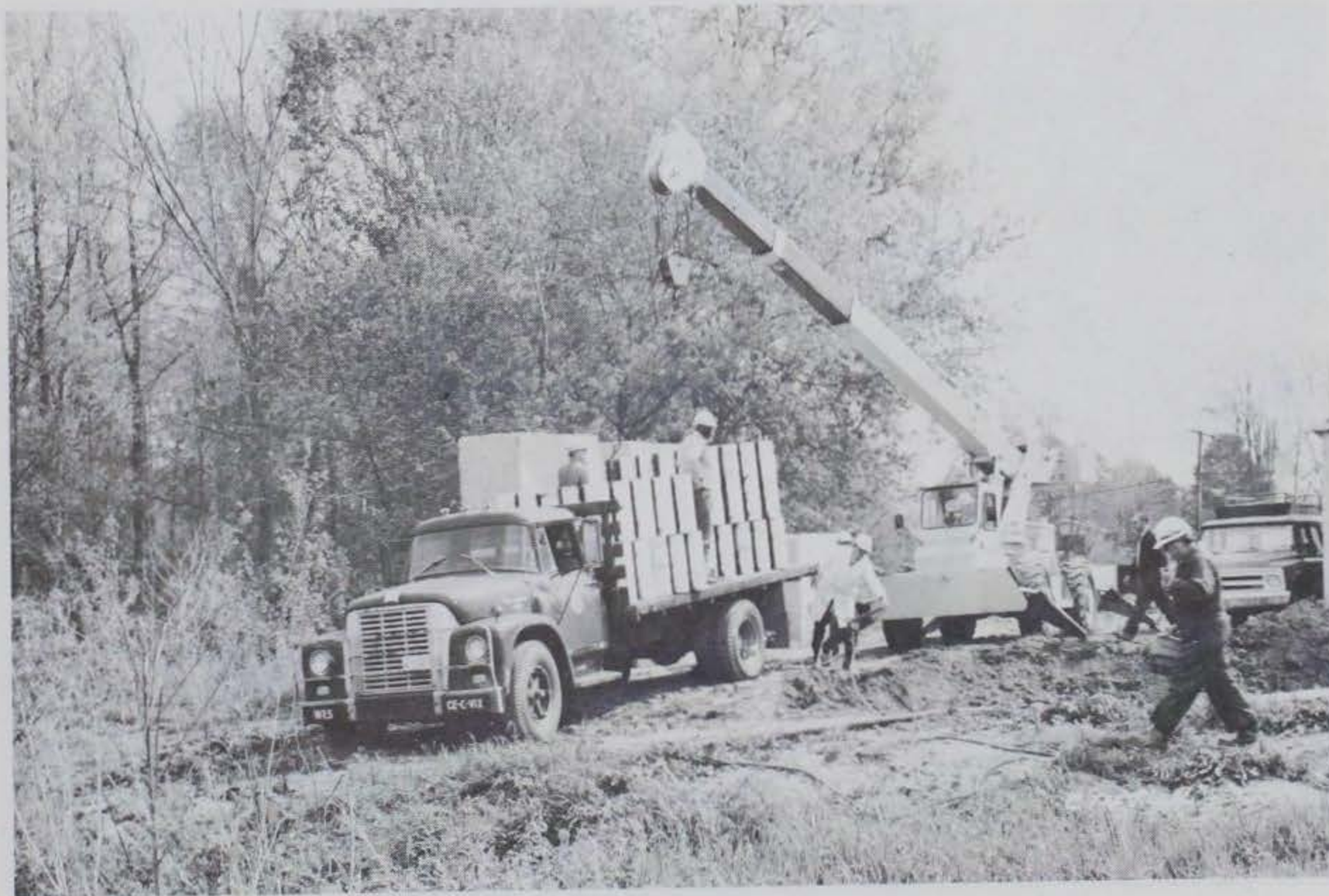
Figure 5.14 Unloading of PVC pipe modules.
