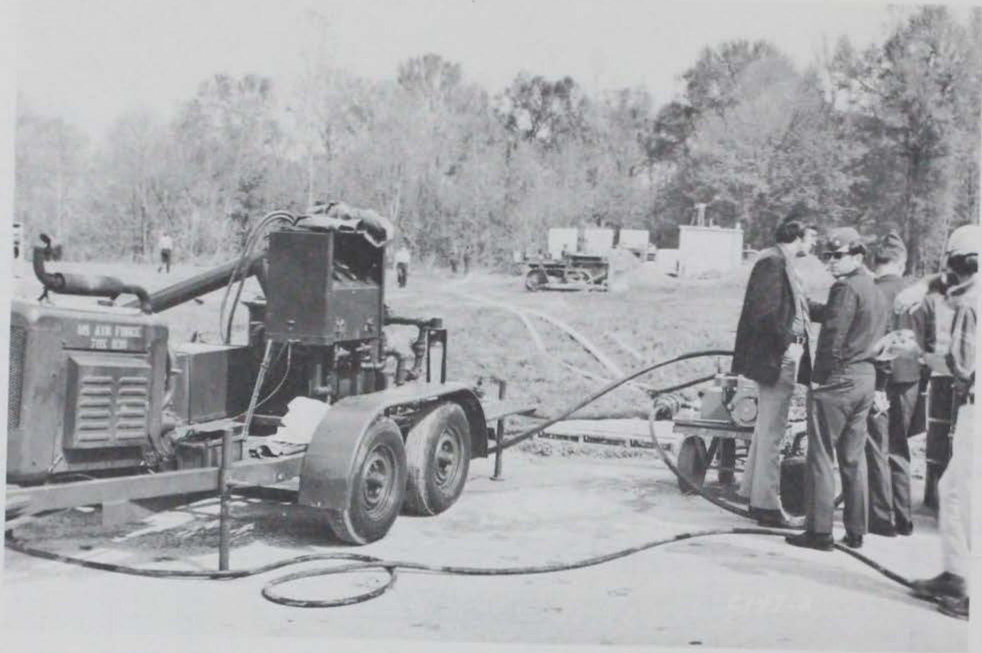
Figure 5.11 Batching and pumping unit - WES one-sixth-size crater trials.
