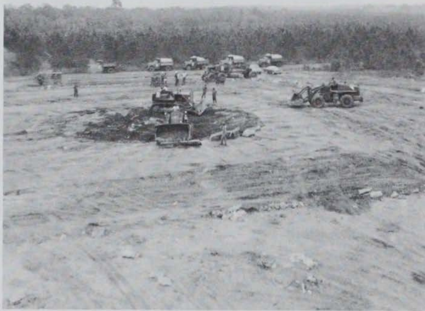
Figure 1.13 Removal of damaged pavement and compaction of debris in crater.
