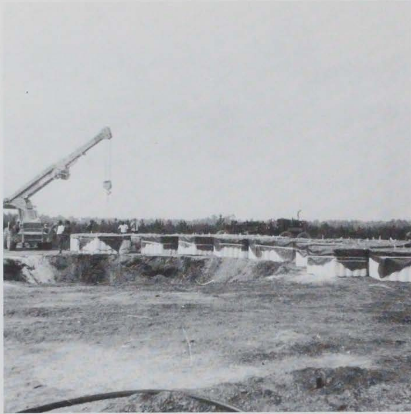
Figure 5.63 Sealed modules ready for placement in the crater.
