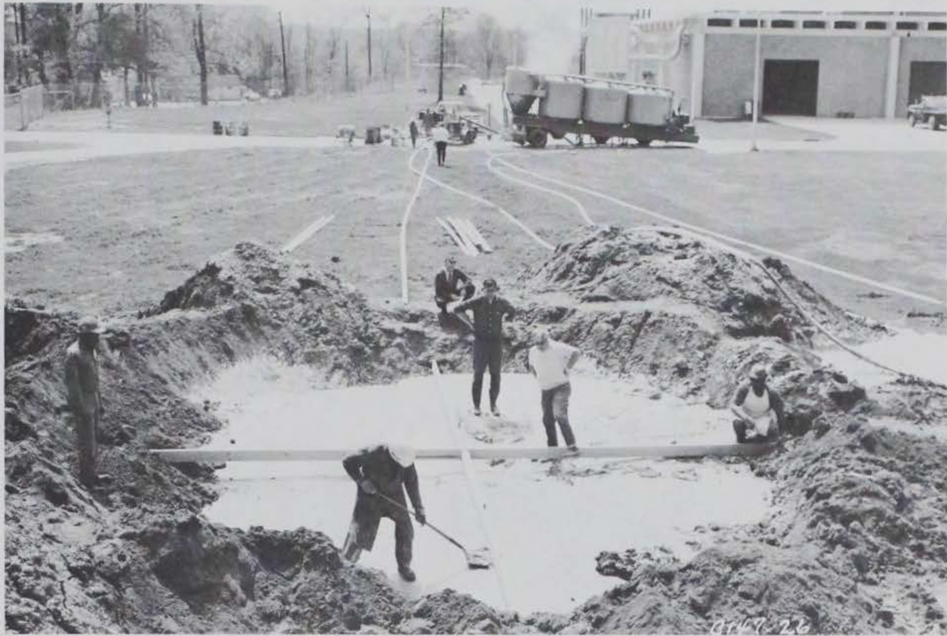
Figure 5.25 Placement of joint boards.
