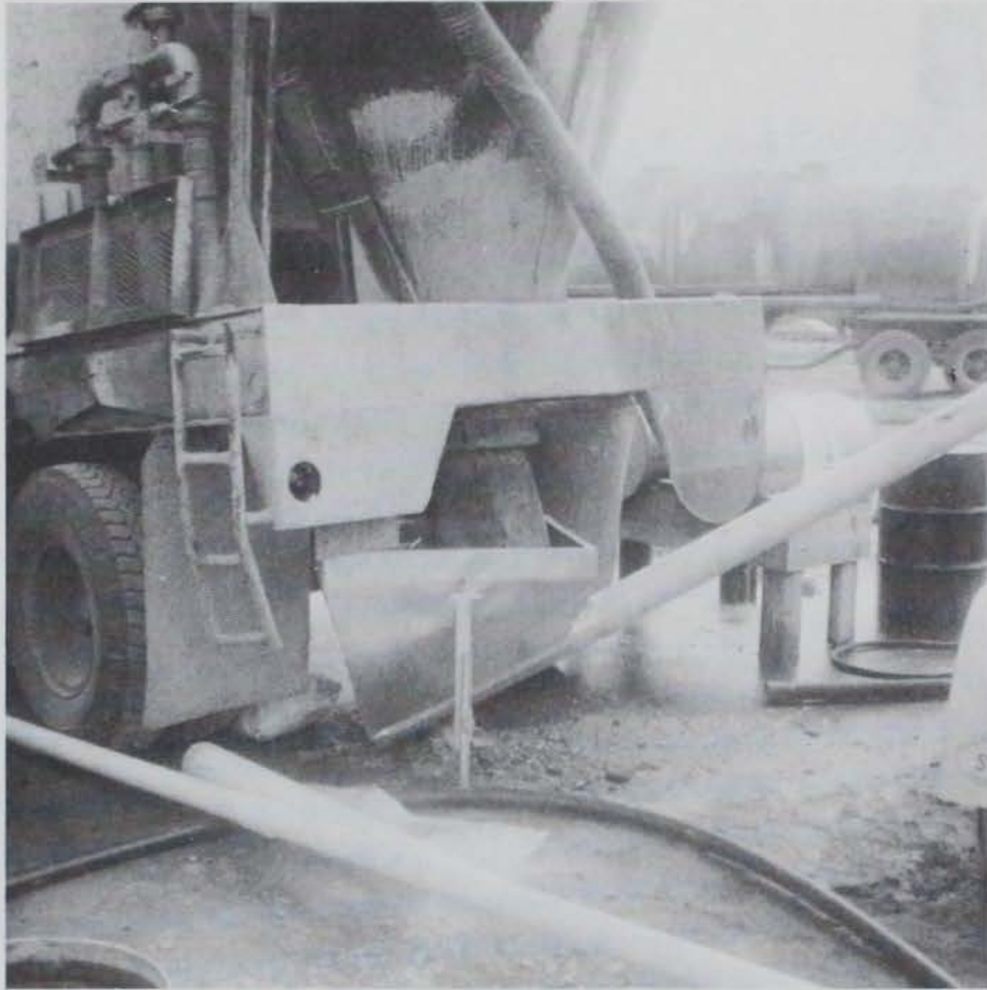
Figure 5.35 Cement feed arrangement.
