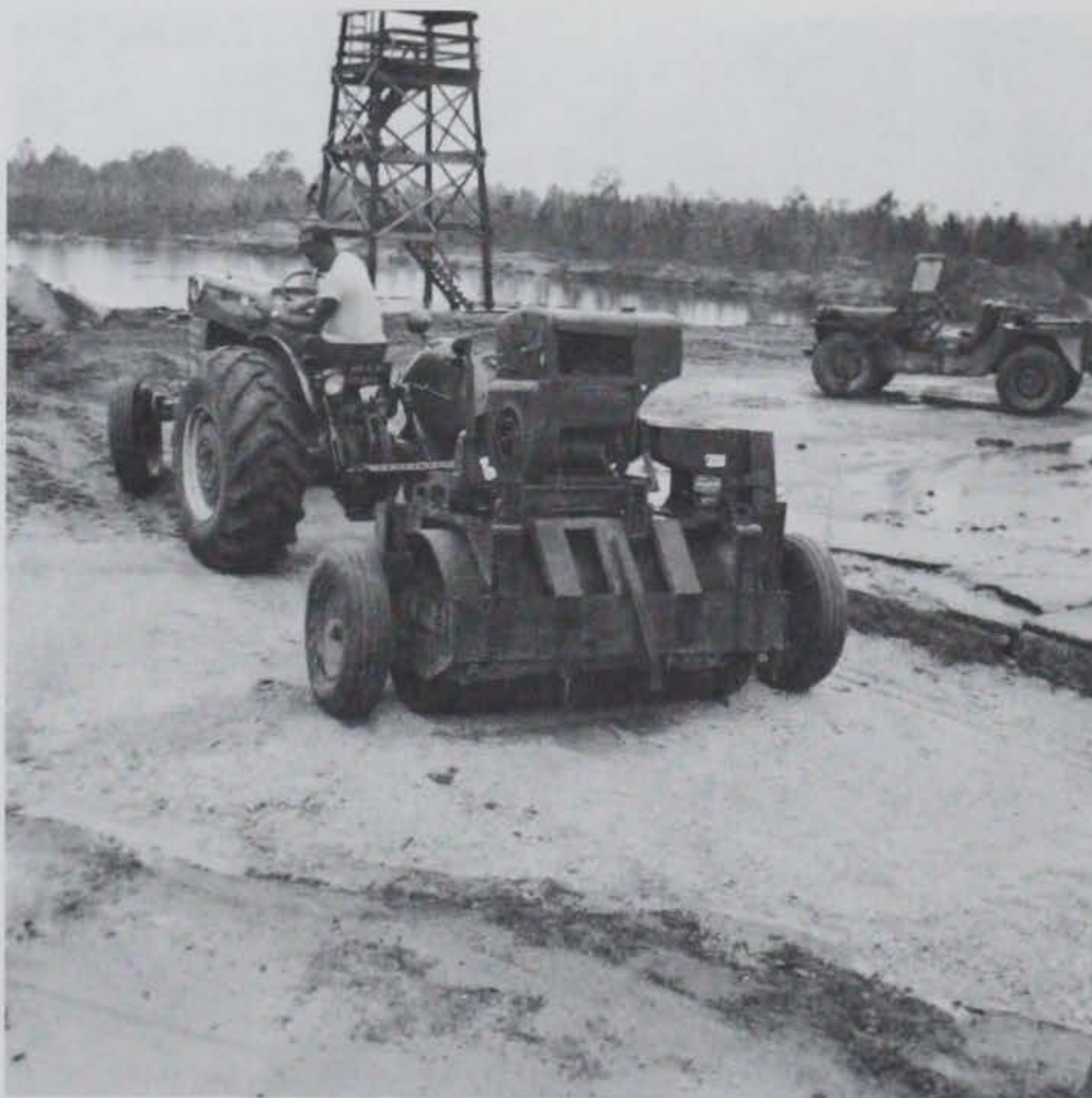
Figure 5.44 Vibratory-roller compaction of fill aggregate.
