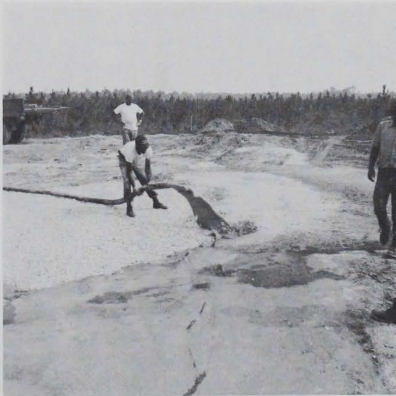
Figure 5.54 Placement of slurry on fill surface.
