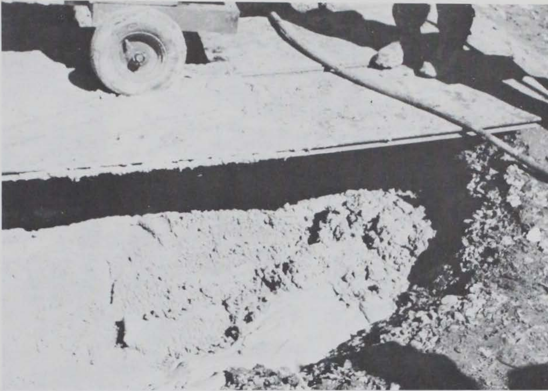
Figure 5.4 Concrete surface immediately after completion of the 65-pcf cellular concrete placement.
