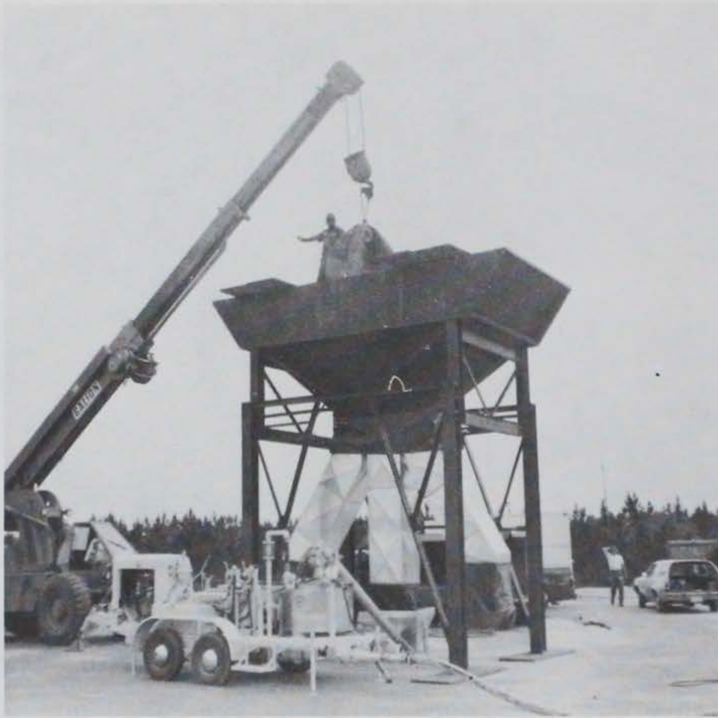
Figure 5.31 Gravity-feed cement storage hopper.
