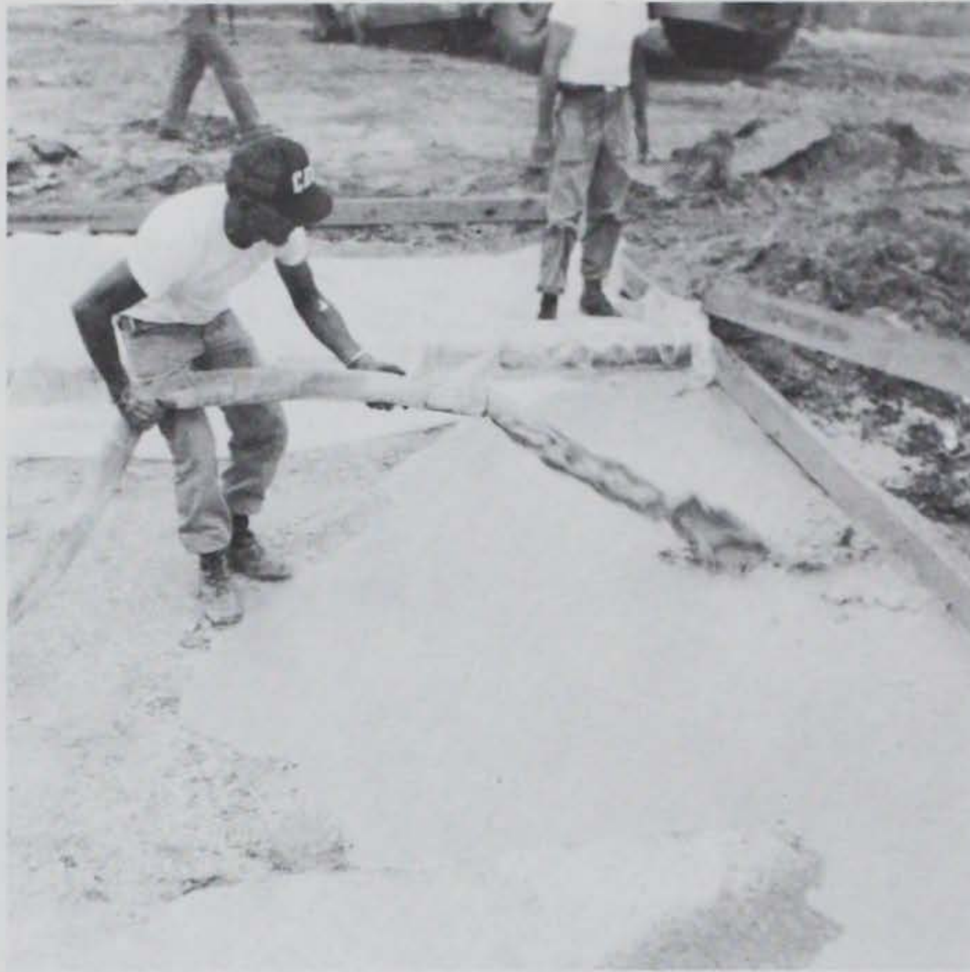
Figure 5.47 Flexible hose for ease of movement during placing.
