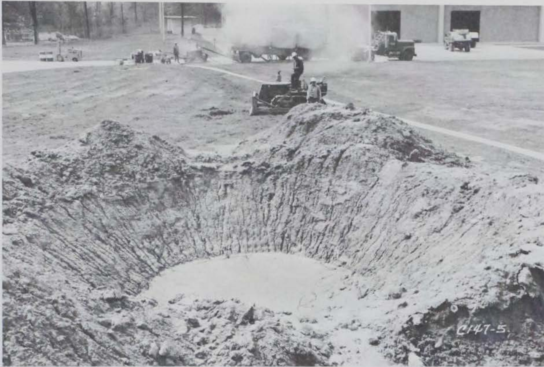
Figure 5.21 Crater for the cellular concrete backfill test.
