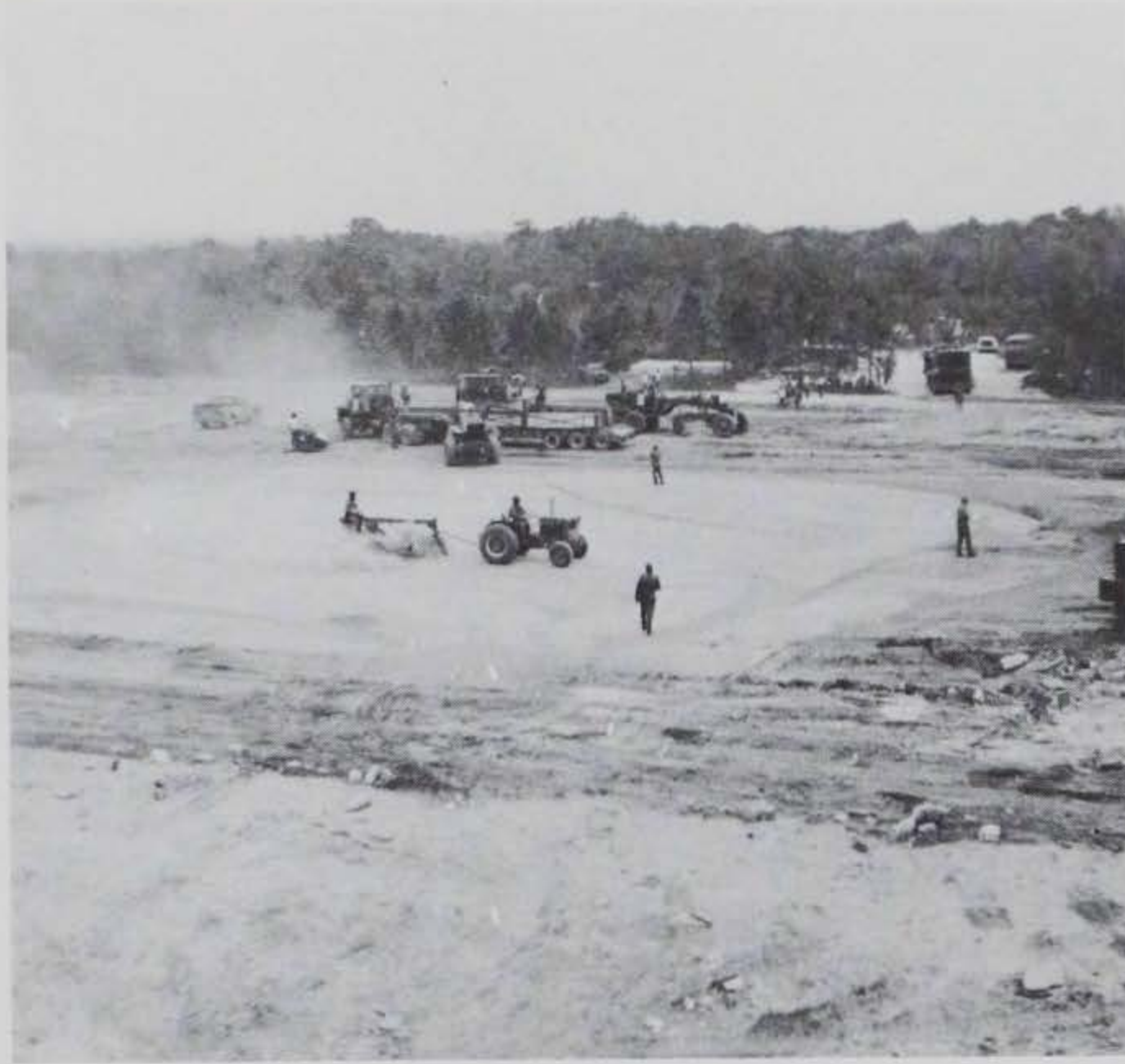
Figure 1.11 Sweeping adjacent area for mat assembly.
