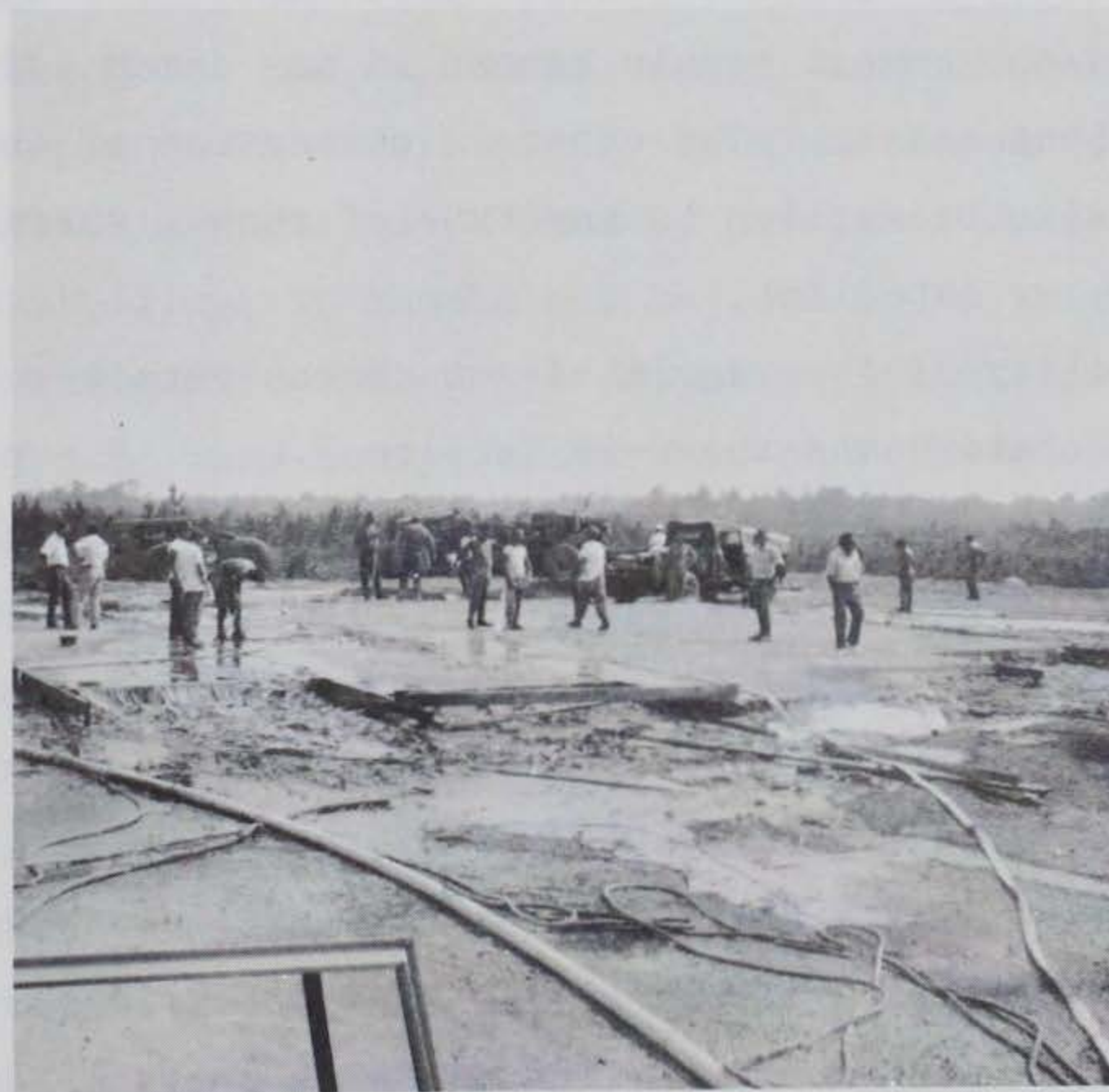
Figure 5.70 Top surface of completed repair.
