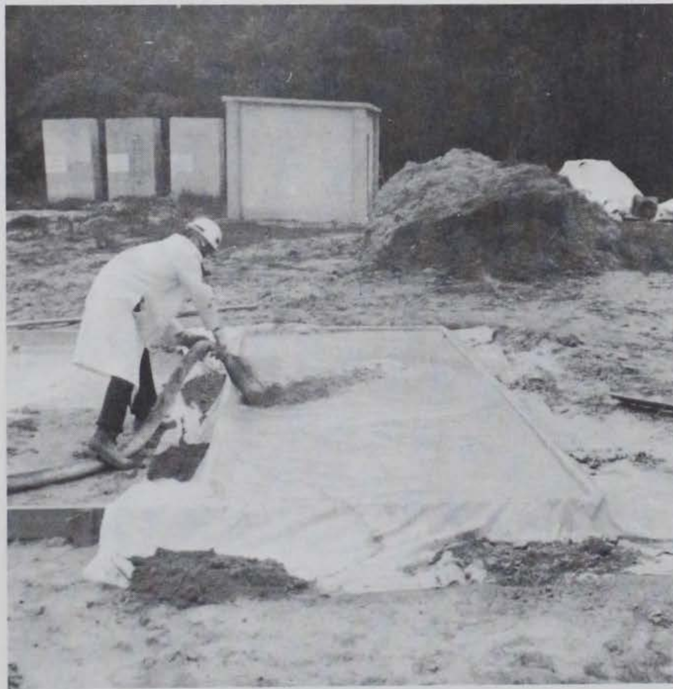
Figure 5.30 Small slab preparation.
