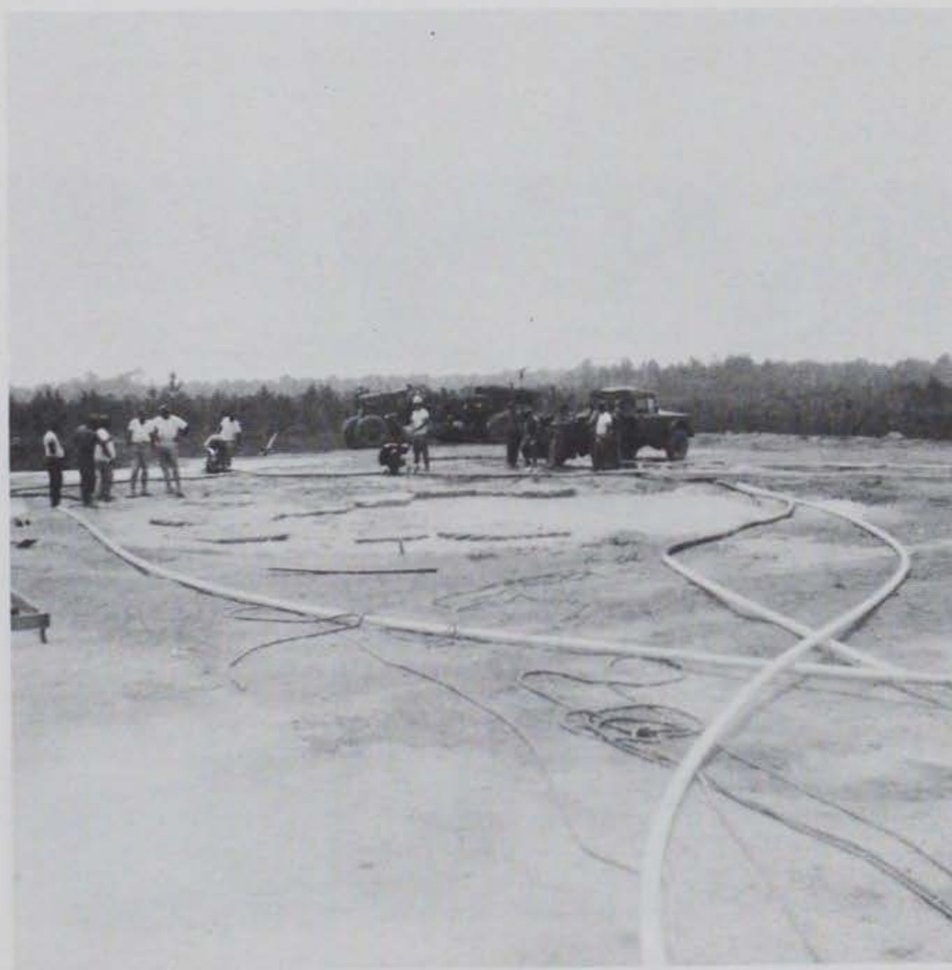
Figure 5.66 Top surface of cellular concrete fill placement.
