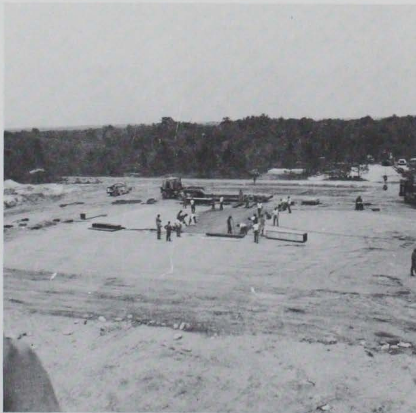
Figure 1.14 Mat surfacing assembly.
