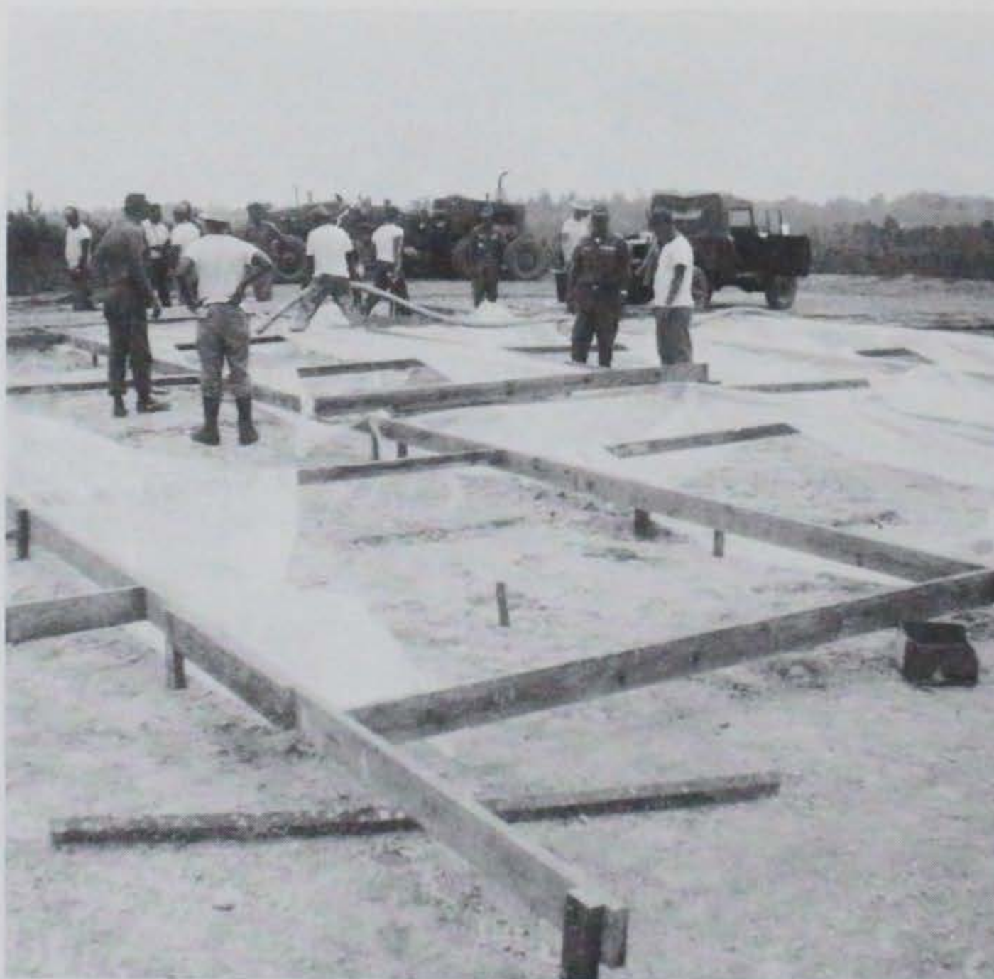
Figure 5.68 Form and joint boards in place over backfilled modules.
