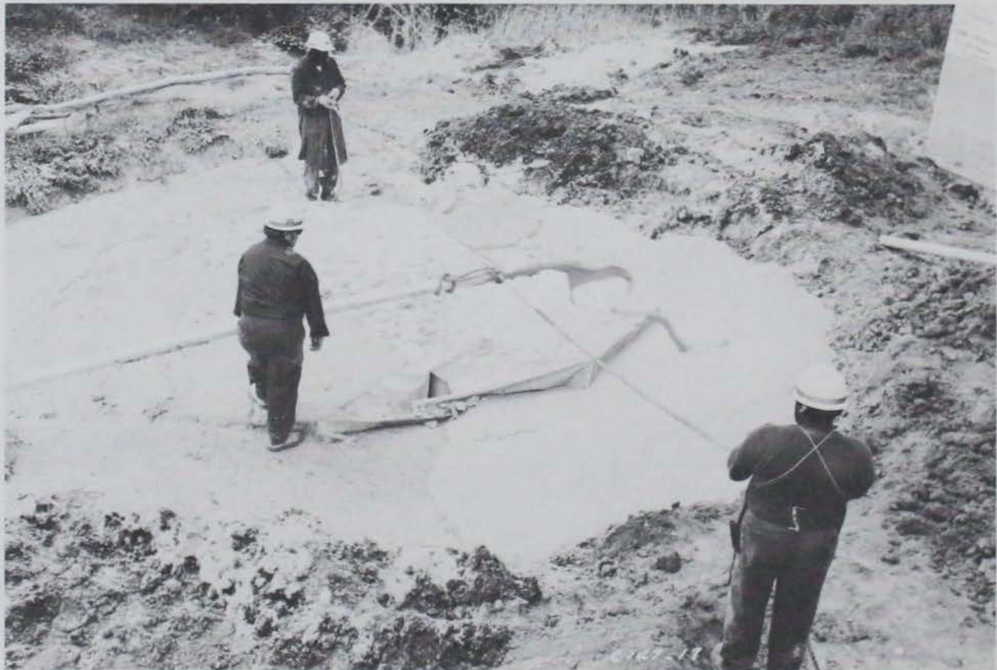
Figure 5.20 Completion of cellular concrete placing.
