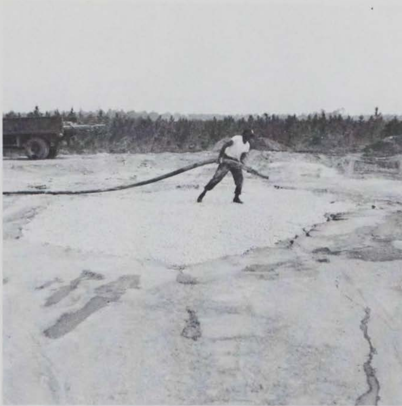
Figure 5.53 Select fill aggregate placed to existing pavement surface.
