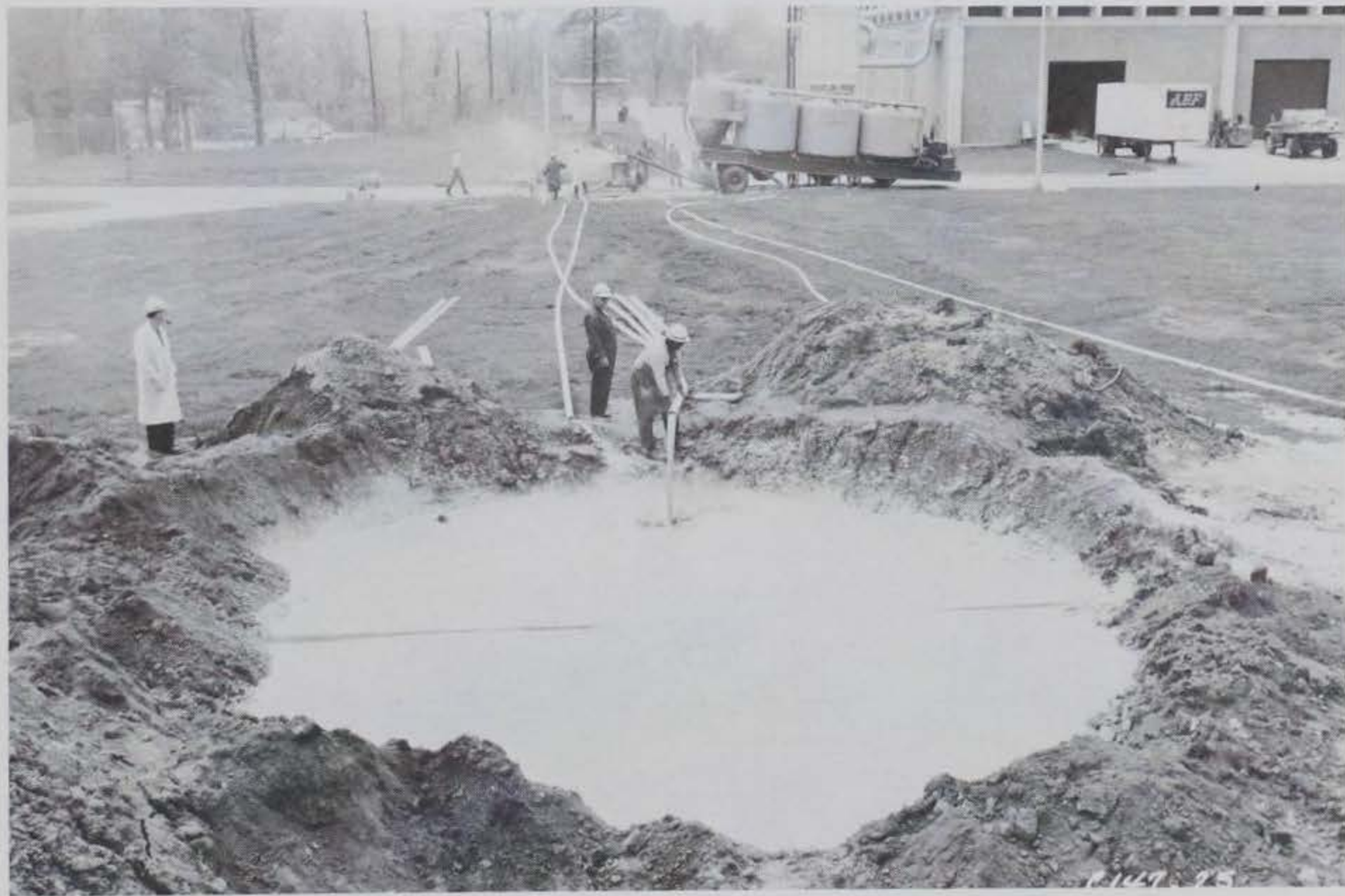
Figure 5.26 Placement of the capping material.
