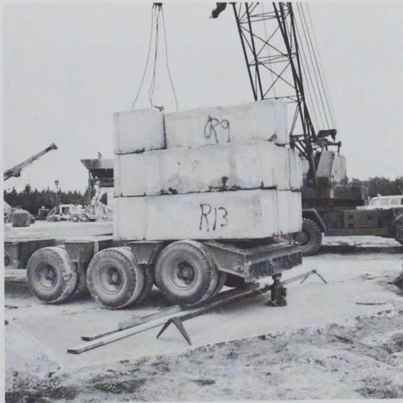
Figure 5.50 Loading of repaired crater by cart loaded with 50,000 pounds of blocks.
