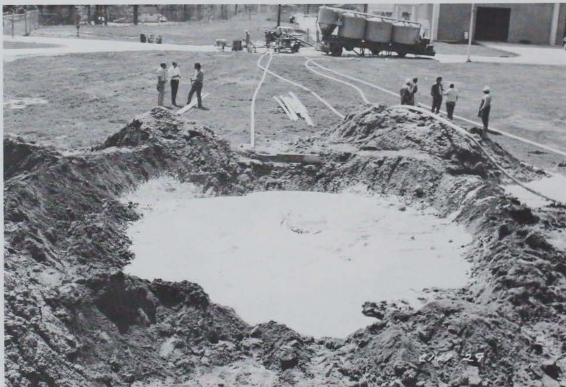
Figure 5.24 Top surface of cellular concrete backfill.
