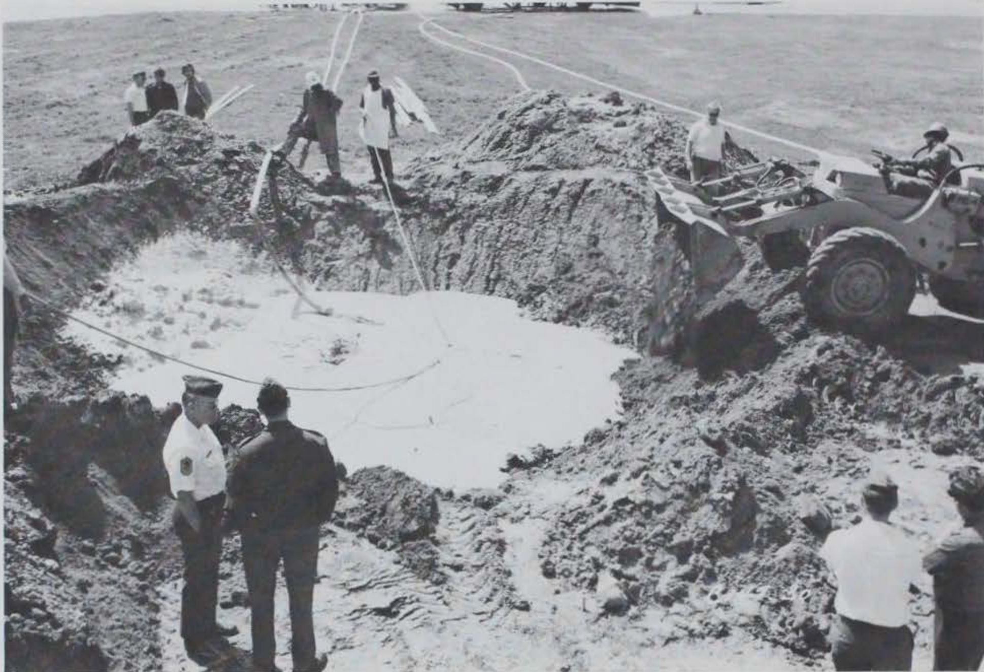
Figure 5.23 Crater half-filled with cellular concrete backfill.
