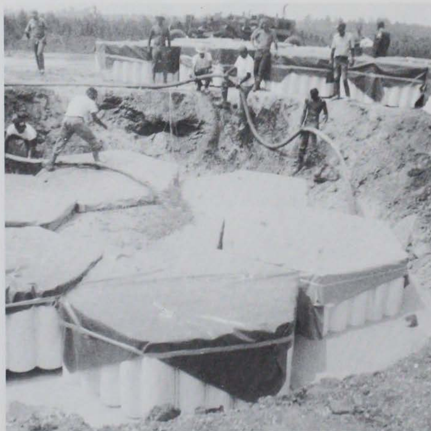
Figure 5.64 Placement of cellular concrete around modules.
