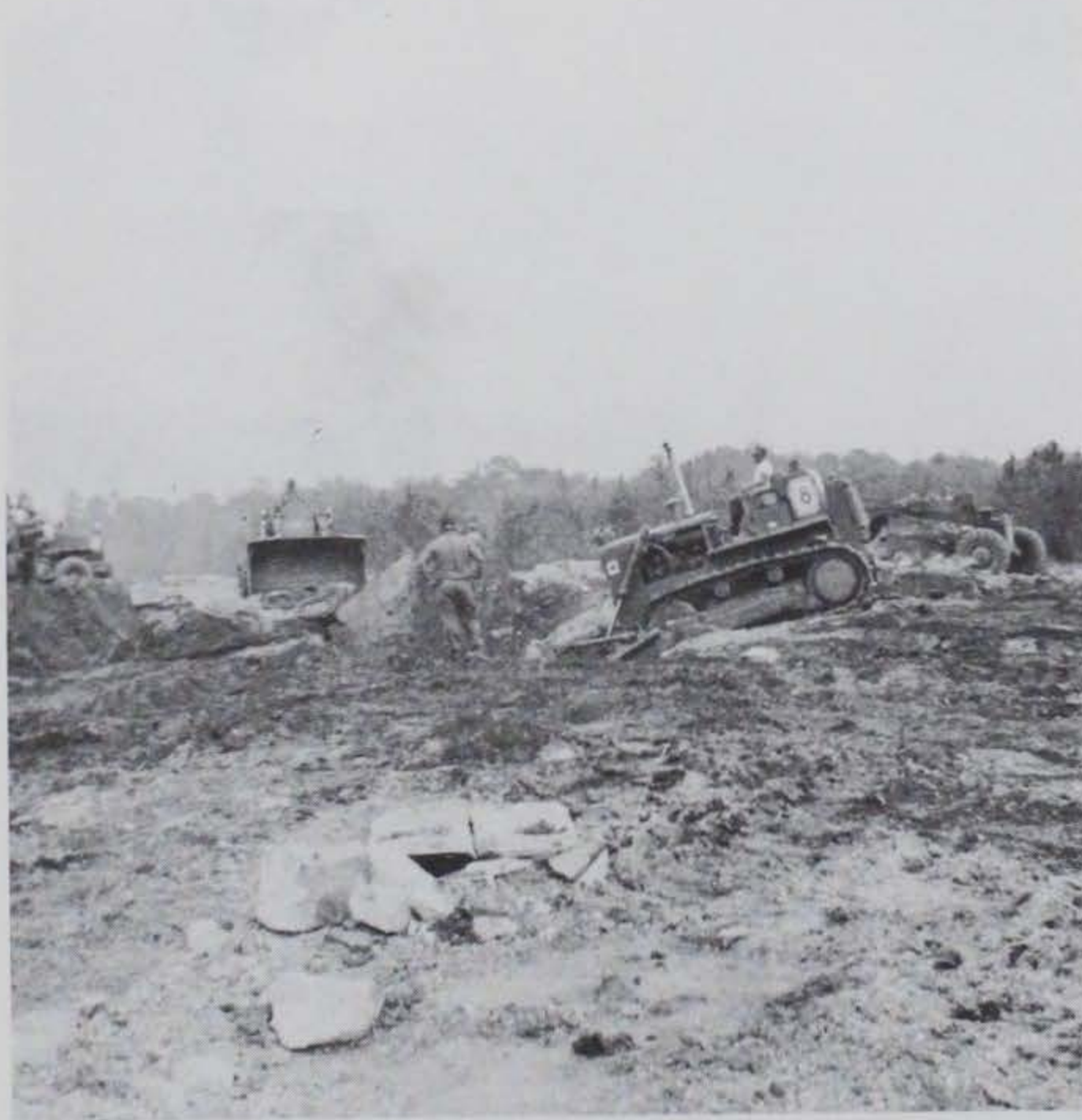
Figure 1.11 Sweeping adjacent area for mat assembly.
