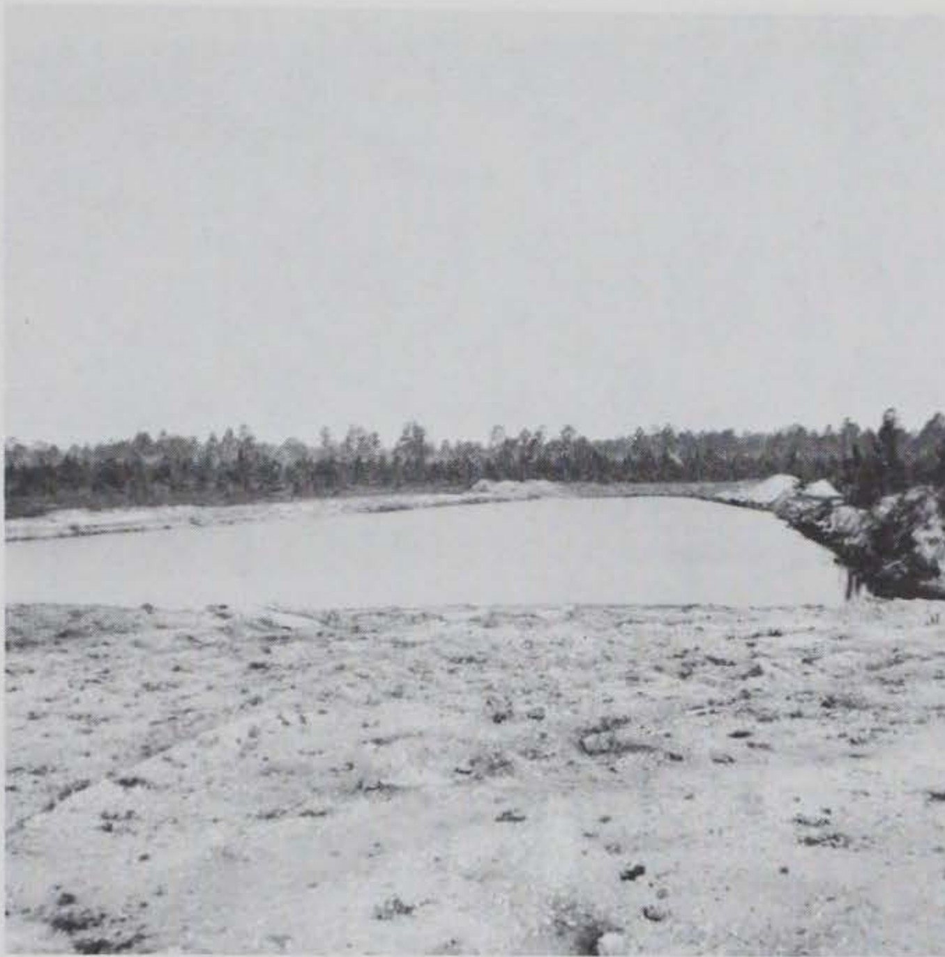
Figure 5.41 Water supply impoundment.
