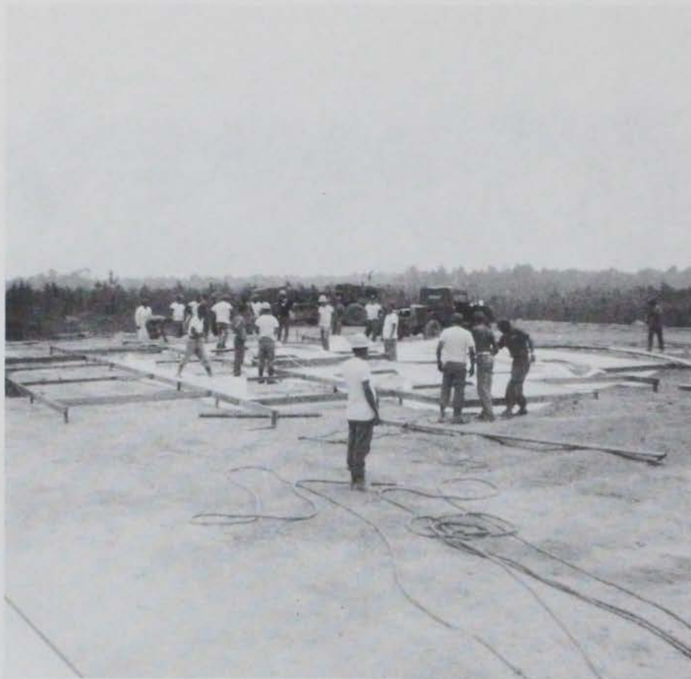
Figure 5.67 Form and joint boards being assembled.
