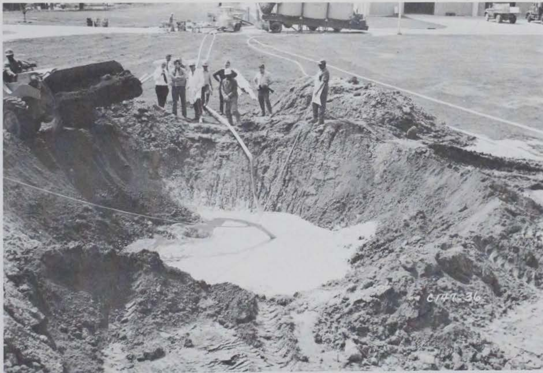
Figure 5.22 Start of the cellular concrete backfill repair.
