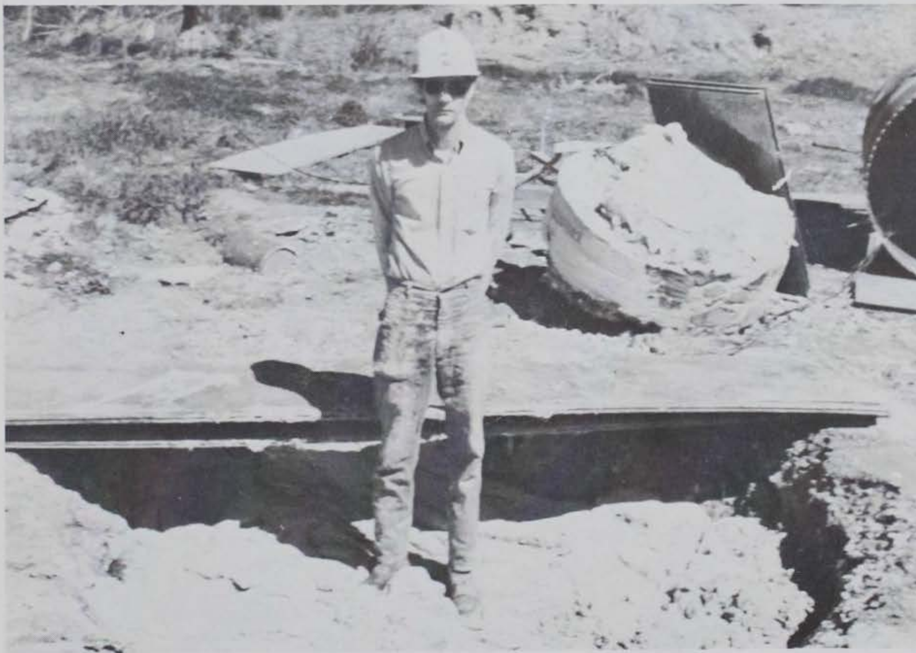
Figure 5.5 Concrete surface 10 minutes after completion of the 65-pcf cellular concrete placement.
