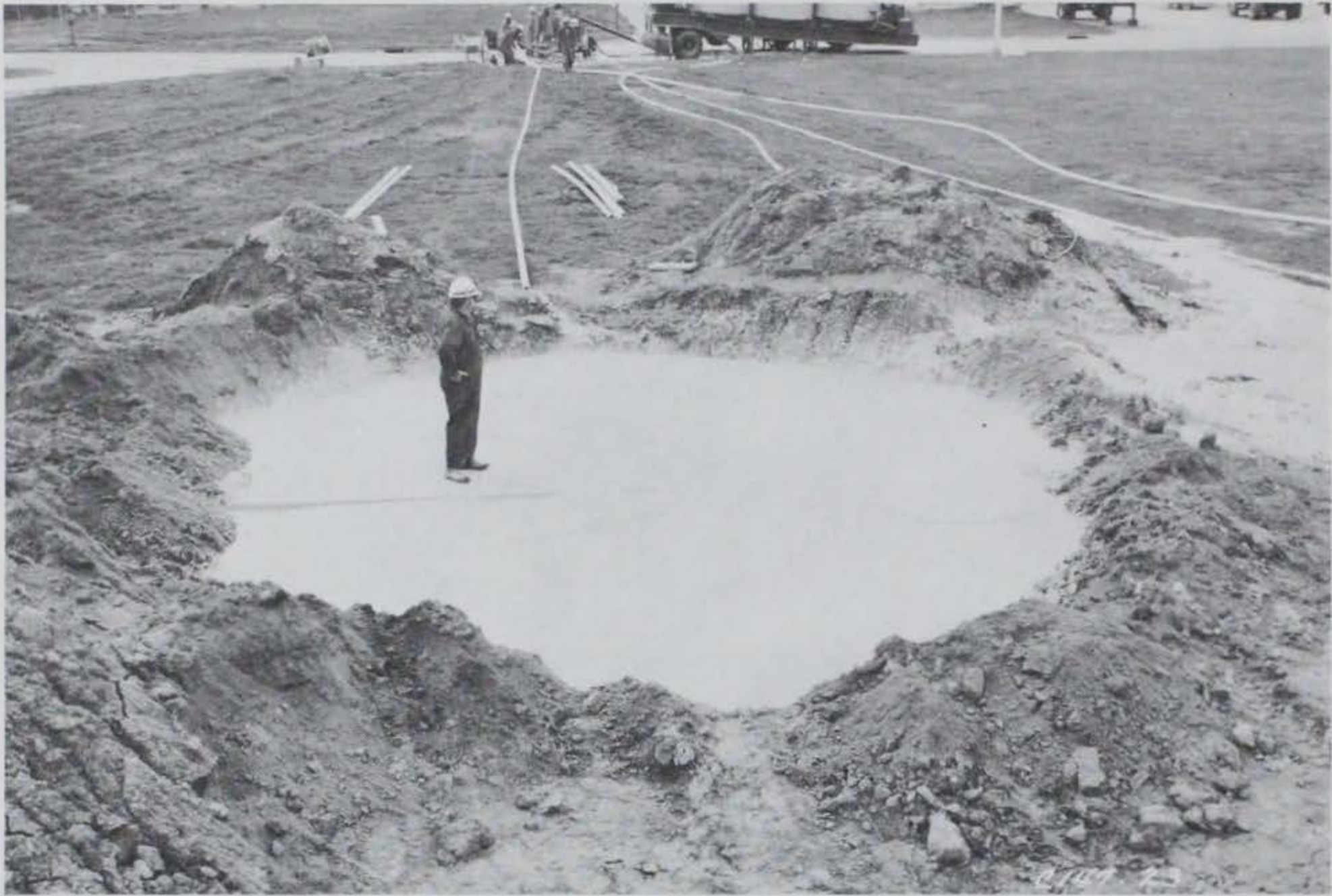
Figure 5.27 Finished repair for the cellular concrete backfill test.
