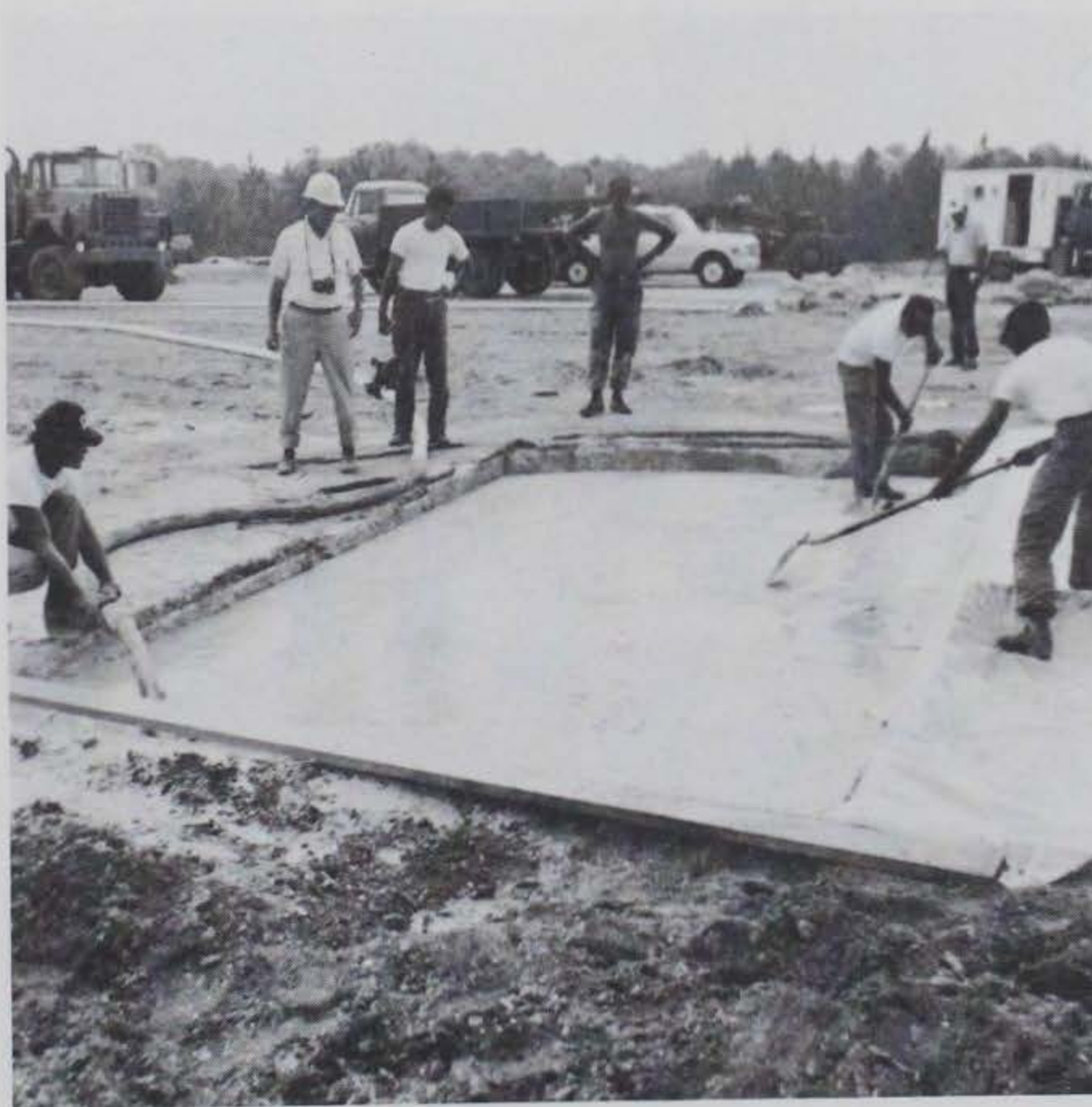
Figure 5.46 Placement of neat cement slurry cap.
