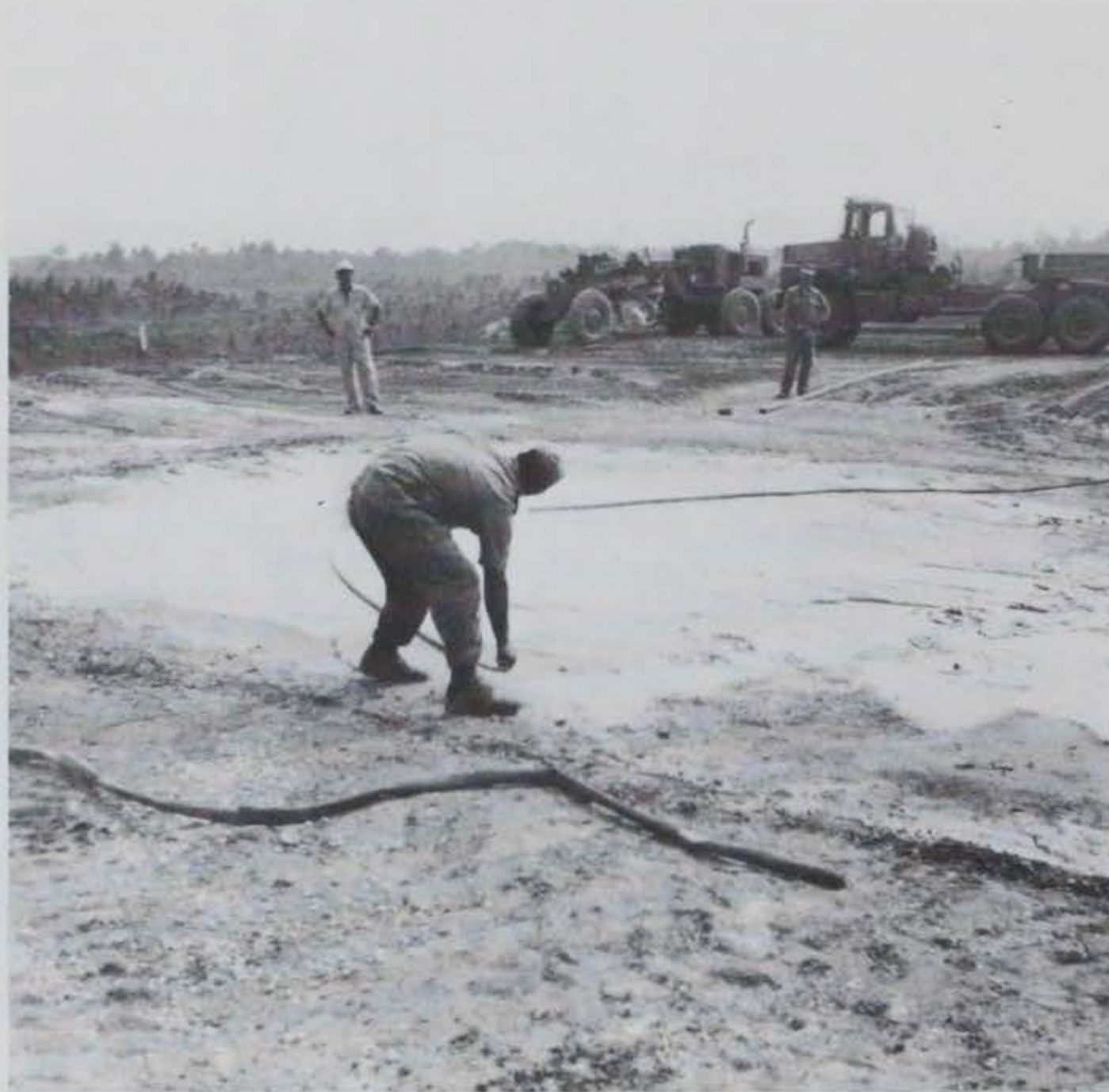
Figure 5.55 Screeding of repair surface.
