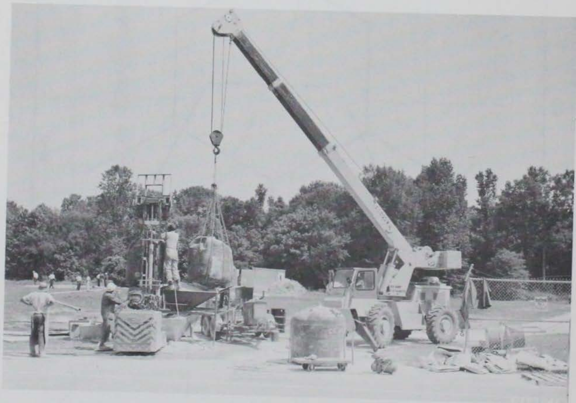
Figure 5.12 Batching operation using rubberized storage bags for cement handling.
