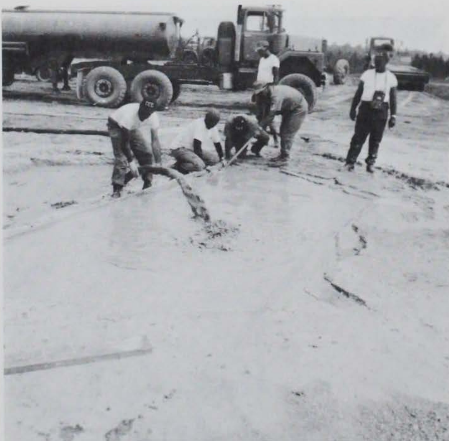
Figure 5.60 Placement of slurry over cellular concrete fill.
