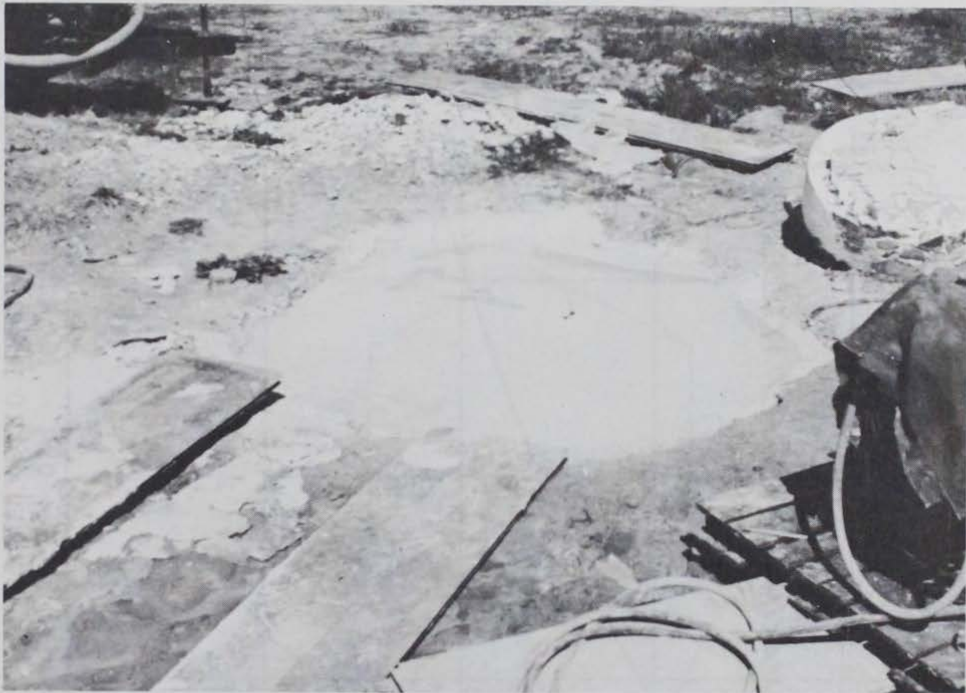
Figure 5.8 Repair surface shortly after additional capping material added.
