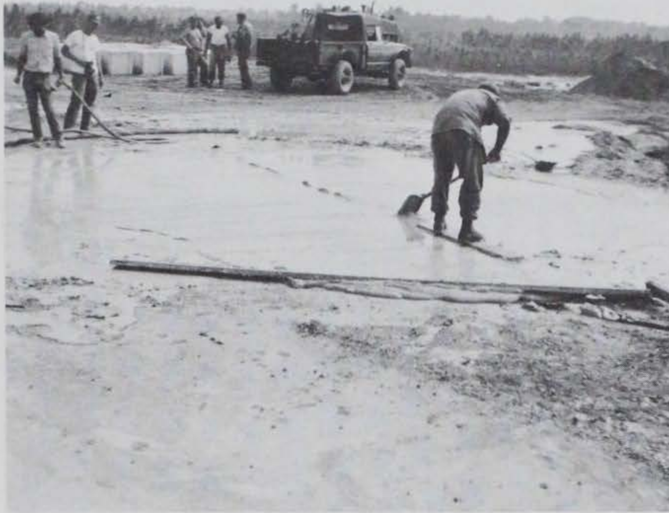
Figure 5.61 Completed surface of blow-out crater 3 repair.
