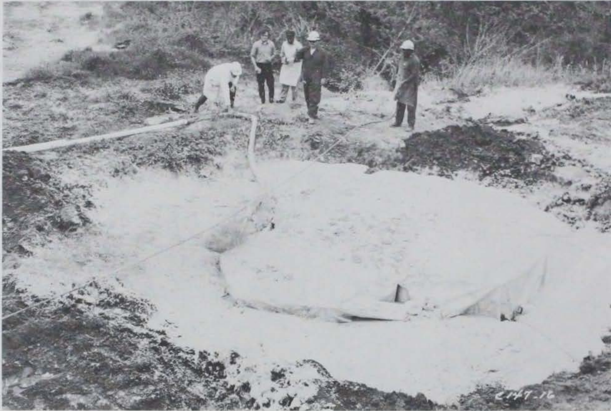
Figure 5.19 Completed sealing of module system.
