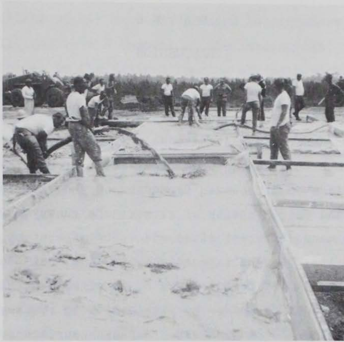
Figure 5.69 Placement of neat slurry capping material.
