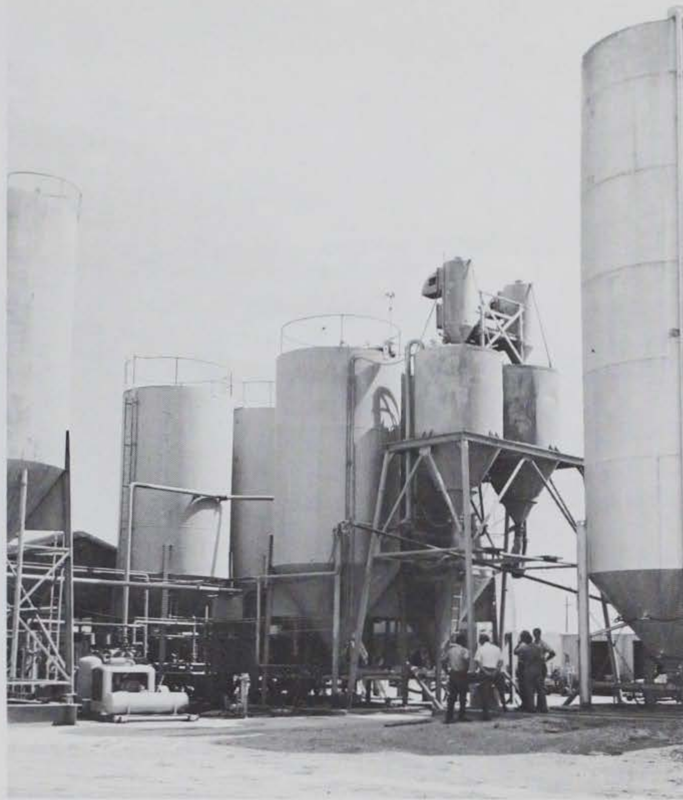
Figure 4.1 Cement storage silos.
