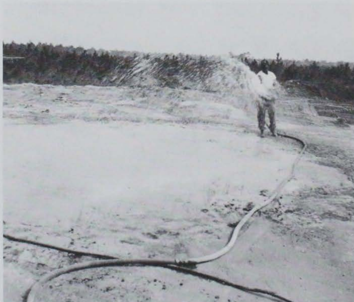
Figure 5.56 Water-curing of repair surface.
