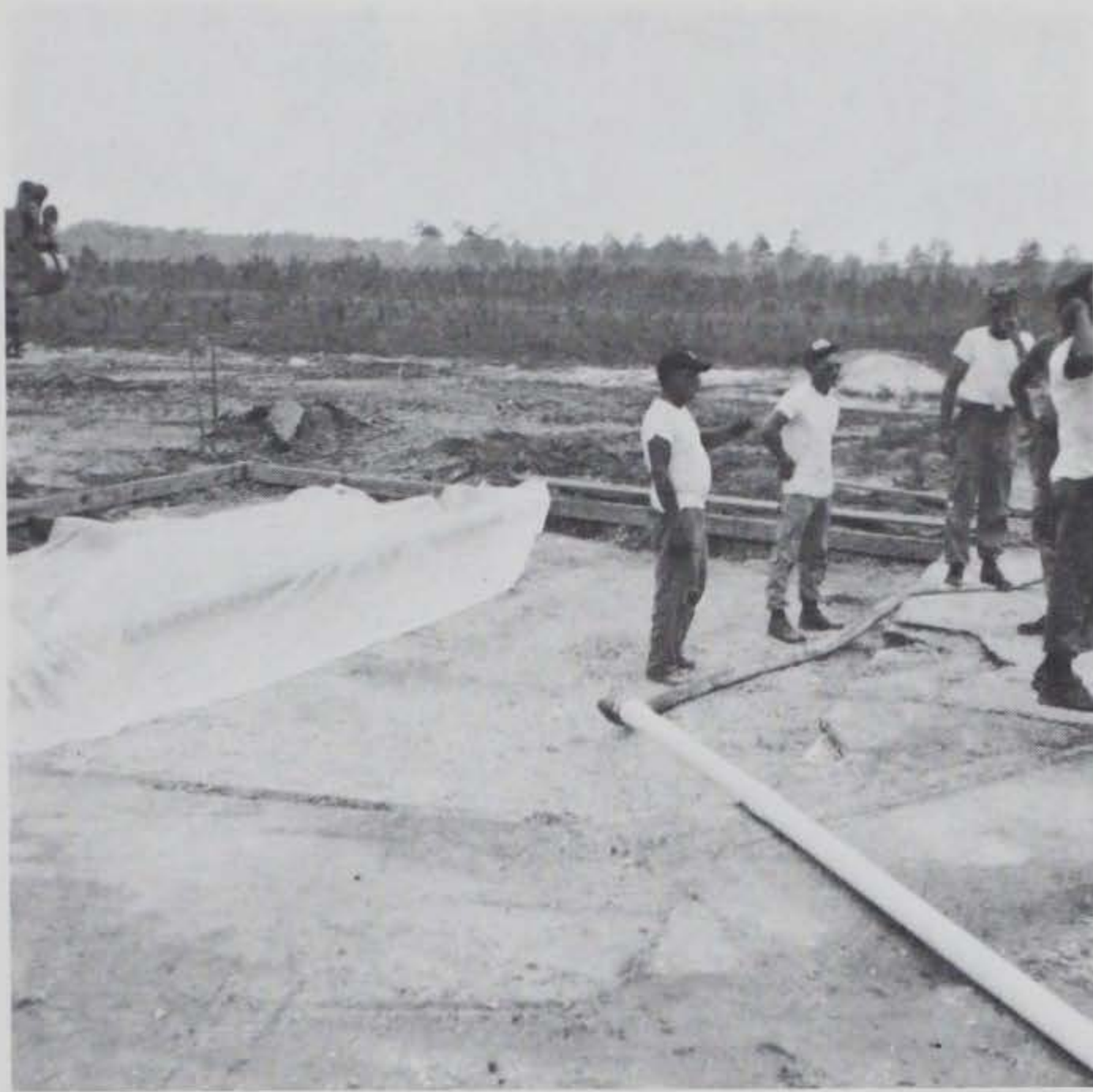
Figure 5.45 Finished surface of base course.
