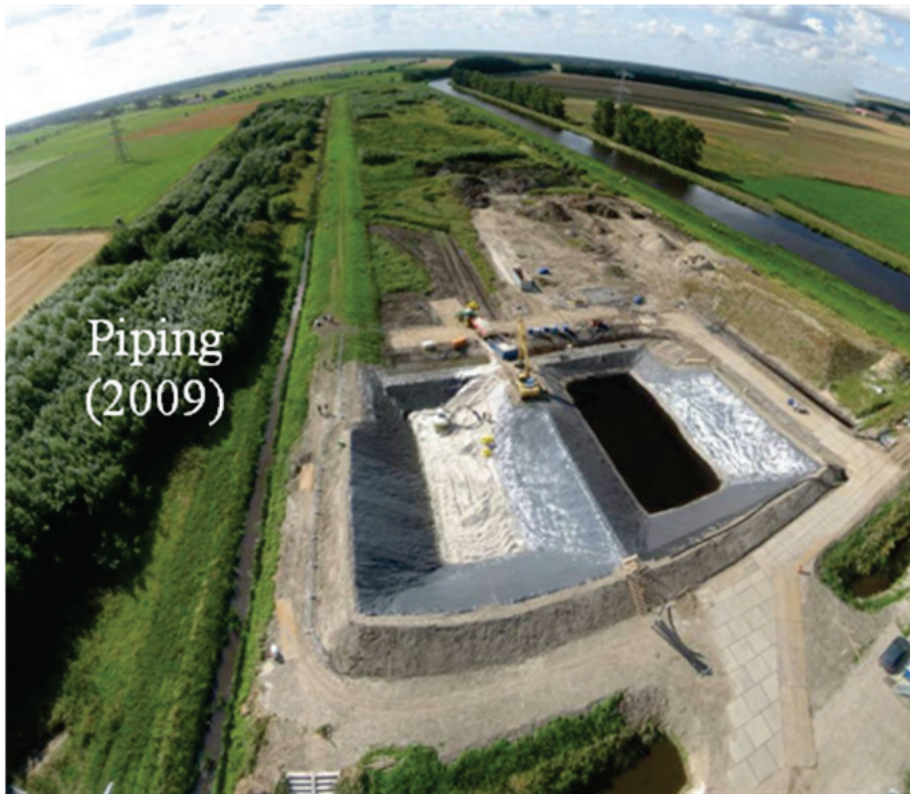
Figure 5-71. Aerial view of IJkdijk test facility and the types of levee failure experiments conducted at this site (Koelewijn 2009, 2012).
