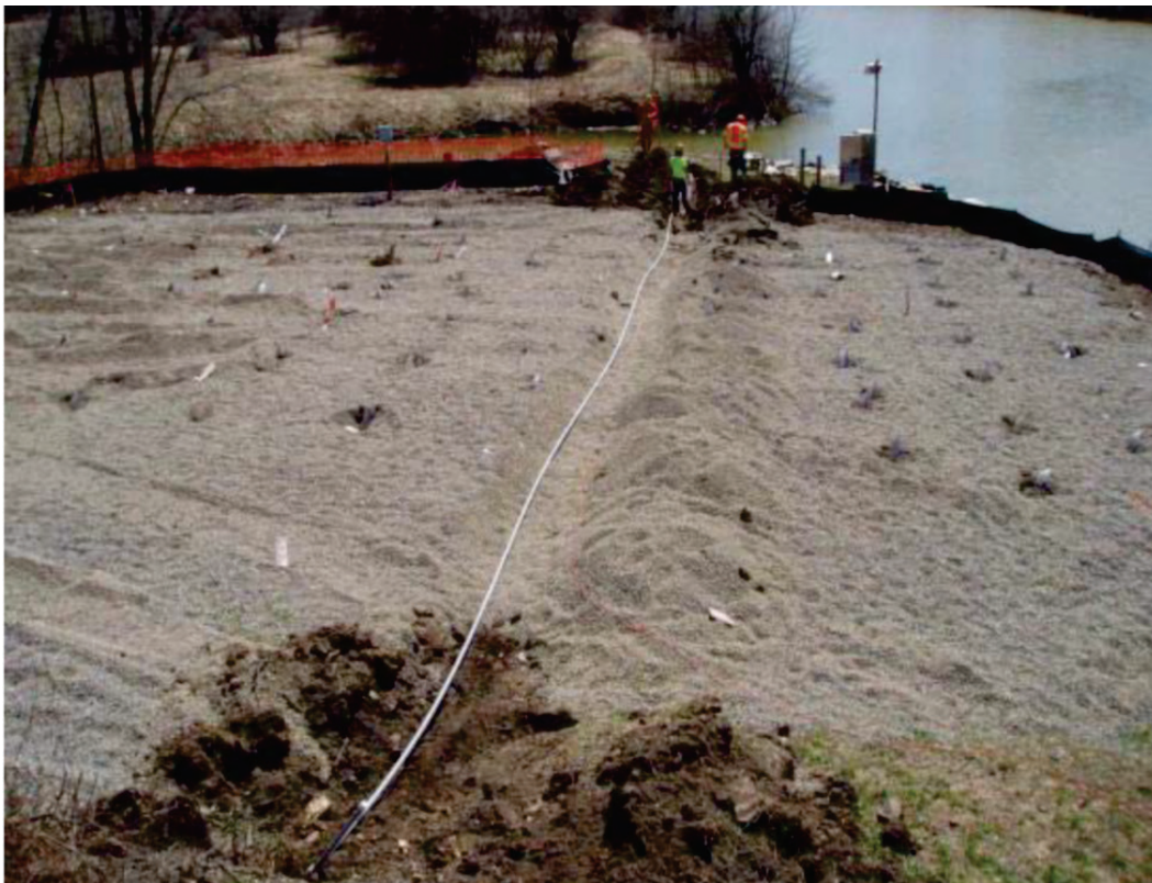
Figure 5-25. SAA/MEMS inclinometer string installation over a wick drain field (Barendse 2012).
