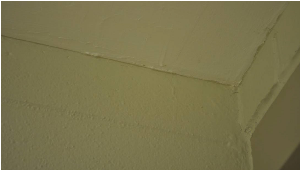
Figure 35. Room 9 with unknown coating in the washroom and on the block walls, after 12 months.
