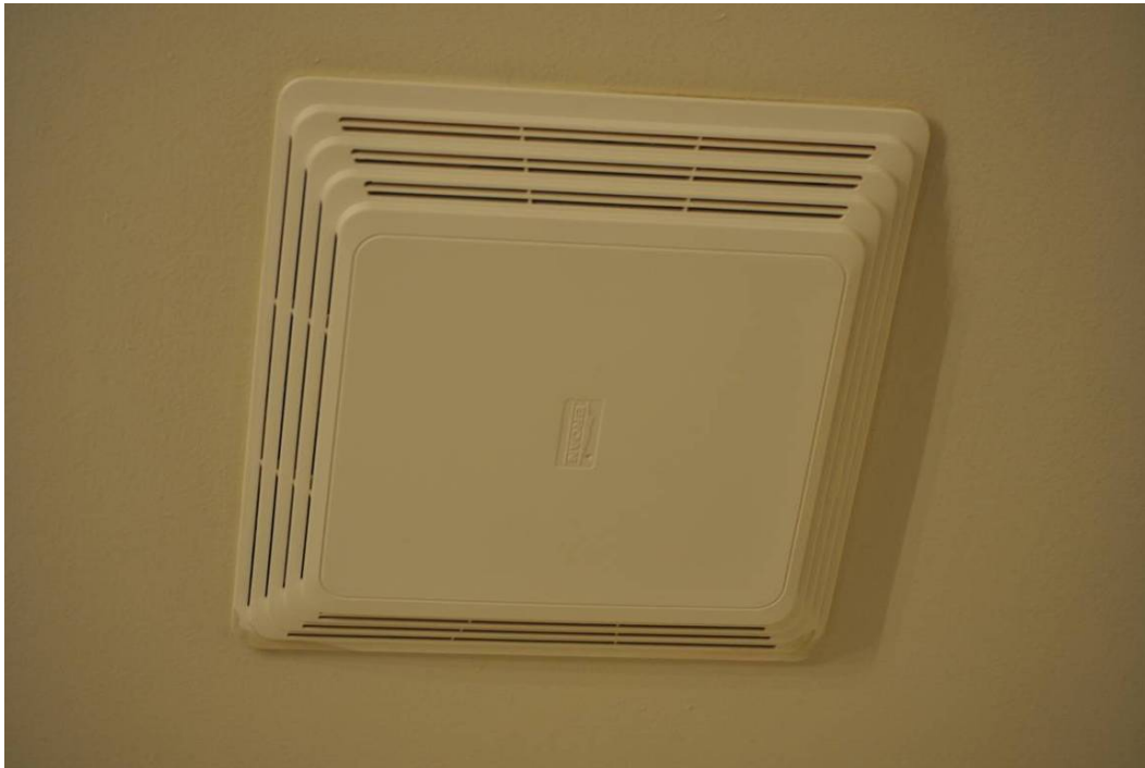
Figure 29. Ceiling vent in the washroom next to Room 14 after 8 months.
