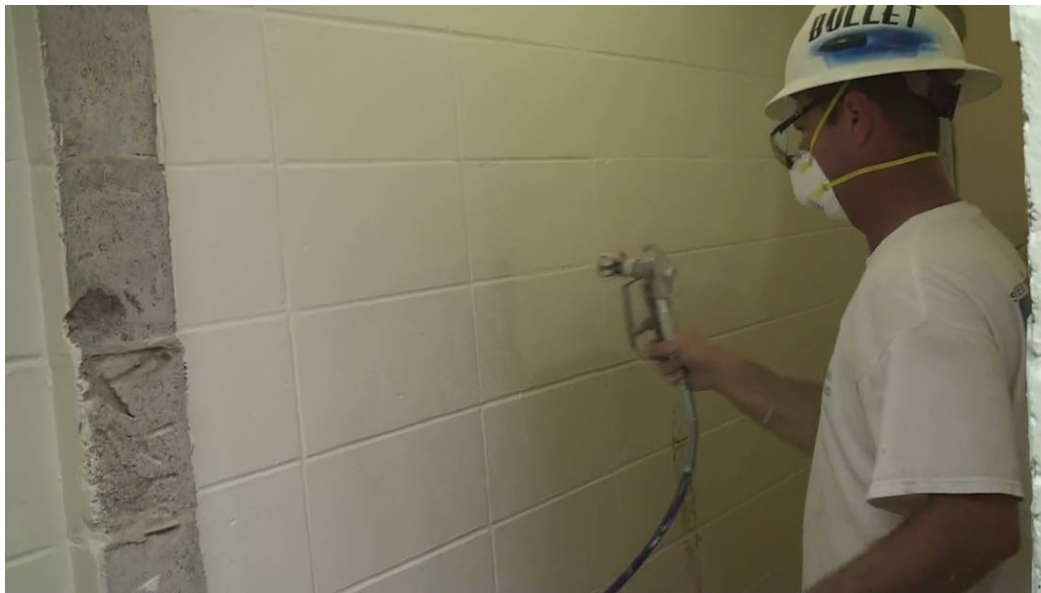
Figure 7. Coating application using conventional airless sprayer for Caliwel and Foster coatings.
