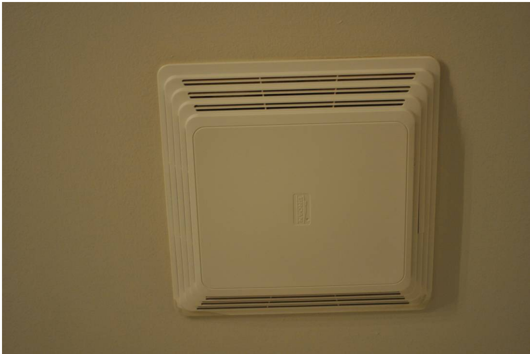
Figure 40. Ceiling vent in the washroom next to Room 14 after 12 months.
