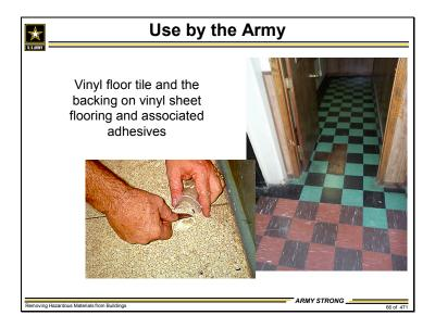
The rule of thumb for considering asbestos content in vinyl floor tile is that smaller tiles (e.g., 9 inch) are likely candidates for asbestos content. Larger tiles (e.g., 12 inch) are unlikely to contain asbestos.
