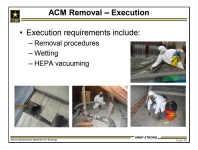
Ideally, all work surfaces are kept wet to limit the fibers becoming airborne. Debris is collected with a High Efficiency Particulate Air (HEPA) vacuum. The filter is fine enough that it catches all material of concern.
