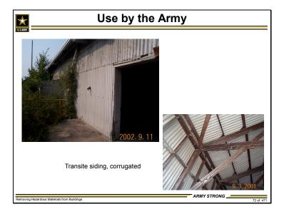
Corrugated transite siding was commonly used on warehouses or other large industrial buildings. It comes in 4 x 8 sheets and was used as both roofing and siding.
