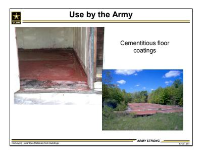
Cementitious floor coating was employed as a durable, fireproof, non-sparking coating in industrial buildings. It is often red-orange in color and can be placed over wood or concrete subflooring. It is also sometimes called "oxy-chloride" flooring, and it contains magnesium oxide, sawdust, asbestos, and fine aggregates.
