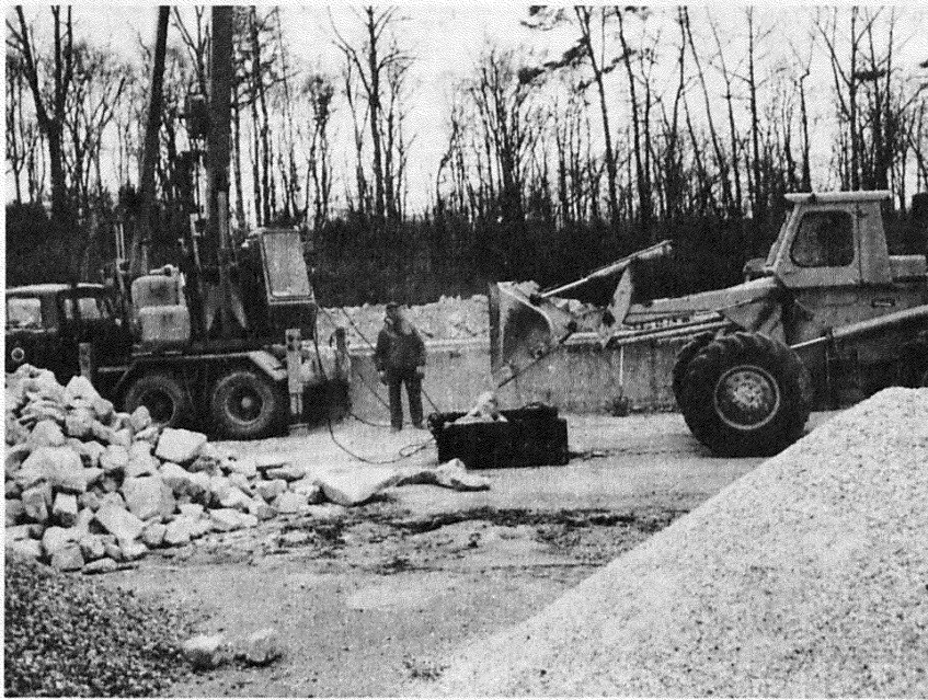
Figure 5. End loader filling skip with riprap.
