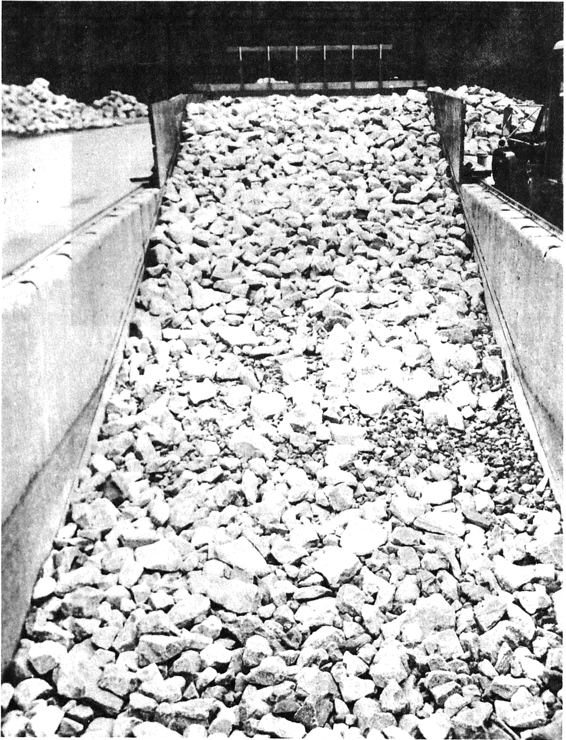
Figure 8. Riprap at failure, tank dry.
