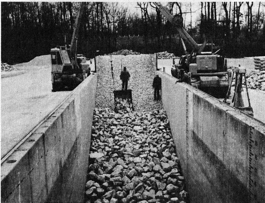
Figure 6. Dumping riprap from skip onto filter layer.
