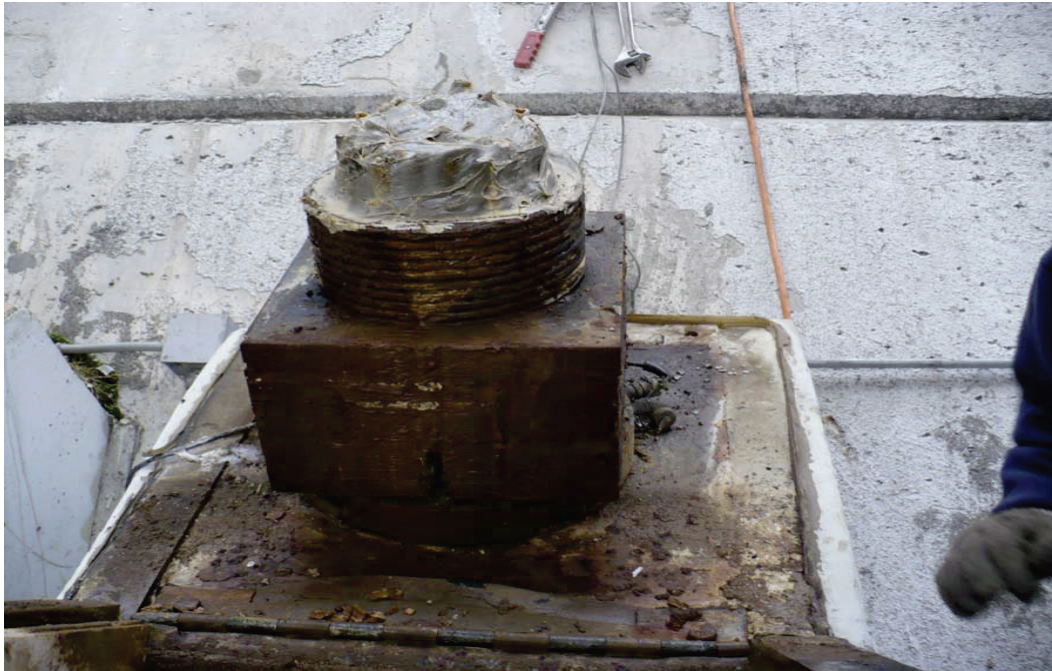
Figure 2.11. Freshly greased anchor head (Cornforth Consultants 2009).
