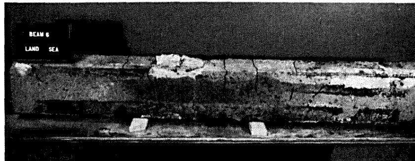
Photo 10. "As received" condition of beam 6 looking east
