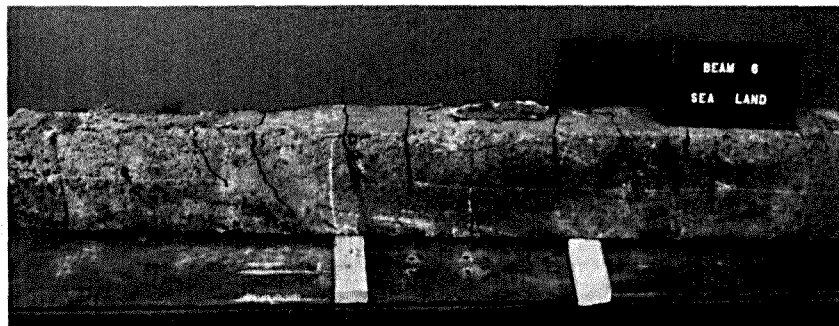
Photo 9. "As received" condition of beam 6 looking west
