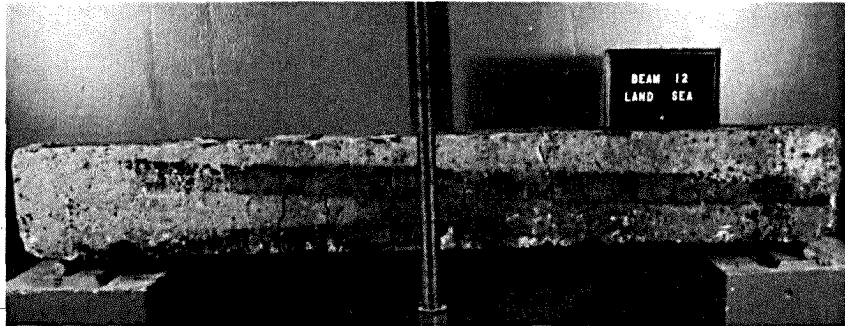
Photo 20. "As received" condition of beam 12 looking east
