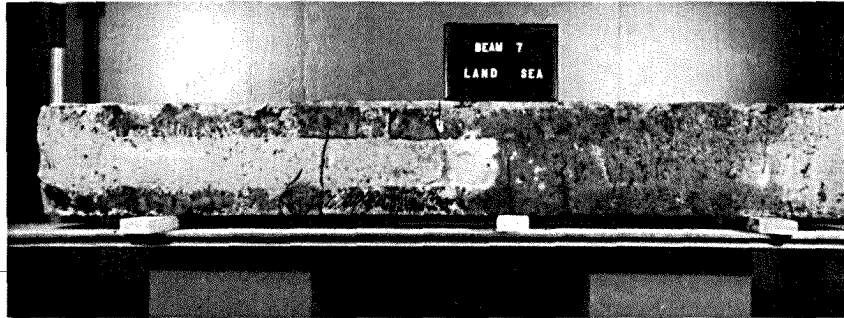
Photo 12. "As received" condition of beam 7 looking east
