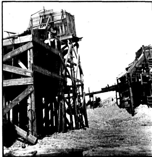
Juban Gravel Co., Inc., Minden, La. The plant is located about 1 mile west of Sibley, La., and operates in Recent sand-gravel aggregate. The view is of the washing plant where that portion on the right of photograph separates sand which goes to stock pile via flume, all gravel sliding down screen to the ground surface. This is picked up with dragline and placed in hopper (upper left) where it is washed and screened and enters bins for loading trucks.
