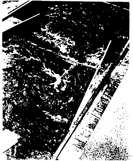
Fig. 4. Pool elev, 800 dischg, 3170 cfs; TW elev, 694.6
