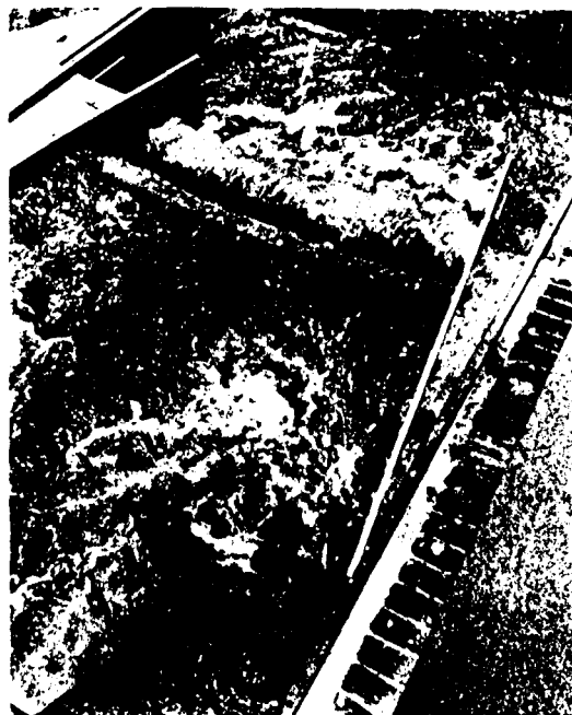
Fig. 10. Pool elev, 800 dischg, 6340 cfs; TW elev 694.6
