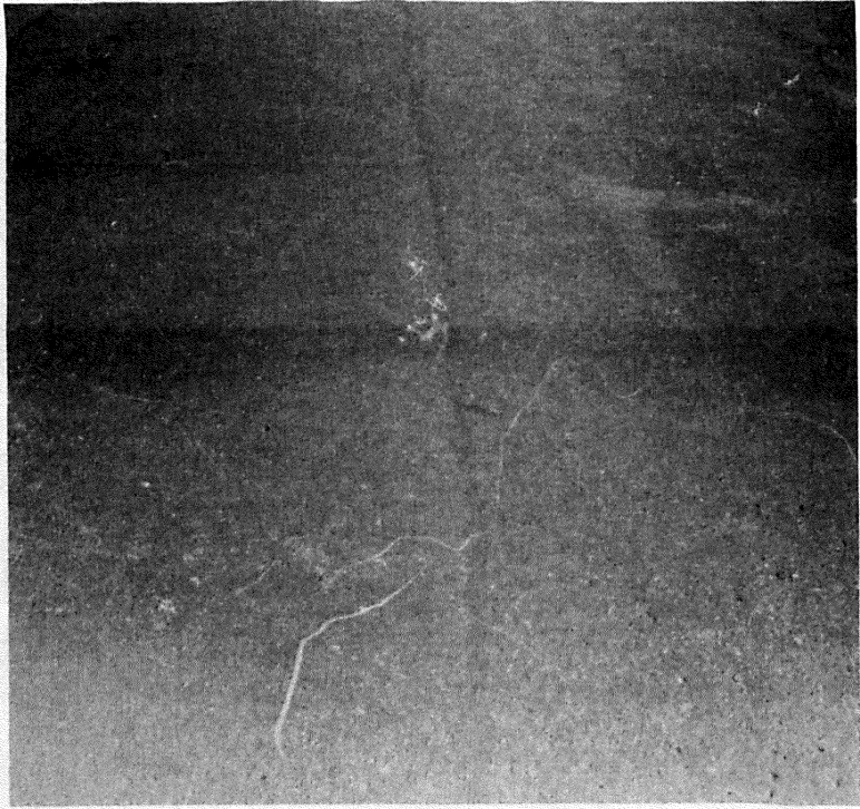
Photo 7. Close-up of parking and maintenance apron. Tar rejuvenator was applied in 1971
