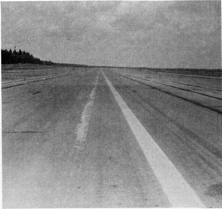
Photo 3. Extension to taxiway A
