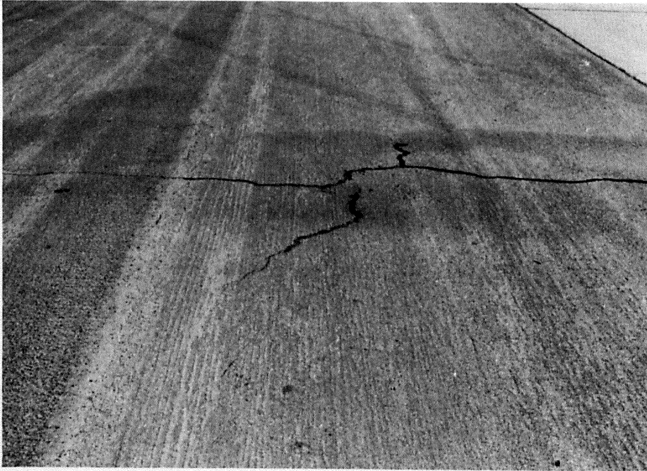
Photo 1. AC portion of runway near north end, east side
