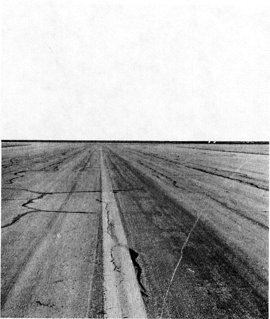
Photo 7. General view of taxiway 4
