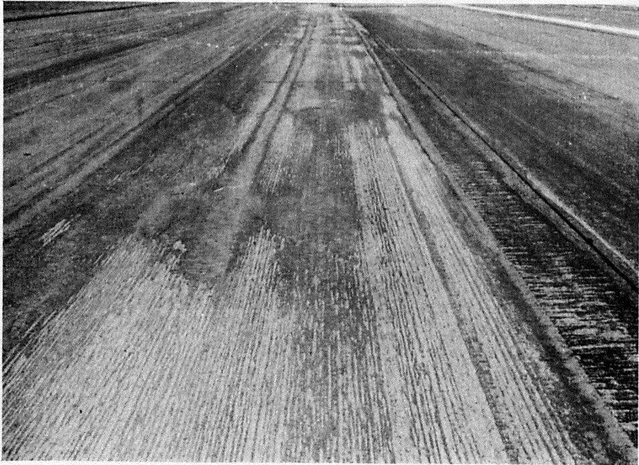
Photo 3. AC portion of runway, 5000 ft from north end, east side
