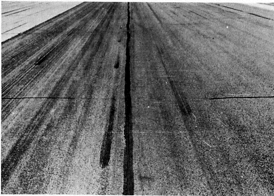
Photo 2. AC portion of runway, 5000 ft from north end, west side
