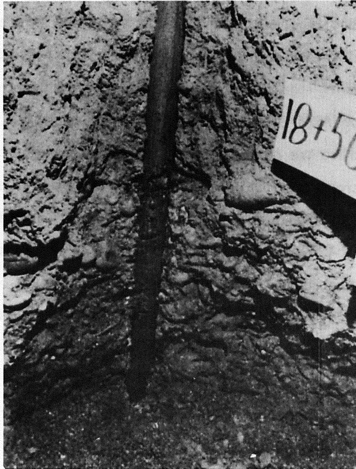
Figure 44. Cone Penetrometer Test Hole (CPT 24) Exposed in Sidewall of Trench at Station 18+50.
