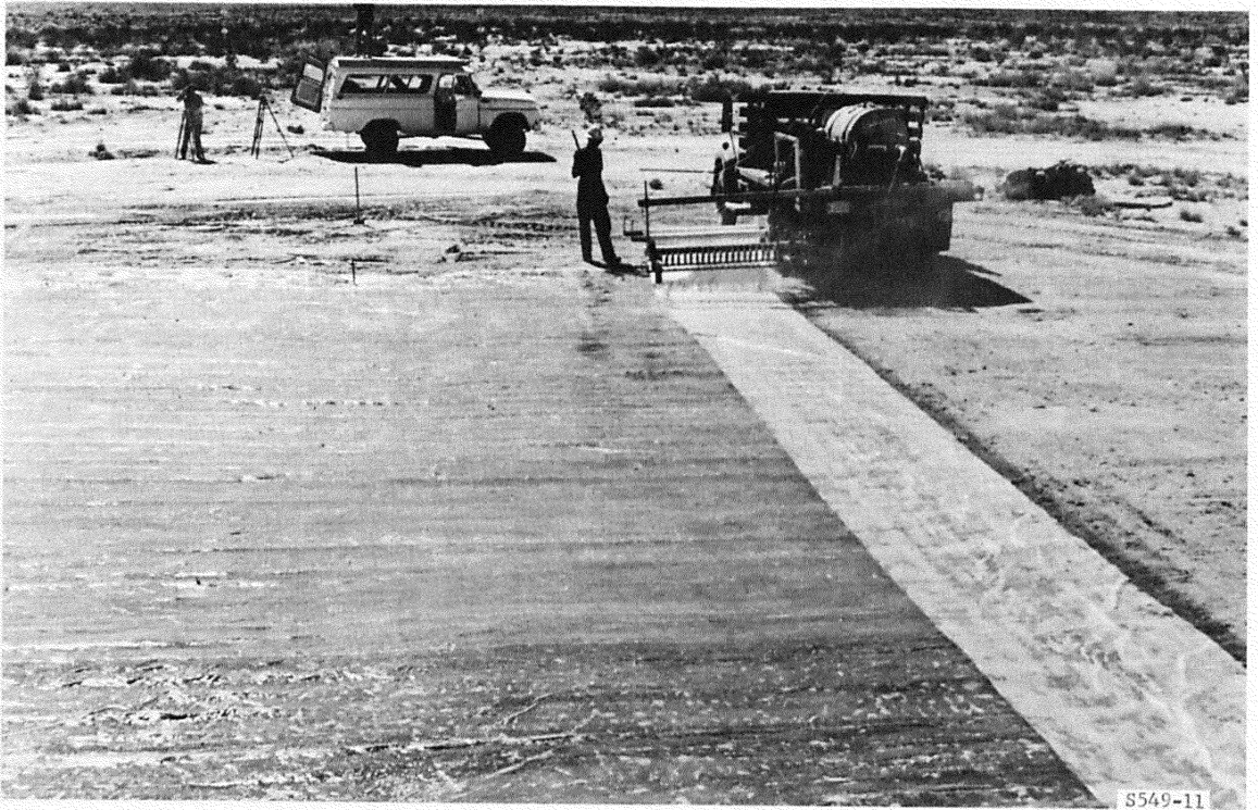
Photograph 27. Placing border of glass fiber and resin
