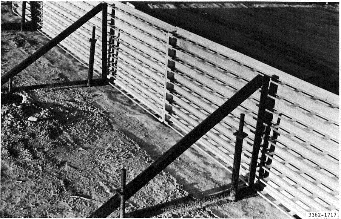
Photograph 19. Anchorage of vertical fence
