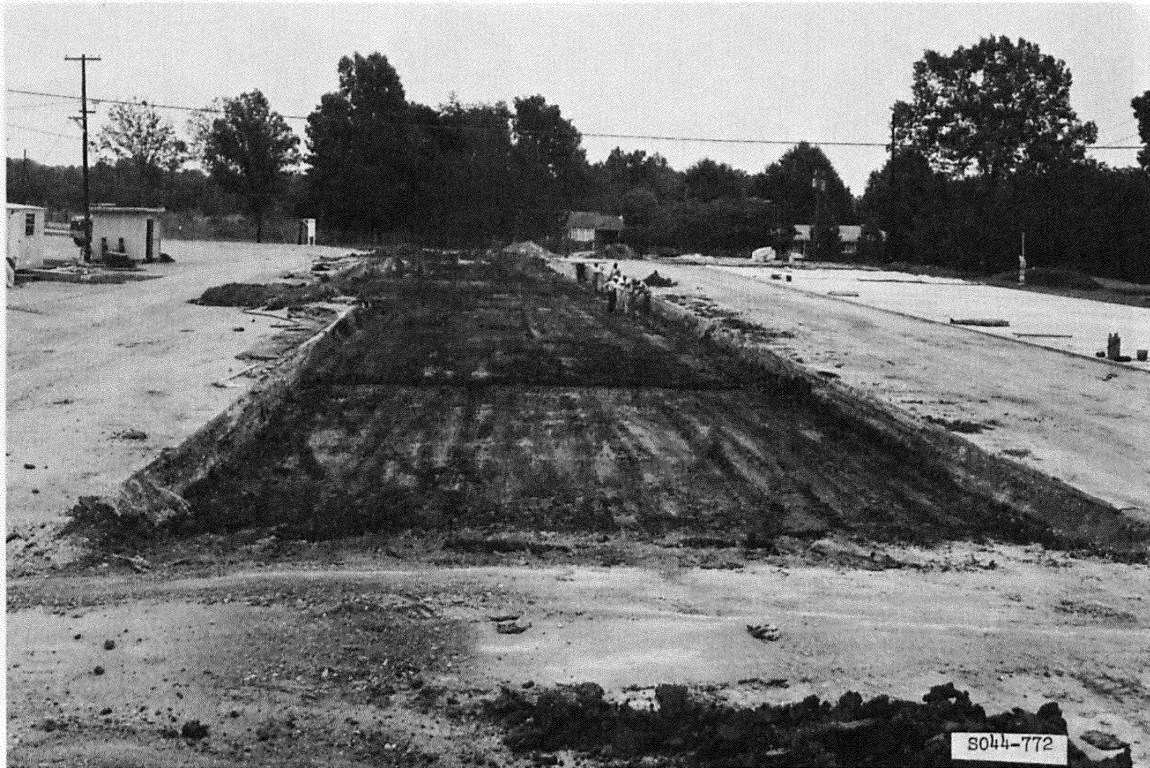
Figure 35. Completed subgrade of the flexible pavement test section
