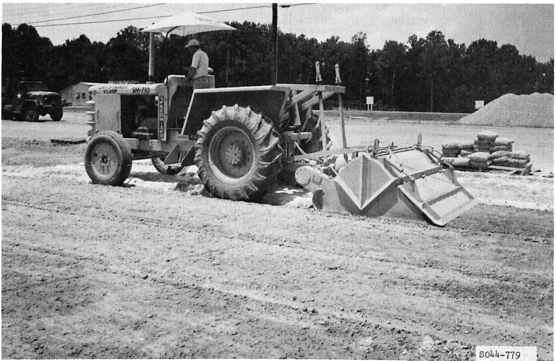
Figure 37. In-place mixing of treated soil with pulvimixer
