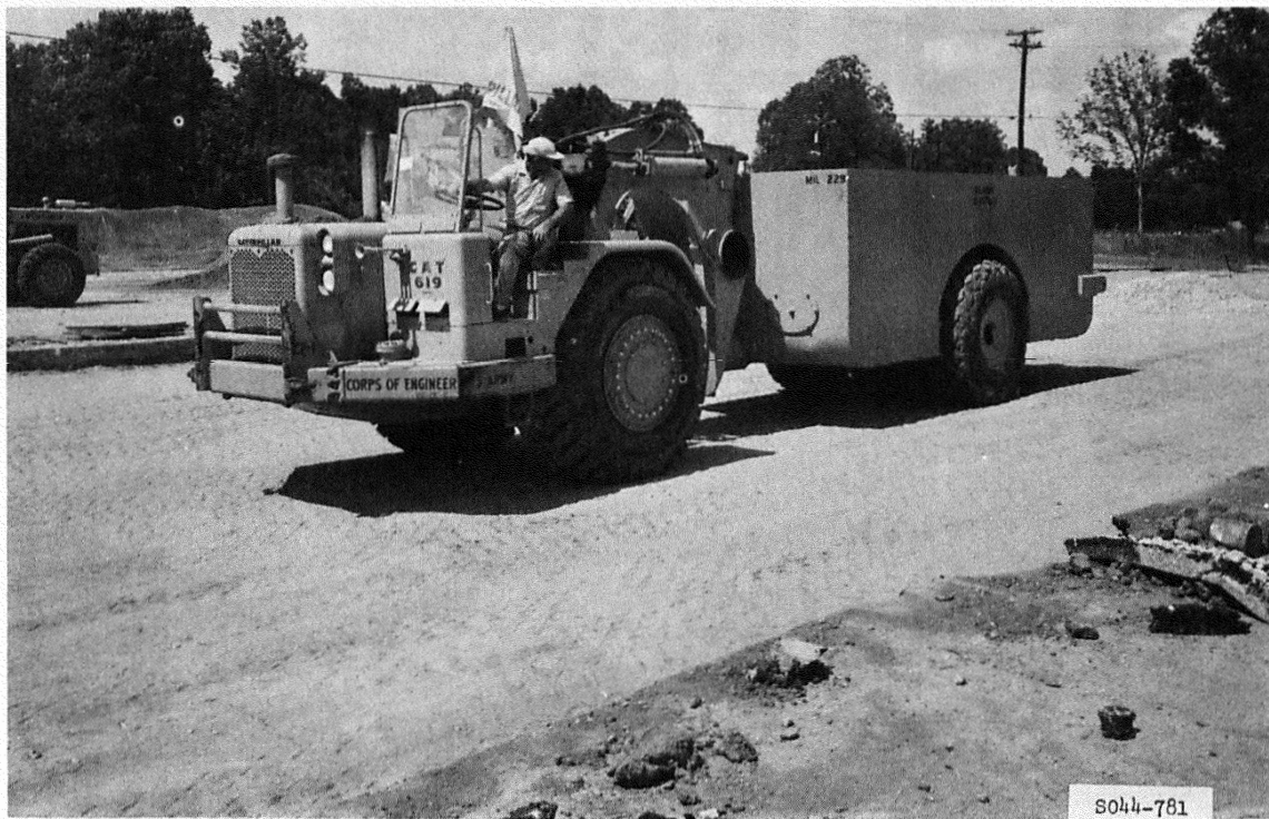
Figure 25. Compaction with the 50-ton pneumatic-tired roller
