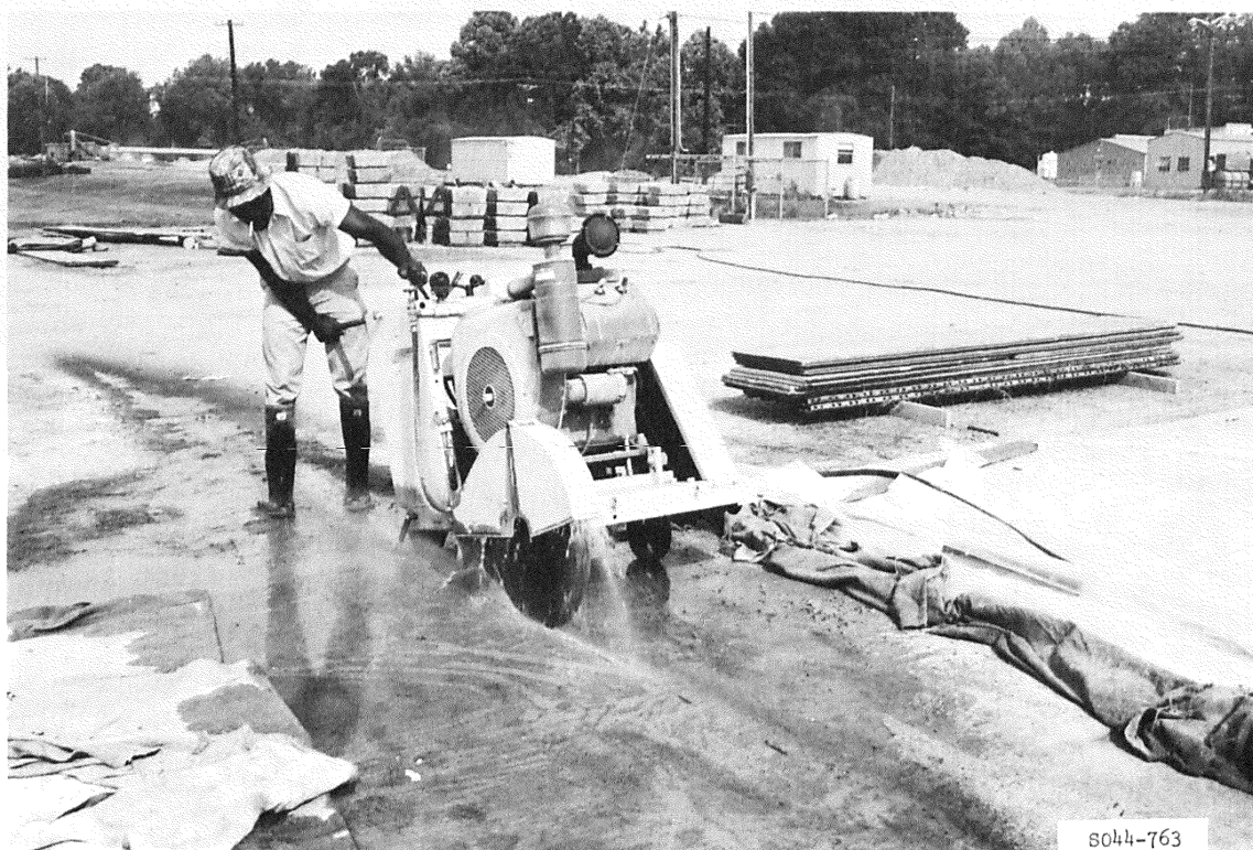
Figure 34. Joint sawing operations in the rigid pavement test section
