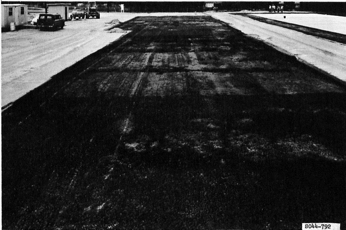
Figure 39. Primed base courses prior to paving flexible pavement test section
