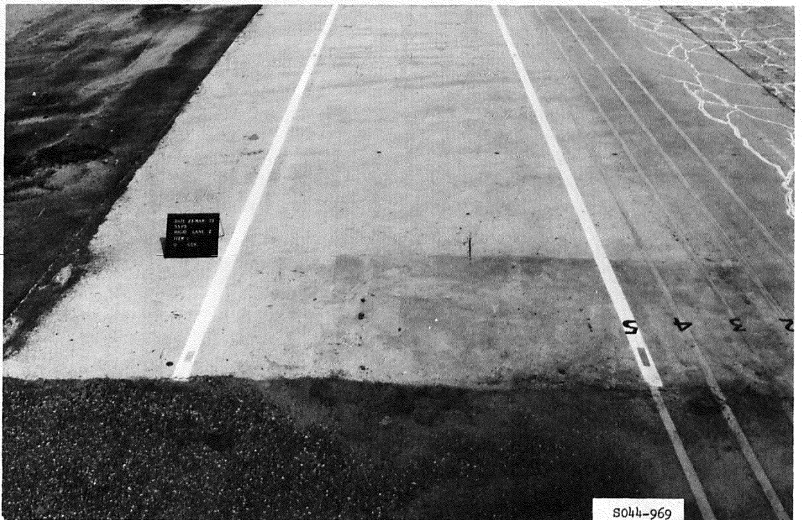
Figure A31. Item 1, lane 2, rigid pavement test section, prior to traffic
