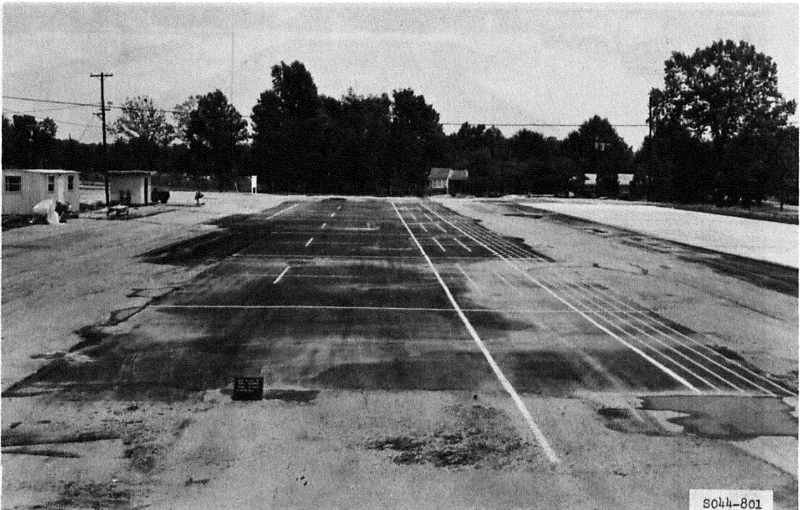
Figure 41. Overall view of completed flexible pavement test section
