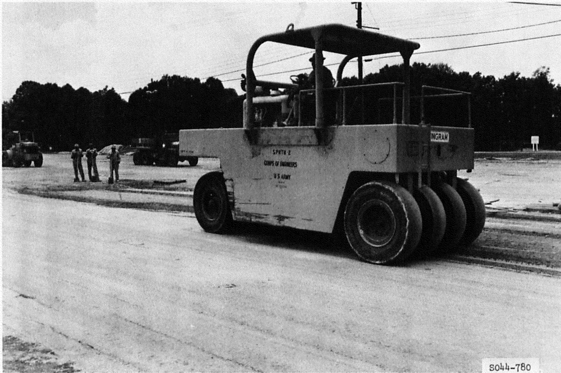
Figure 24. Compaction with the 30-ton self-propelled pneumatic-tired roller
