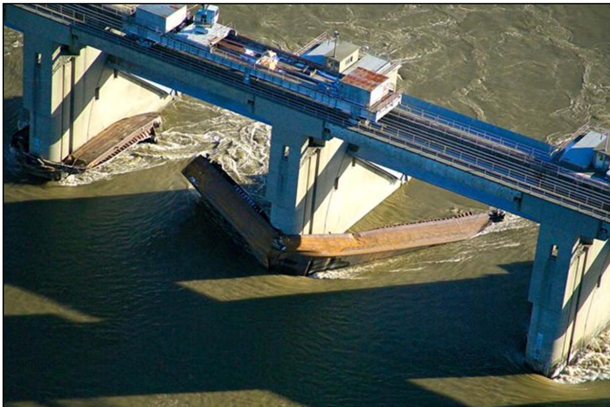
Figure 1. Barge accident, Belleville Locks and Dam, Ohio River, January 2005.
