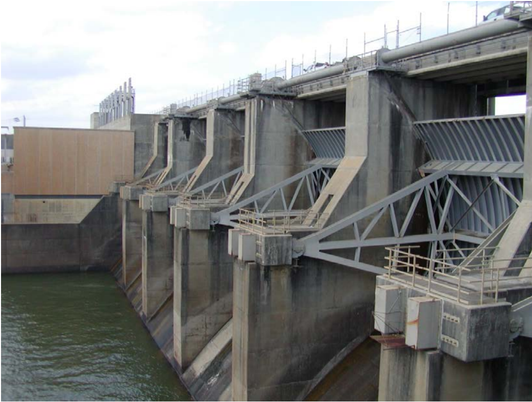
Figure 2. Typical tainter gates and trunnions.
