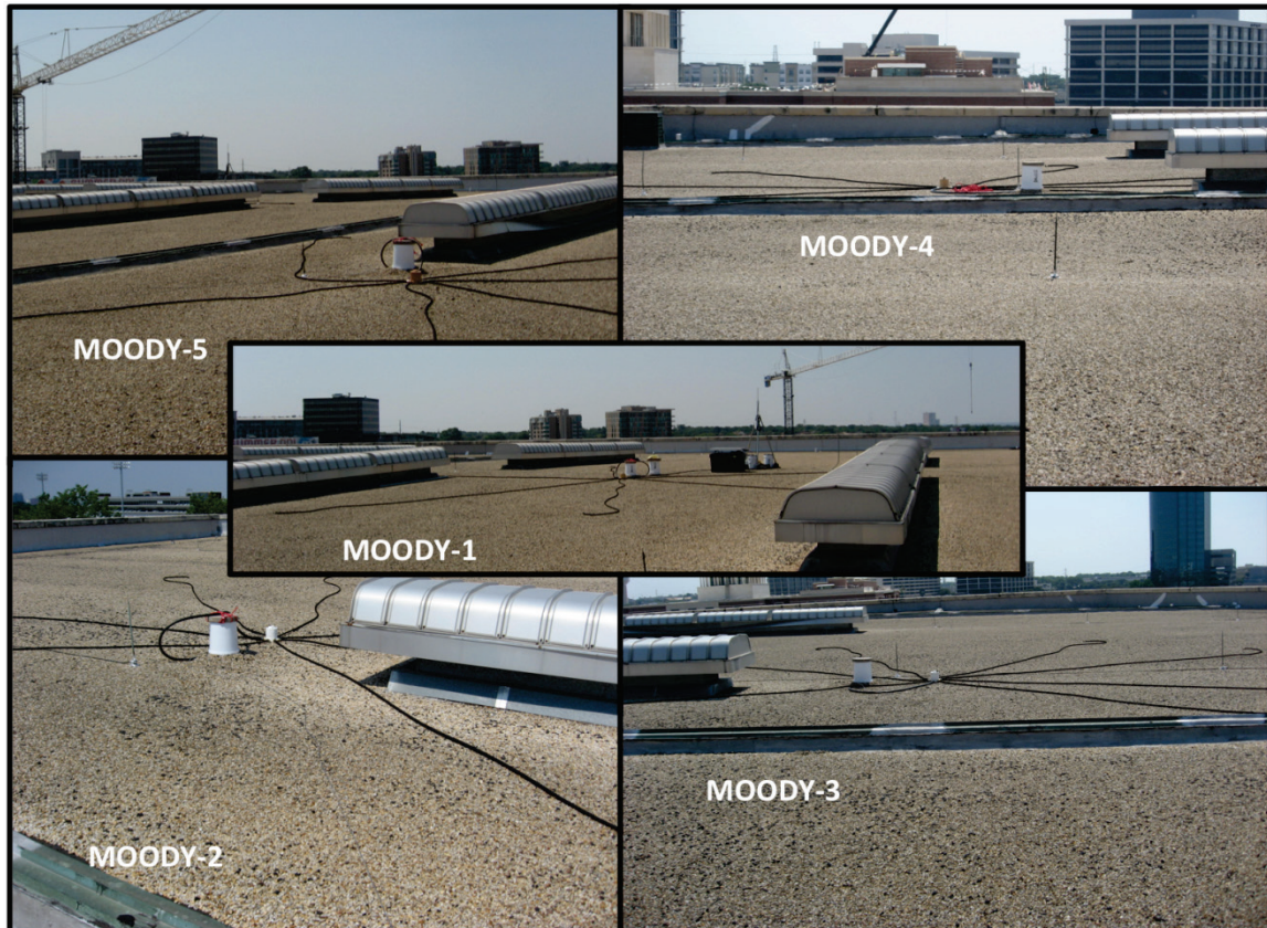
Figure 3. Photograph of Moody rooftop array. Highlights include the roof infrastructure, roof vents and the raised edge, which could create a complex noise environment for the array.
