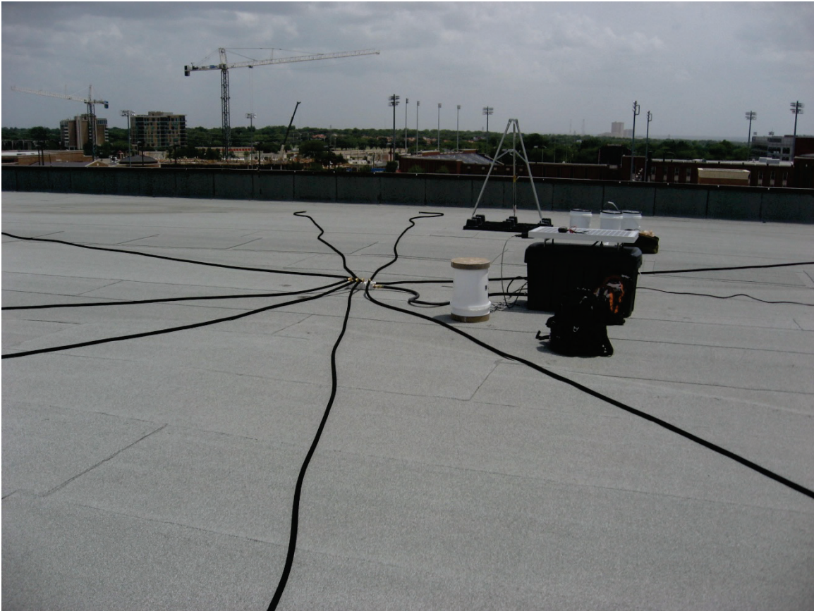
Figure A9. Multi-rooftop array Collins Hall.
