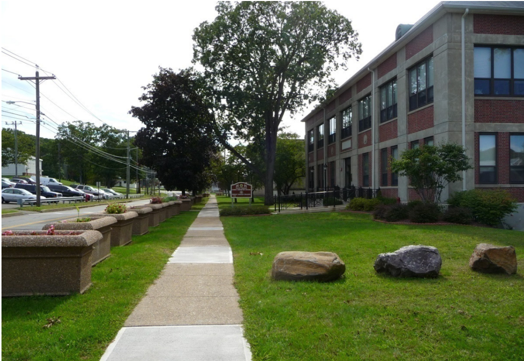
Figure 106. Force protection planters in front of Building 172 (ERDC-CERL, 2012).
