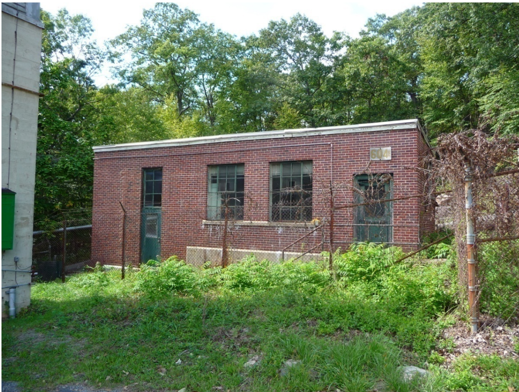
Figure 192. Southeast elevation of Building 604E (ERDC-CERL, 2012).
