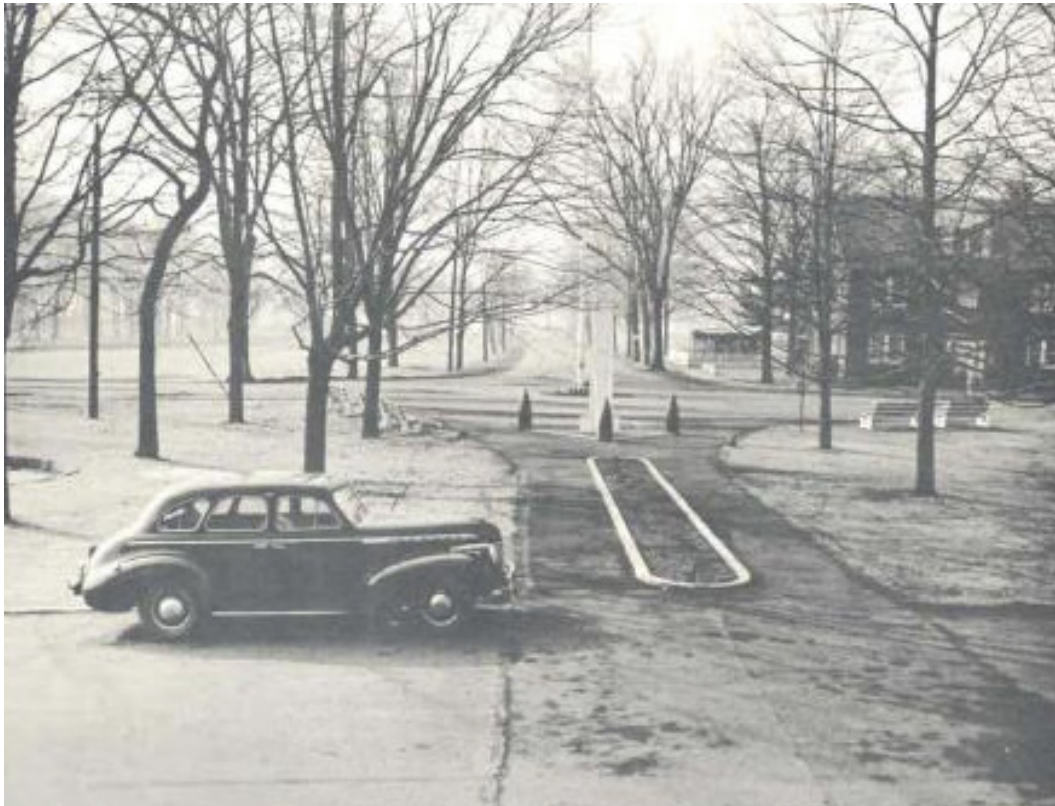
Figure 120. View from Building 151 of intersection of Farley Avenue and Parker Road, ca. 1958 (PICA Cultural Resources Office).
