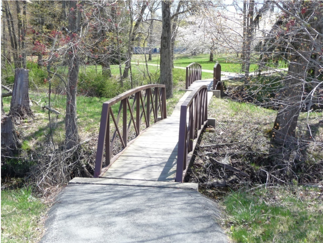
Figure 44. Bridge connecting Buildings 151 to 162 (ERDC-CERL, 2012).
