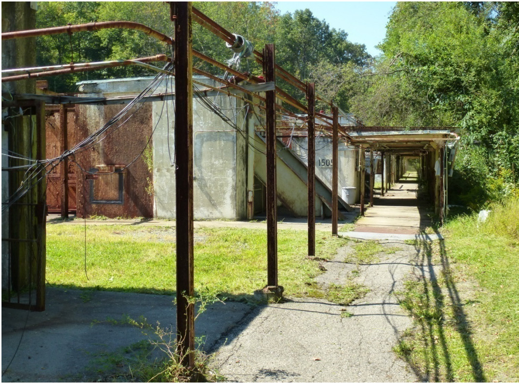
Figure 229. Concrete walkways connect the test stands in the Testing Area of the historic district (ERDC-CERL, 2102).
