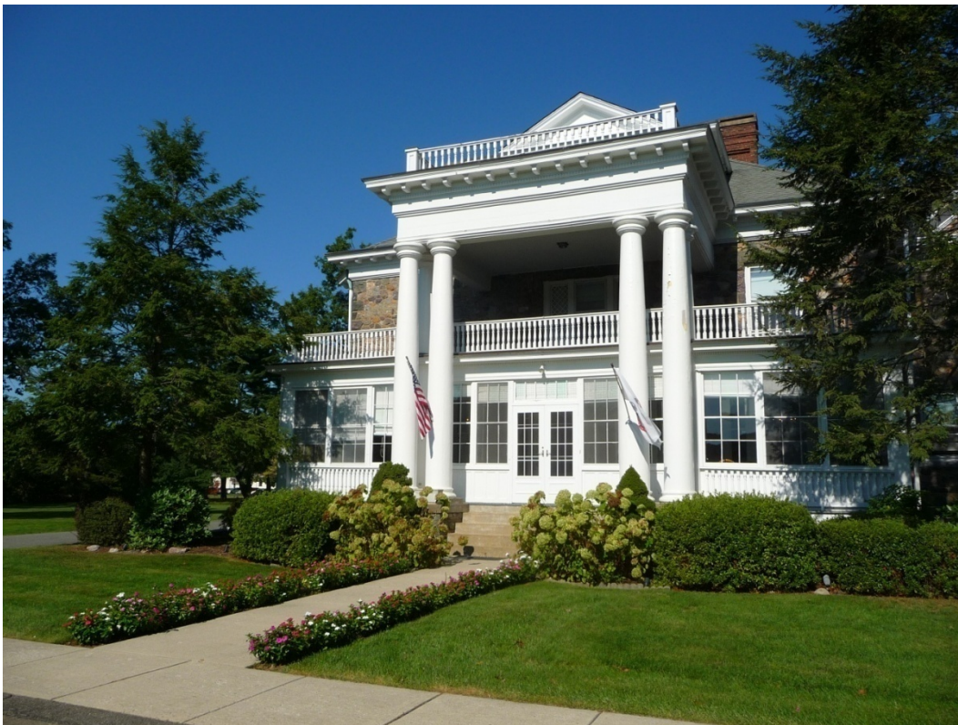
Figure 52. East elevation of Building 112 (ERDC-CERL, 2012).
