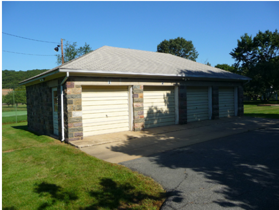
Building 123 – Garage (1939) (ERDC-CERL, 2012).
