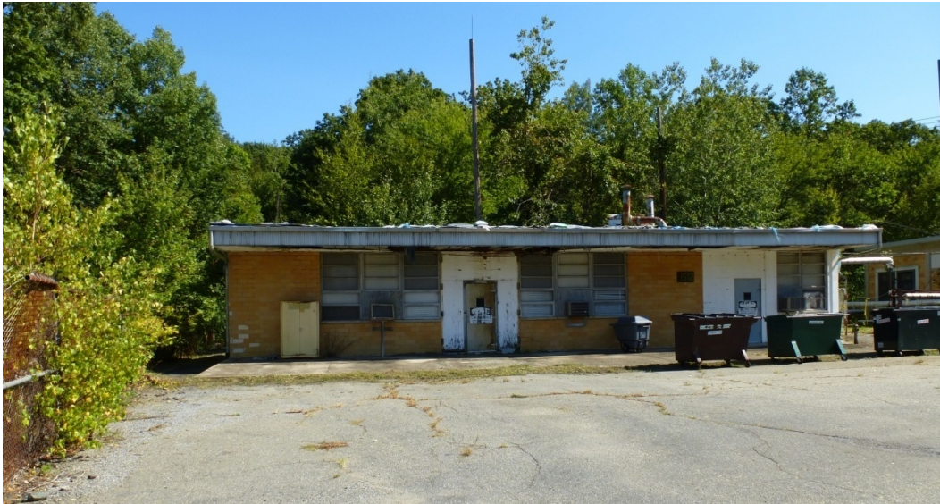
Figure 256. Building 1512, Physics Laboratory northwest elevation (ERDC-CERL, 2012).
