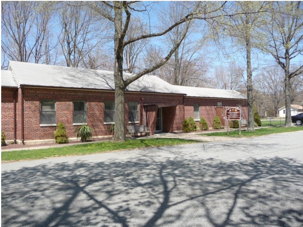
Figure 72. East elevation of Building 176 (ERDC-CERL, 2013).
