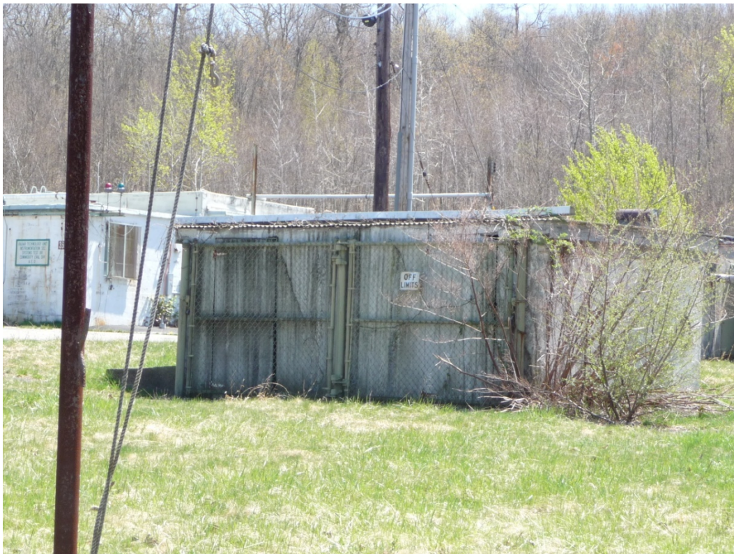
Figure 294. Building 3602, NARTS Liquid Propellant Storage (ERDC-CERL, 2013).
