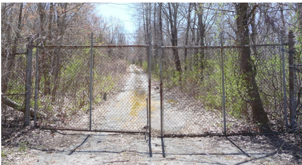
Figure 312. Chain-link fencing and gate at the entrance to NARTS Test Area E (ERDC-CERL, 2013).
