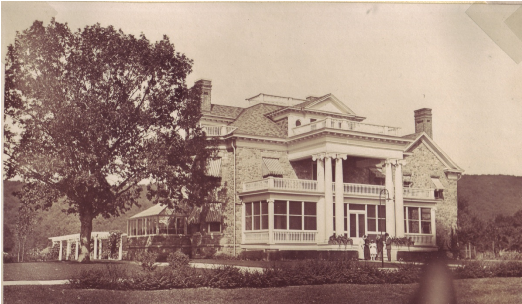
Figure 13. Historic photograph of Building 112, 1913 (PICA Cultural Resources Office).
