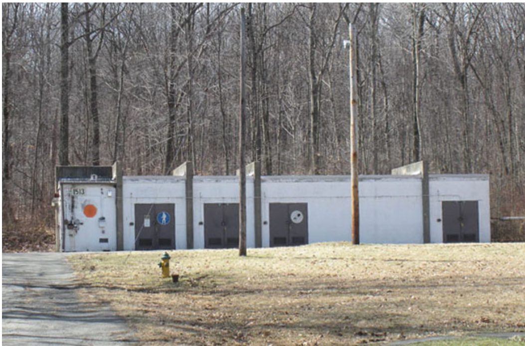
Figure 258. View south at Building 1513, General Purpose Magazine (PICA Cultural Resources Office, 2012).
