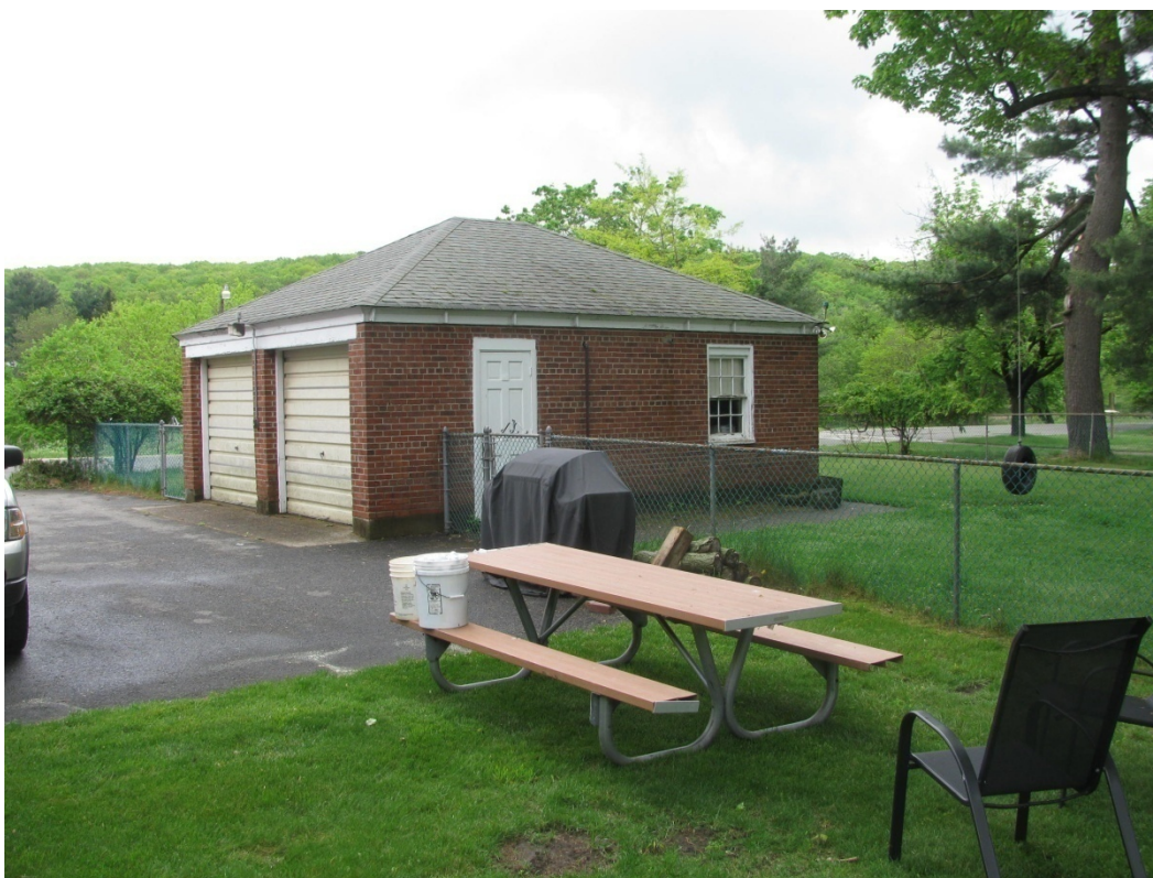
Figure 60. Northwest oblique of Building 115A (PICA Cultural Resources Office).
