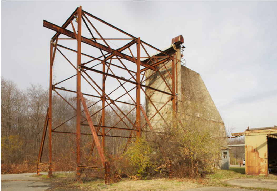
Figure 295. View west at Buildings 3603 (PICA Cultural Resources Office, 2010).
