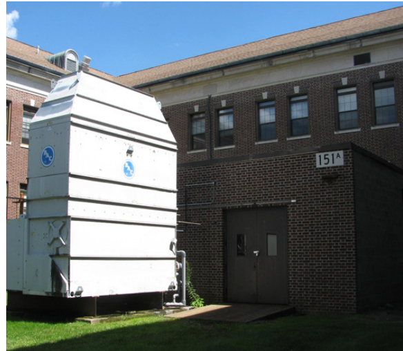
Building 151A – HVAC Building (1985) (PICA, 2011).
