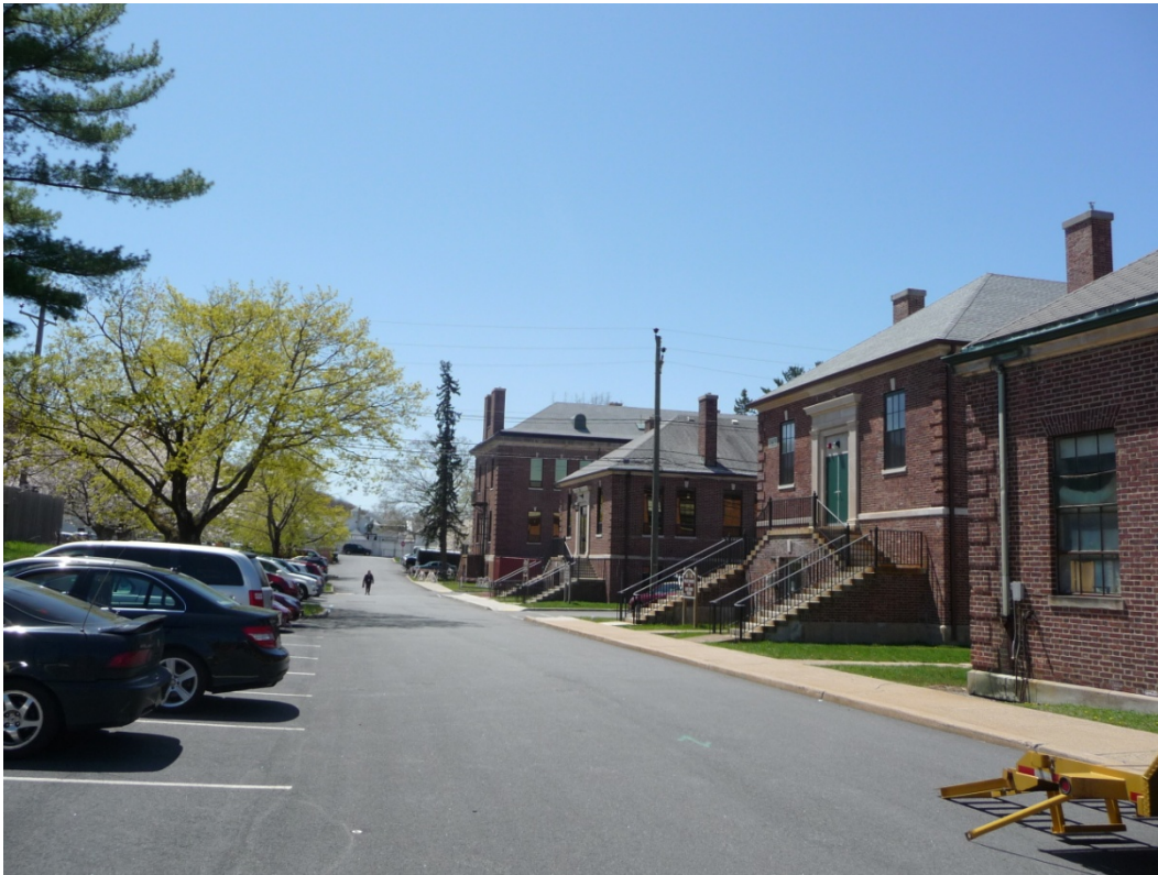
Figure 138. Looking south along Kibler Road in Chemistry Row (ERDC-CERL, 2013).
