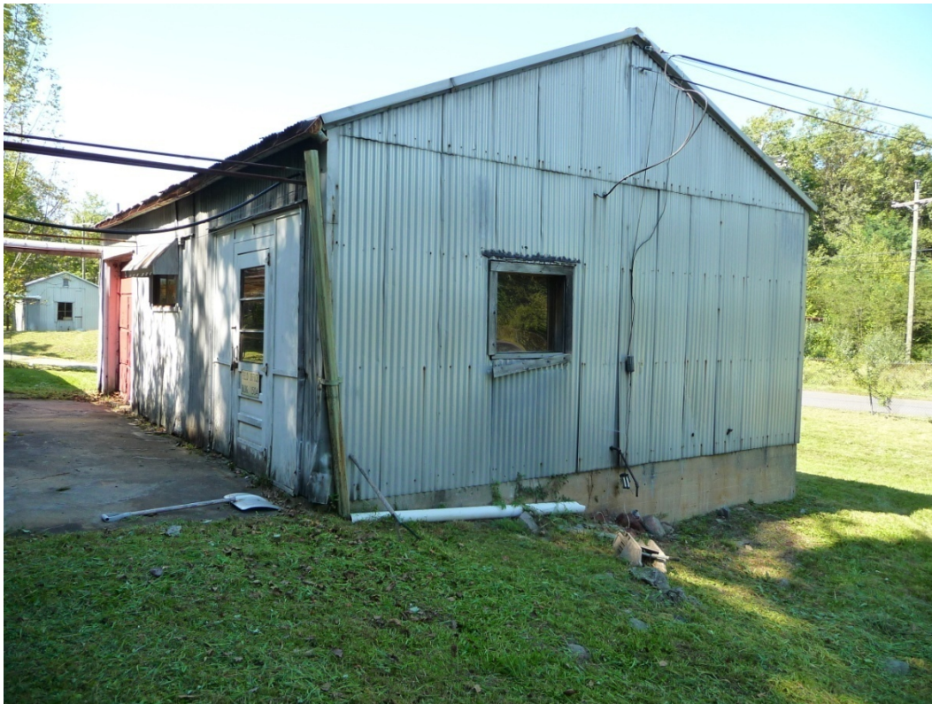
Figure 240. West elevation of Building 1504 (ERDC-CERL, 2013)).
