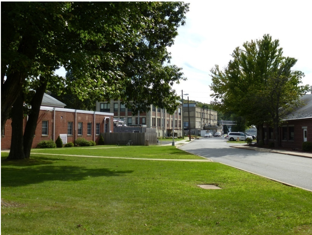
Figure 139. Looking south on 5 th Avenue in Chemistry Row area (ERDC-CERL, 2012).
