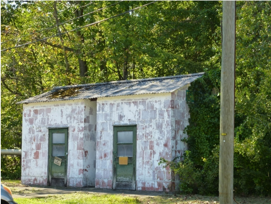
Figure 254. East elevation of Building 1510A, which was recently demolished (ERDC-CERL, 2012).
