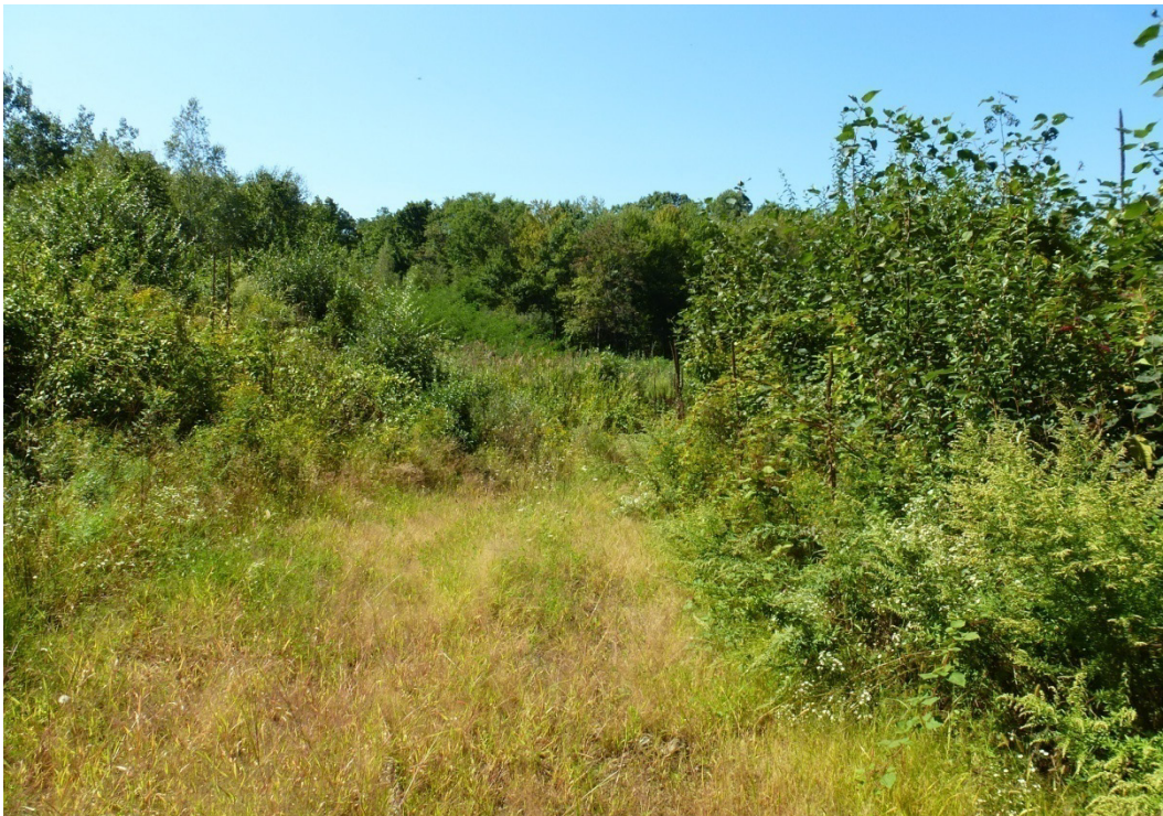
Figure 268. Overgrown vegetation on an earthen barricade (ERDC-CERL, 2012).
