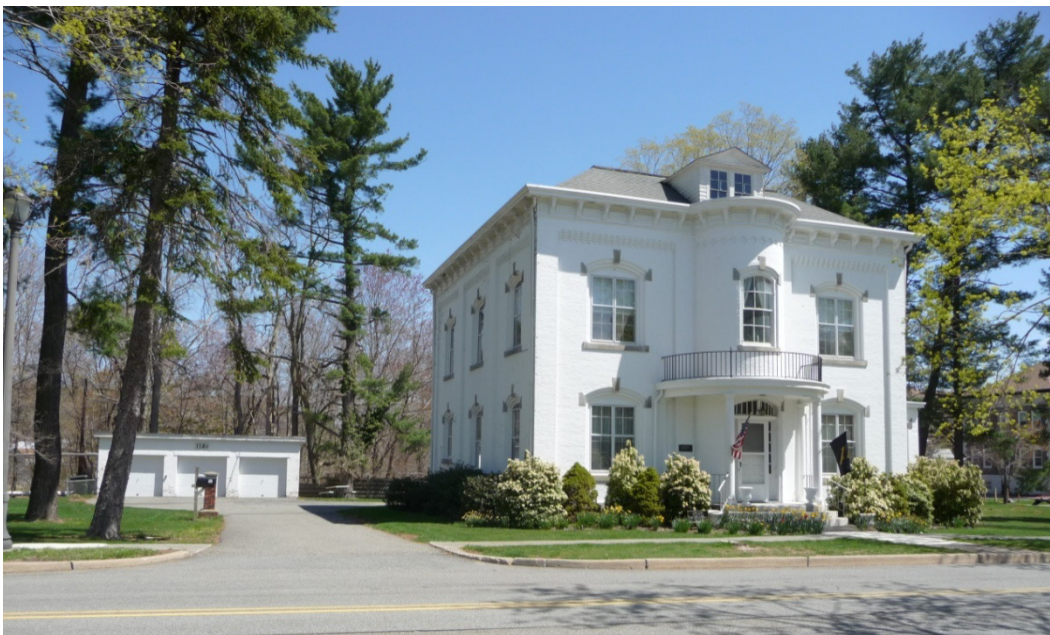
Figure 57. Southwest elevation of Building 114 (ERDC-CERL, 2013).
