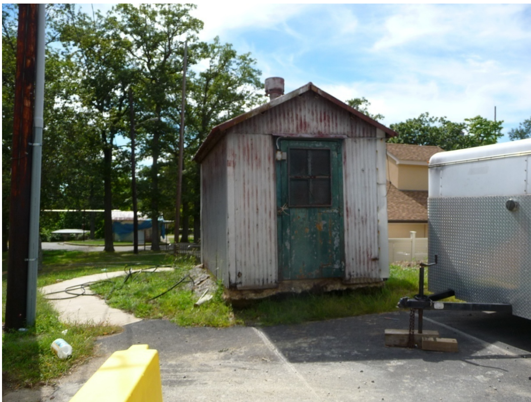
Figure 202. North elevation of Building 617F (ERDC-CERL, 2012).
