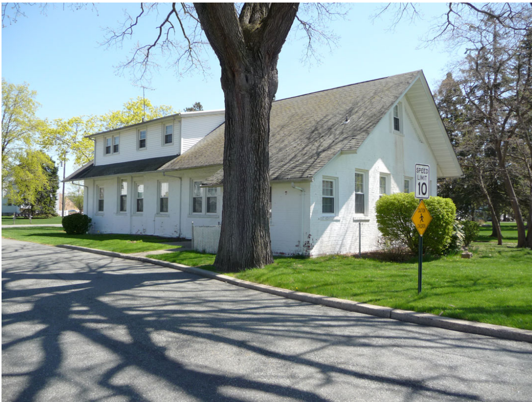
Figure 163. View of front and northwest facades of Building 108, former storehouse (ERDC-CERL, 2013).
