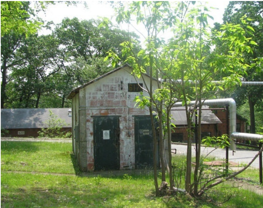
Figure 200. West elevation of Building 617A (PICA Cultural Resources Office).
