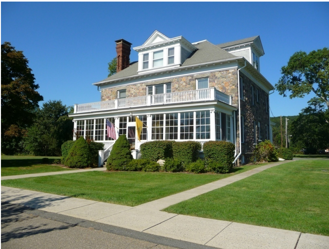
Figure 55. East elevation of Building 113 (ERDC-CERL, 2012).
