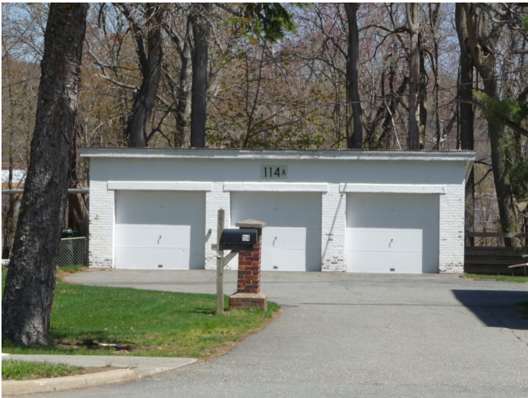
Figure 58. Southwest elevation of Building 114A (ERDC-CERL, 2013).
