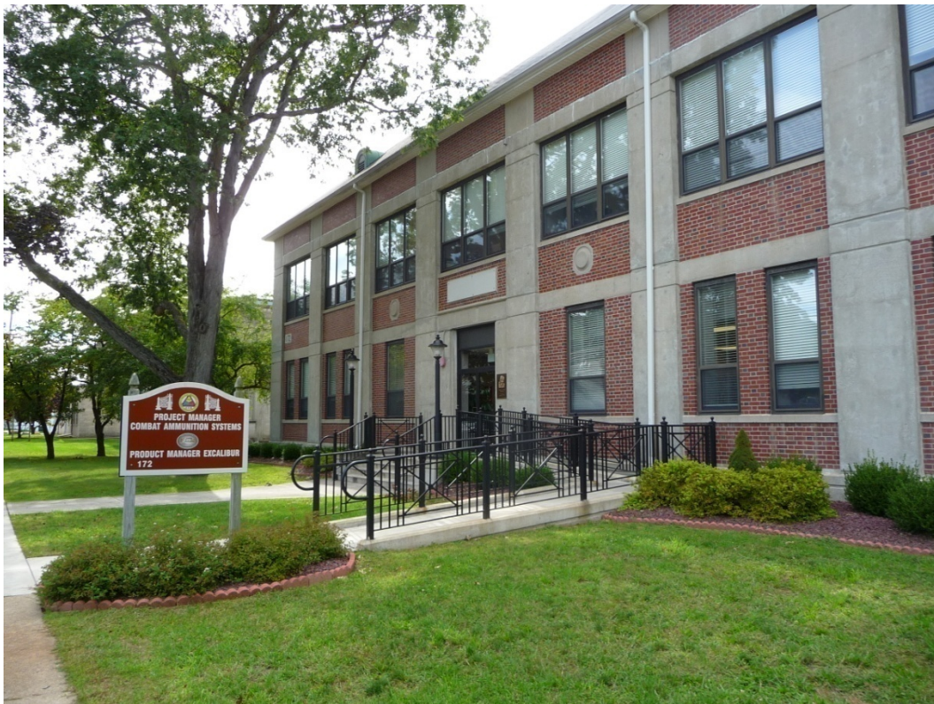
Figure 69. East elevation of Building 172 (ERDC-CERL, 2012).
