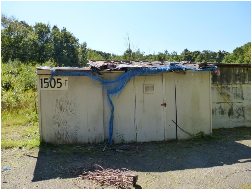
Figure 247. North elevation of Building 1505F (ERD-CERL, 2012).
