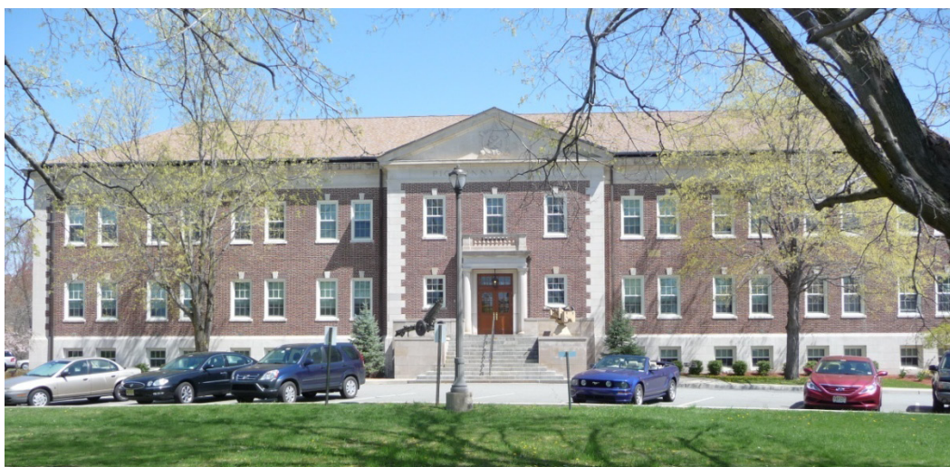
Figure 62. Southwest elevation of Building 151 (ERDC-CERL, 2012).
