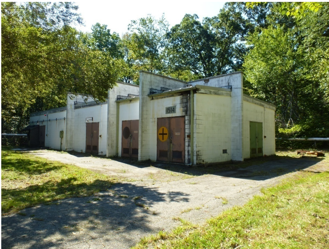
Figure 259. View south of Building 1514, Pyrotechnic R&D Laboratory (ERDC-CERL, 2012).
