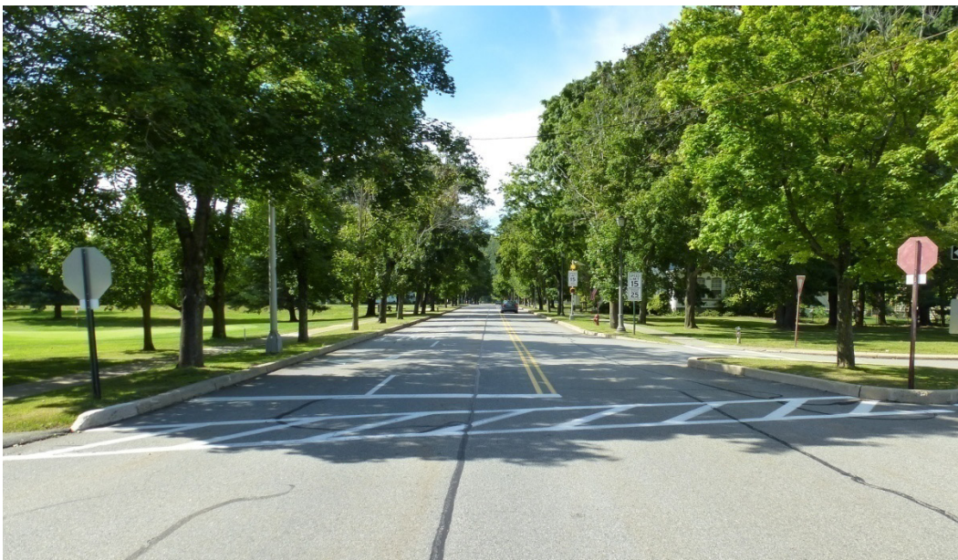
Figure 123. View looking west along Farley Avenue from the intersection with Parker Road (ERDC-CERL, 2012).
