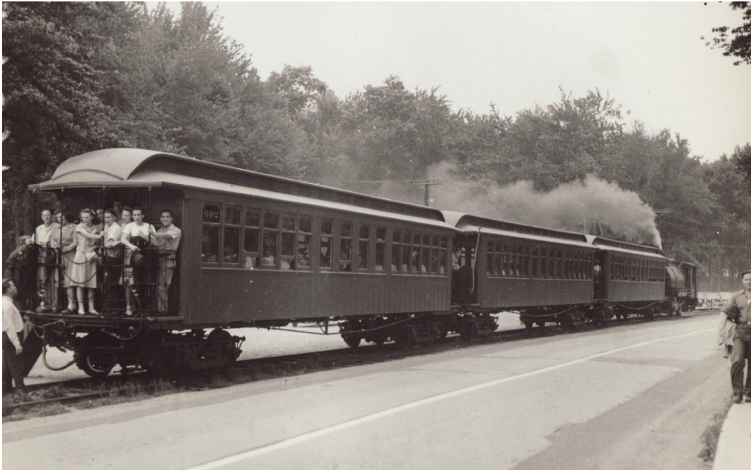
Figure 37. Train taking passengers (workers) to Back Line, 1940s (PICA Cultural Resources Office).
