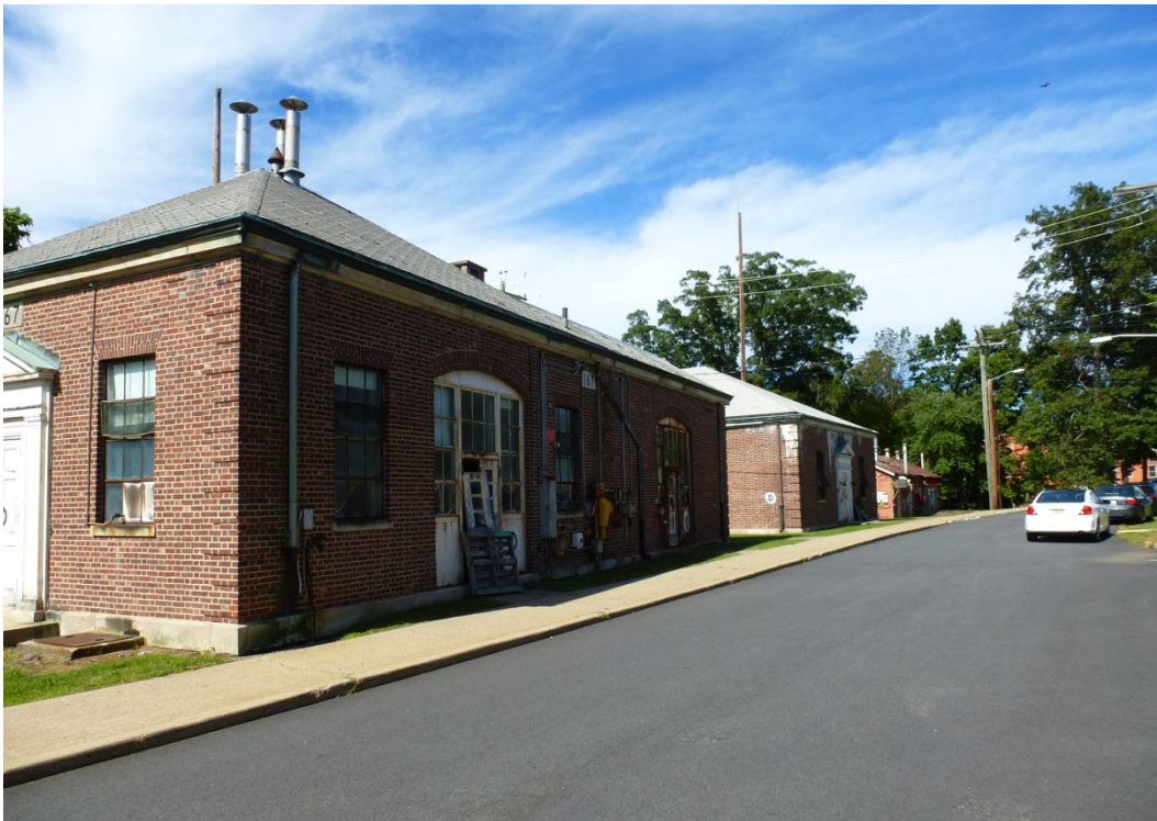
Figure 137. Chemistry Row, looking north showing the east sides of Buildings 167 (left) and 197 (right) along Kibler (ERDC-CERL, 2012).
