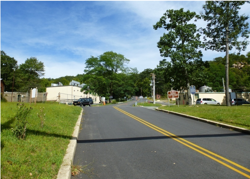
Figure 178. Looking north 20th Avenue leading to the 600 Test Area; Building 611 is at the left behind the parked car (ERDC-CERL, 2012).
