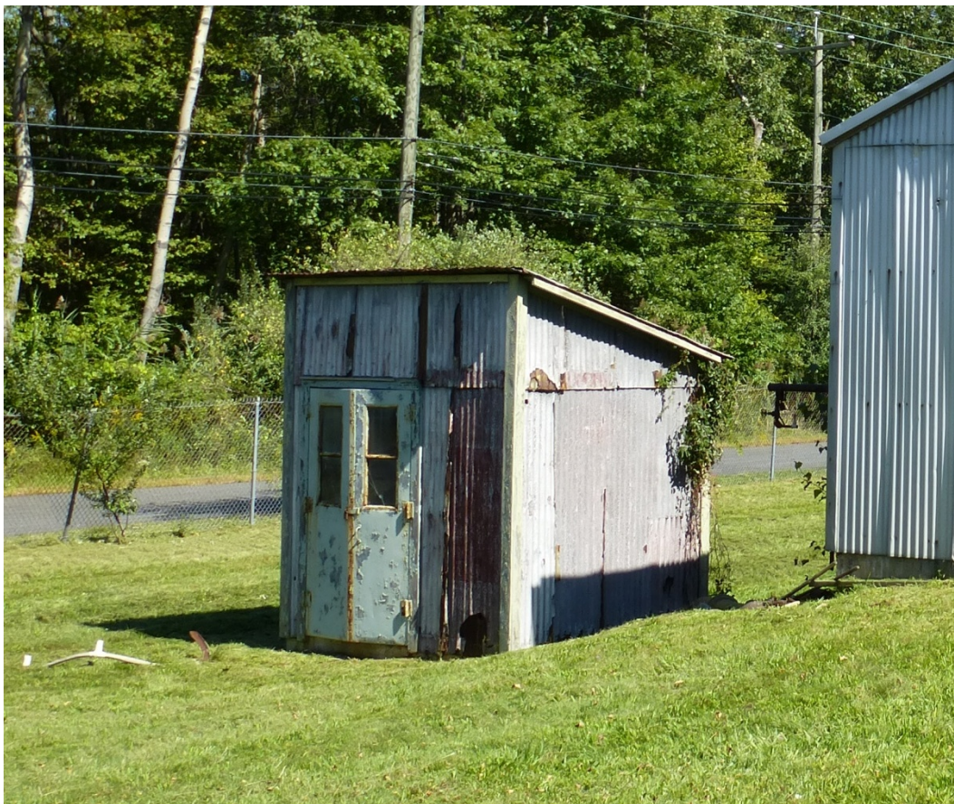
Figure 241. Southwest oblique of Building 1504A [Building 1504 is to right] (ERDC-CERL, 2012).
