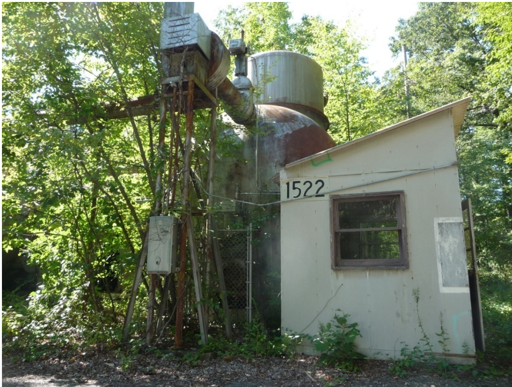
Figure 265. East elevation of Building 1522, now demolished (ERDC-CERL, 2012).
