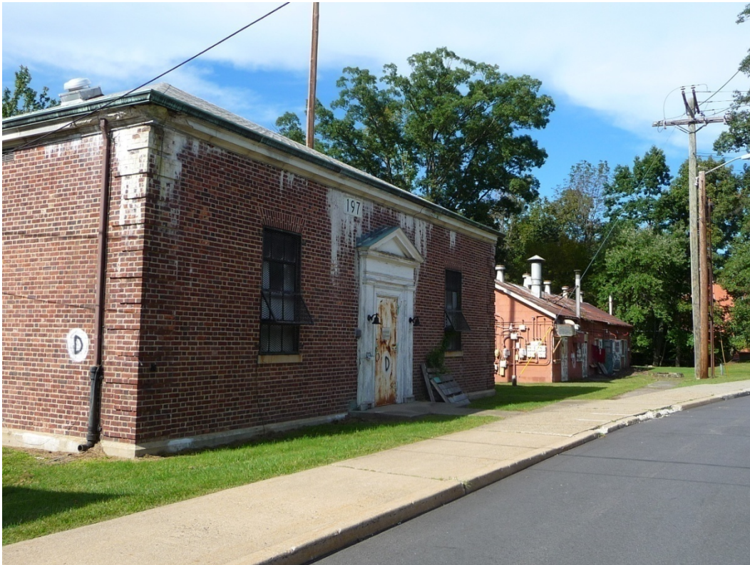
Figure 74. East elevation of Building 197 (ERDC-CERL, 2012).
