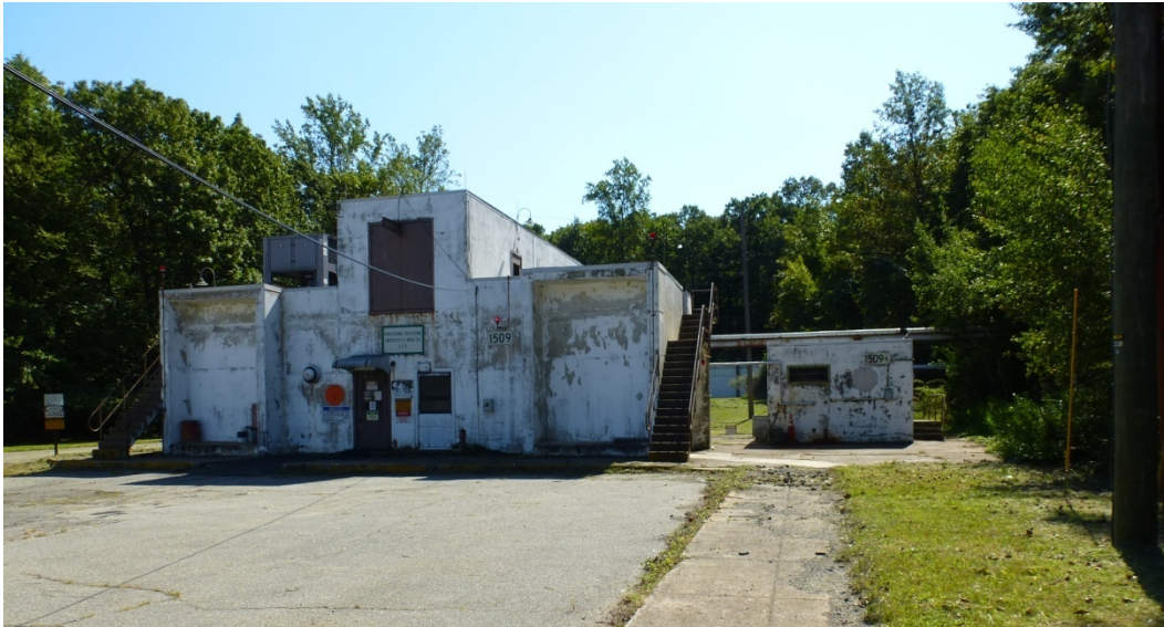
Figure 252. North elevation of Building 1509 (ERDC-CERL, 2012).
