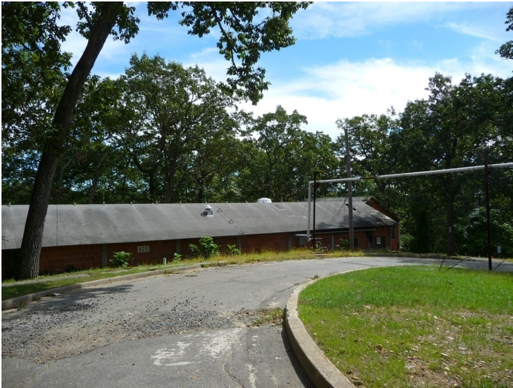
Figure 182. View looking south at 20 th Circle and Building 620 (ERDC-CERL, 2012).
