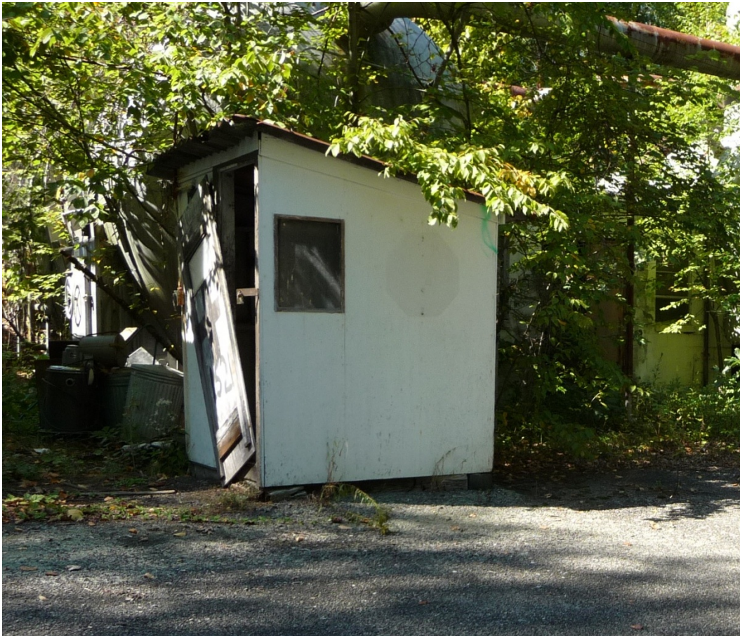
Figure 264. Building 1521, now demolished (ERDC-CERL, 2013).
