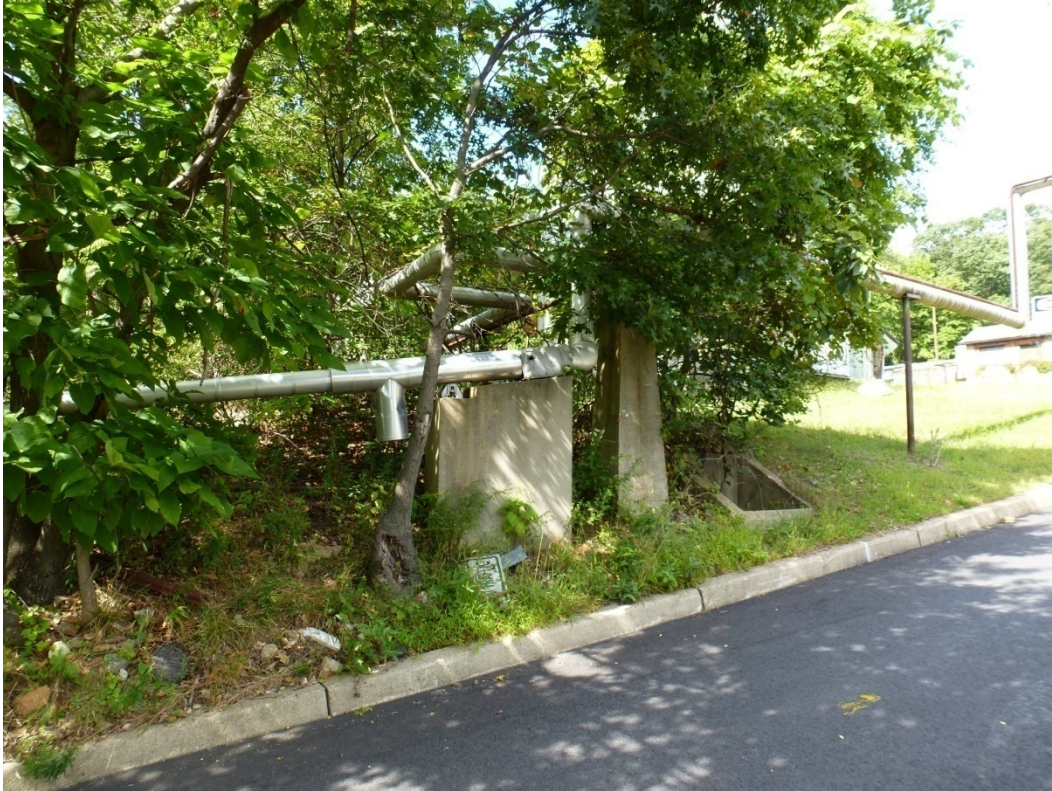
Figure 217. Remove vegetation from steam lines (ERDC-CERL, 2012).
