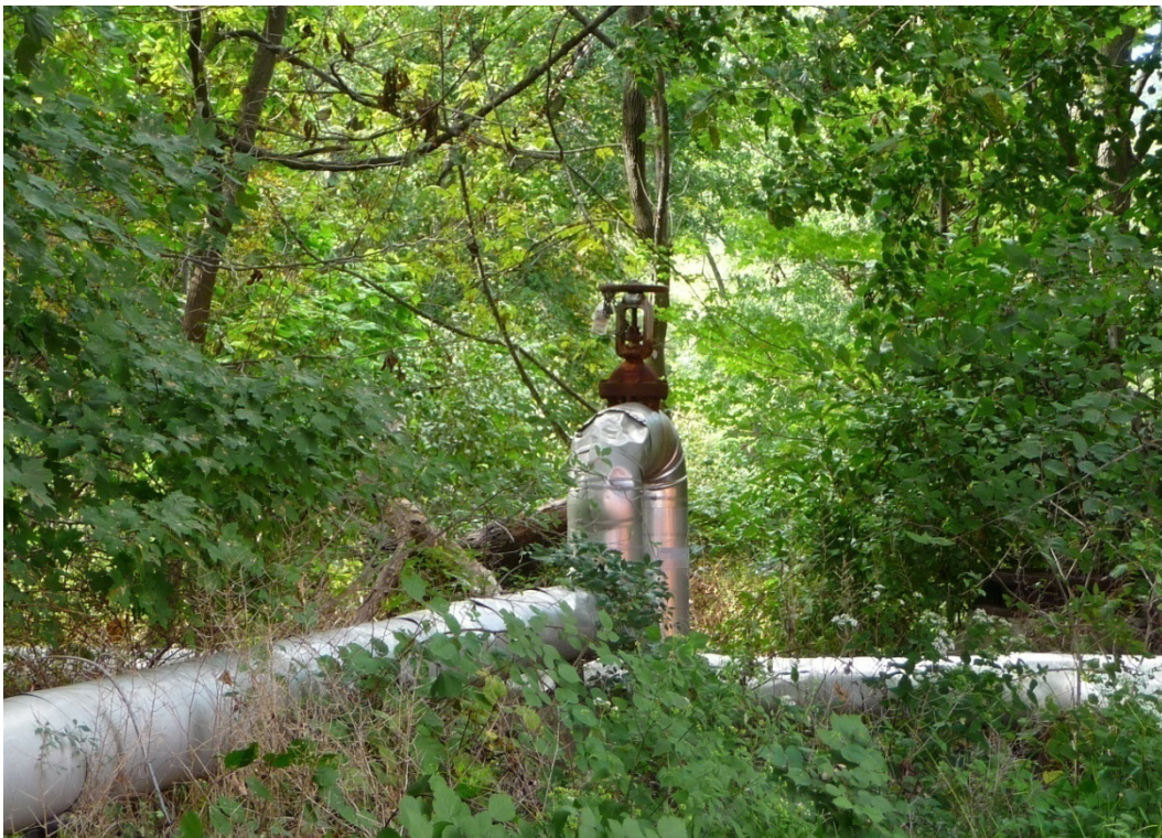
Figure 154. Overgrown vegetation around the steam lines in the Administrative and Research Historic District (ERDC-CERL, 2012).
