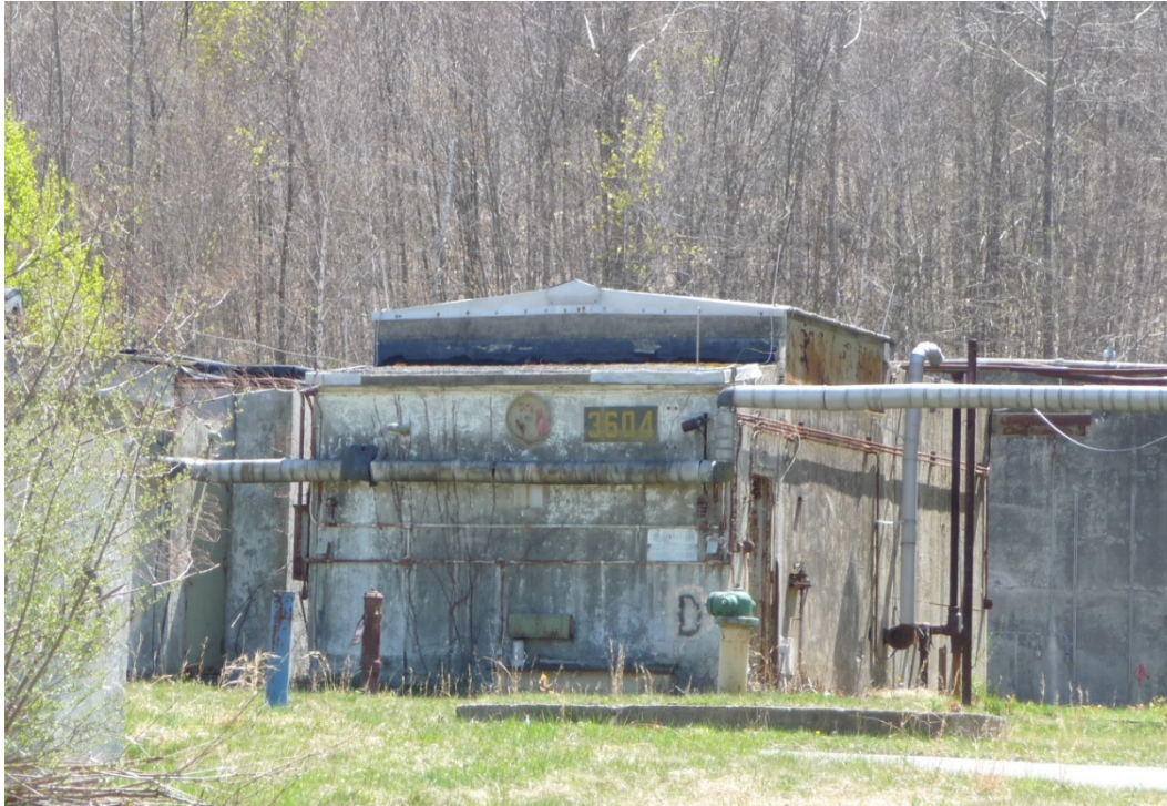
Figure 296. View south at Building 3604 (ERDC-CERL, 2013).
