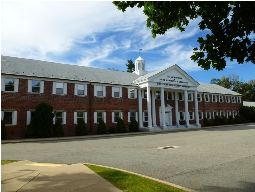
Figure 50. Building 1, Administration Building/Post Headquarters (ERDC-CERL 2012).
