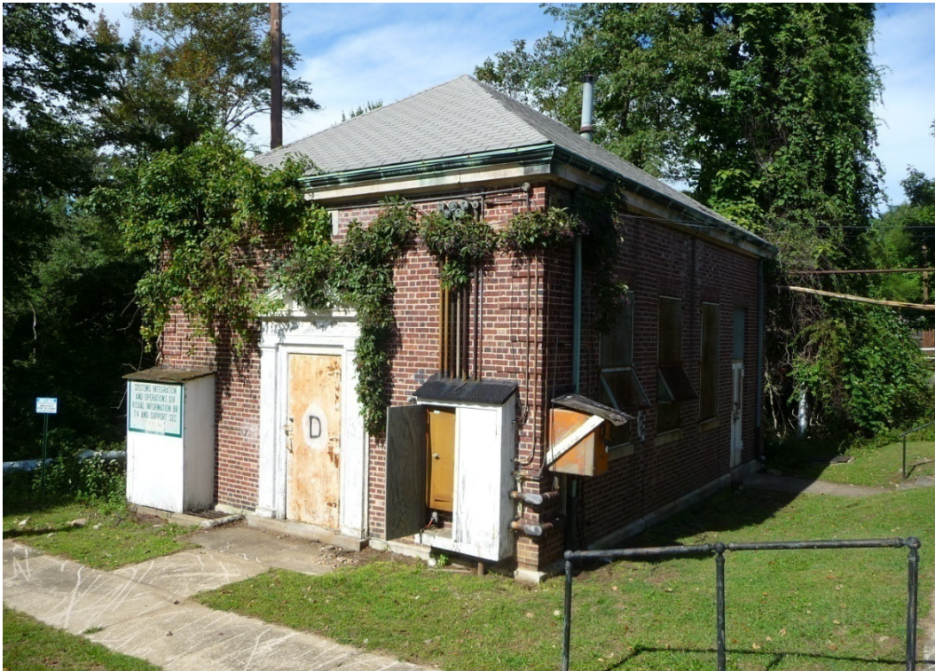
Figure 65. Southwest elevation of Building 164 (ERDC-CERL, 2012).
