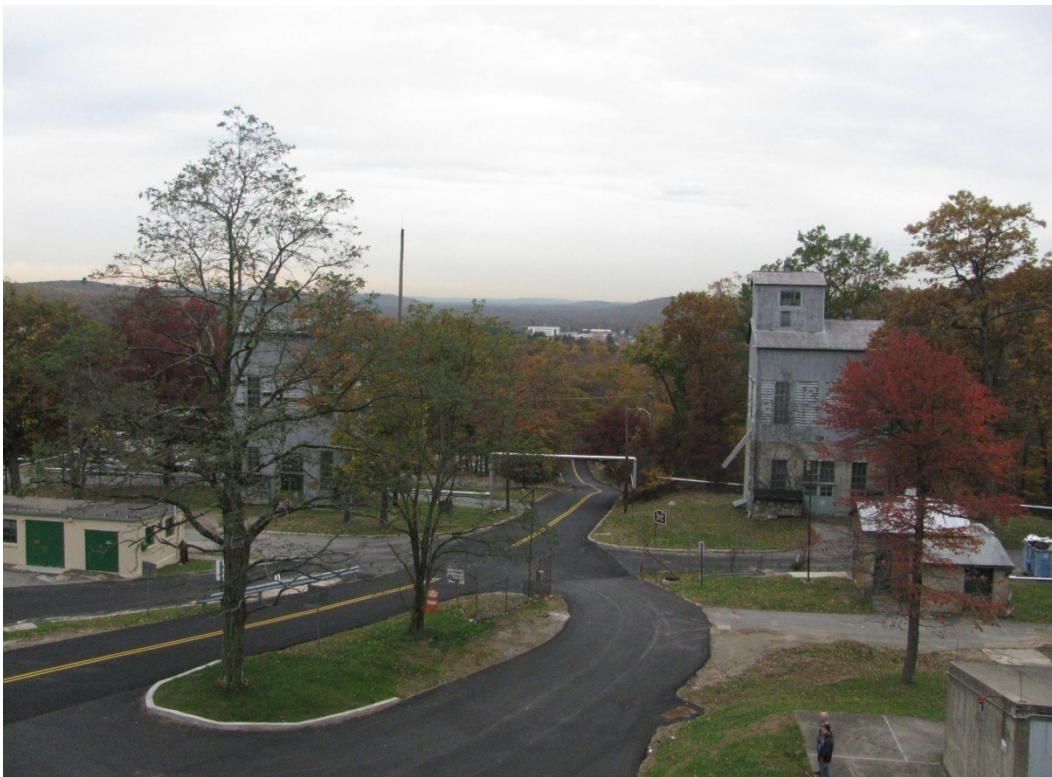
Figure 175. View from hillside, looking south on 20th Avenue (PICA Cultural Resources Office).
