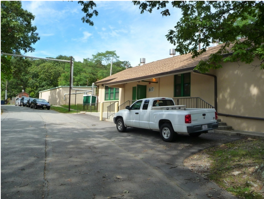
Figure 199. South elevation of Building 617 (ERDC-CERL, 2012).
