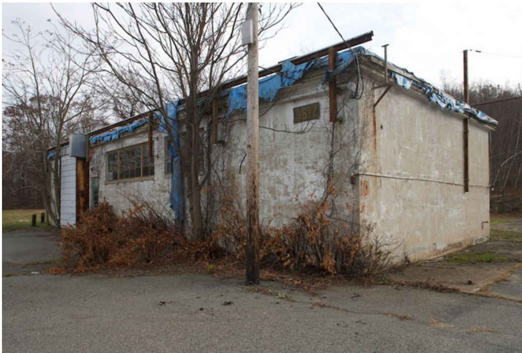
Figure 304. Building 3612, NARTS Components Testing (PICA Cultural Resources Office, 2010).
