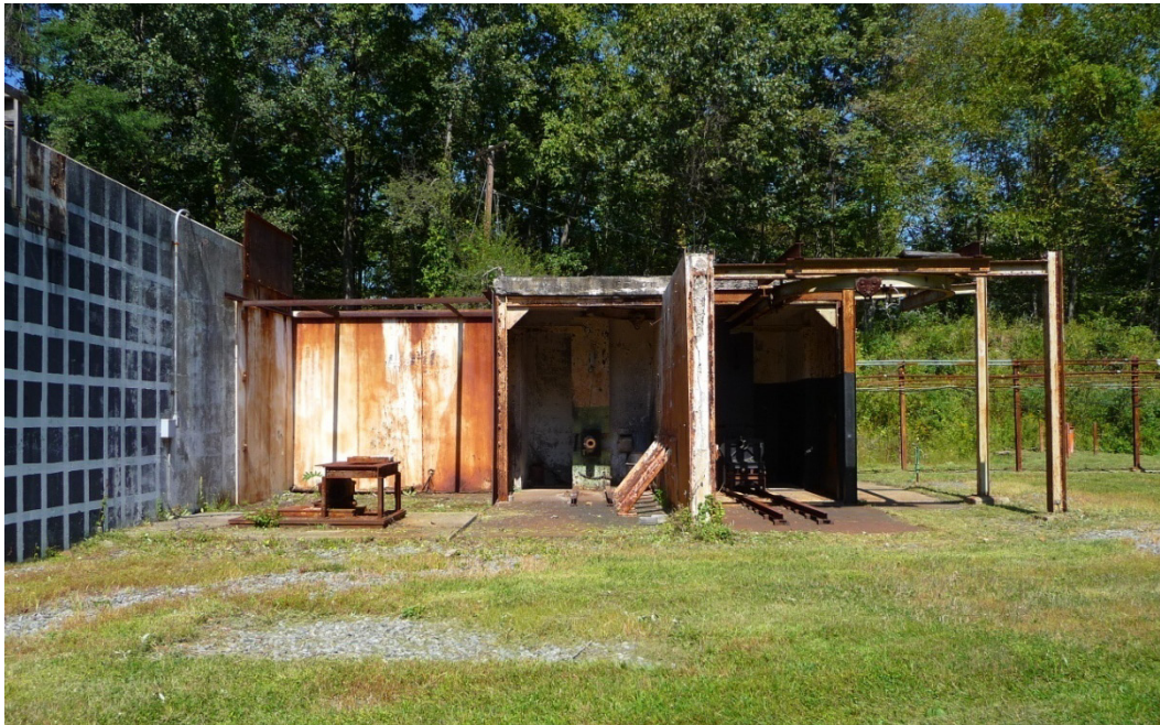
Figure 243. Building 1505A (left) and Building 1505B (right), Test Cells (ERDC-CERL, 2012).
