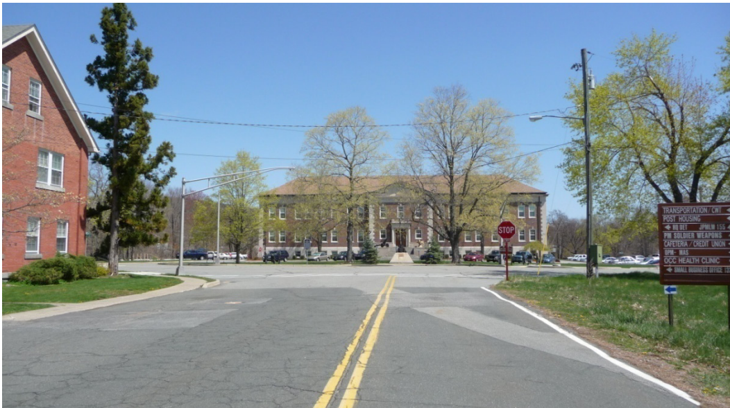
Figure 117. View north on Parker Road looking at Building 151 (ERDC-CERL, 2013).
