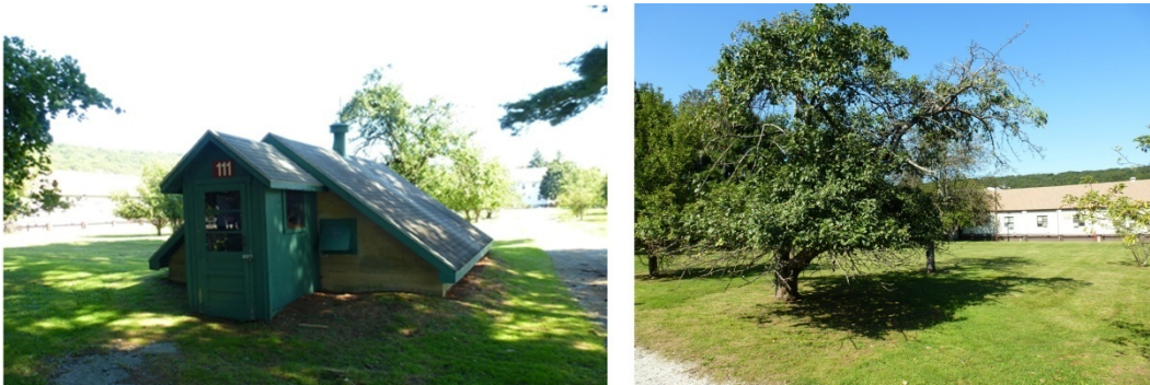
Figure 159. Root cellar (Building 111) and orchard located behind Building 112 (ERDC-CERL, 2012).
