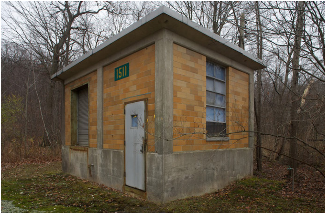
Figure 255. Northwest oblique of Building 1511 (PICA Cultural Resources Office, 2012).
