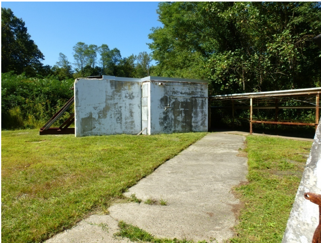
Figure 246. East elevation of Building 1505E and covered walkway (ERDC-CERL, 2012).
