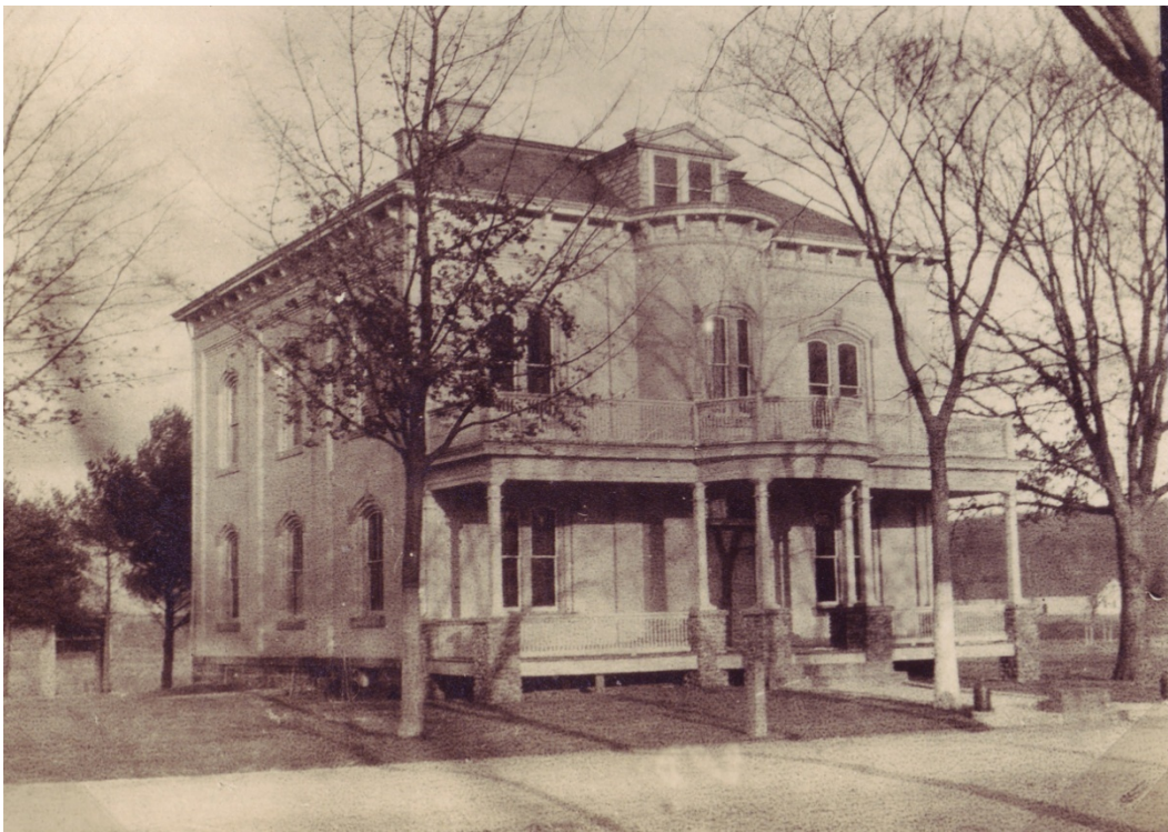
Figure 14. Historic photograph of Building 114, 1913 (PICA Cultural Resources Office).
