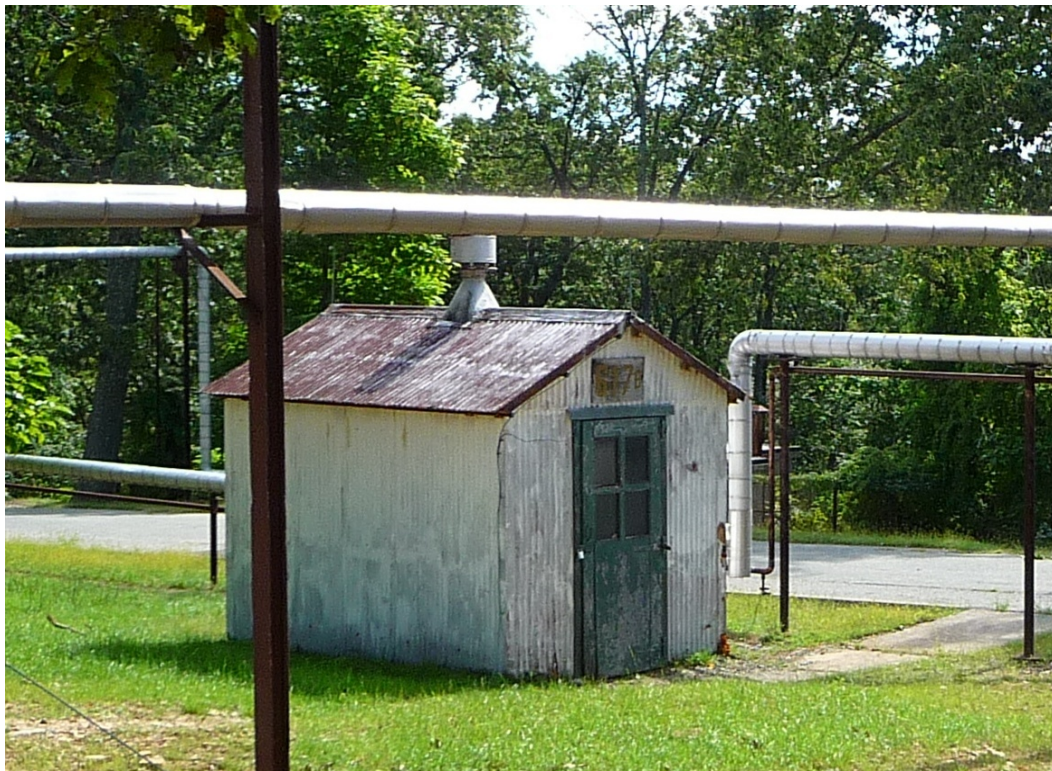
Figure 201. Northwest oblique of Building 617B (ERDC-CERL, 2012).
