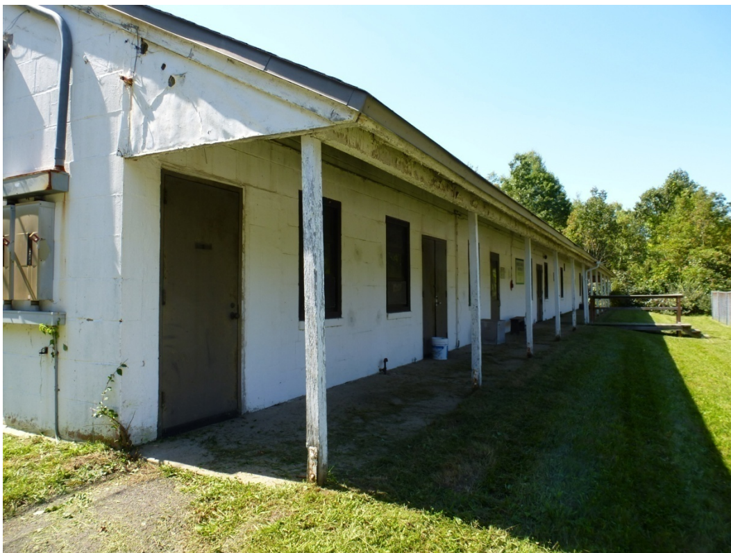
Figure 237. Left side of the north elevation of Building 1501 (ERDC-CERL, 2012).
