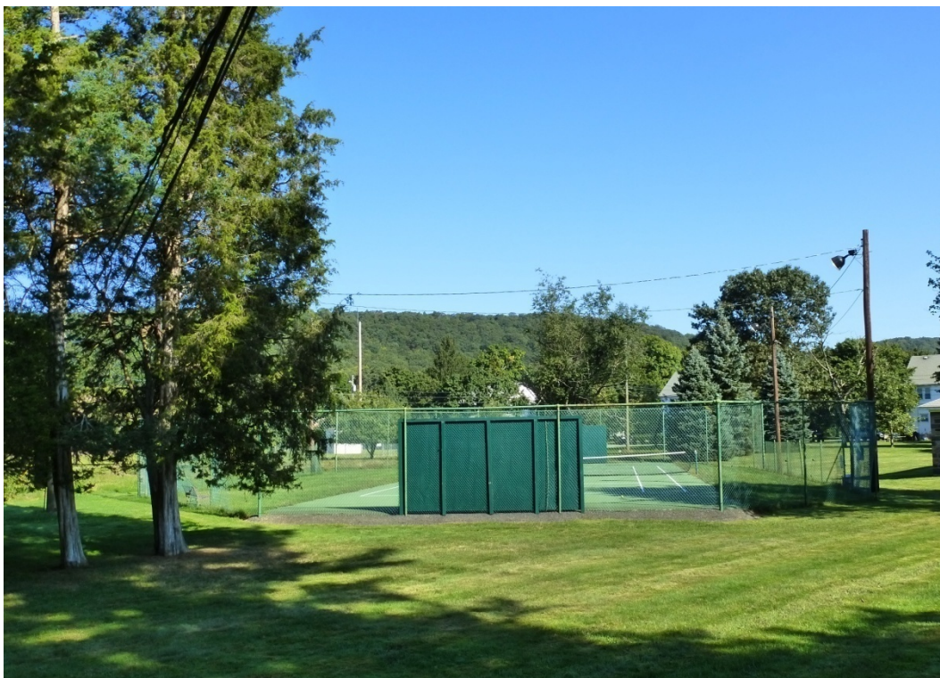
Figure 53. Looking north towards Building 112A, Tennis Courts (ERDC-CERL, 2012).
