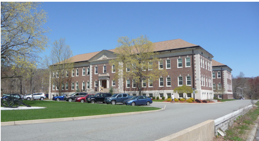
Figure 118. Looking north from Farley Avenue at the south elevation of Building 151 (ERDC-CERL, 2013).
