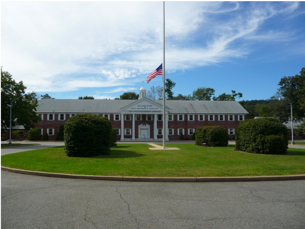
Figure 132. East elevation of Building 1 (Headquarters) (ERDC-CERL, 2012).
