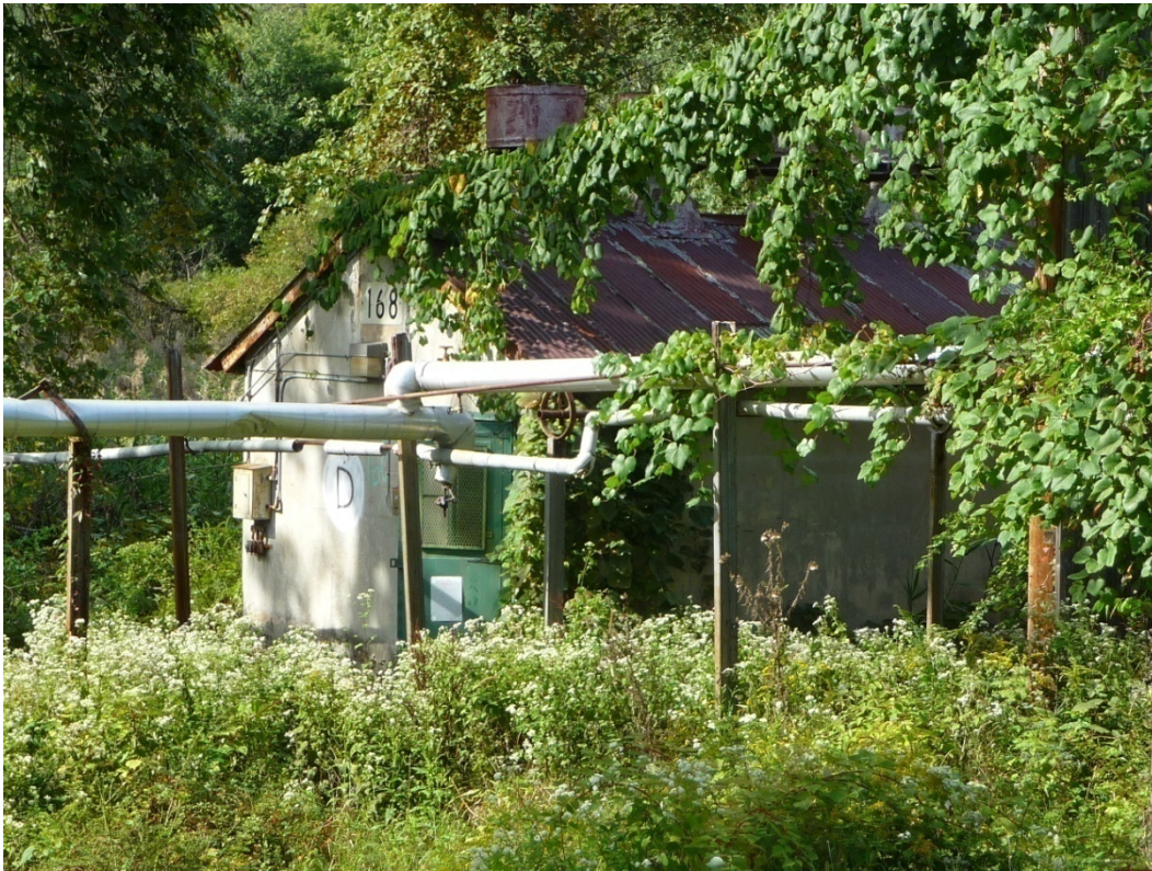
Figure 68. Look north at Building 168 (ERDC-CERL, 2012).
