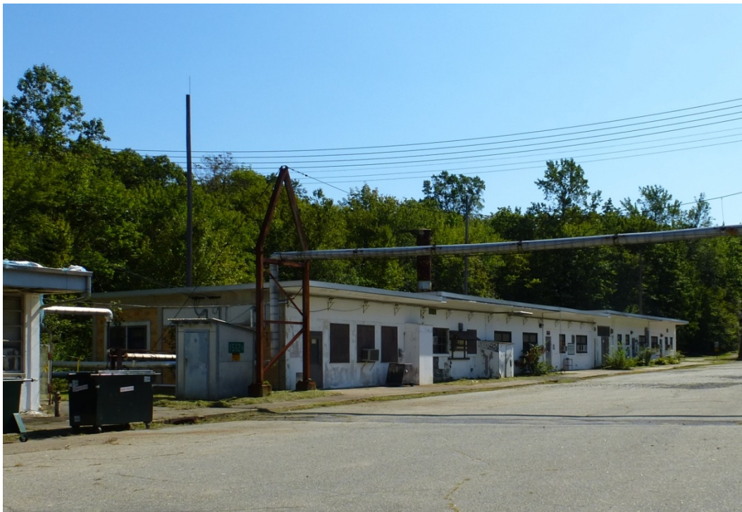
Figure 260. View south of Building 1515 (ERDC-CERL, 2012).
