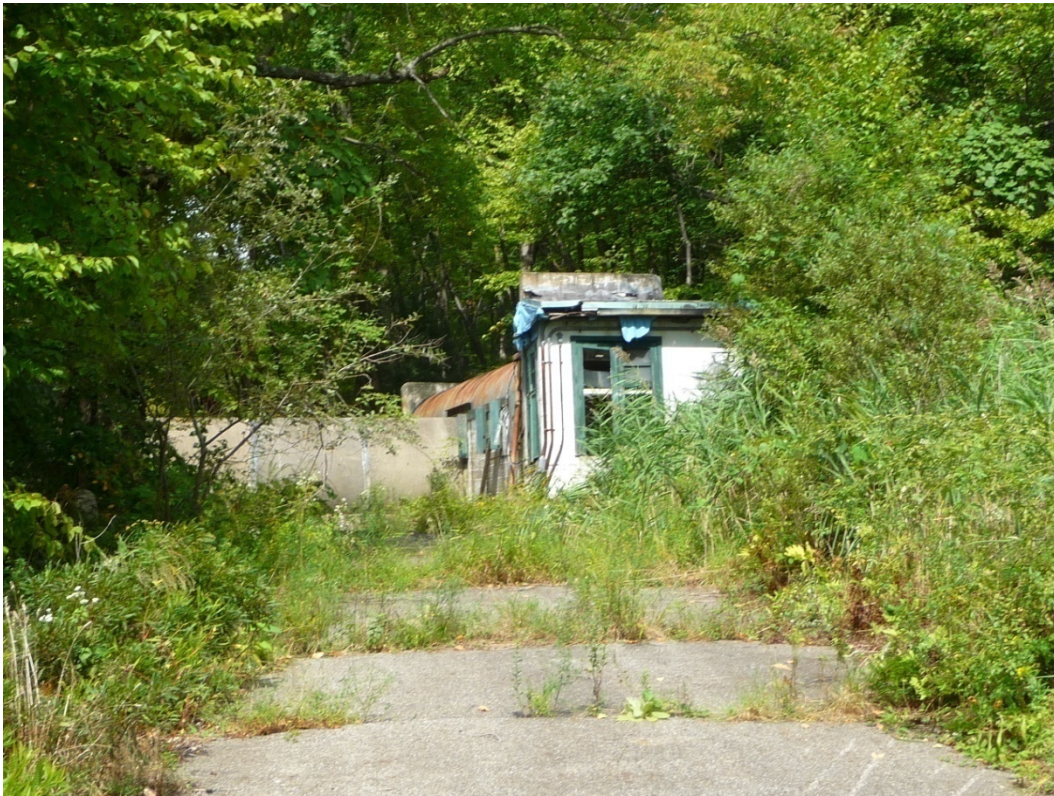
Figure 196. Looking north at Building 611B, Gas Gun Test Tunnel (ERDC-CERL, 2012).
