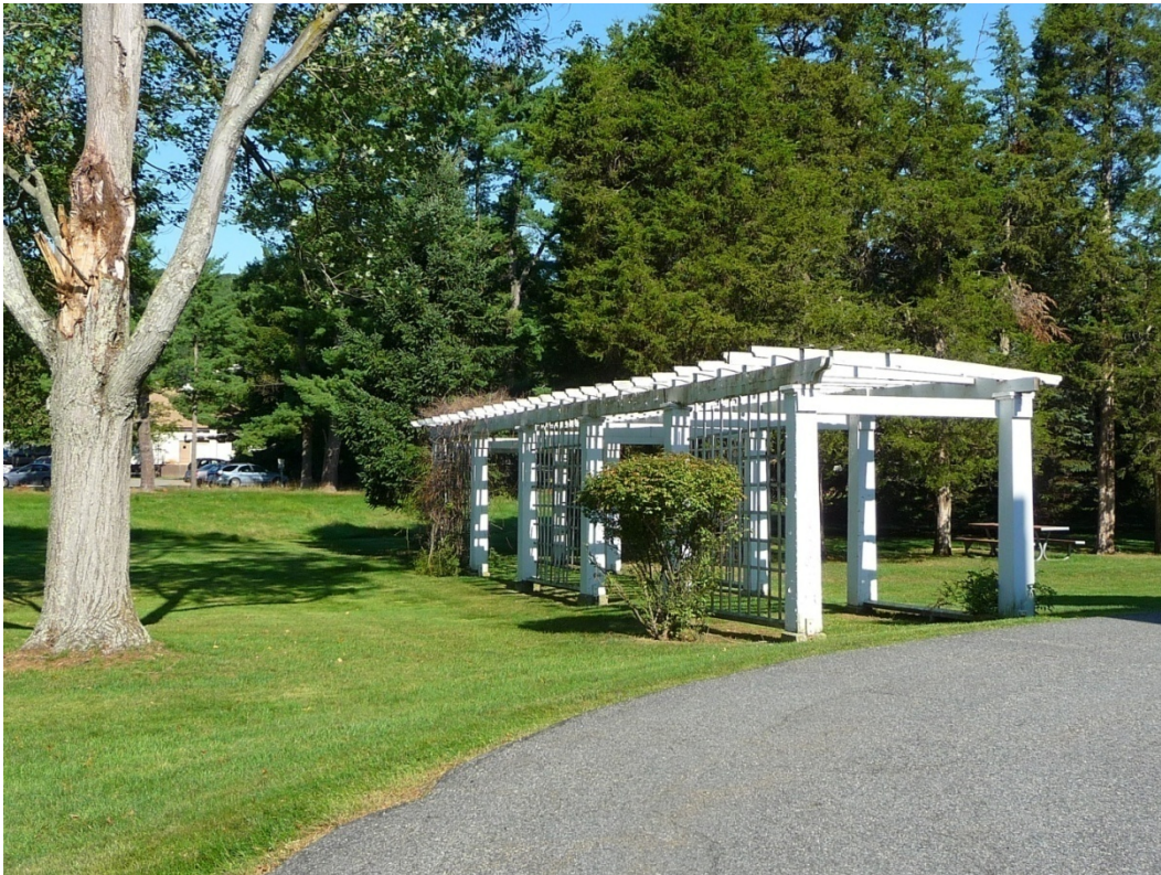
Figure 54. View of Building 112B, pergola (ERDC-CERL, 2012).
