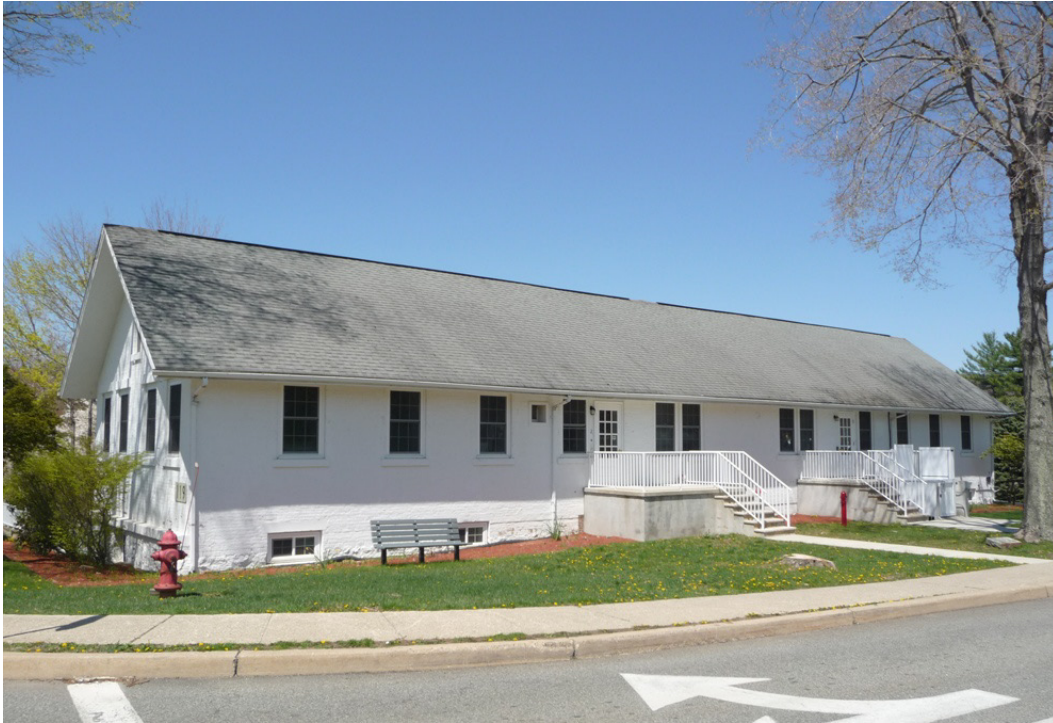
Figure 22. Building 119 after addition of wheelchair lifts in 2010 (ERDC-CERL, 2013).
