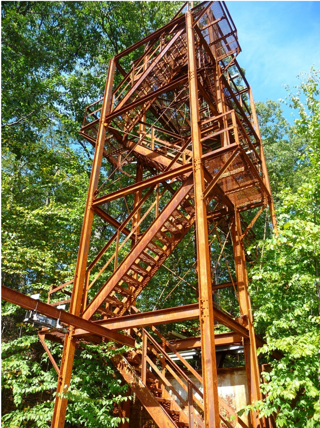
Figure 191. Building 604D, Drop Tower (ERDC-CERL, 2012).
