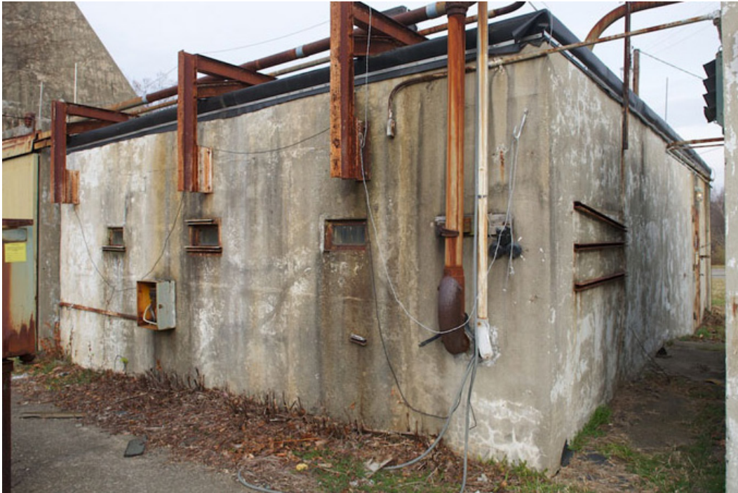
Figure 297. Southeast oblique of Building 3605, NARTS Control House (PICA Cultural Resources Office, 2010).
