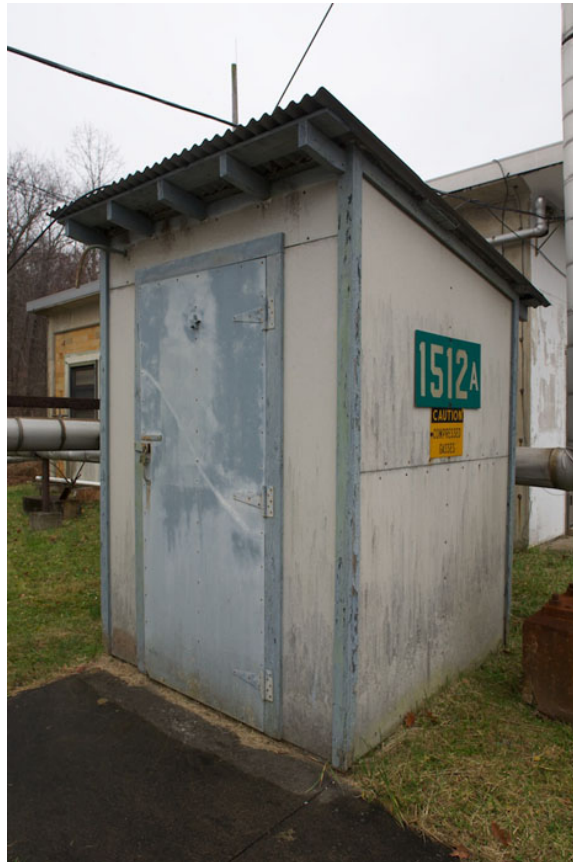
Figure 257. View south of Building 1512A, General Purpose Storehouse (PICA Cultural Resources Office, 2012).
