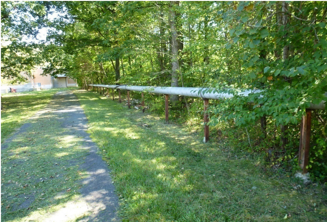
Figure 266. Remnants of steam conduit supported on cast stone piers (ERDC-CERL, 2012).
