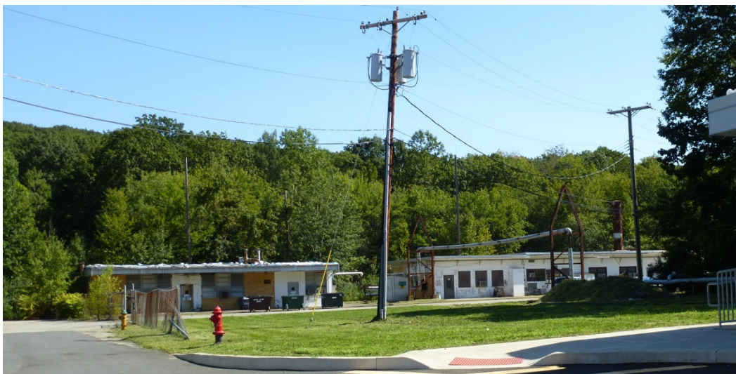
Figure 232. Buildings 1512 (left) and 1515 (right) in the Storage and Laboratory Area on the east side of the district (ERDC-CERL, 2012).
