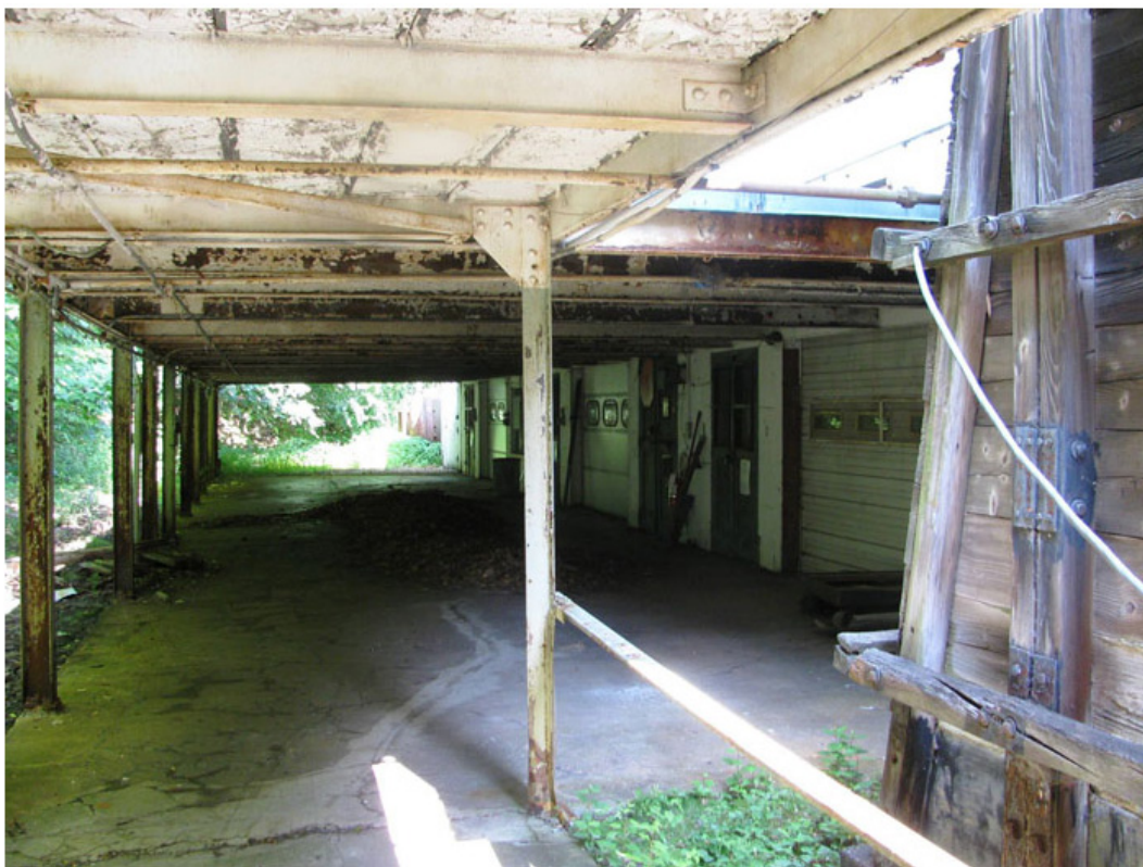
Figure 239. Southwest side of Building 1503 (PICA Cultural Resources Office).
