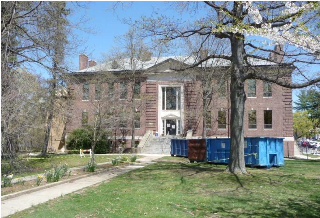
Figure 63. South elevation of Building 162 (ERDC-CERL, 2013).
