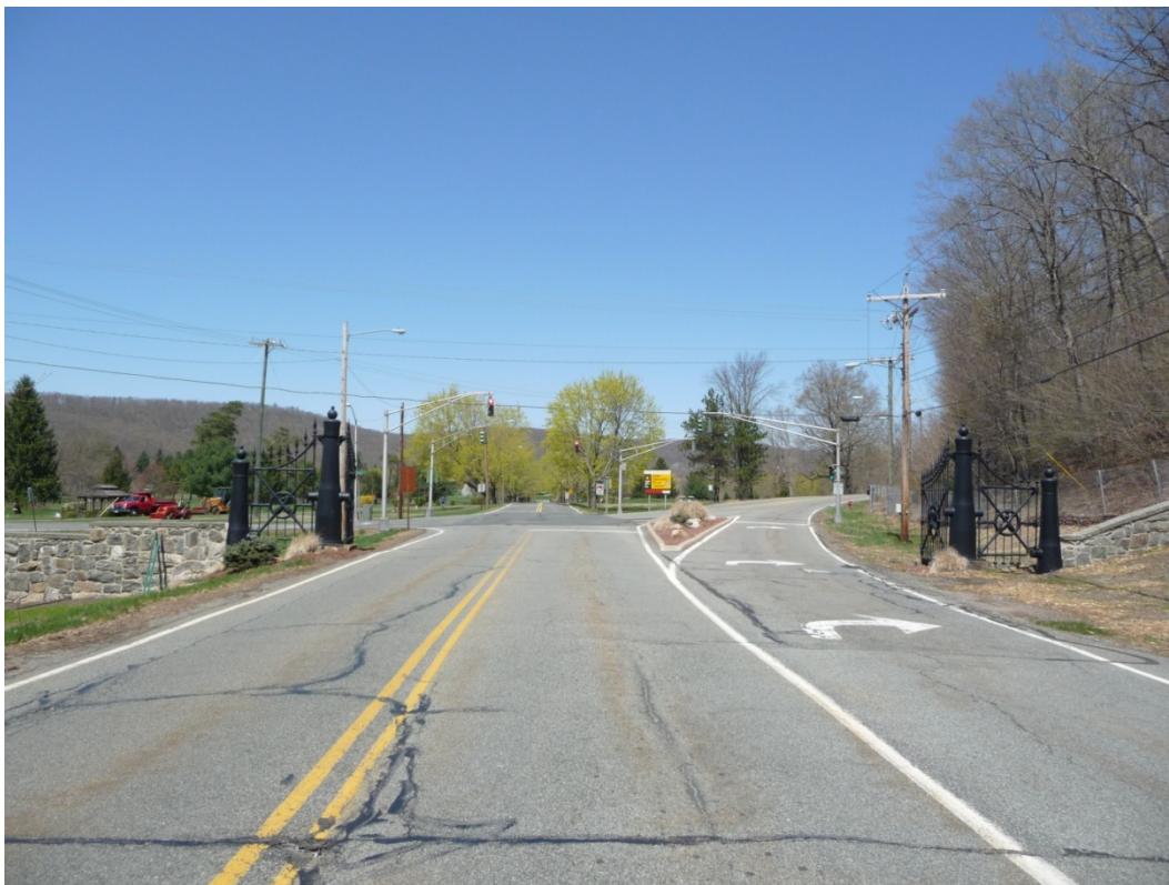
Figure 148. View looking north from outside the installation toward Cannon Gates (ERDC-CERL, 2012).
