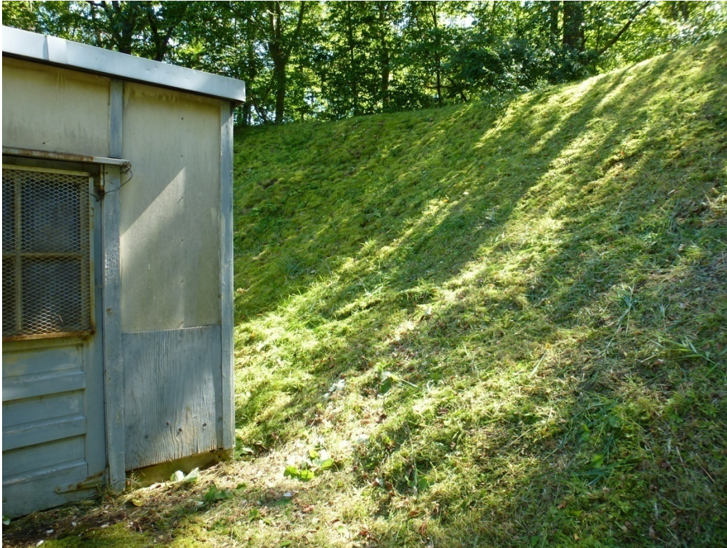
Figure 274. Relationship of building and earth barricade (ERDC-CERL, 2012).
