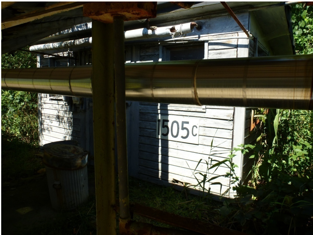
Figure 244. Building 1505C (ERDC-CERL, 2012).
