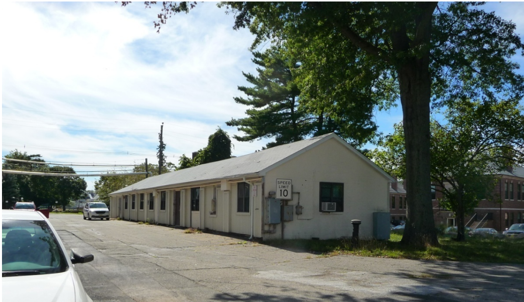
Figure 71. East elevation of Building 174 (ERDC-CERL, 2012).
