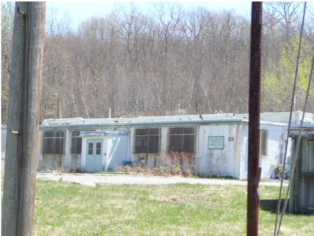
Figure 299. Building 3607, Central Control Room (ERDC-CERL, 2013).
