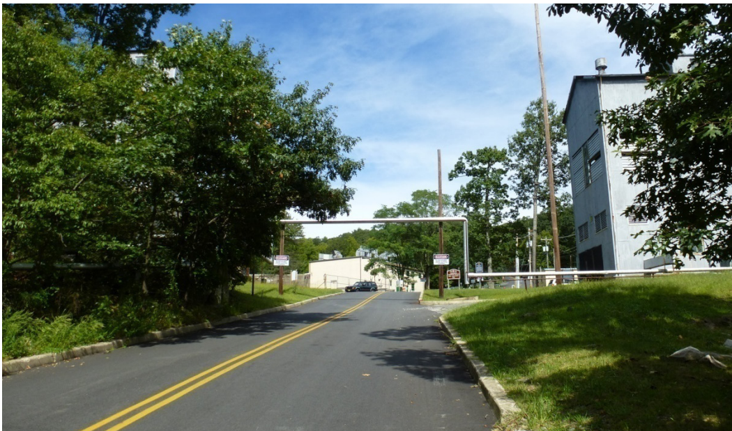
Figure 207. Elevated steam lines stretch over 20 th Avenue (ERDC-CERL, 2012).
