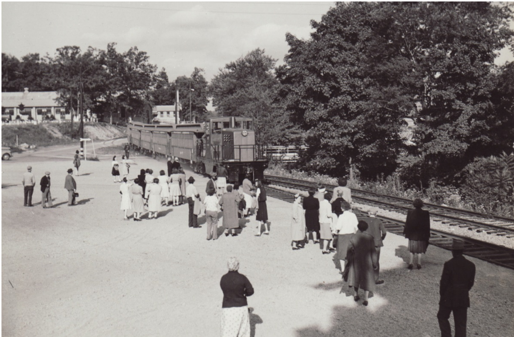
Figure 38. Train cars taking employees from the gate to the far end of the loading area, 1943 (PICA Cultural Resources Office).
