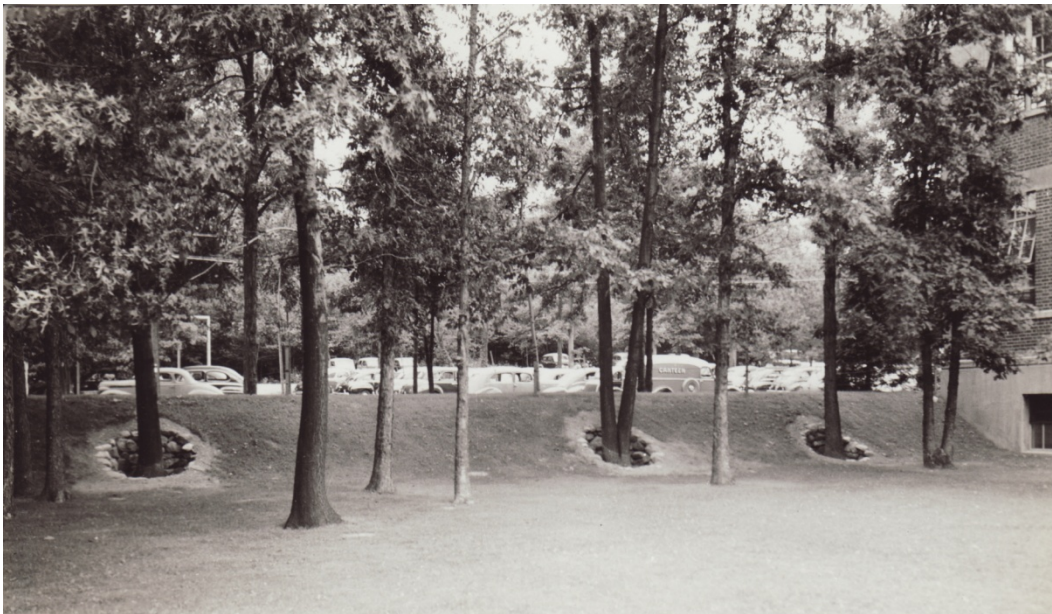
Figure 90. Historic photo of typical tree wells for tree protection on north side Building 172, 1943 (PICA Cultural Resources Office).
