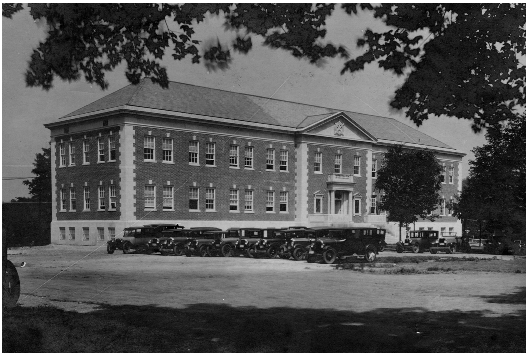
Figure 23. Historic photograph of Building 151, circa 1930s (PICA Cultural Resources Office).
