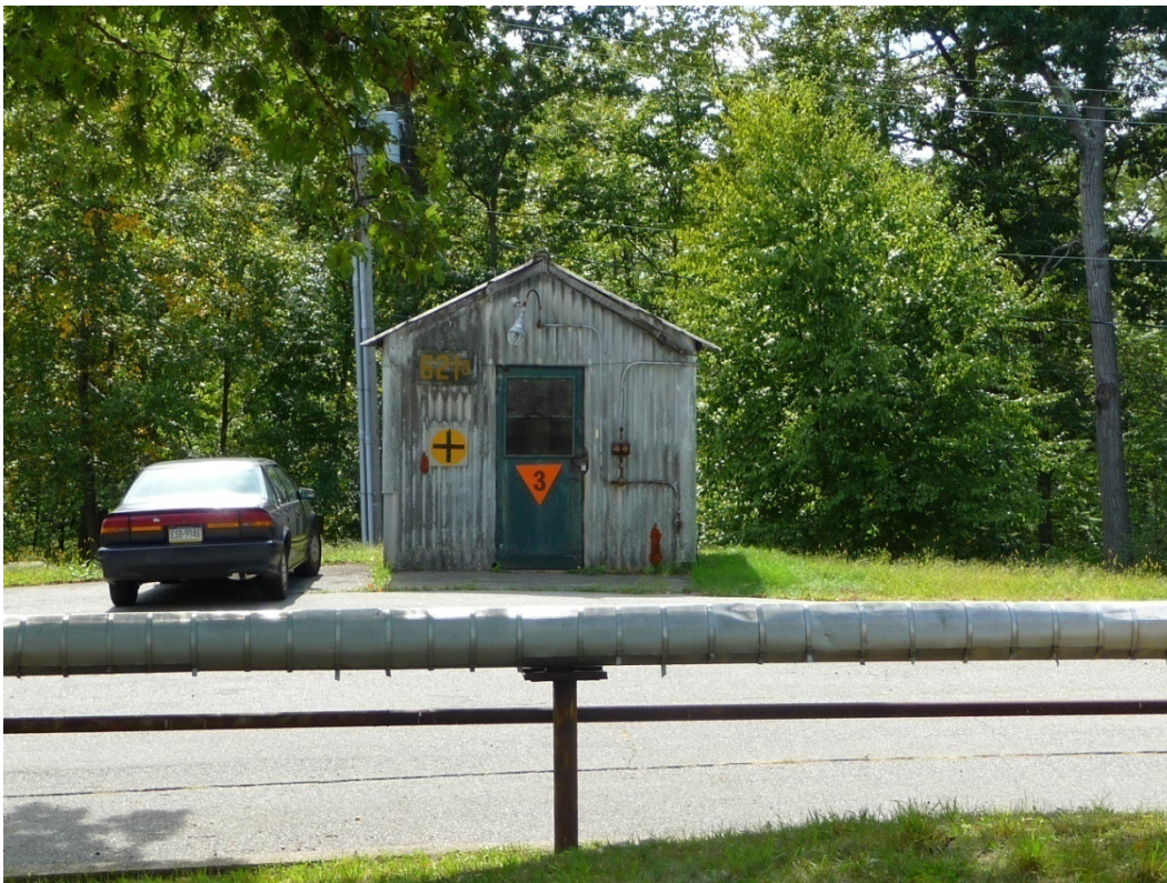
Figure 206. View of front façade of Building 621B (ERDC-CERL, 2012).
