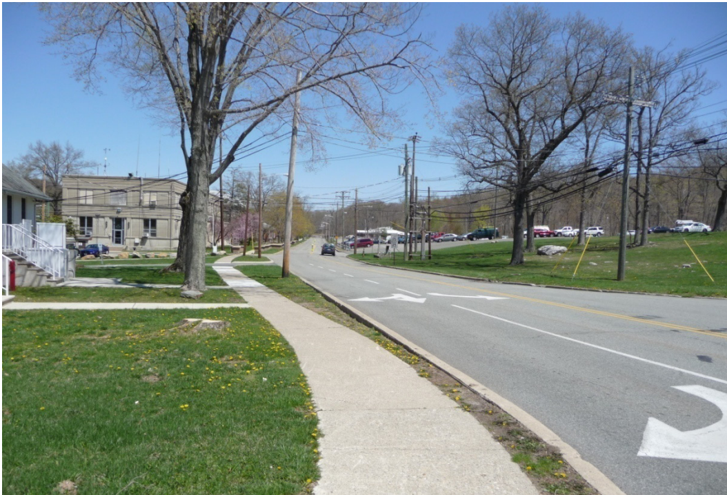
Figure 141. Looking north down Buffington Road from intersection at Farley Avenue (ERDC-CERL, 2013).
