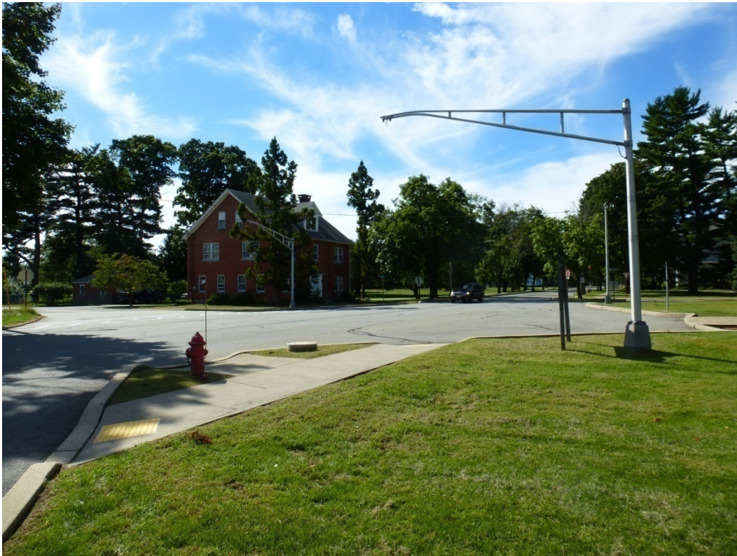
Figure 122. View looking southeast at the intersection of Parker Road and Farley Avenue (ERDC-CERL, 2012).
