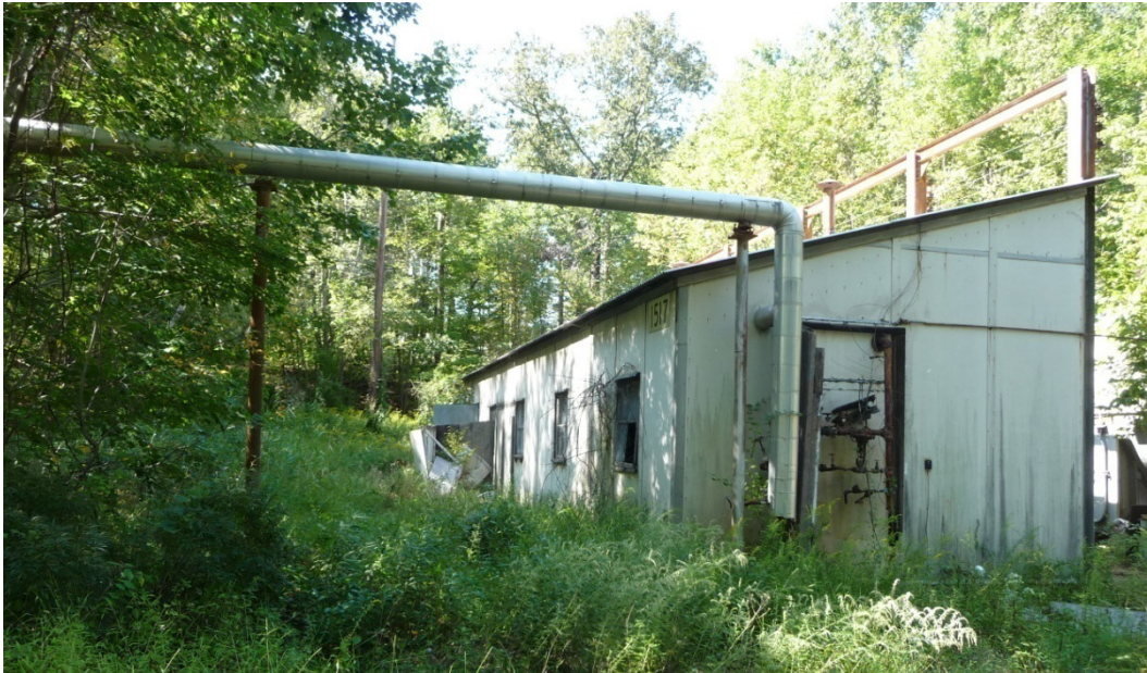
Figure 261. Building 1517, now demolished, consisted of two large, connected chambers and a number of associated, connected buildings (ERDC-CERL, 2012).
