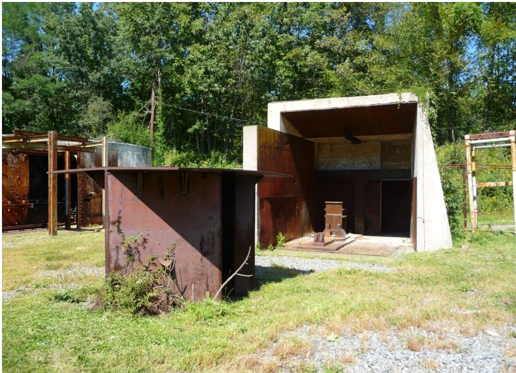
Figure 245. Building 1505D, Test Cell (ERDC-CERL, 2012).
