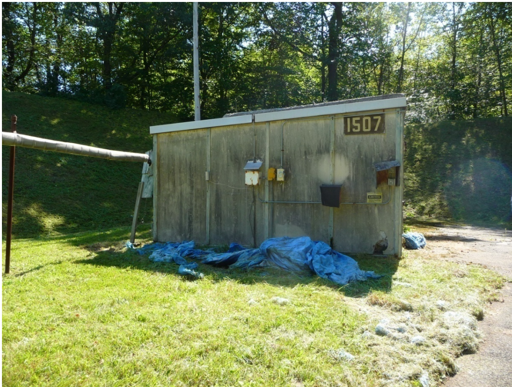
Figure 250. North elevation of Building 1507 (ERDC-CERL, 2012).
