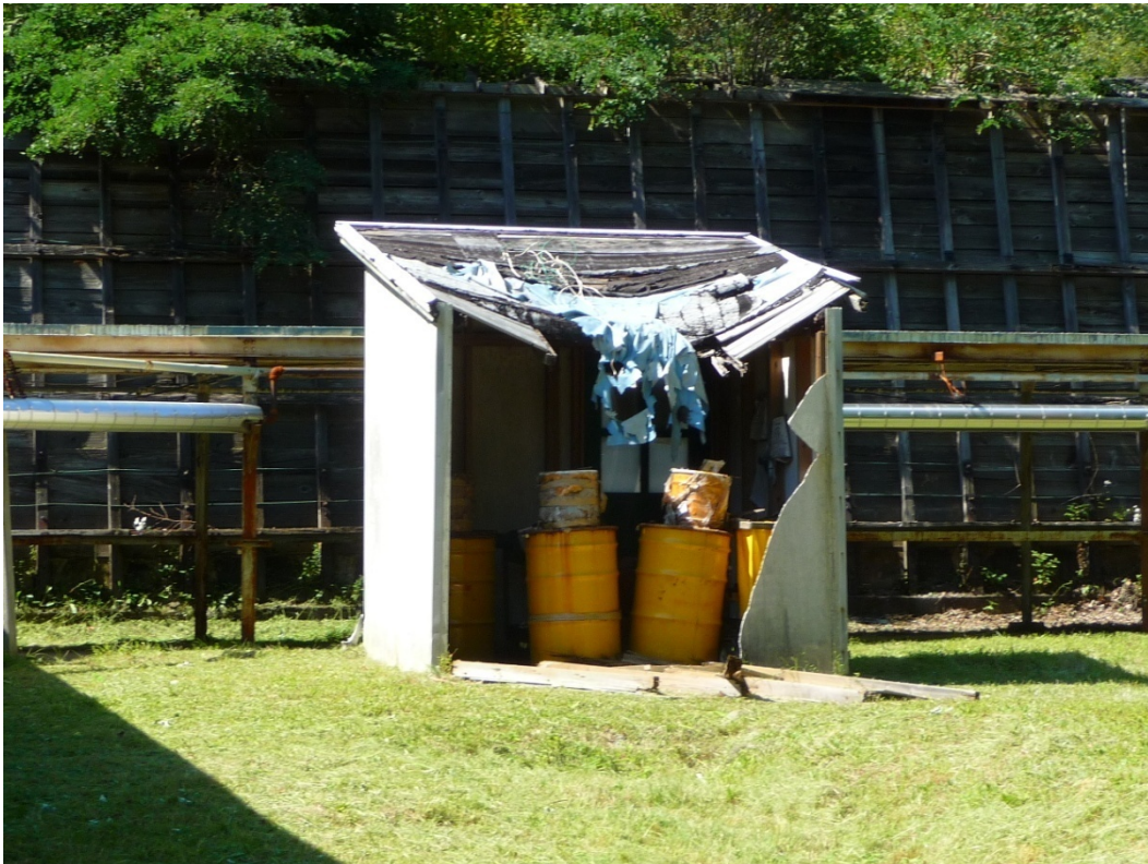
Figure 251. Building 1508, High Explosives Magazine (ERDC-CERL, 2012).
