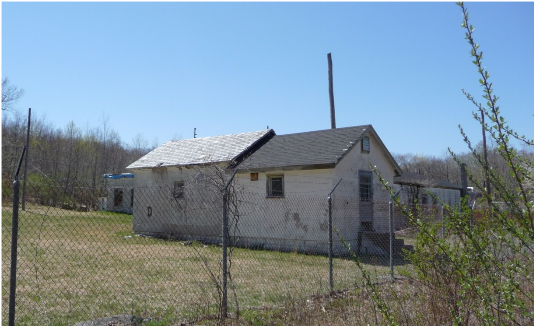
Figure 306. Northwest oblique of Building 3615, NARTS Utility House (ERDC-CERL, 2013).
