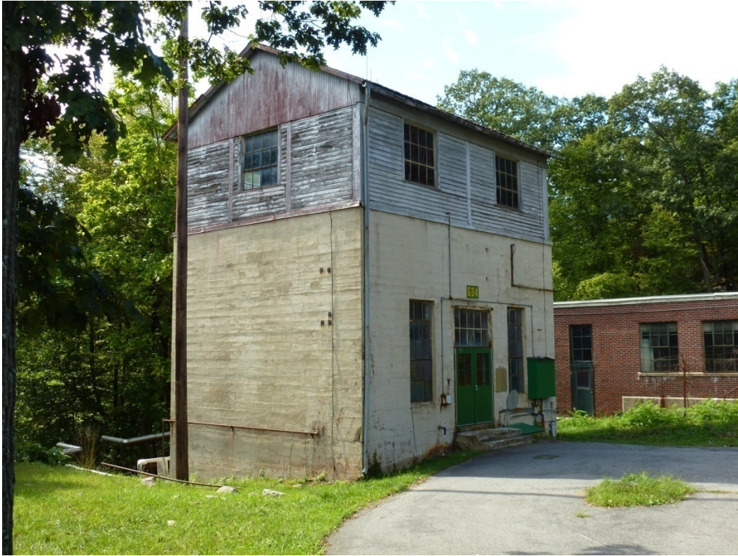
Figure 187. Building 604, northeast oblique (ERDC-CERL, 2012).
