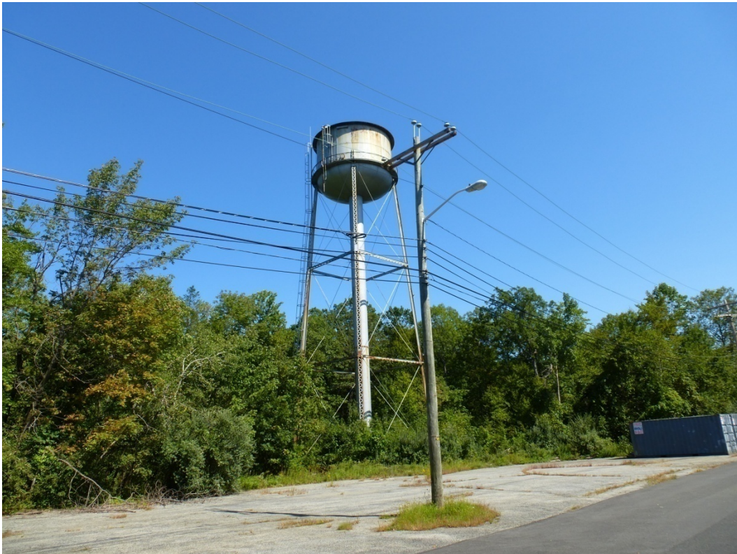
Figure 236. Current condition of the water tower, Building 1500 (ERDC-CERL, 2012).
