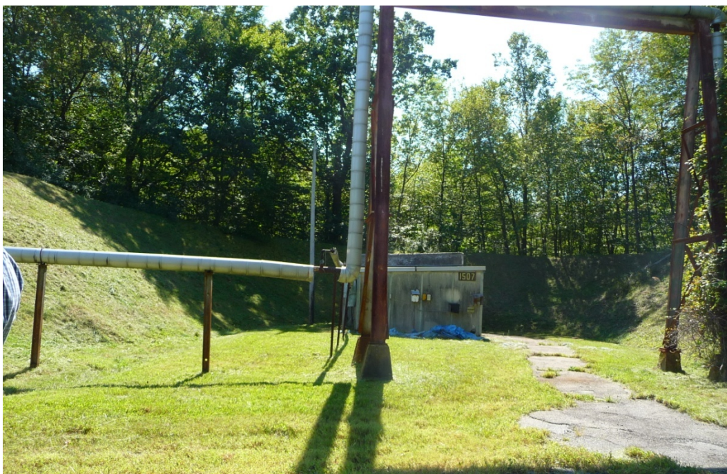
Figure 273. Earth barricades around Building 1507 (ERDC-CERL, 2012).
