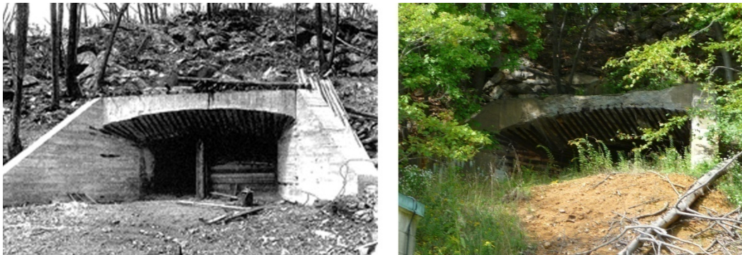
Figure 184. Comparison photographs of a slug butt (611B); on the left is historic photograph (taken from Picatinny website, undated), and on the right is a current photograph of the same structure which is now partially obstructed by debris (ERDC-CERL, 2012).
