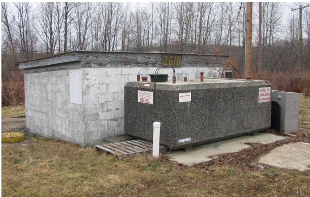
Figure 302. Building 3610, NARTS Liquid Propellant Storage (PICA Cultural Resources Office, 2010).
