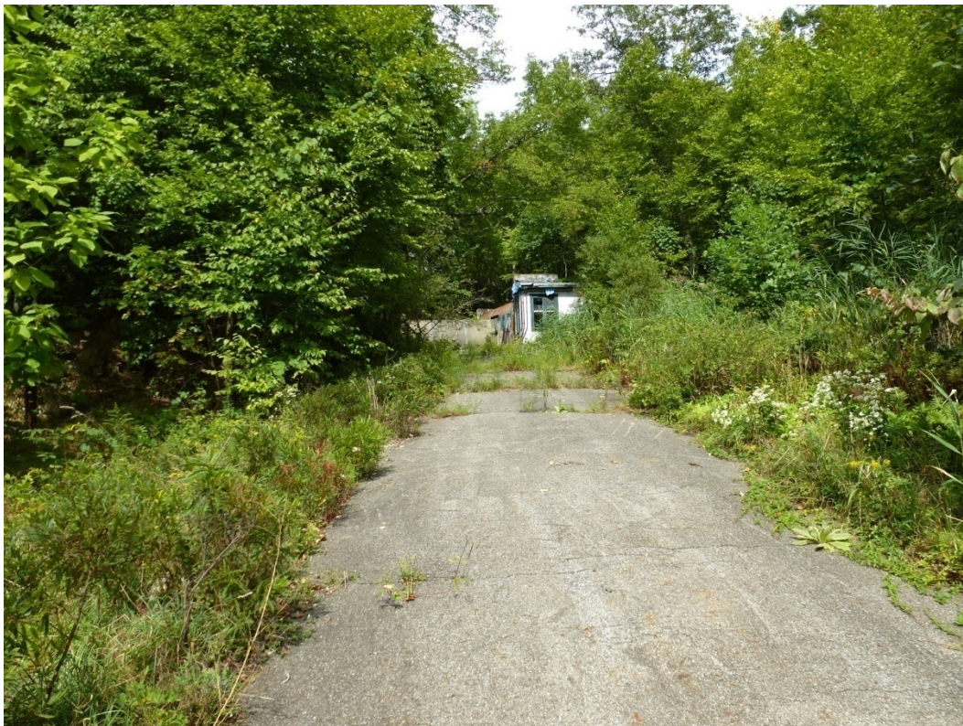
Figure 177. Looking north towards Building 611B (ERDC-CERL, 2012).
