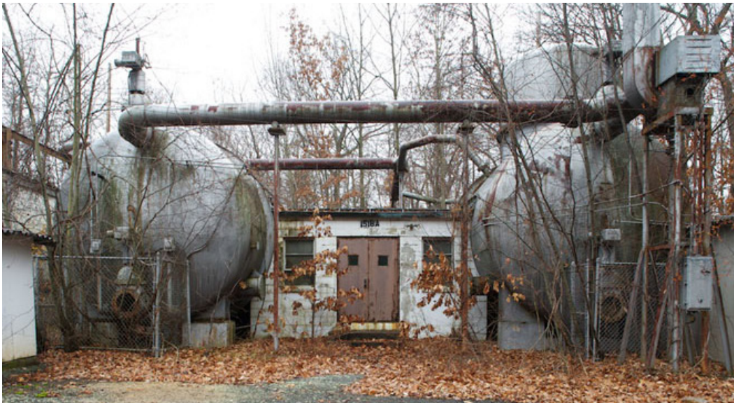
Figure 262. Building 1518, now demolished, connected Chambers #1 and #2 with Building 1517A in the middle (PICA Cultural Resources Office, 2011).
