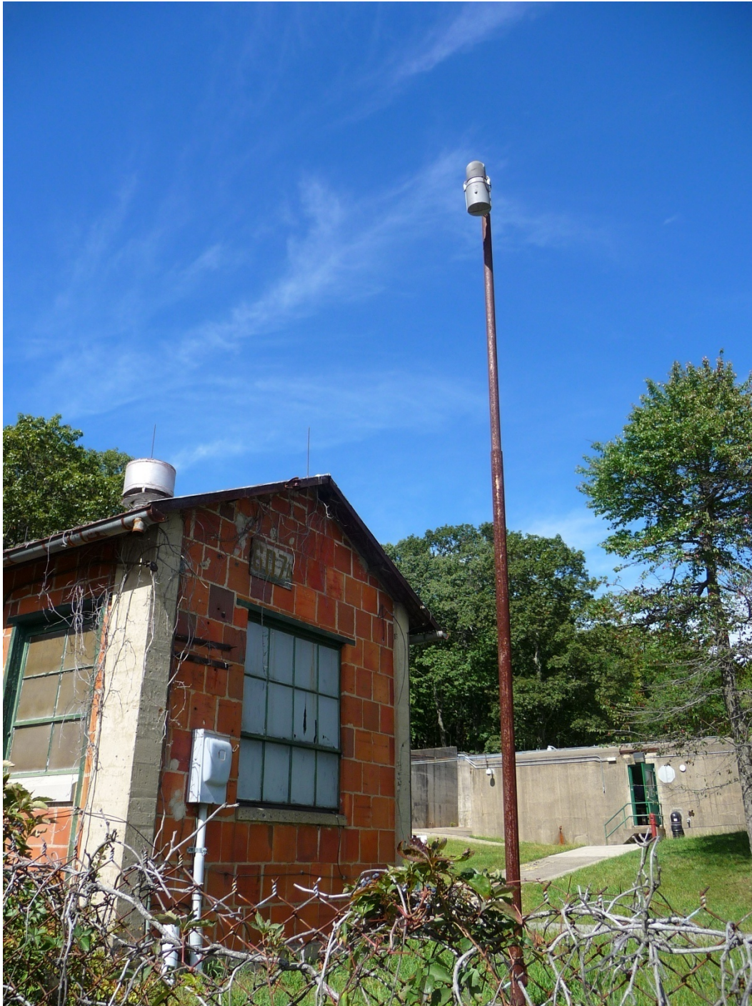
Figure 215. Large lightning rod adjacent to Building 607A (ERDC-CERL, 2012).
