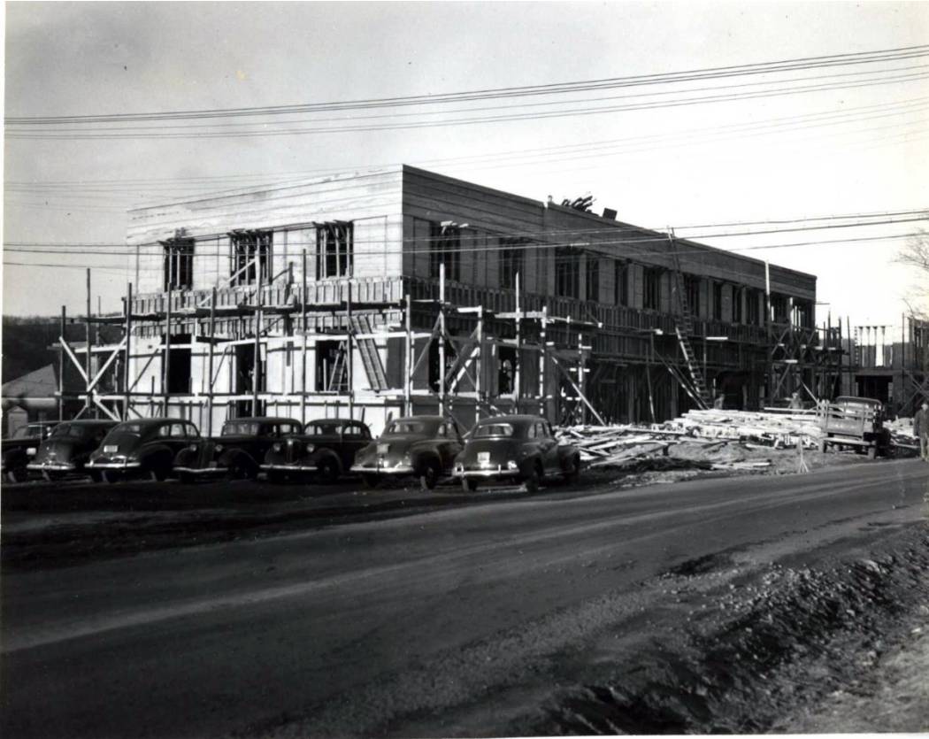
Figure 18. Construction of Building 173, 1942 (PICA Cultural Resources Office).
