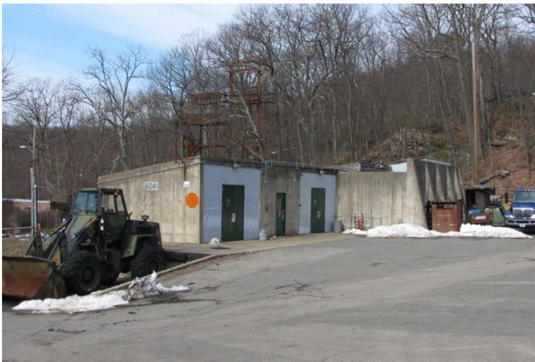
Figure 190. North elevation of Building 604C, Sectioning Chamber; drop-tower is visible behind it (PICA Cultural Resources Office, 2011).
