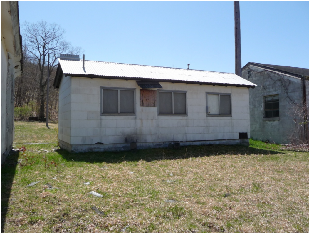
Figure 305. North elevation of Building 3613, NARTS Area D Lunch Room (ERDC-CERL, 2013).
