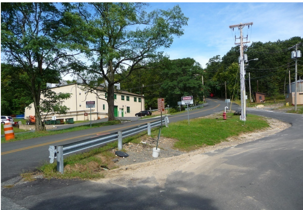
Figure 176. View looking north on 20th Avenue; Building 611 is on the left (ERDC-CERL, 2012).
