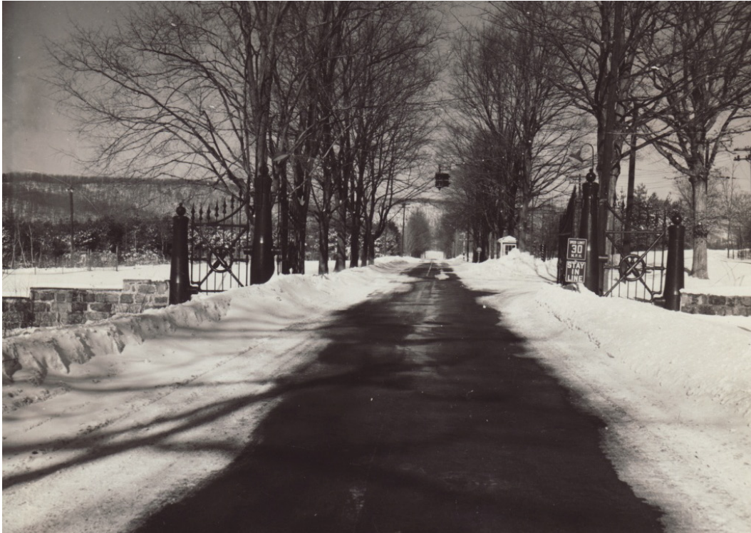
Figure 110. View toward Cannon Gates, 1940s (PICA Cultural Resources Office).
