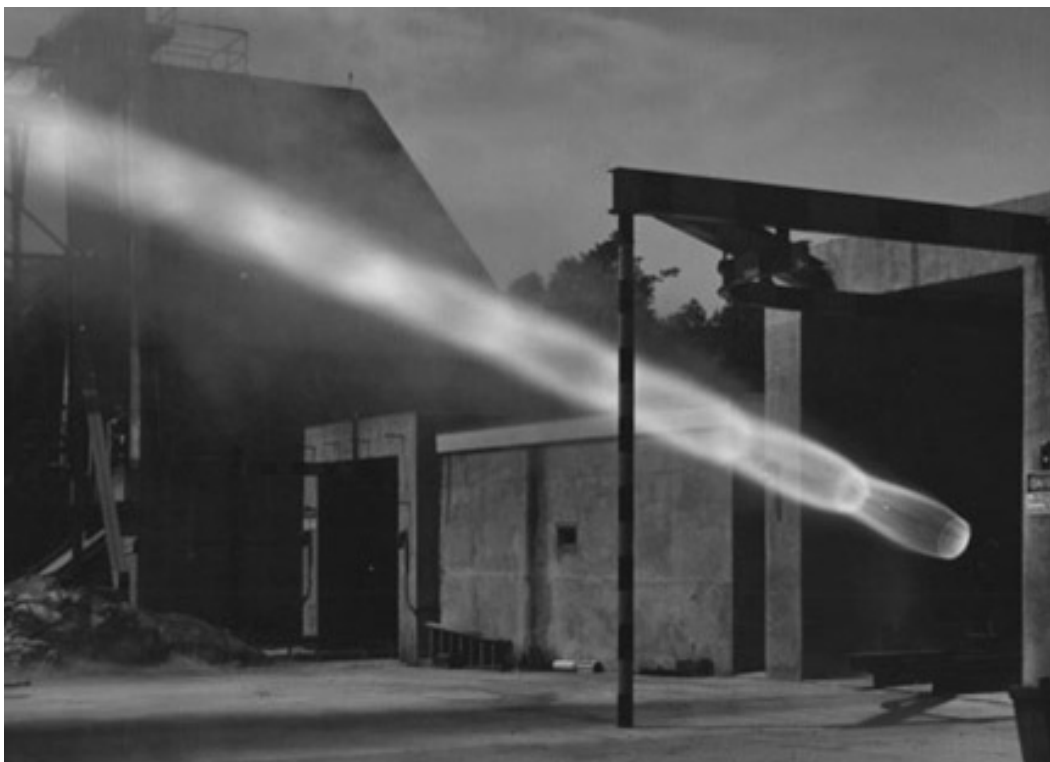
Figure 284. Historic photograph of rocket motor tests at Building 3606, no date (PICA Cultural Resources Office).
