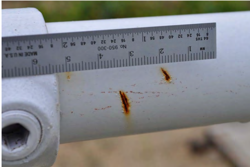
Figure B4. Coated Steel Railing
