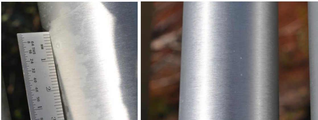
Figure 32. Aluminum railing coupon at FRF (left) and KTA (right) after 6 months of exposure.
