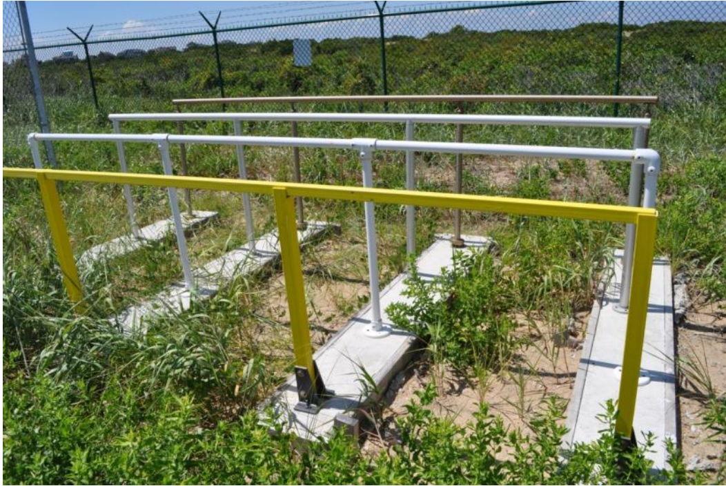
Figure 8. Railing test sections installed at the FRF.
