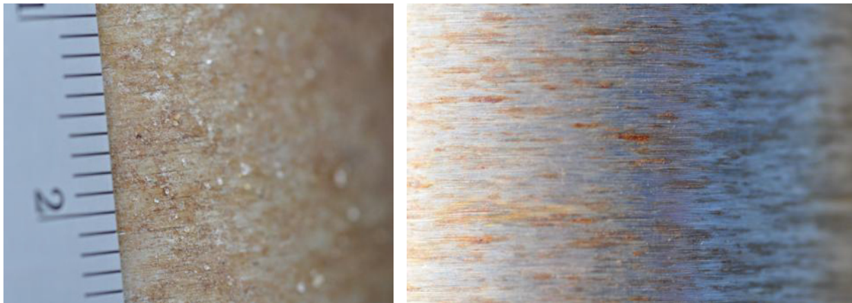
Figure 35. Stainless steel railing coupon at FRF (left) and KTA (right) after 12 months of exposure.
