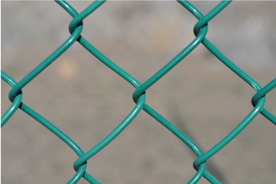
Figure A7. Fuse-bonded PVC after 6 months exposure.
