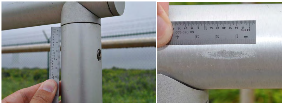
Figure B8. Fabricated Aluminum Railing
