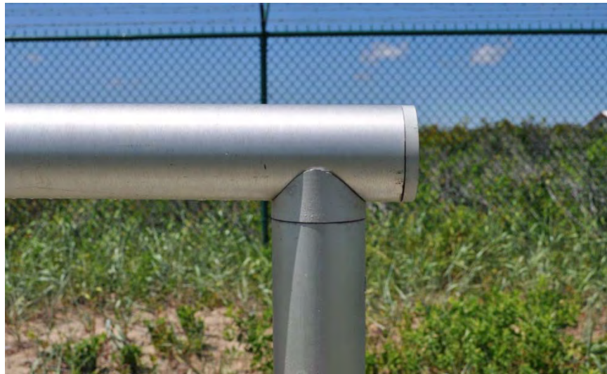
Figure B28. Fabricated Aluminum Railing
