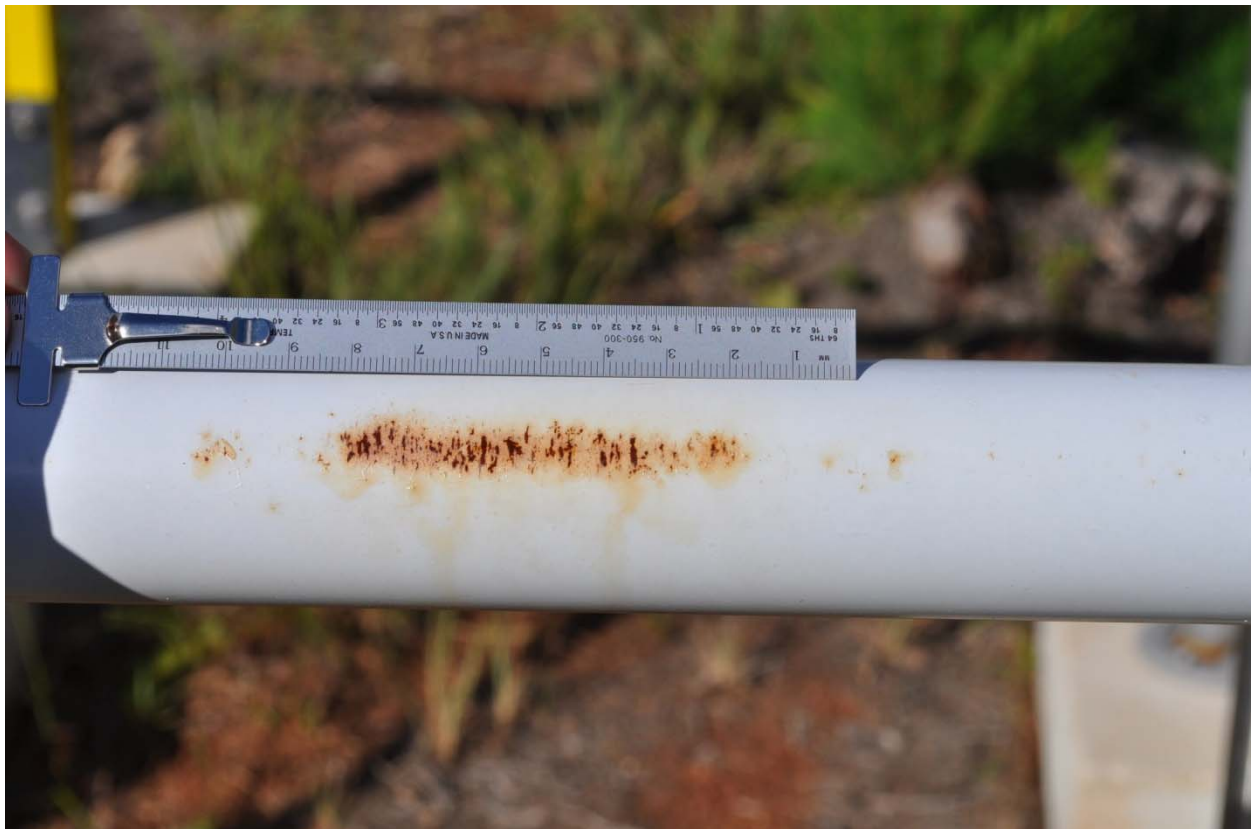
Figure B80. Coated Steel Railing
