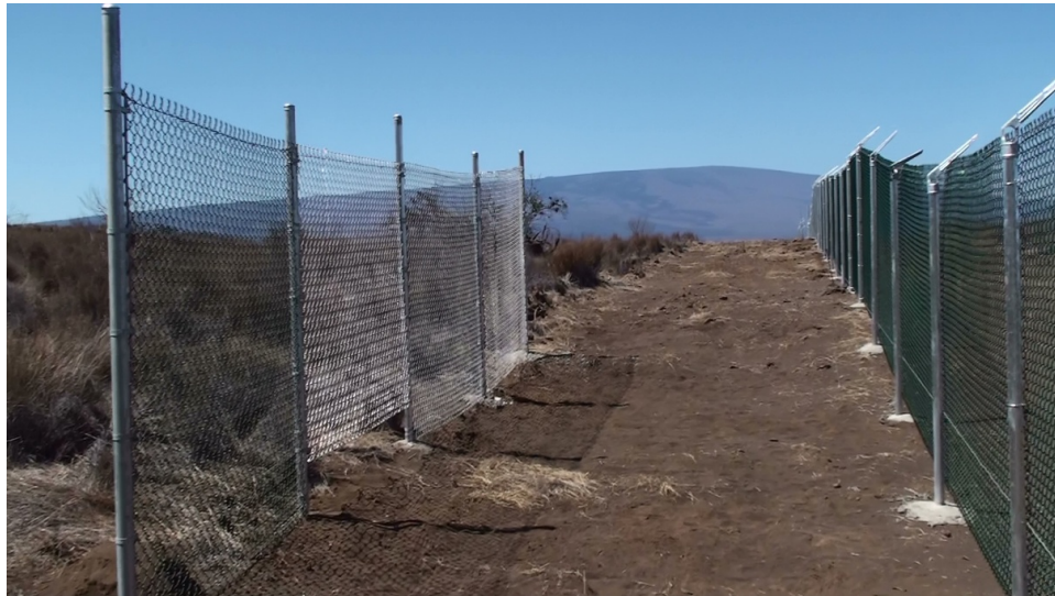
Figure A3. Fuse-bonded PVC fencing at west BAA perimeter from Old Saddle Road to New Saddle Road (right) and four test sections of control materials (left).
