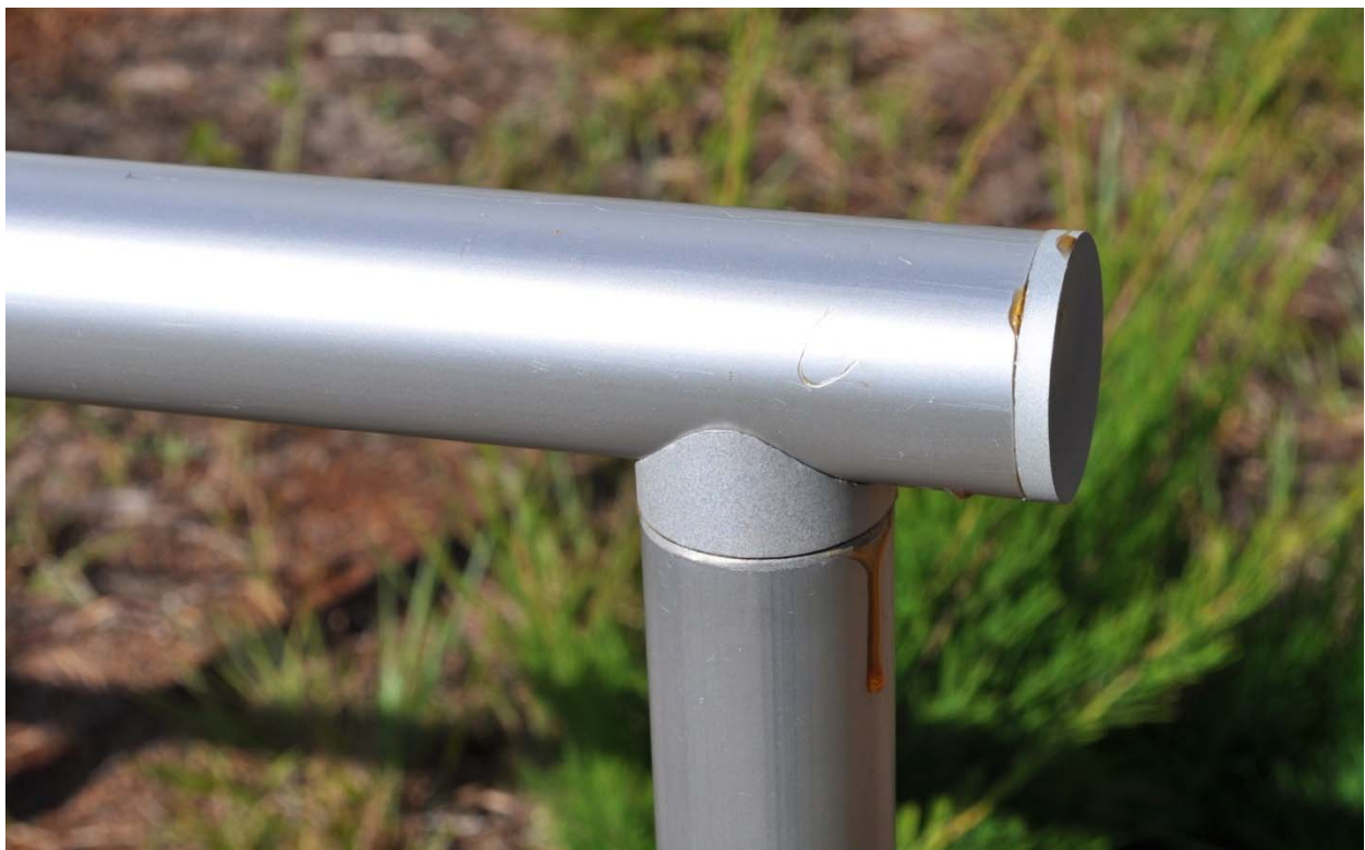
Figure B84. Fabricated Aluminum Railing
