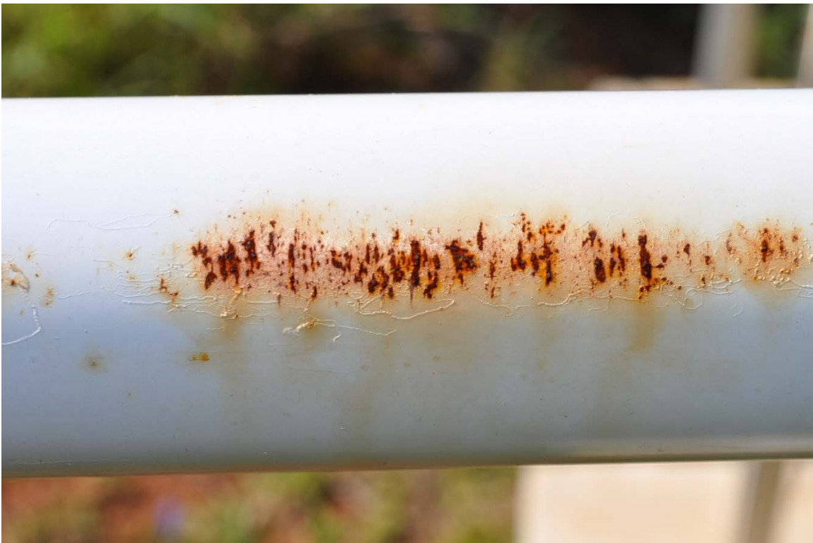
Figure B120. Coated Steel Railing
