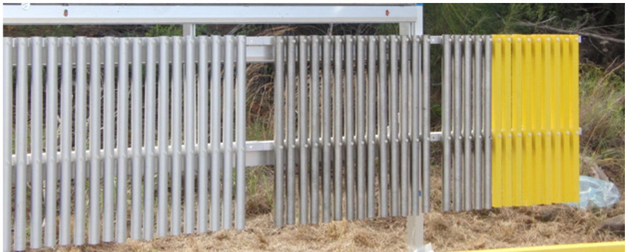
Figure 10. Railing and wire coupons installed on an ASTM G7 exposure rack placed at 45 degree angle at the FRF.
