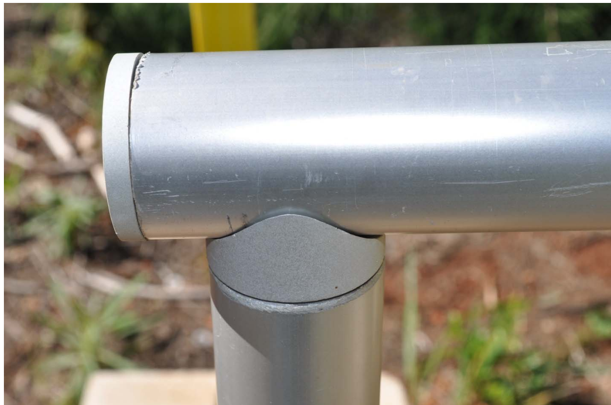
Figure B124. Fabricated Aluminum Railing
