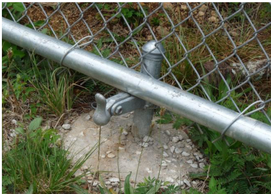
Figure 6. Position-locking hardware for vehicle gates.
