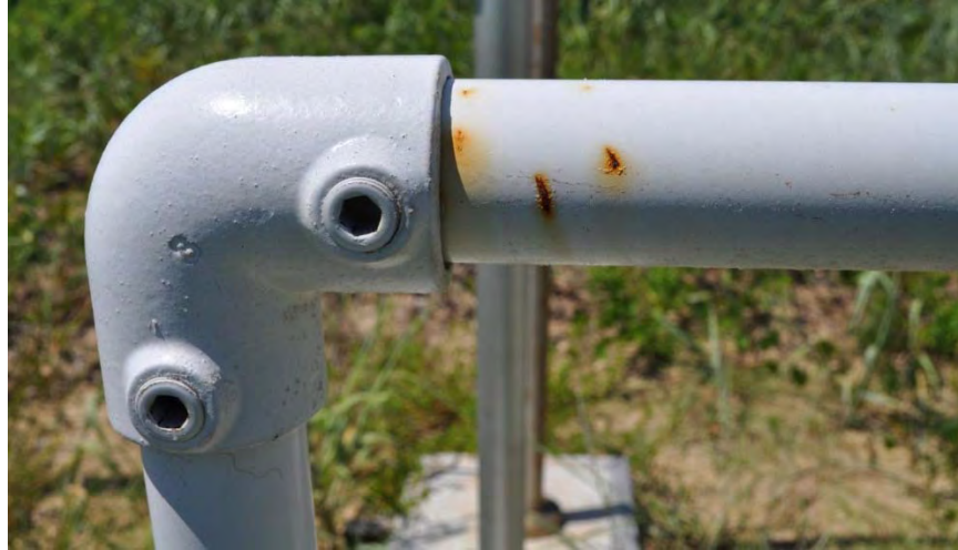
Figure B24. Coated Steel Railing
