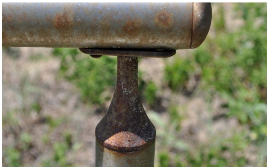
Figure B26. Stainless Steel T-fittings on fabricated railings
