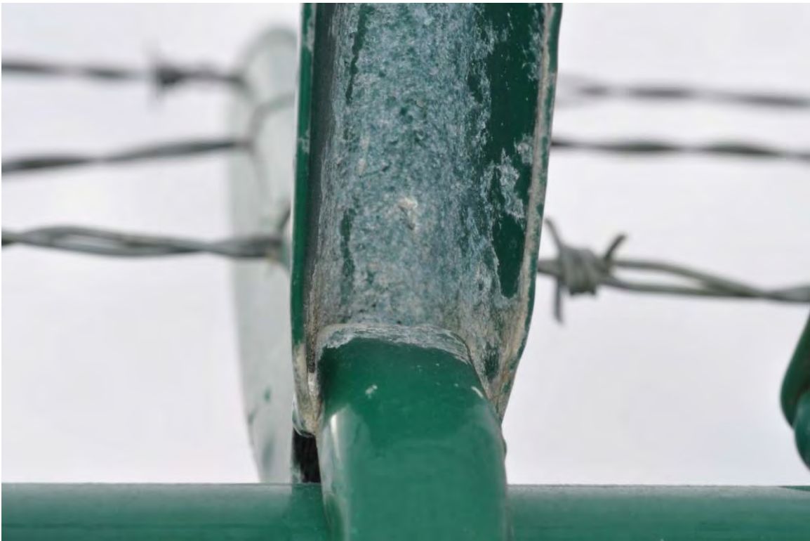
Figure B63. Fuse Bonded PVC Coated Galvanized Wire Fencing Hardware
