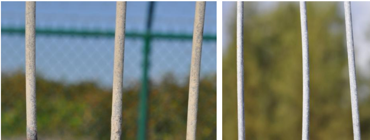
Figure 21. Galvan wire coupon at FRF (left) and KTA (right) after 6 months of exposure
