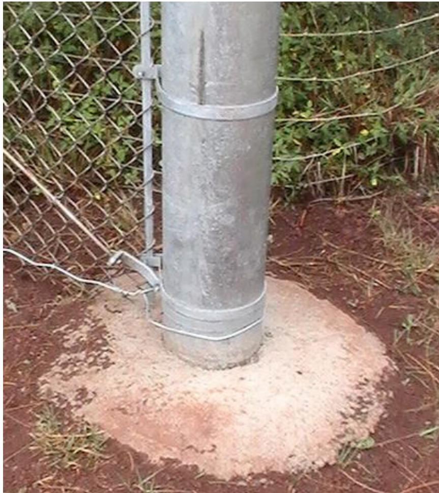
Figure 5. Fencing pole anchored in concrete.
