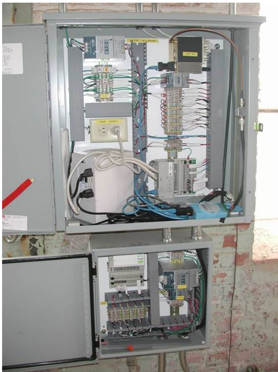
Figure 11. Typical SCADA box at Fort Bragg.
