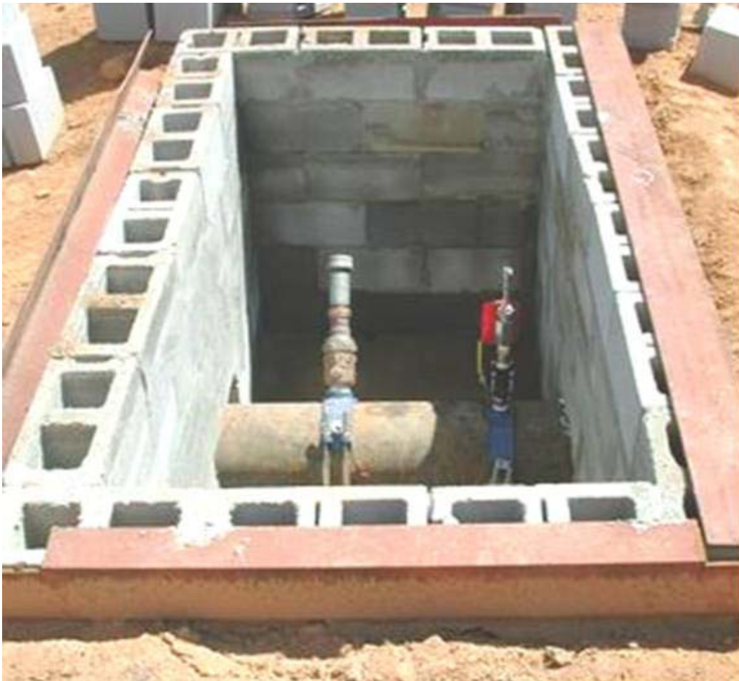
Figure 9. Corrosion sensor in new vault at Tank Hill.
