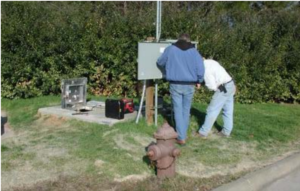
Figure 7. New vault and SCADA box at Simmons Army Airfield
