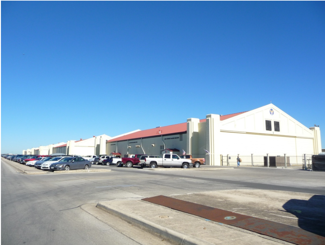
Figure 50. Row of hangars, 2012 (ERDC-CERL).
