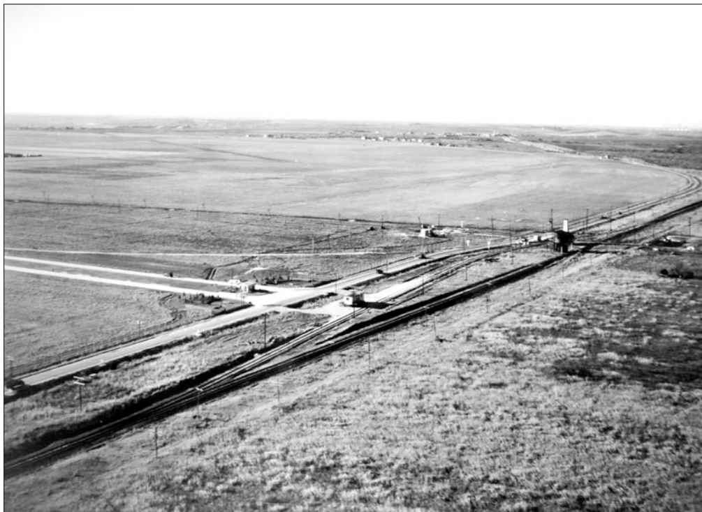
Figure 33. Main entrance to Randolph Field during the 1930s showing the Old Seguin Road and the Southern Pacific Railroad (Norfleet Giddings Bone Papers, University of Texas at San Antonio Libraries Special Collections).
