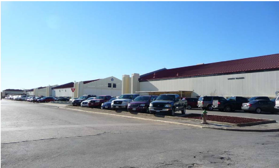
Figure 198. Loss of grassed area, sidewalks, and trees between roads and hangars, 2012 (ERDC-CERL).
