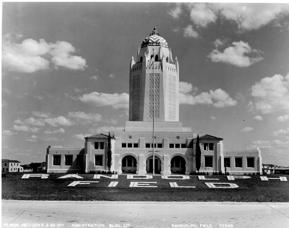
Figure 30. The highly ornamented and visually distinct Administration Building, also known as the Taj Mahal (Bone Collection Randolph AFB Cultural Resources).
