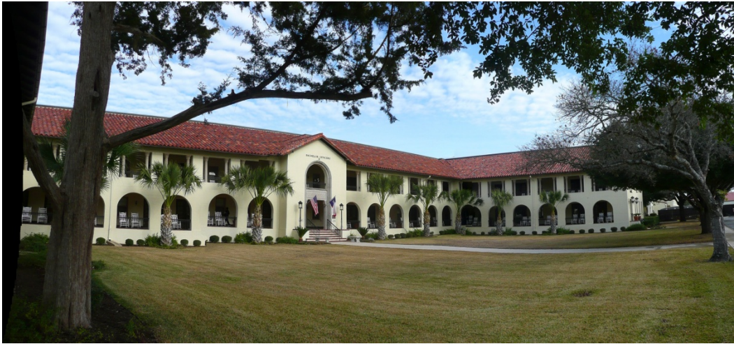
Figure 100. South elevation of the BOQ, 2012 (ERDC-CERL).
