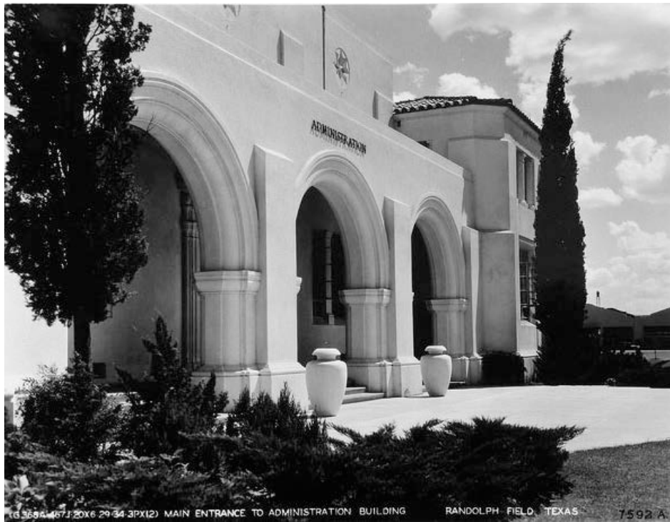
Figure 120. Main entrance to the Administration Building showing the elaborate planting patterns most likely designed by Lt. Bone, undated (NARA RG342 Box1072 B20821).
