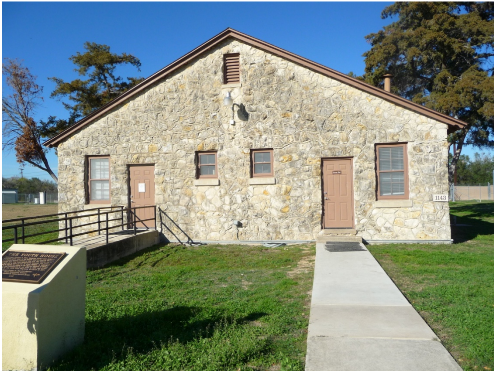
Figure 193. The Youth House plaque in association with the WPA building, 2012 (ERDC-CERL).
