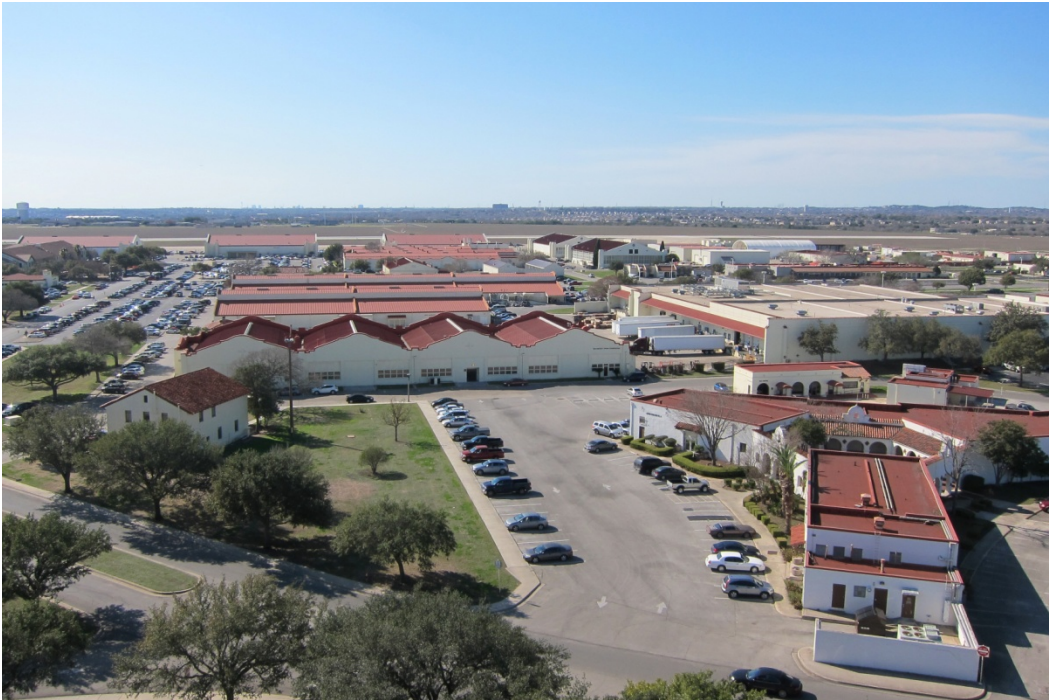
Figure 48. The warehouse and shop area conveys the same visual aesthetics as the rest of the base, 2012 (ERDC-CERL).
