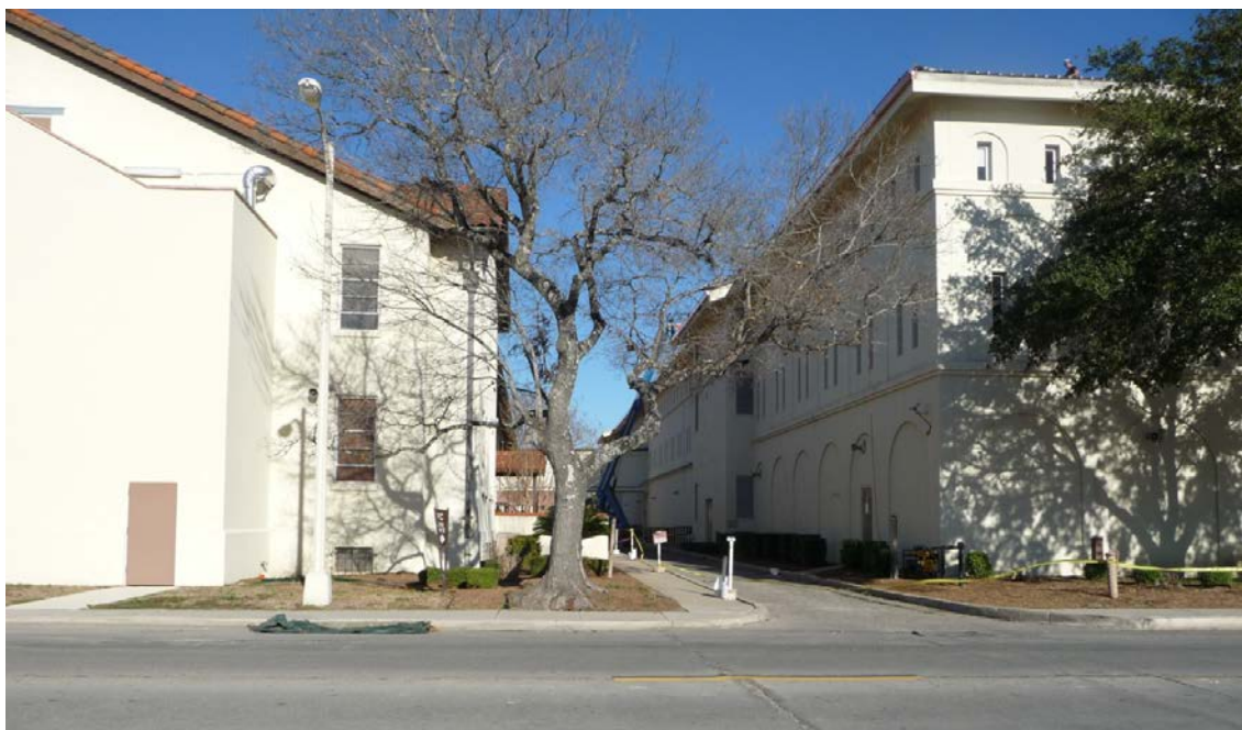
Figure 199. Enlisted men's barracks on the west side, 2012 (ERDC-CERL).
