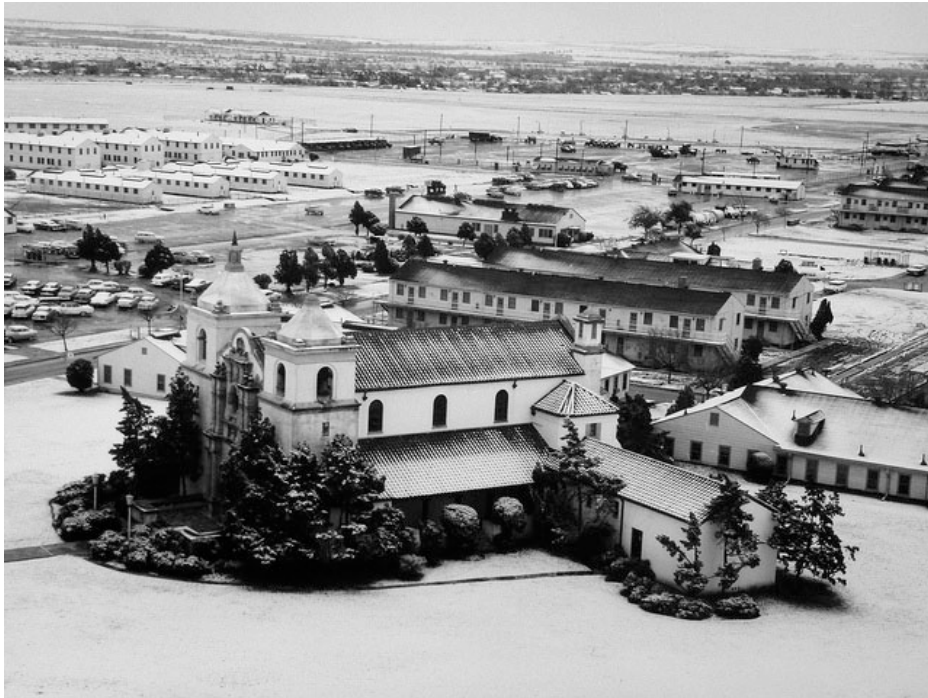
Figure 124. The chapel was another important area in the base. By the 1950s, the front of the chapel had been elaborately landscaped with a variety of evergreen shrubs and small trees, 1958 (NARA RG342 Box 300).
