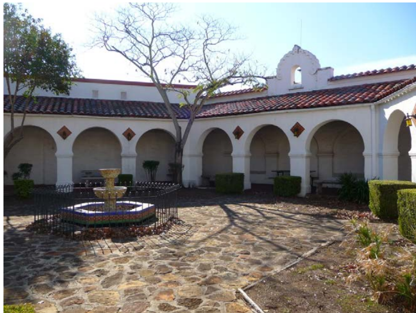
Figure 130. The current planting design of the PX courtyard consists of boxwood hedges pruned into cubes and a few ornamental trees, 2012 (ERDC-CERL).
