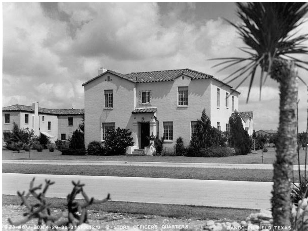
Figure 75. Another of Marriot's two variations on two-story officers' quarters, showing the squared-door surround, with tile-decorated window above, 1930s (NARA RG342 Box 1072 B20755).
