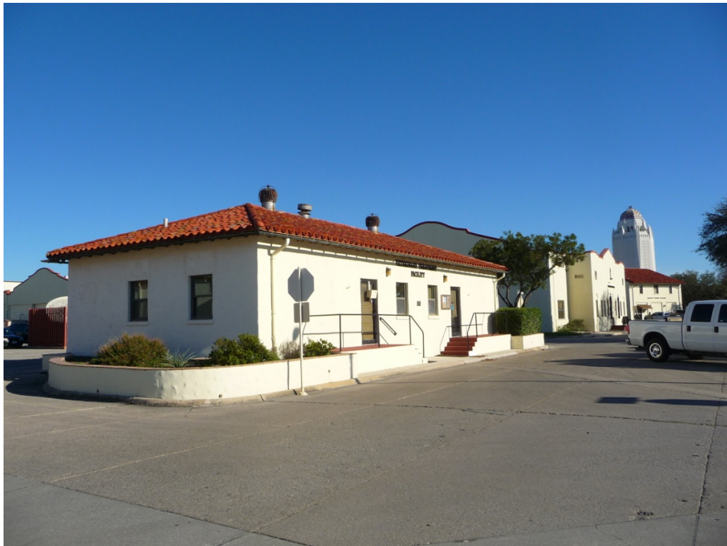
Figure 135. The planters that were incorporated onto the east and west sides of this building now have a few scattered species on one side and box hedges on the other, 2012 (ERDC-CERL).
