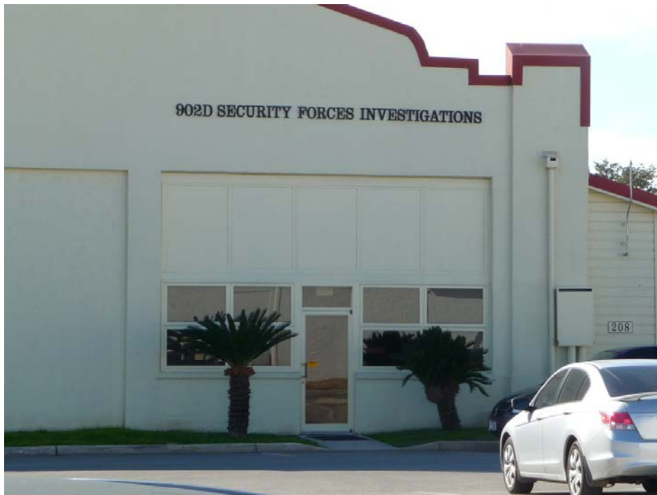
Figure 133. Two palms placed on either side of an entrance to one of the former warehouses, 2012 (ERDC-CERL).
