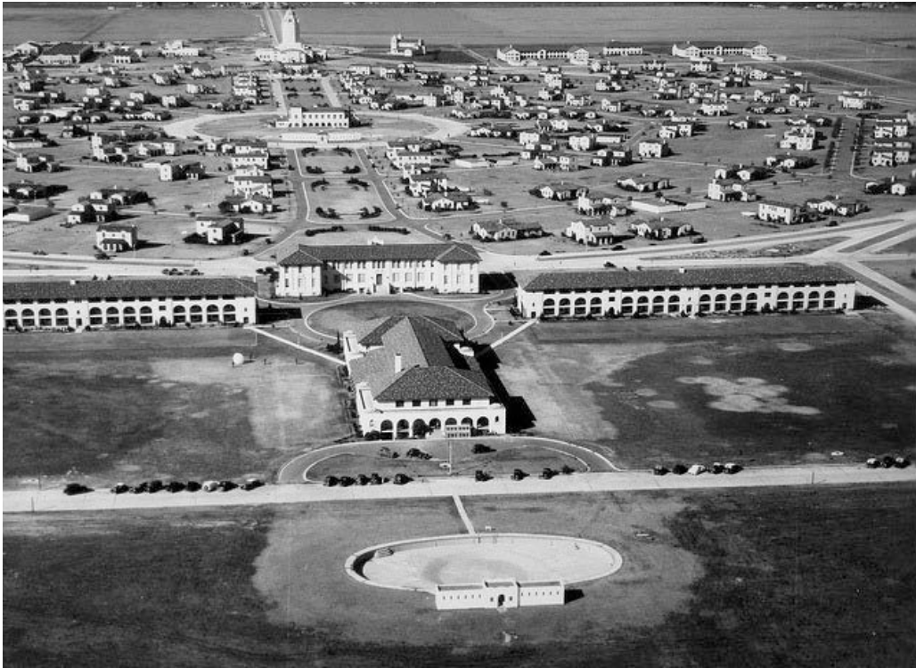
Figure 55. Cadet Complex during construction in the 1930s, before the additional barracks were added (NARA RG342 Box 1071 B20695).
