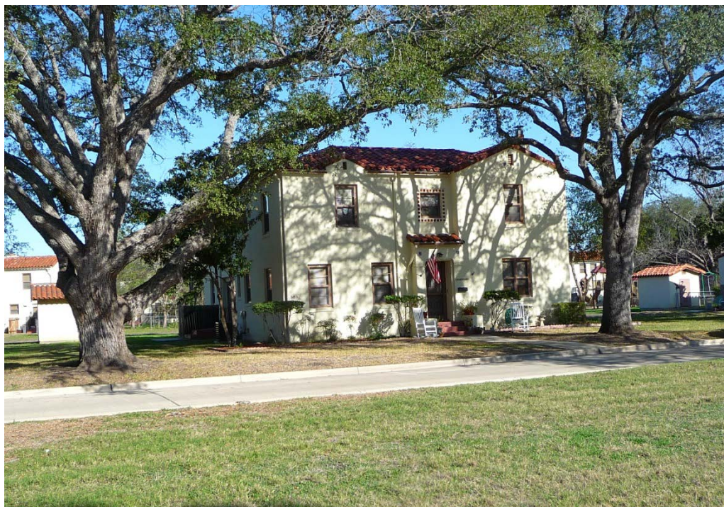
Figure 76. Another current example of Marriot's variation of two-story officers' quarters, with squared-door surround and tile-decorated window above, 2012 (ERDC-CERL).
