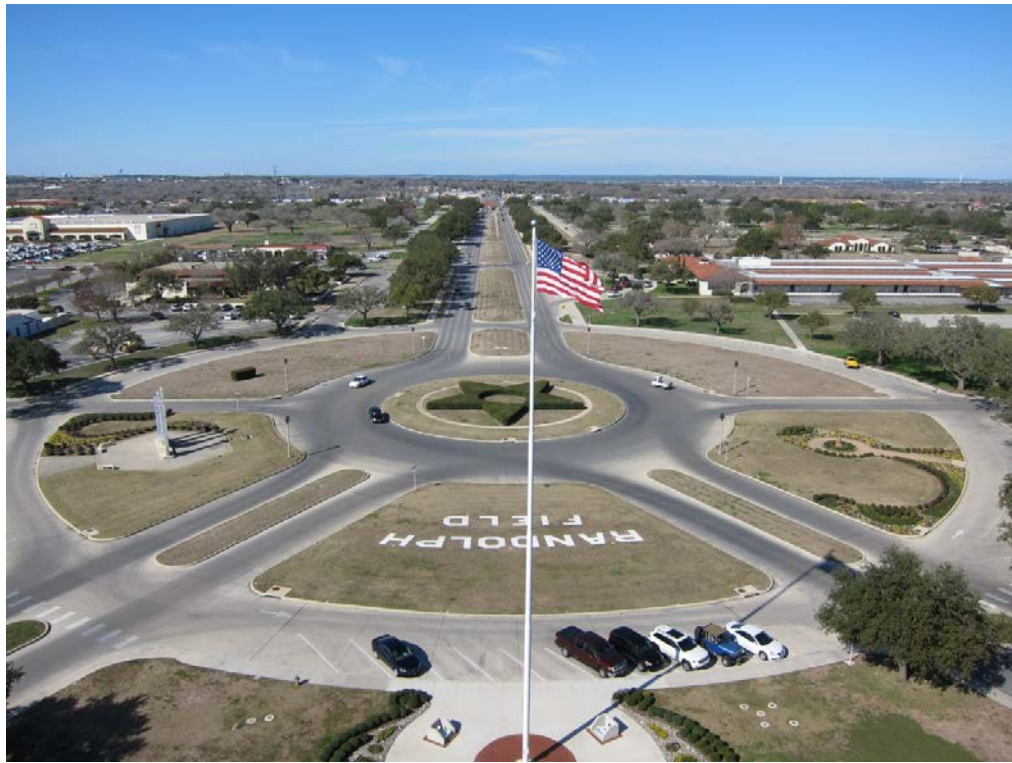
Figure 31. View from the Taj Mahal toward the main entrance. The base flagpole is located north of the Administration Building, on axis with the main entrance, 2012 (ERDC-CERL).
