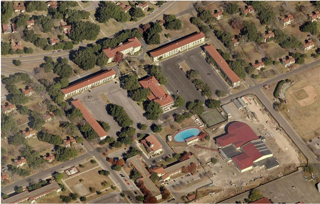
Figure 57. Aerial view of the former Cadet Complex, 2012 (bing.com/maps).
