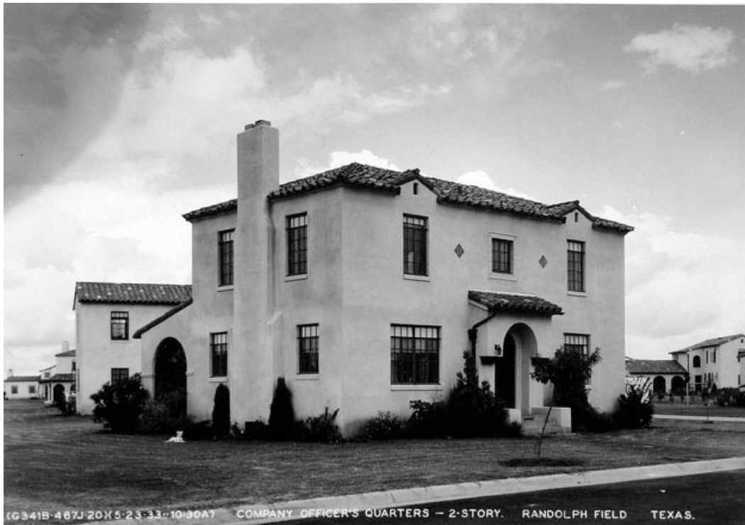
Figure 73. One of Marriot's variations of the two-story officers' quarters had an arched door surround, 1930s (NARA RG342 Box 1072 B20784).
