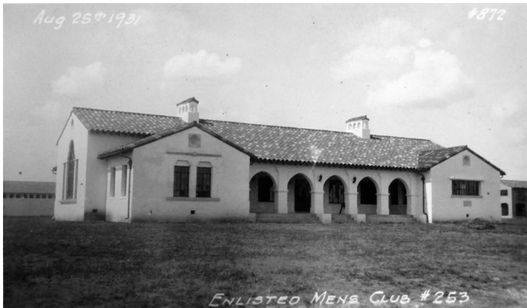
Figure 93. Exterior of the western enlisted men's club in 1931 (then designated as Building #253), (Norfleet Giddings Bone Papers, University of Texas at San Antonio Libraries Special Collections).
