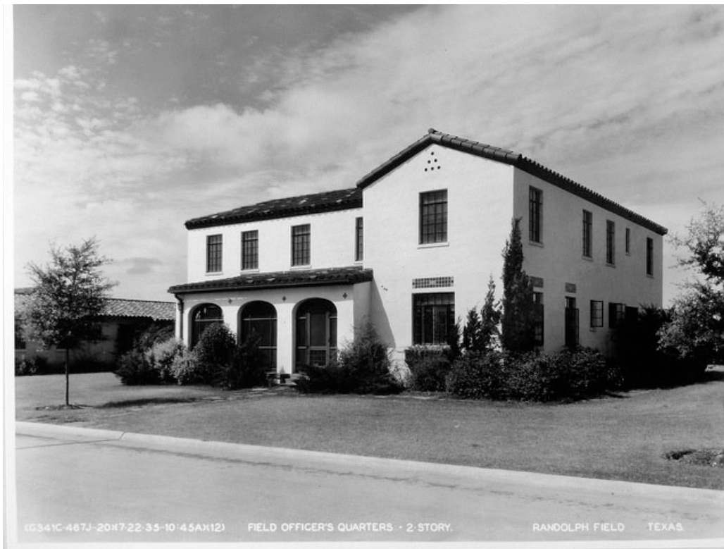
Figure 79. An example of one of the variations on the two-story officers' quarters in the 1930s (NARA RG342 Box 1072 B20783).
