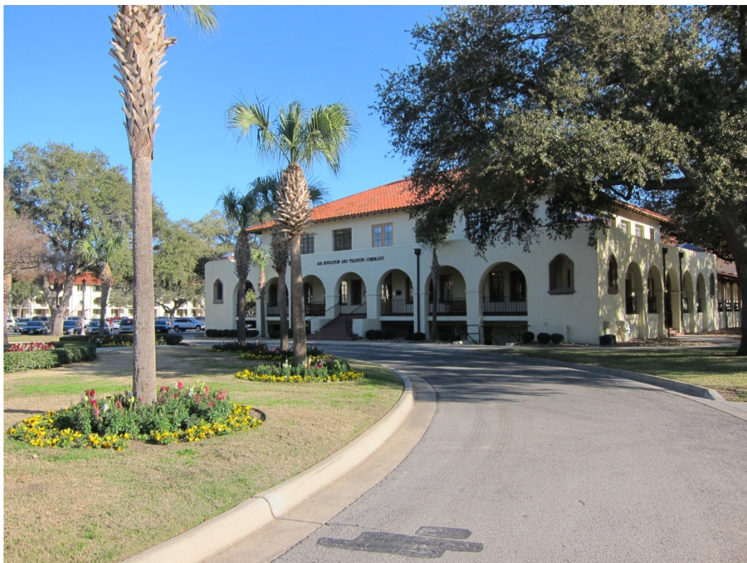
Figure 61. The former Cadet Administration Building, 2012 (ERDC-CERL).
