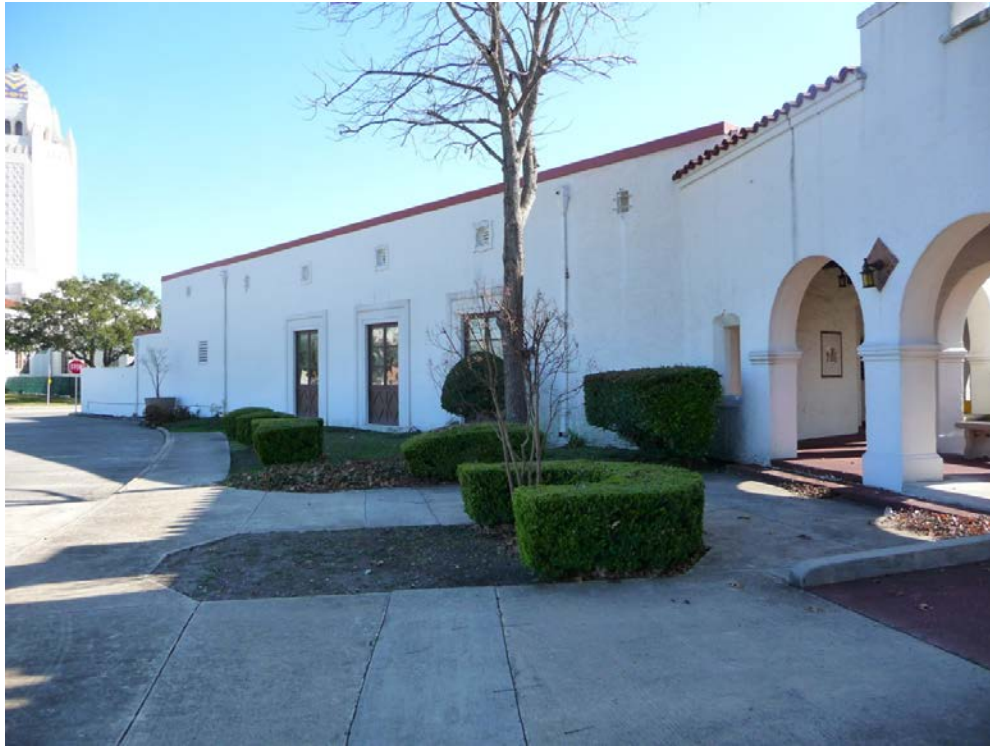
Figure 127. One of the entrances to the former PX courtyard, 2012 (ERDC-CERL).
