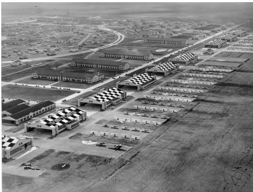
Figure 4. Aerial view of the hangars and aprons on the west flight line, undated but soon after construction, undated (NARA RG 342 Box 1071 B20672).
