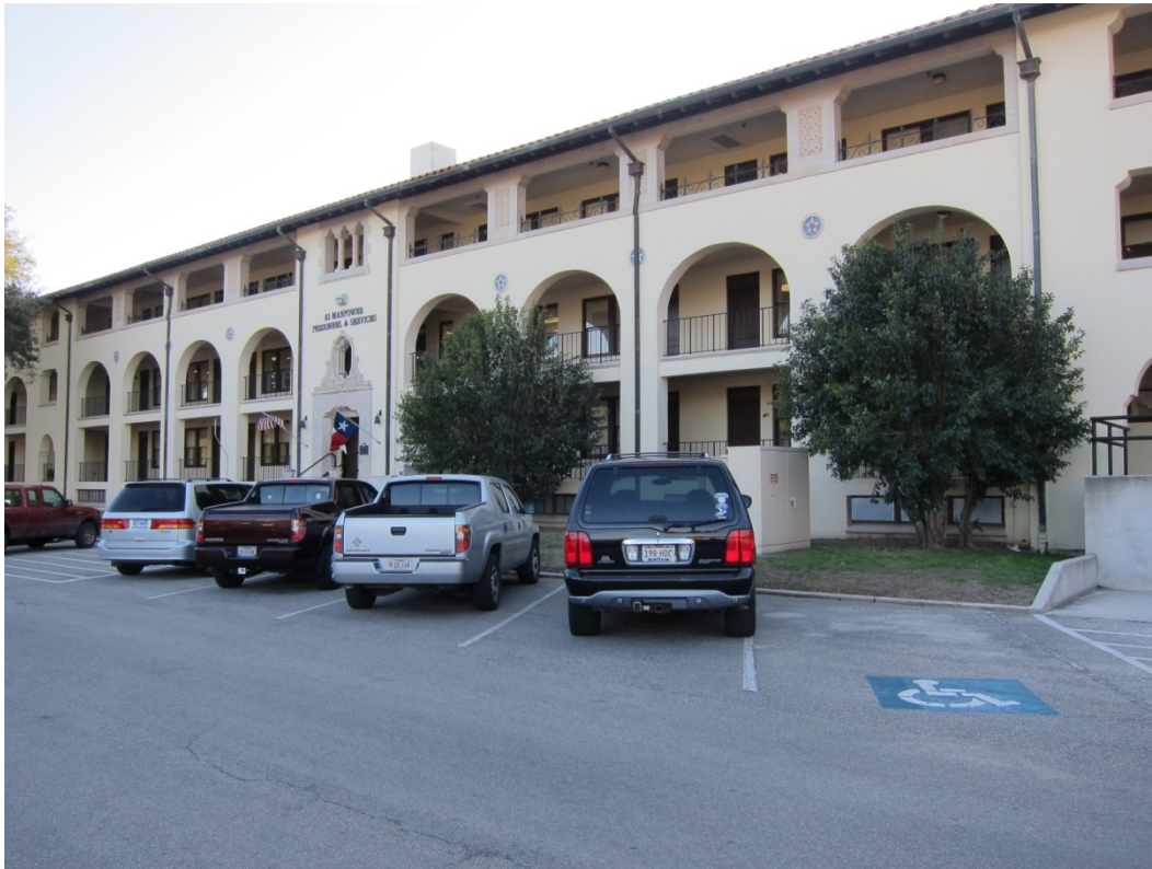
Figure 63. Cadet Complex Barracks, now converted to offices, 2012 (ERDC-CERL).
