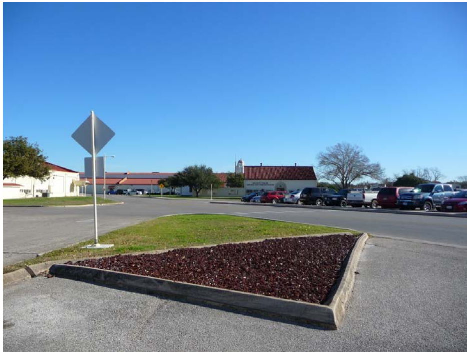
Figure 114. Because of the intricate circular road network, there are many dividers and medians throughout the base. The extensive planting strategies of Lt. Bone had many of these small spaces planted. Maintenance on these spaces has been gradually reduced to mowing grass or, as this image shows, being filled with no-maintenance lava rocks, 2012 (ERDC-CERL).
