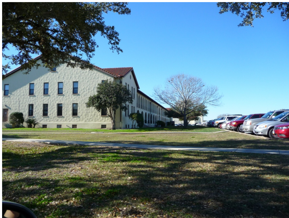
Figure 150. The current plantings around the former enlisted men's barracks buildings are unified in a cohesive design. Many ornamental plants stand alone or are part of broken hedges, 2012 (ERDC-CERL).
