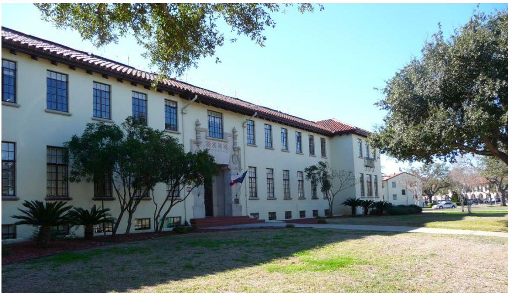
Figure 68. The former School of Aviation Medicine building, 2012 (ERDC-CERL).
