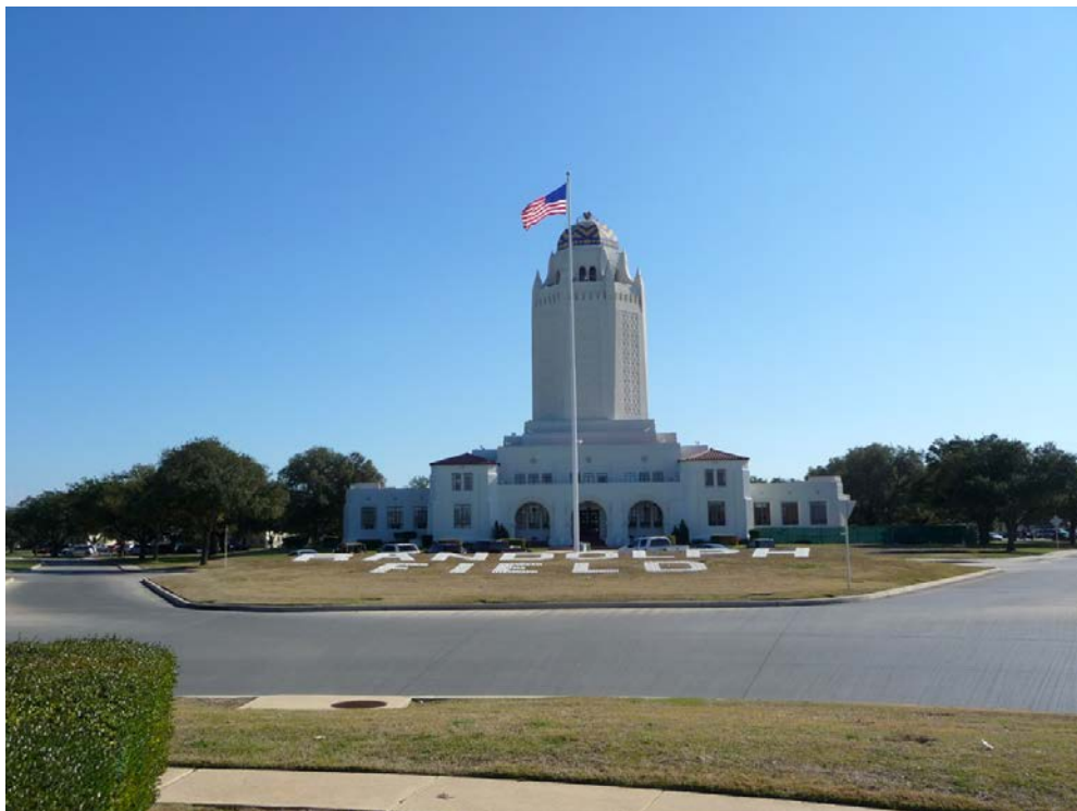
Figure 122. The “Taj Mahal” in 2012. The north façade plantings have again changed. The entrance between the hedge row has been widened and a few evergreens have been planted on either side of the arched entrance, 2012 (ERDC-CERL).
