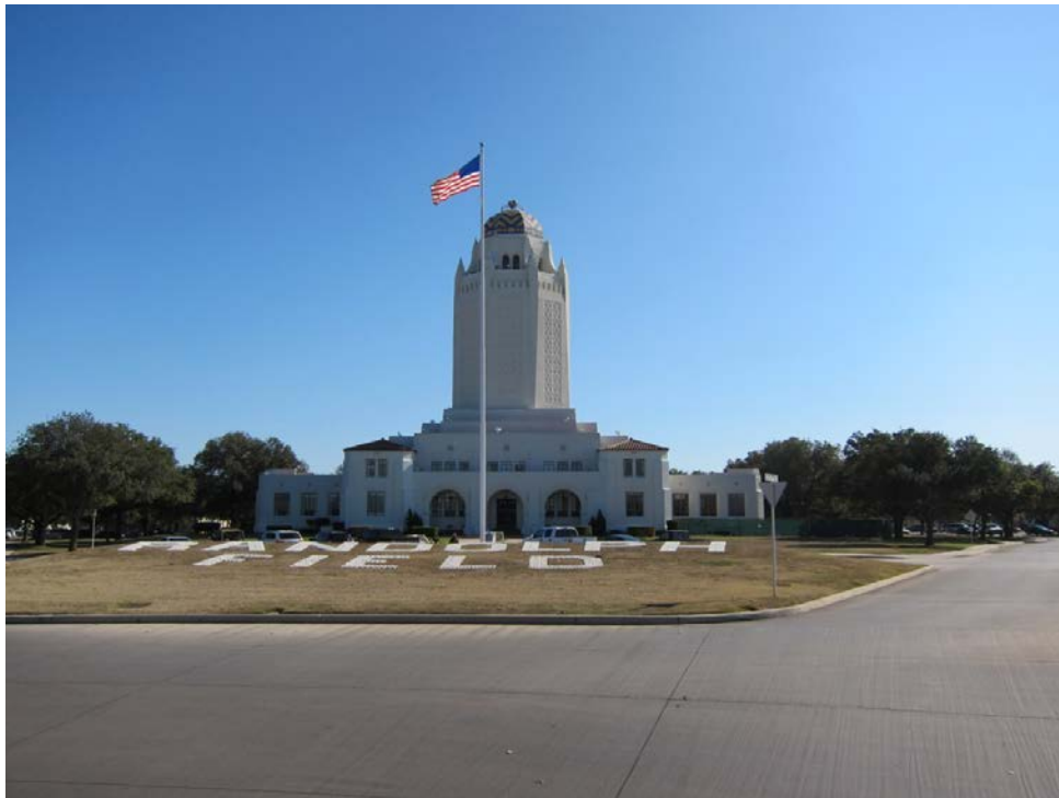
Figure 165. Flagpole and Randolph Field sign in front of the Taj Mahal, 2012 (ERDC-CERL).
