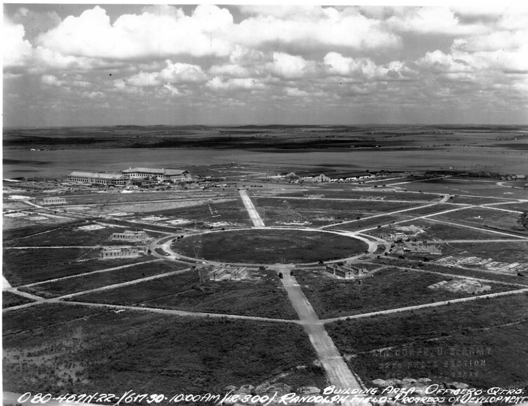
Figure 3. The road system was laid out and constructed by 1929, before building construction started, 1930 (University of Texas San Antonio, Norfleet Giddings Bone Papers).
