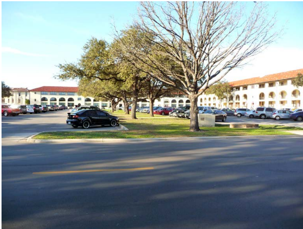
Figure 153. The Cadet Complex barracks were originally surrounded by open green spaces, but by the 1940s parking lots had been introduced along the barracks while retaining some of the original green space. By 2012, the east and west spaces between the buildings has been converted to parking lots with a strip of open space and a few trees, 2012 (ERDC-CERL).
