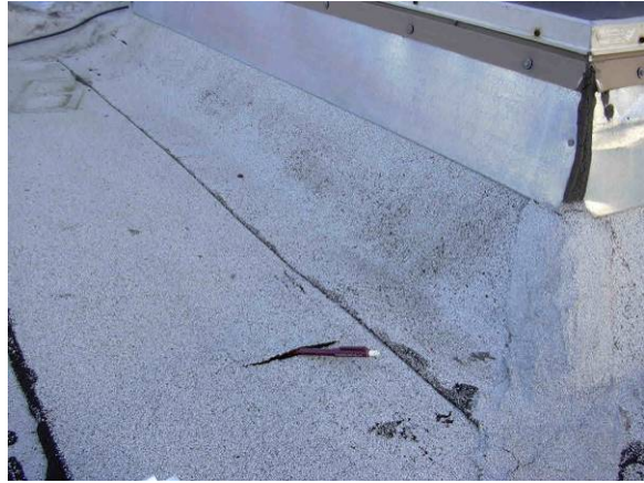
HL-H-1: All holes are considered high severity due to their high leak potential.
