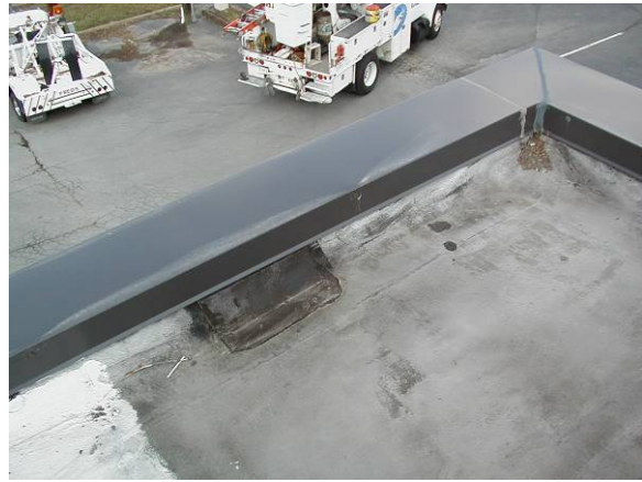
BF-L-3: Flashing has permanent repairs.
