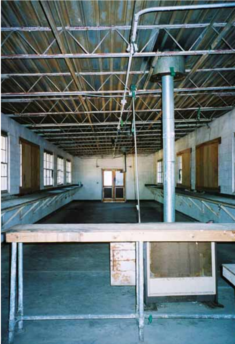
Figure 350. 1966 Bldg 427 range mess hall interior, Fort Gordon, GA, January 2004.
