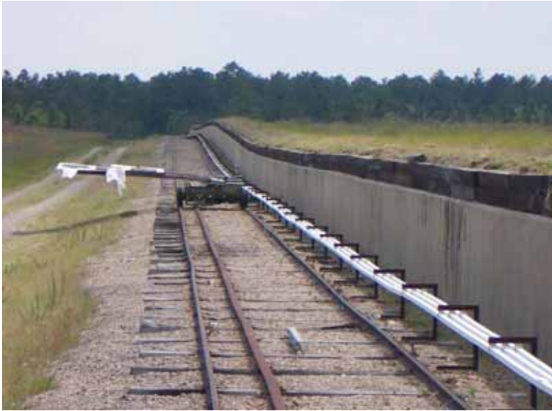
Figure 301. Pop-up target mounted on a dolly moving along a target track protected by an embankment, Fort Bragg, 17 May 2006.
