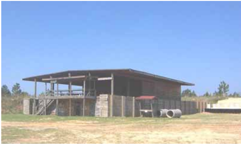
Figure 354. Range firing tower, Fort Bragg, 17 May 2006.
