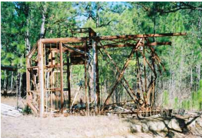
Figure 314. Remains of 1966 observation tower (near Bldg421), Fort Gordon, GA, July 2004.
