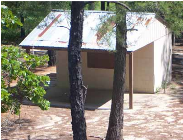
Figure 336. Range ammunition storage building, Fort Bragg, 17 May 2006.
