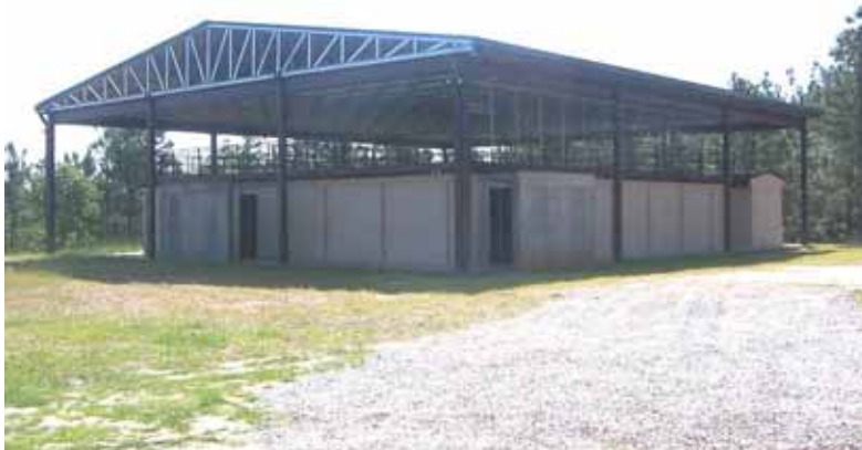
Figure 355. Range firing tower, Fort Bragg, 17 May 2006.
