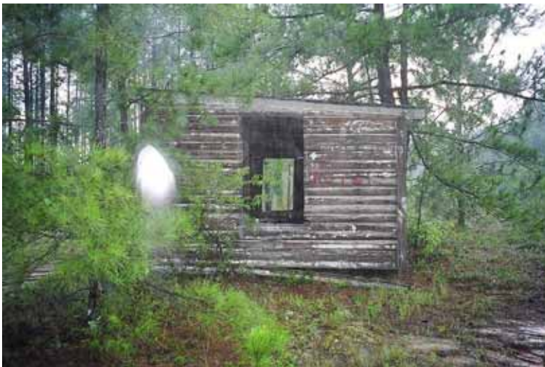
Figure 324. Remains of WWII range target shed Bldg R161, Fort Gordon, GA, January 2004.
