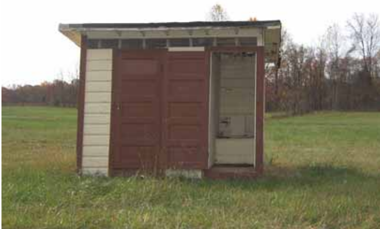
Figure 339. Remains of WWII latrine Bldg 9347, Fort Knox, KY, November 2005.
