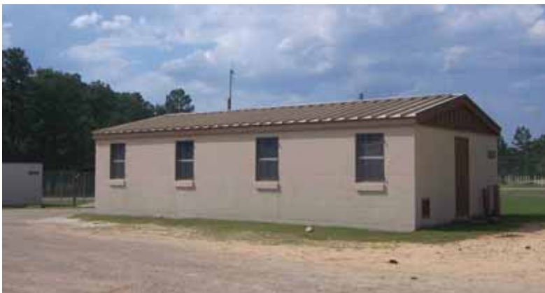
Figure 328. Range storage building, Fort Bragg, 17 May 2006.
