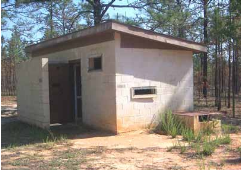
Figure 343. Range latrine, Fort Bragg, 17 May 2006.
