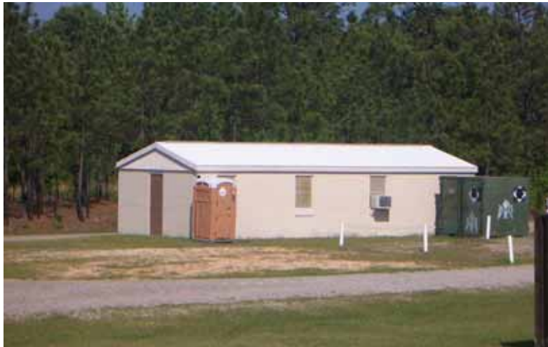
Figure 329. Range storage building, Fort Bragg, 17 May 2006.
