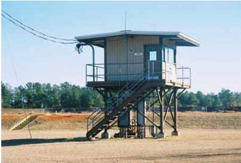
Figure 315. 1987 range building 486, Fort Gordon, GA, January 2004.
