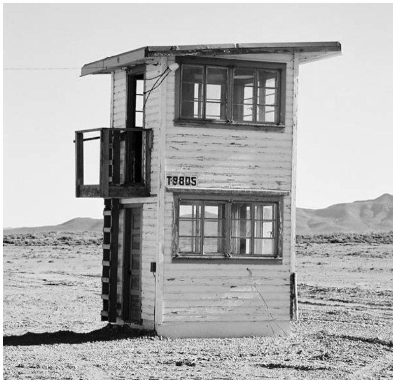
Figure 305. WWII observation tower Bldg 9805, Fort Bliss, TX, November 2005.
