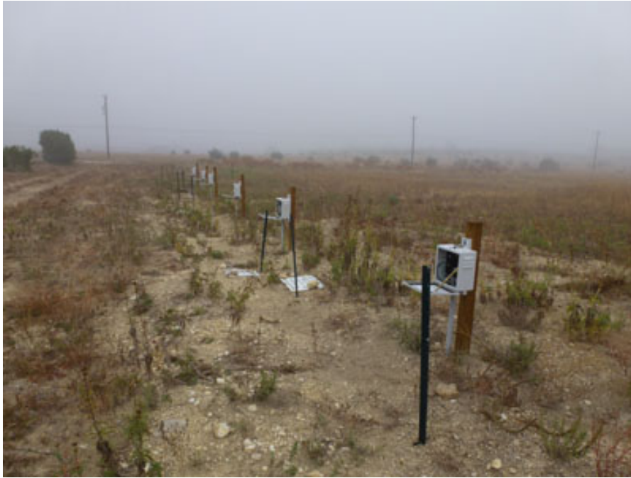
Figure 3. Overall view of the test terminal boxes for the six pipe sections.
