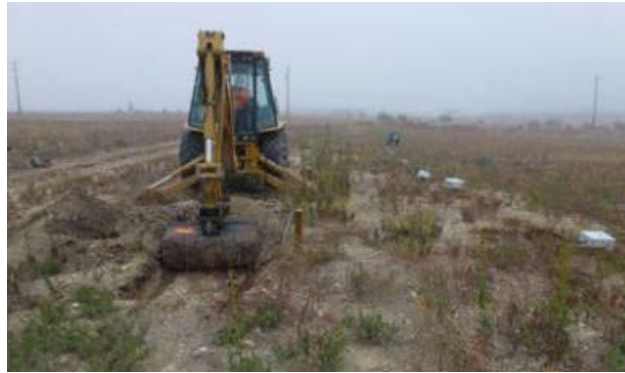
Figure 7. Excavation of pipe test sections after 13 months exposure in flowable fill.
