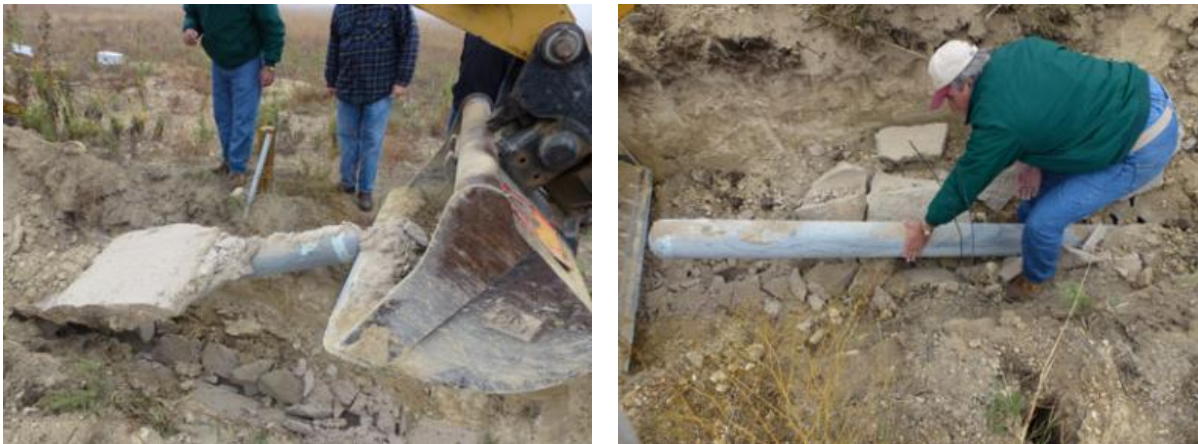
Figure 8. Removal of alternative fills and initial pipe inspection after excavation.
