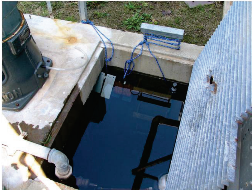
Figure 14. Test panel rack suspended from far edge of sump.
