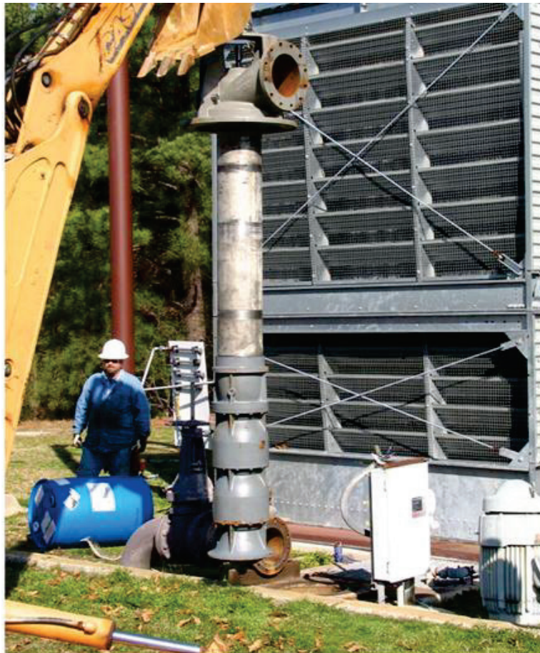
Figure 13. New pump 5 being installed.
