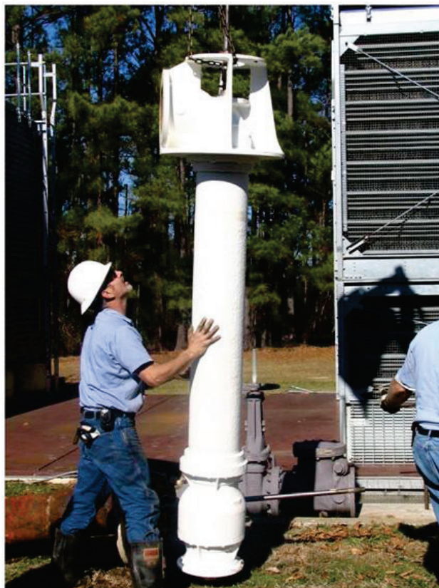
Figure 11. Pump 4 being reinstalled.
