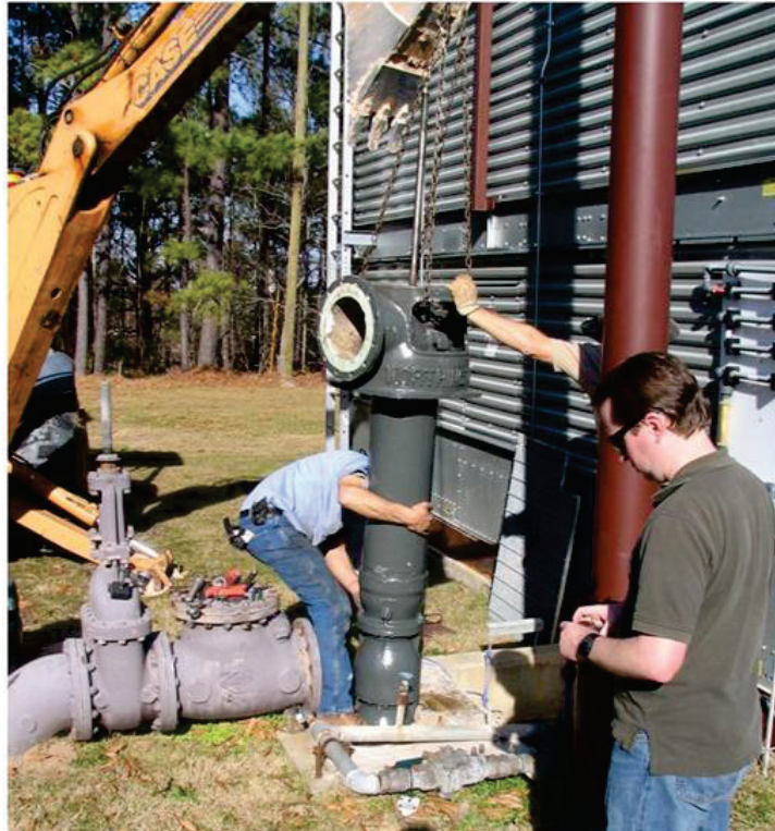
Figure 10. Pump 3 being reinstalled.
