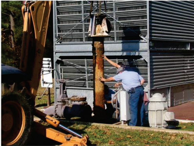
Figure 5. Pump 3 being removed from sump.
