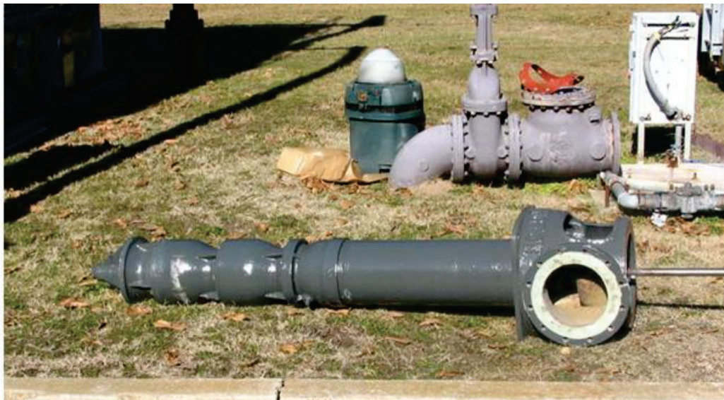
Figure 9. Pump 3, after coating.
