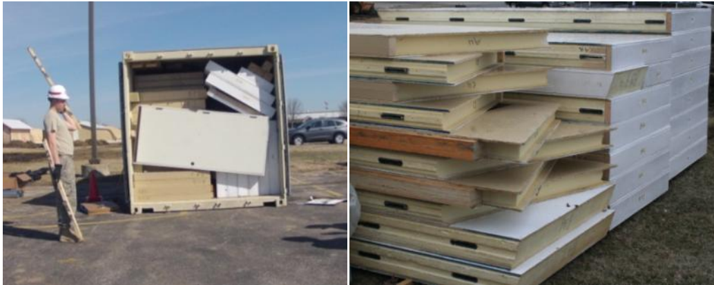
Figure 3-6. SIP unloaded/staged (right).
