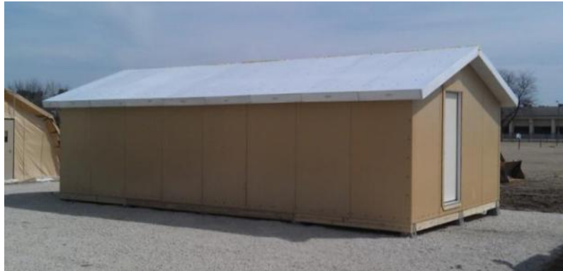
Figure 3-14. Completed SIP hut on CERL's EFOB-L.
