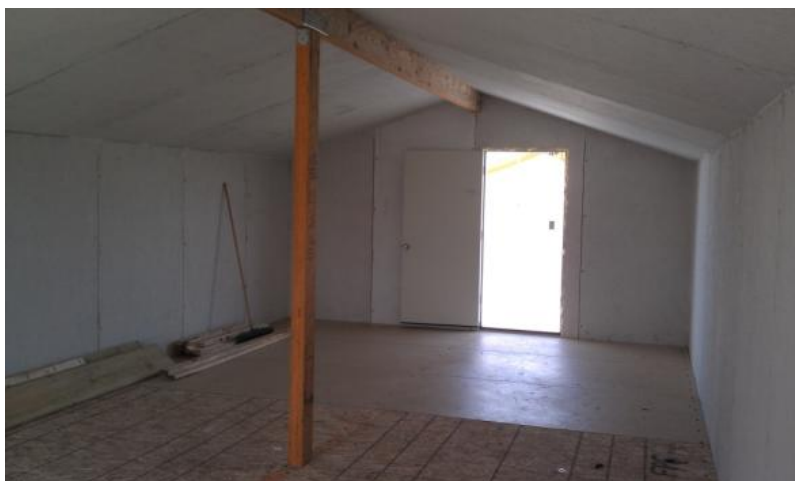
Figure 3-16. Completed SIP hut – Interior.
