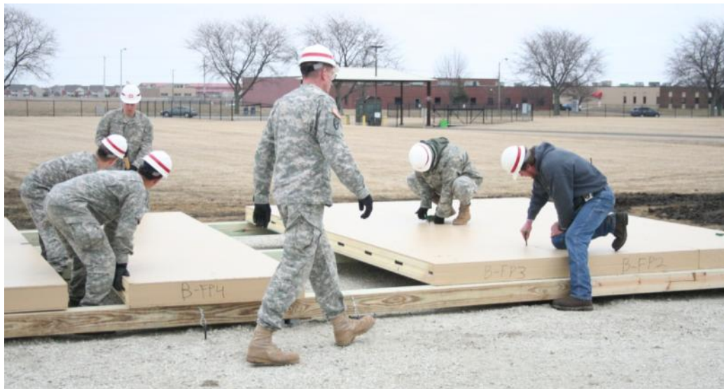
Figure 3-7. Placing floor panels and locking cam-lock.
