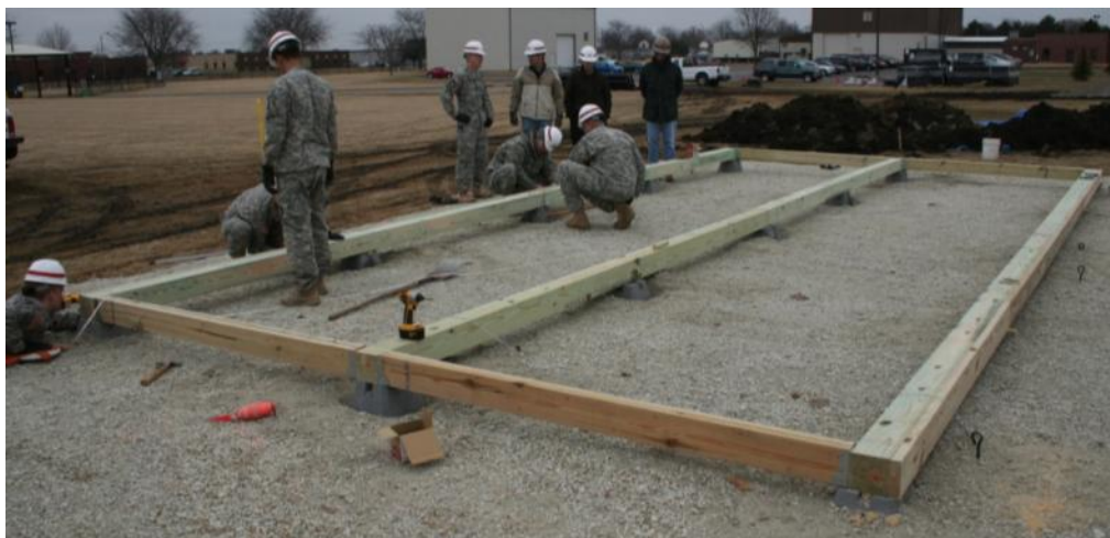
Figure 3-5. Finishing the foundation.
