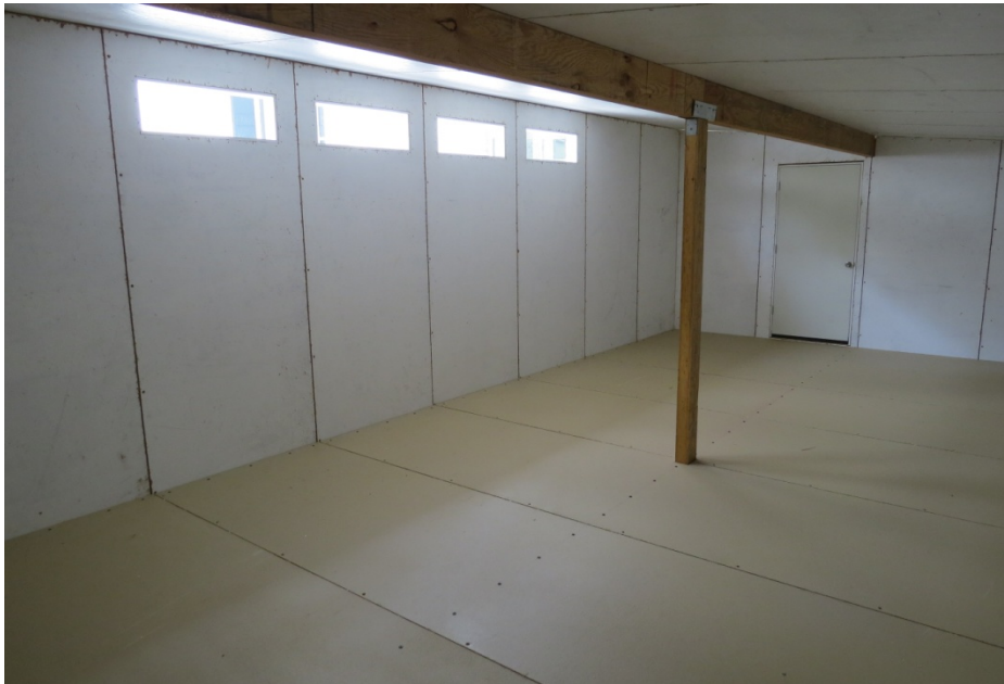
Figure 3-18. SIP hut 4.0 interior showing windows.
