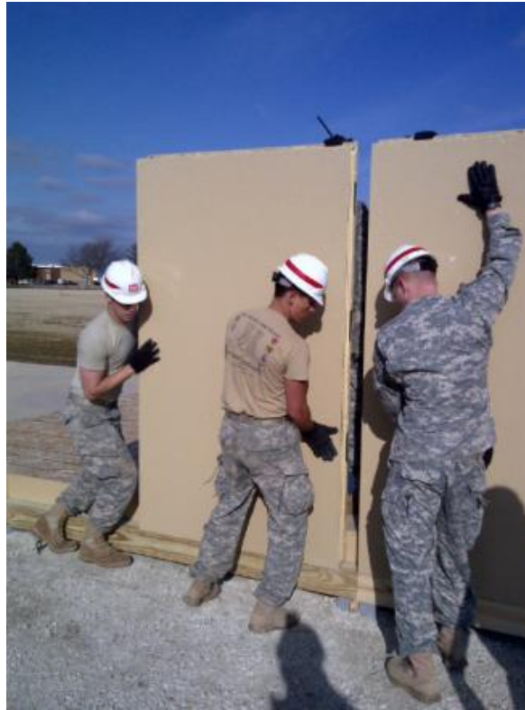
Figure 3-8. Wall panel placement.
