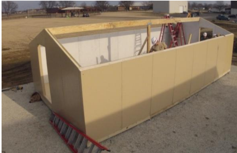
Figure 3-10. SIP hut pre-roof construction.
