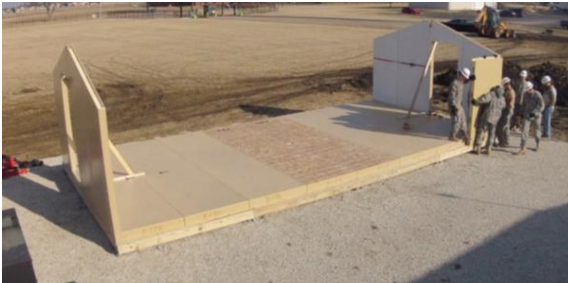
Figure 3-9. SIP hut wall construction.
