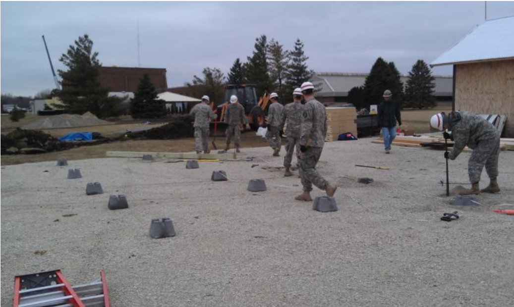
Figure 3-2. Setting up SIP hut foundation piers.
