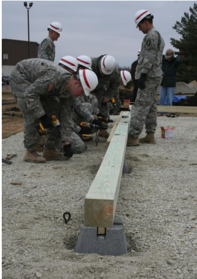
Figure 3-4. Foundation beam cleat.
