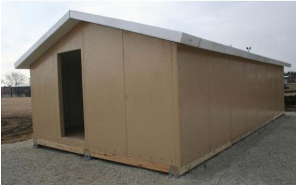
Figure 3-12. SIP hut before finishing.
