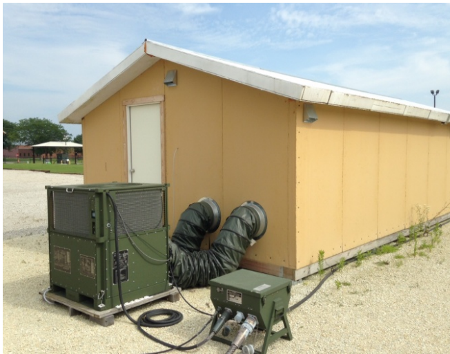
SIP hut and environmental control unit
