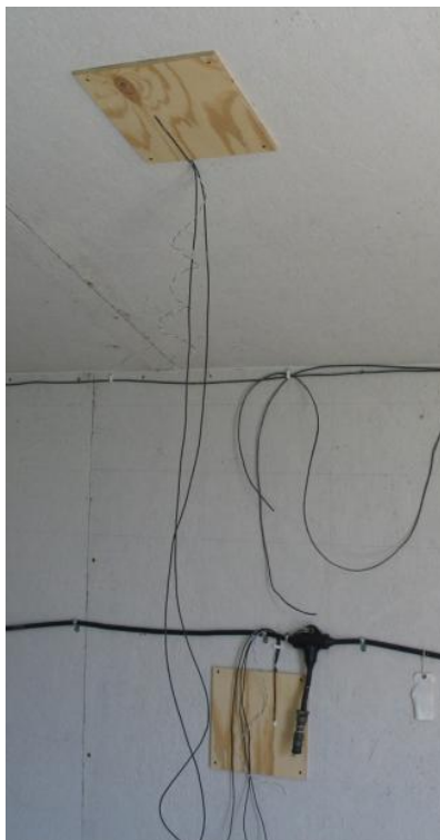
Figure 4-9. HFTs on wall and roof.
