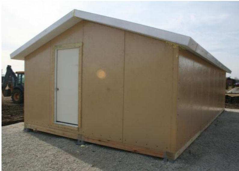
Figure 3-15. Completed SIP hut – north face.
