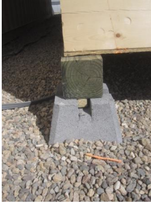
Figure 2-2. Site conditions at Camp Roberts.
