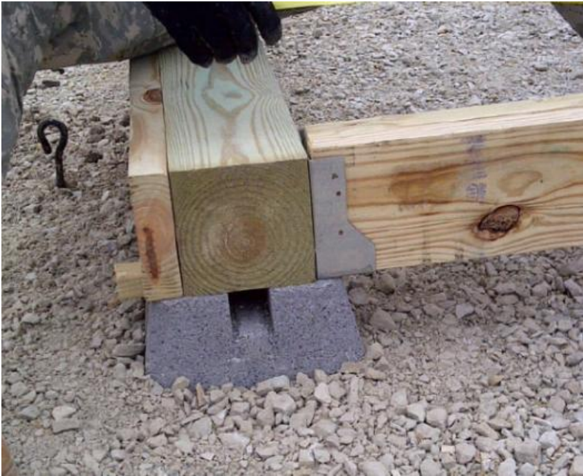
Figure 3-3. Foundation connection detail.
