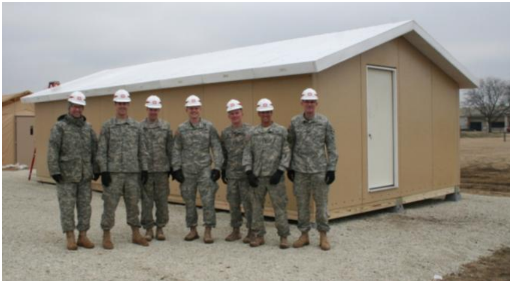
Figure 3-13. Completed SIP hut and partial build crew.
