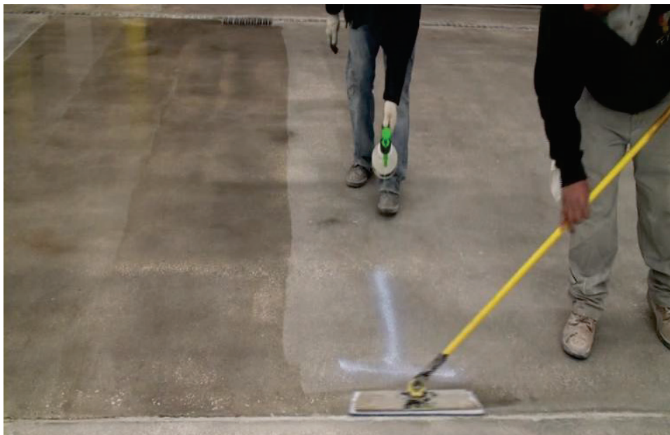
Figure 15. Application of Pentra Guard® (HP).
