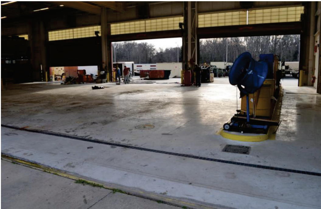
Figure 8. Vehicle maintenance bays.
