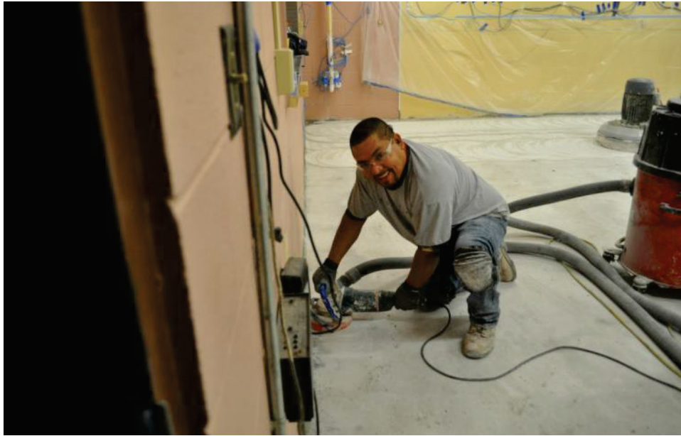
Figure 12. Hand grinding in close quarters.
