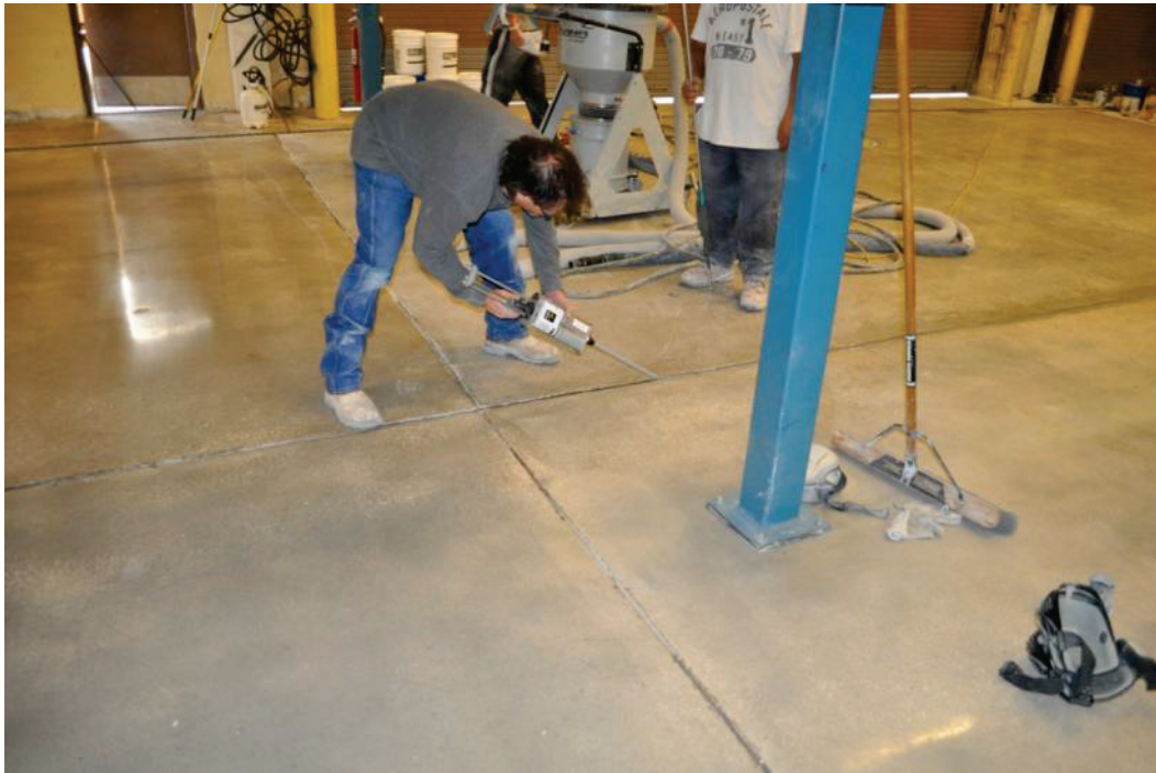
Figure 17. Application of joint sealer.
