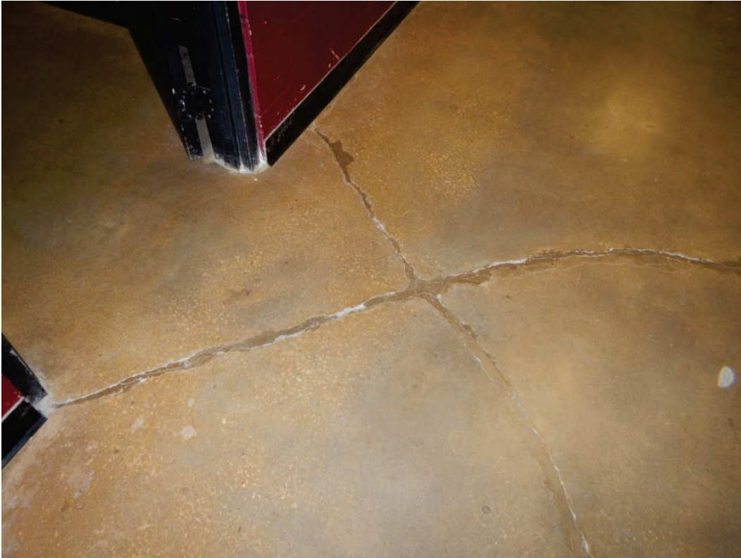
Figure 24. Repaired cracks, showing lighter areas of repair-material deterioration.
