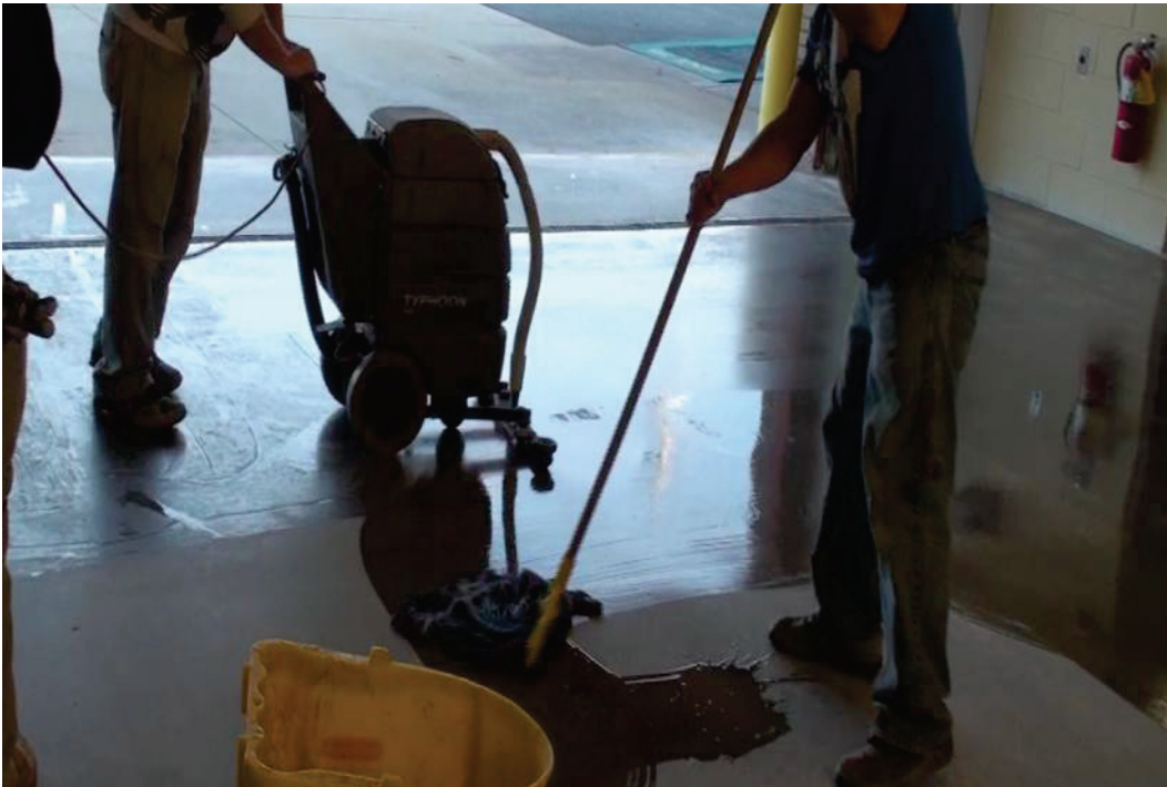
Figure 11. Application of Pentra-Sil® 244+.
