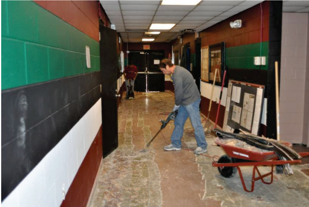
Figure 9. Chisel removal of floor tile
