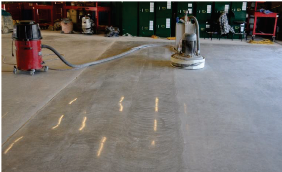
Figure 14. Finish grind with 800 grit abrasive.
