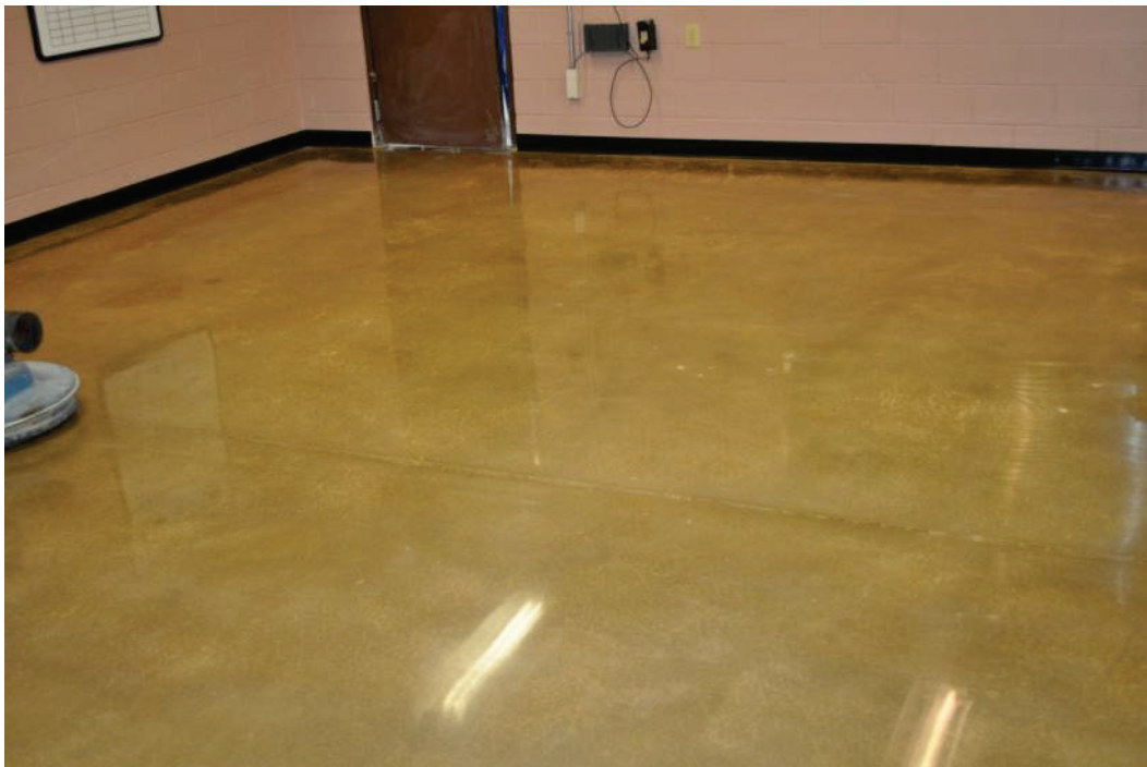
Figure 20. Completed training room showing concrete with applied stain.
