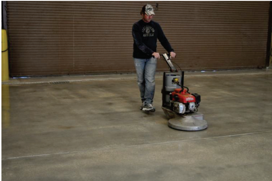
Figure 16. Final burnishing of sealant topcoat with 1,500 grit abrasive pad.
