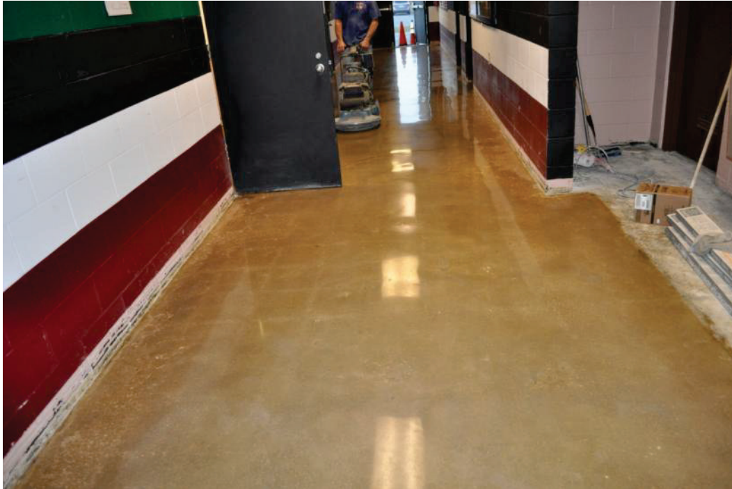
Figure 19. Completed hallway showing concrete with applied stain.
