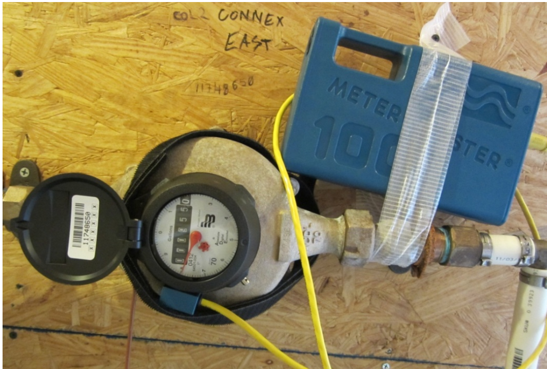
Figure 52. Flow recorder attached at badger meter in FOB.
