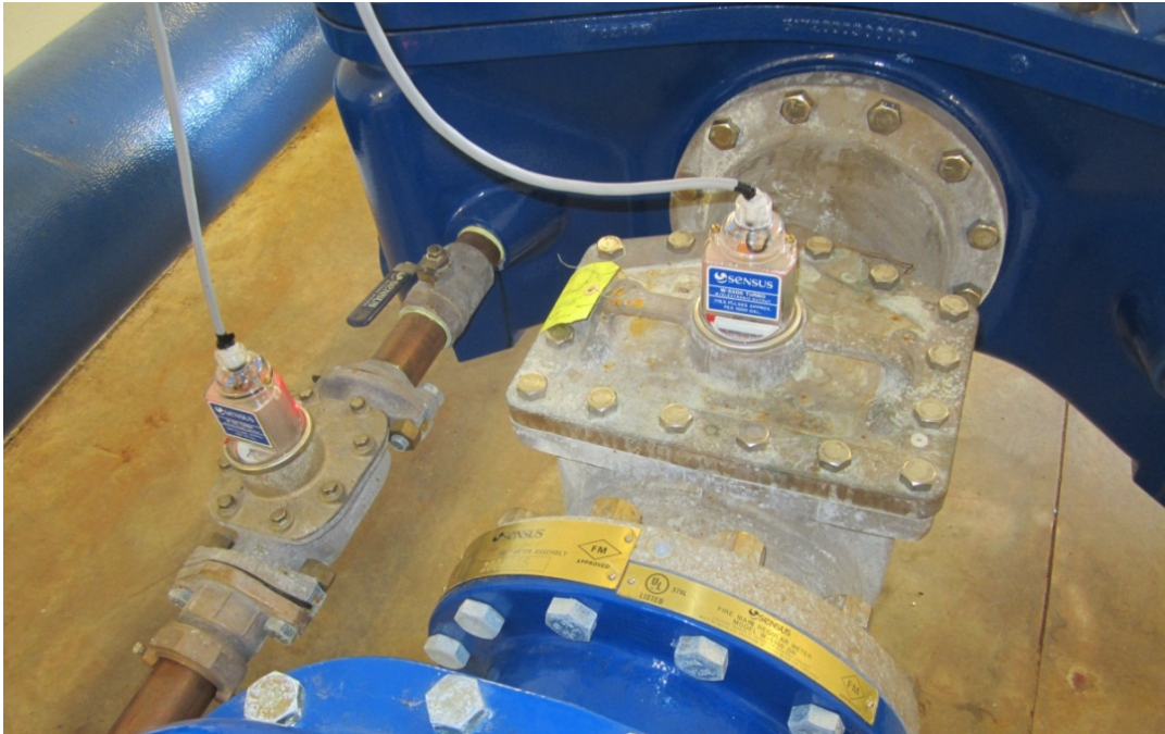
Figure 50. Main meter set composed of two meters.
