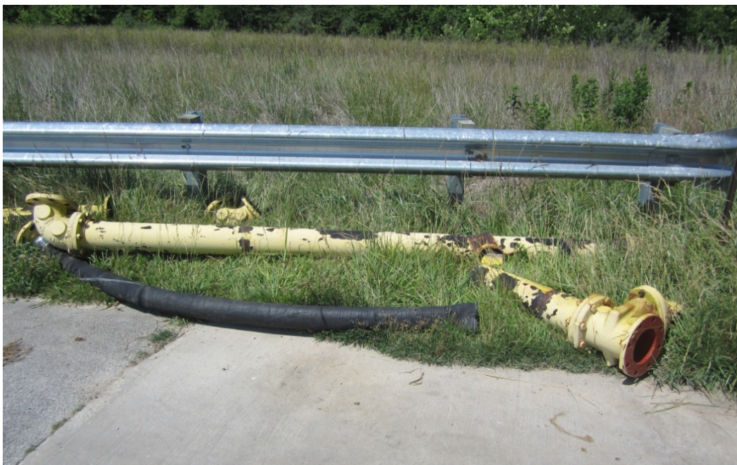
Figure 41. Six-inch pipe replaced due to poor condition at bulk water station.
