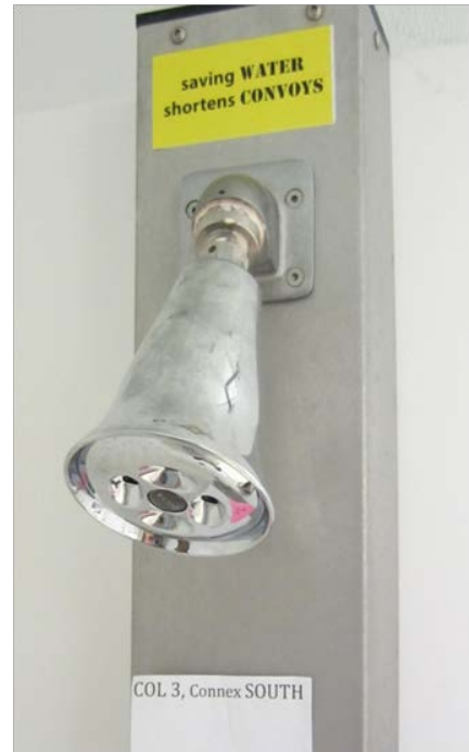
Figure 32. New showerhead installed at FOB 3.
