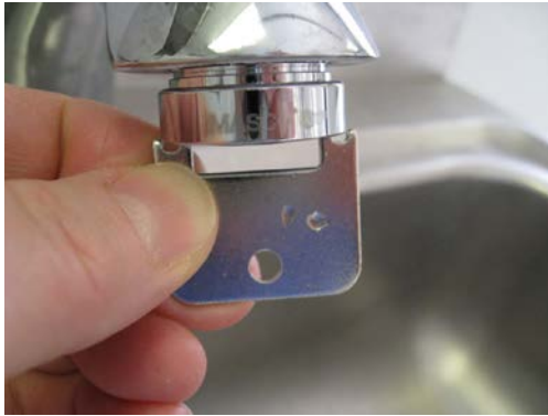
Figure 33. Installation of new aerator.
