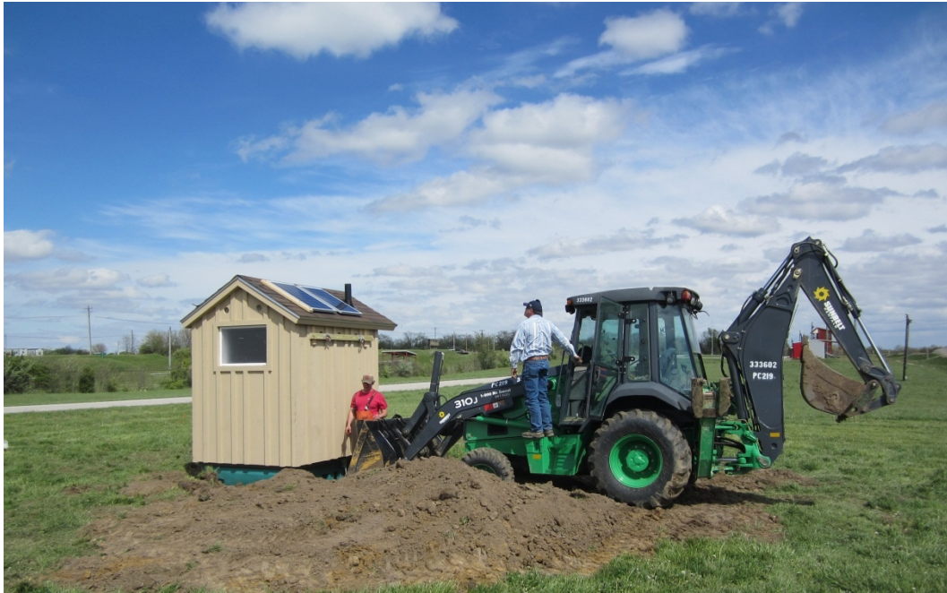
Figure 42. Composting toilet installation.
