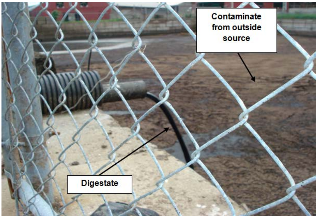
Figure A-5. View of the digestate leaving the digester. The brown crust on top of the digestate is manure from outside contamination, not from the digester.
