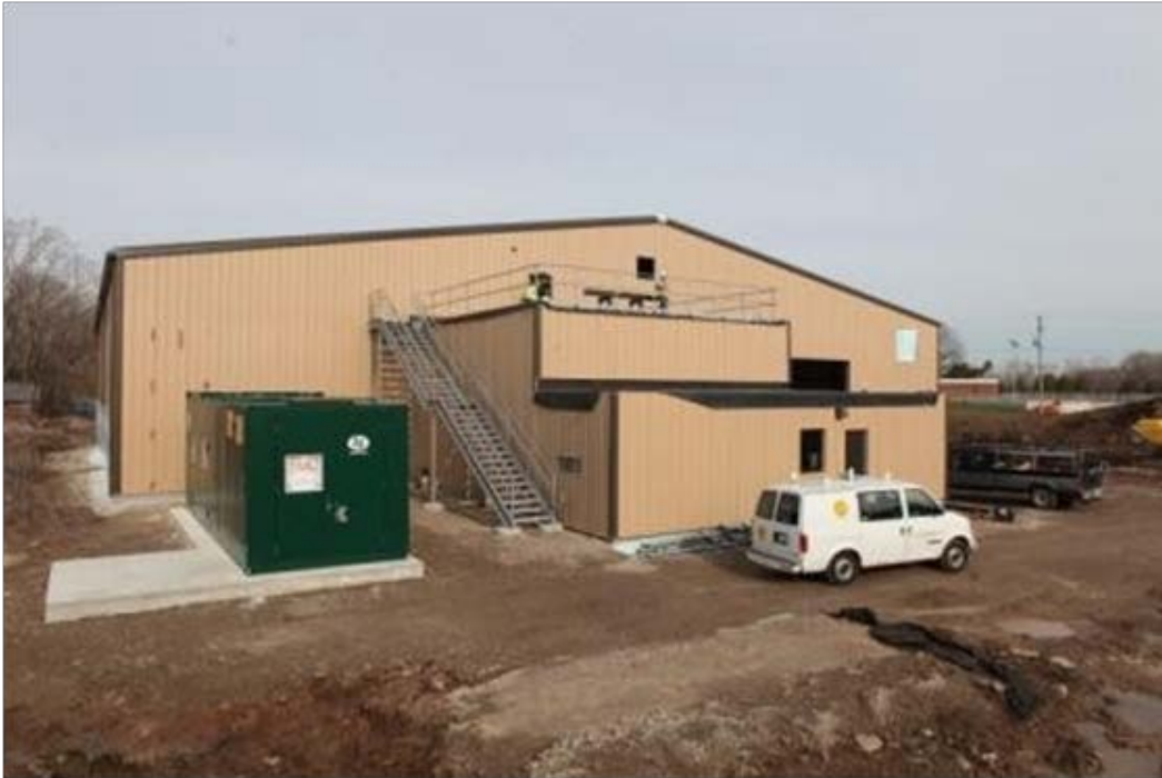
Figure 2-2. The University of Wisconsin Oshkosh digester is complexly contained inside this building, helping to further reduce the smell as well as the sight of food waste (UWO Photo Gallery – Biodigester 2011).
