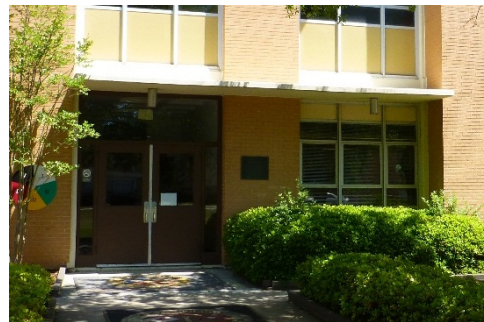
Entry bay on the south elevation with a flat concrete canopy and ceiling-mounted light fixtures.
