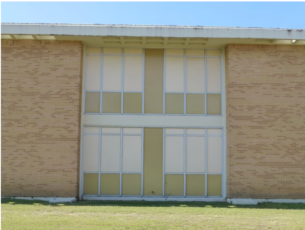
Figure 48. Modified window openings with newer panel inserts, Building 29816, Fisher Hall (ERDC-CERL, 2015).
