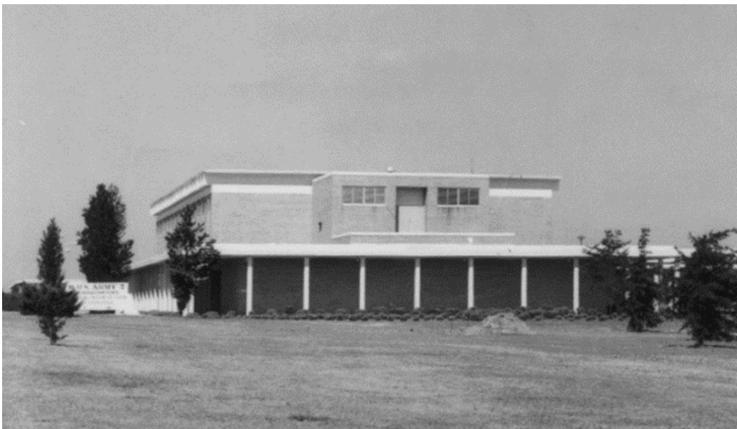
Figure 233. East elevation of Building 29805, Alexander/Olmstead Halls, April 1978 (National Archives at College Park, MD).
