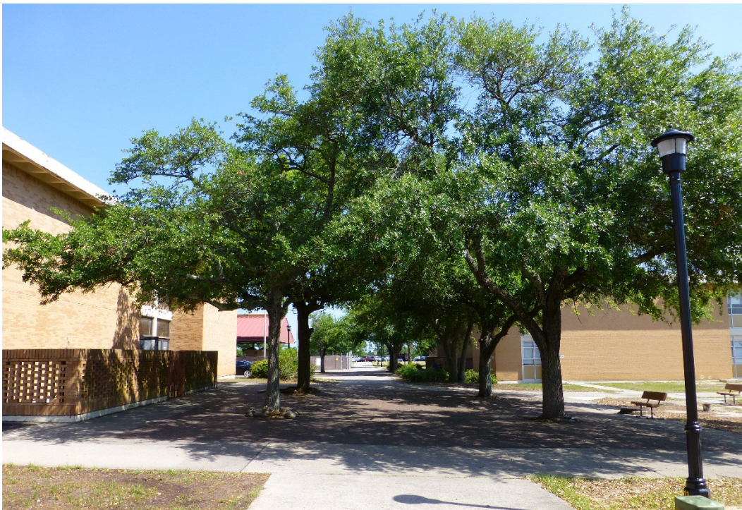
Figure 104. East side of Building 29811, Saltzman Hall, the most intact brick plaza with the four original oak trees (ERDC-CERL, 2015).
