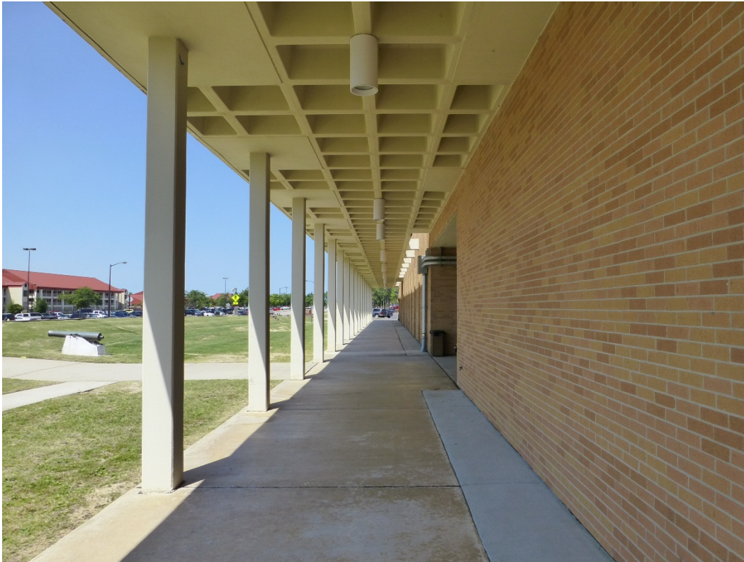
Figure 66. Extensive wrap-around concrete waffle canopy connects the main administration buildings: Building 29805, Alexander/Olmsted Halls; Building 29807, Museum (Conrad Hall); and Building 29808, Signal Towers (ERDC-CERL, 2015).
