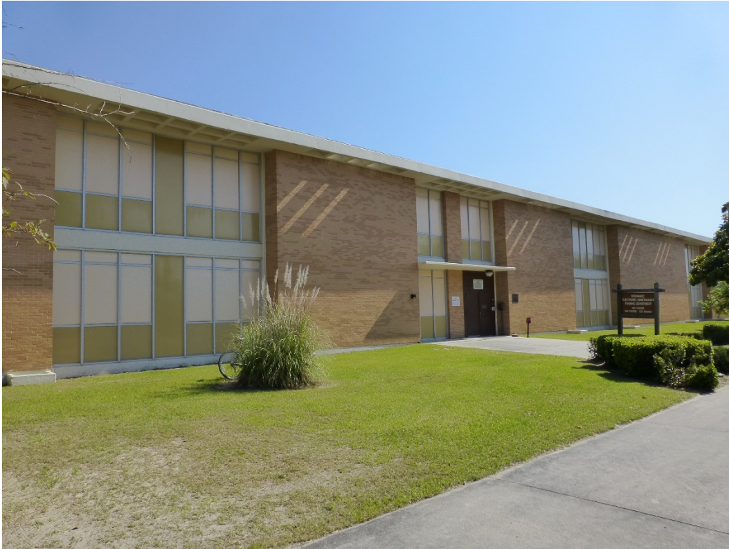
Figure 405. South elevation of Building 29817, Allison Hall (ERDC-CERL, 2015).
