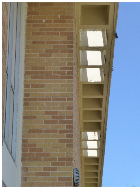
Perforated concrete waffle overhang.
