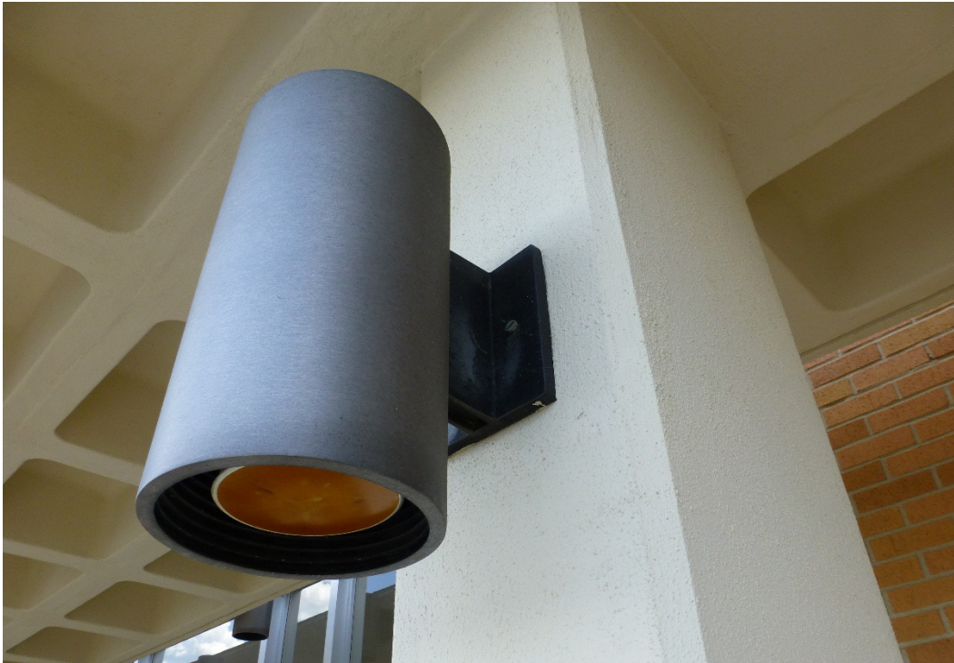
Figure 79. In-kind replacement cylinder—bronze wall-mounted light fixture—located near the main entry on the south elevation of Building 25810, Brant Hall (ERDC-CERL, 2015).
