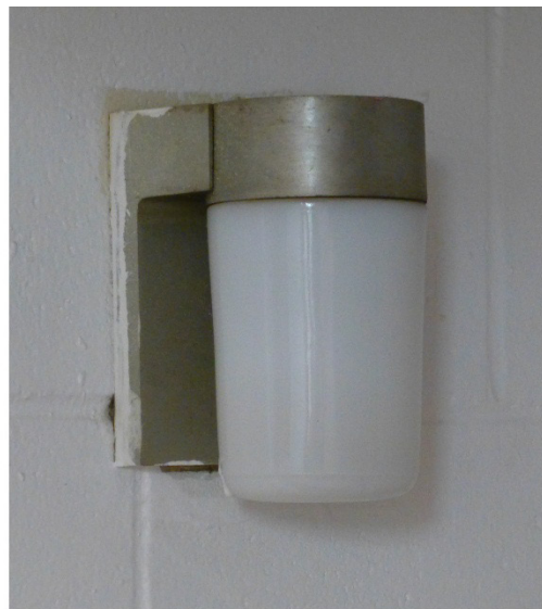
Figure 149. Wall-mounted pendant light fixture – comparison of the original design drawing and light fixture type from 1966 [left] to the current condition of the wall-mounted light fixture [right] (ERDC-CERL, 2015).
