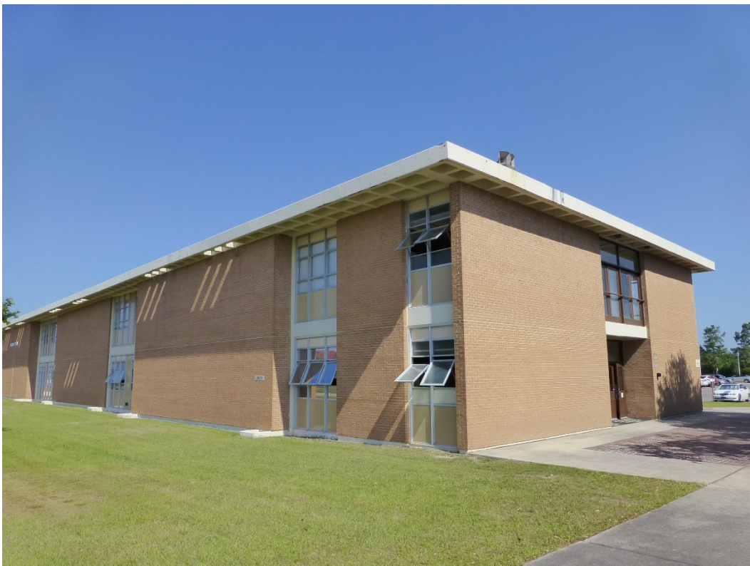
Figure 29. Rectangular massing, Building 29815, Hazen Hall (ERDC-CERL, 2015).
