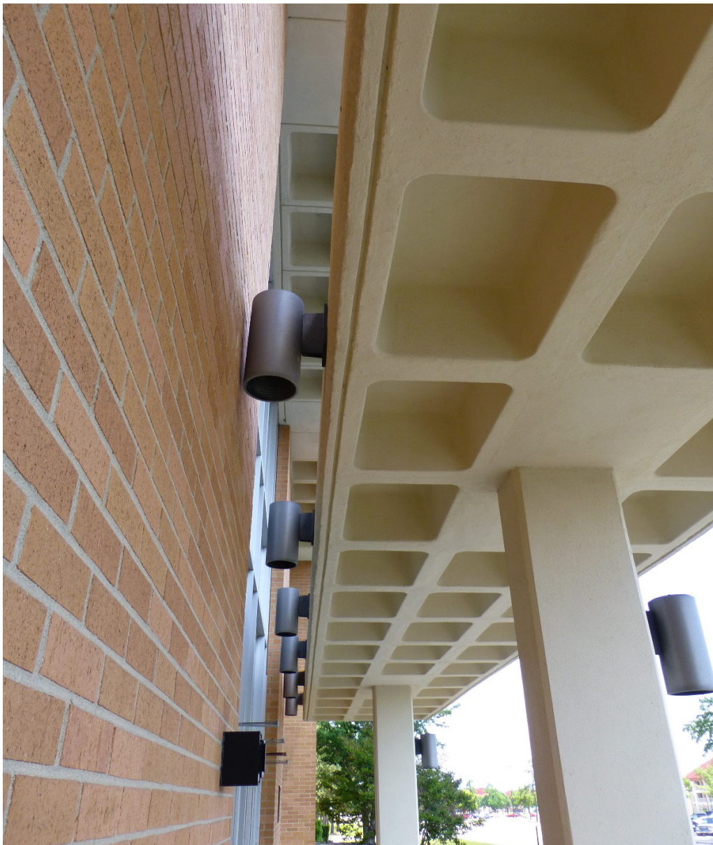
Figure 65. Close-up of the flat concrete waffle canopy highlighting the main entry into Building 25810, Brant Hall (ERDC-CERL, 2015).
