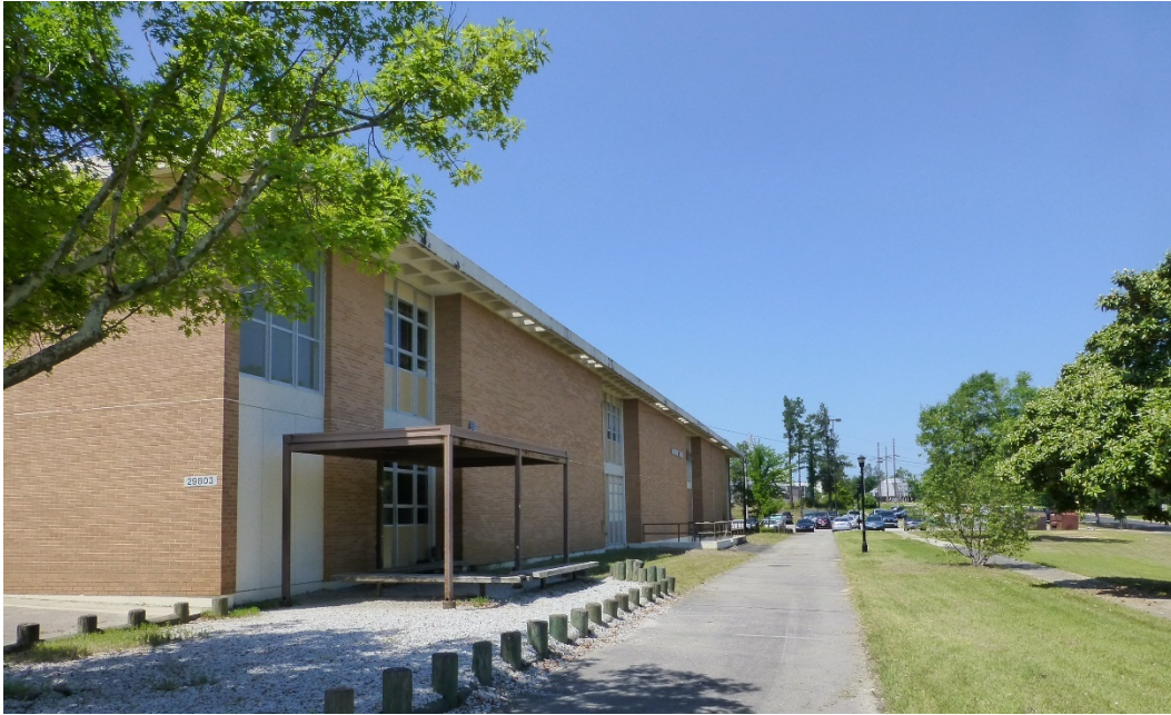
Figure 214. North elevation of Building 29803, Moran Hall north (ERDC-CERL, 2015).
