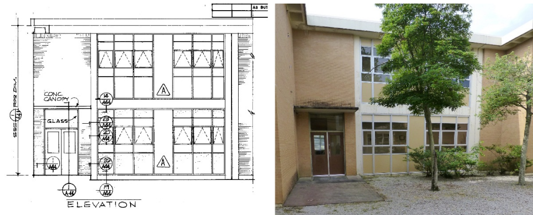
Figure 338. North wall of the right courtyard south wall of the left courtyard – comparison of the original design and materials from 1964 [left] to the present day [right] (ERDC-CERL, 2015).
