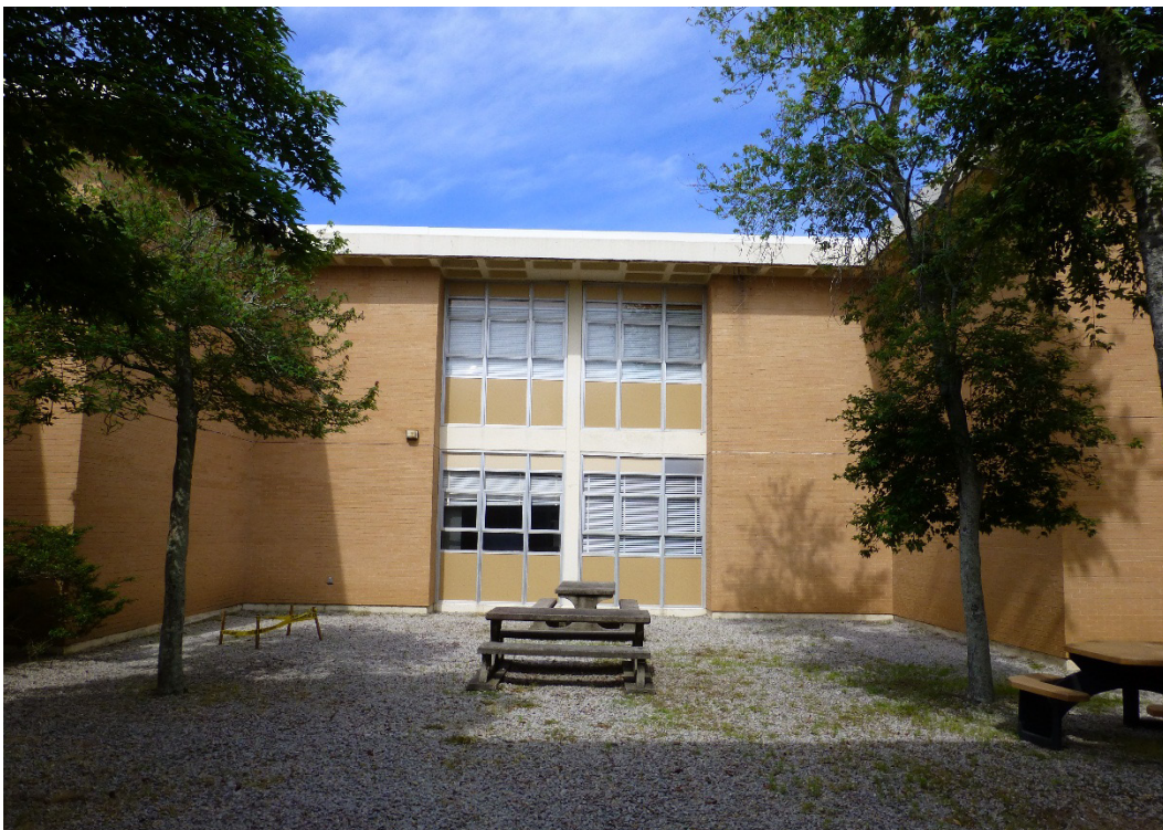
Figure 94. Interior view of the east courtyard in Building 29813, Allen Hall, showing the designed landscape of the four trees placed within the courtyard (ERDC-CERL 2015).
