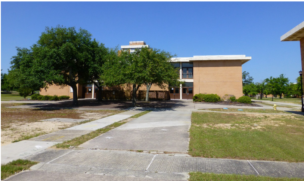
Figure 275. East elevation of Building 29809, Greely Hall (ERDC-CERL, 2015).
