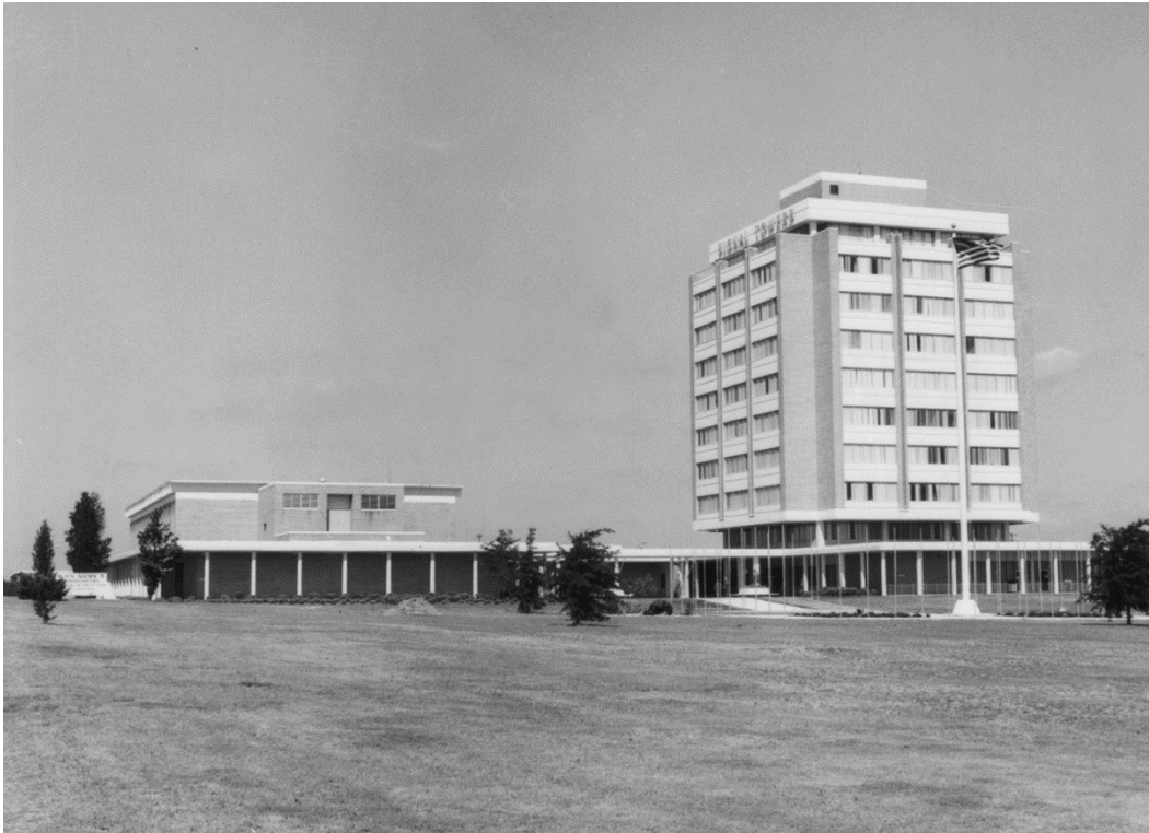
Figure 234. General view of the east elevations of the administration complex of Buildings 29805 [left], 29807 [middle], and 29808 [right], April 1978 (National Archives at College Park, MD).
