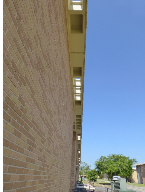
Perforated concrete waffle overhang.
