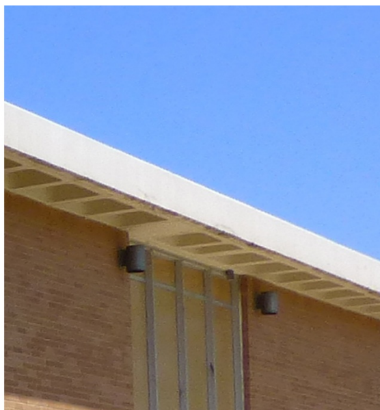
Figure 212. Wall-mounted light fixtures - comparison of the original drawing detail from 1966 [left] to the current condition of the wall-mounted light fixtures on the east and west elevations [right] (ERDC-CERL, 2015).
