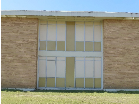
Window pattern; window bay with six bright-aluminum framing insulated panels and separated by an insulated panel. Exposed concrete structural system divides the first and second-floor window groups.
