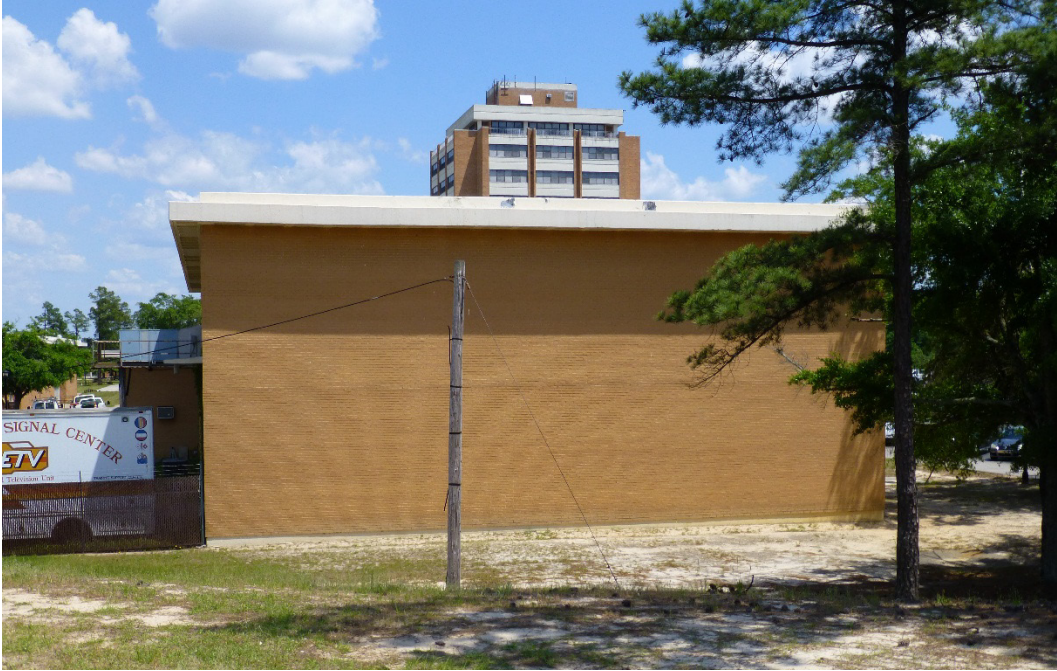
Figure 194. West elevation of Building 29801, Nelson Hall (ERDC-CERL, 2015).
