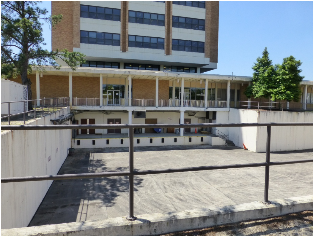
Figure 262. Basement level and loading area on the north side of Building 29808, Signal Towers (ERDC-CERL, 2015).
