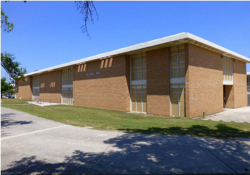
Figure 205. Southeast oblique of Building 29802, Moran Hall south (ERDC-CERL, 2015).
