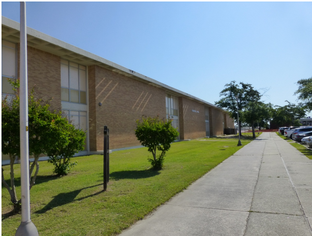
Figure 441. South elevation of Building 29819, Stansell Hall (ERDC-CERL, 2015).
