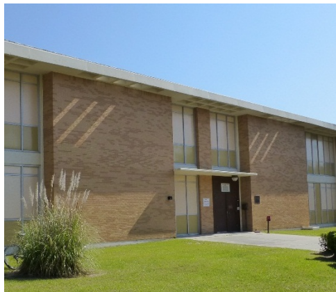
"Light pattern" created by the perforated concrete waffle overhang.
