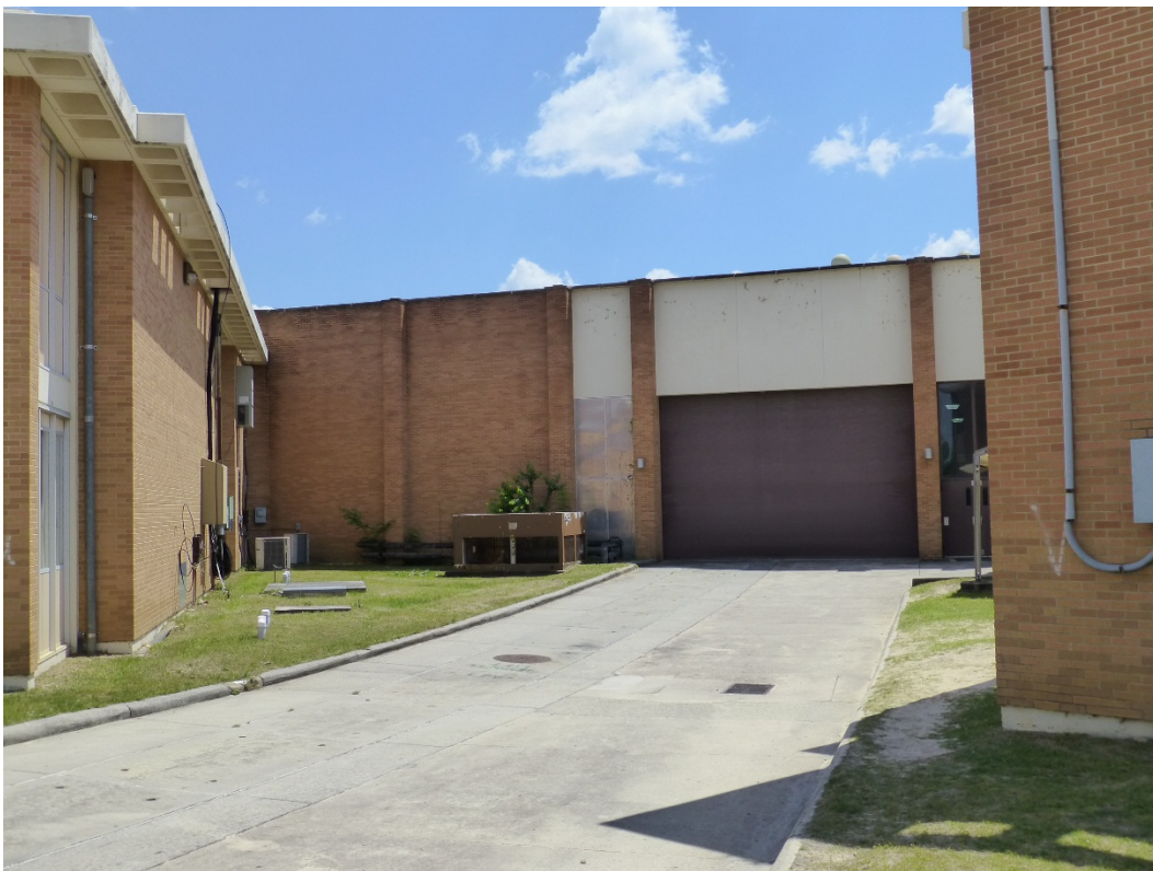
Figure 178. North side of the six-sided middle structure (ERDC-CERL, 2015).
