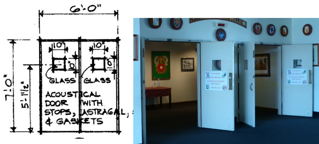
Figure 244. Interior auditorium doors - Comparison of the original drawing detail from 1966 [left] to the current condition of the acoustical doors [right] (ERDC-CERL, 2015).
