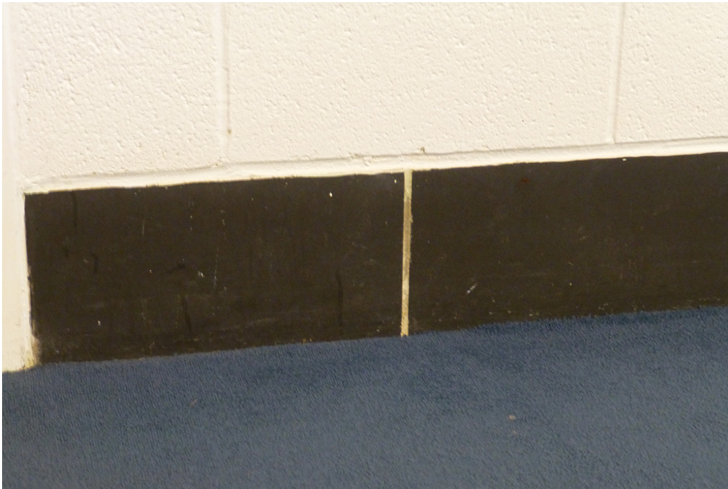
Figure 131. Example of glazed concrete block utilized as a baseboard (ERDC-CERL, 2015).
