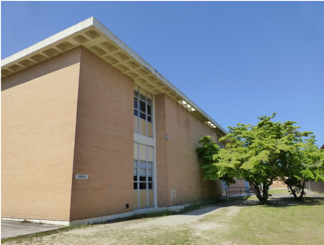
Figure 423. North elevation of Building 29818, Johnston Hall (ERDC-CERL, 2015).
