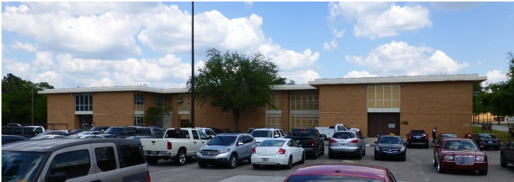
Figure 207. West elevation of Building 29803 [left] and Building 29802 [right] (ERDC-CERL, 2015).
