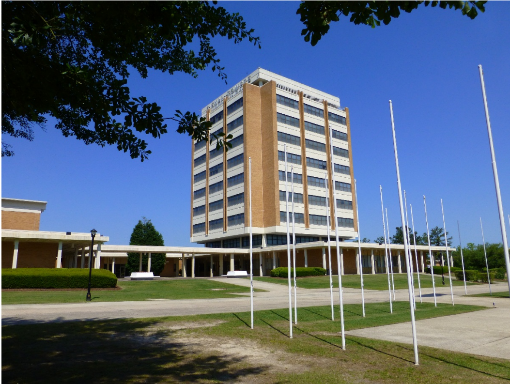
Figure 258. Southeast oblique of Building 29808, Signal Towers (ERDC-CERL, 2015).
