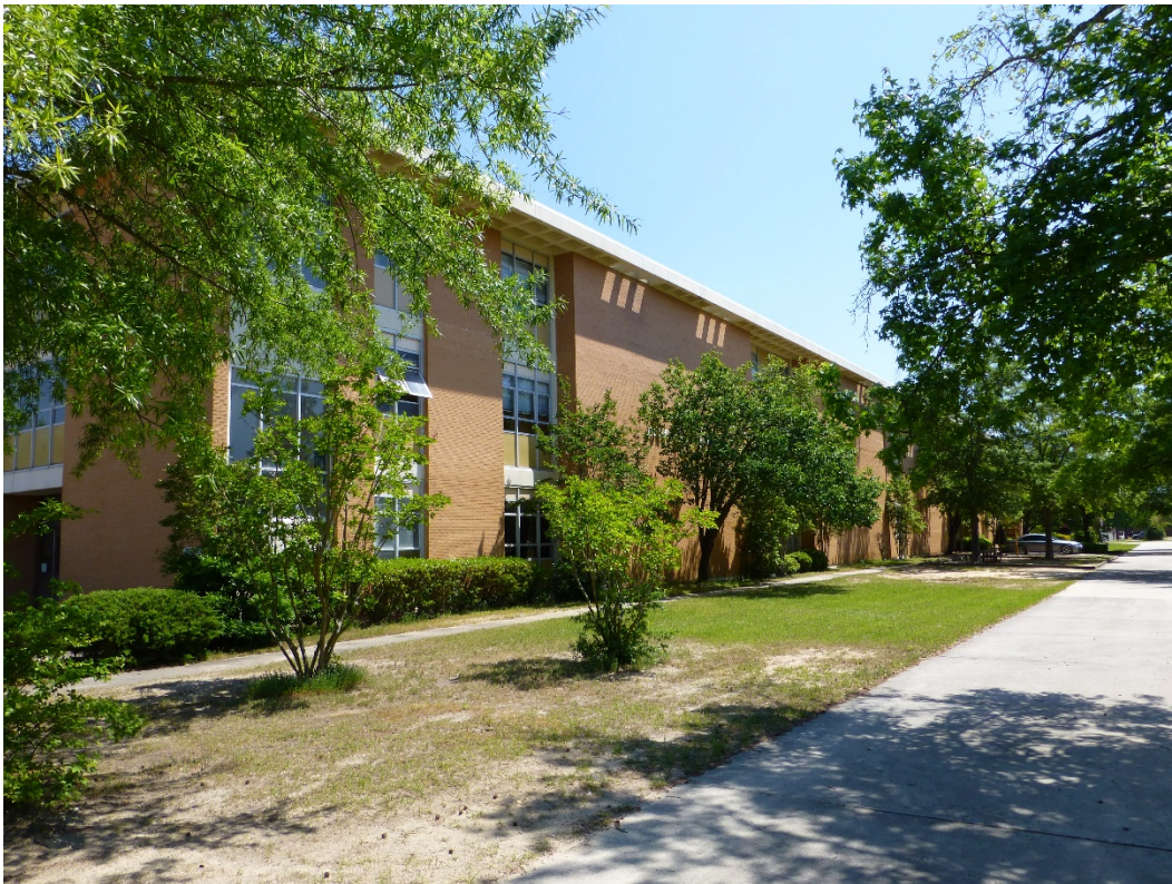
Figure 302. South elevation of Building 29810, Burkhardt Hall (ERDC-CERL, 2015).
