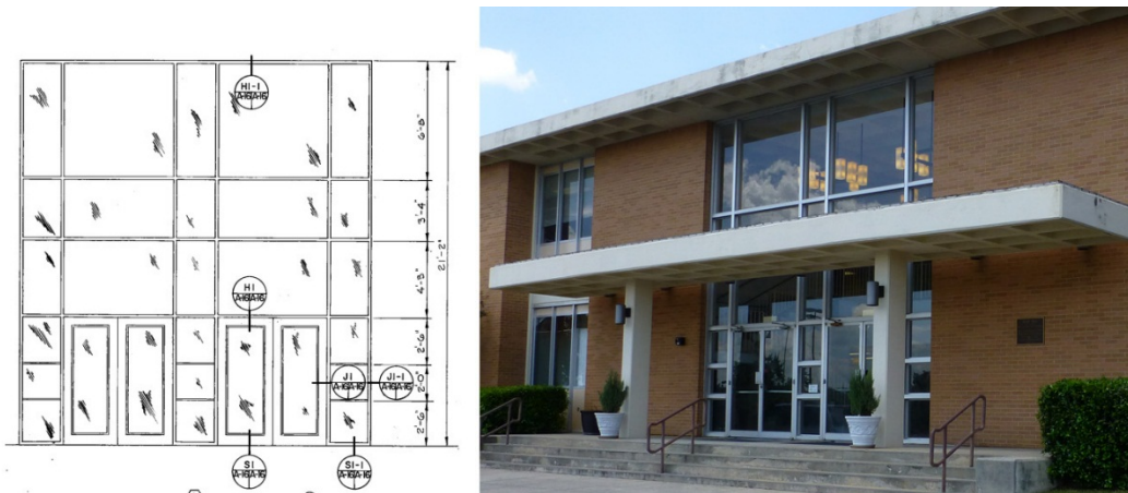
Figure 185. Main entry on the south elevation – comparison of the original drawing detail from 1973 [left] to the current condition of the bright-aluminum and plate-glass windows and doors [right] (ERDC-CERL, 2015).
