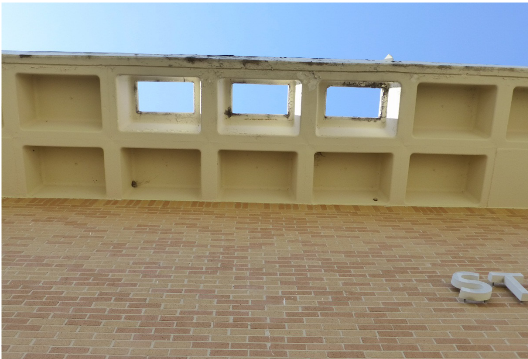
Figure 39. Close-up of concrete waffle overhang, Building 29819, Stansell Hall (ERDC-CERL, 2015).
