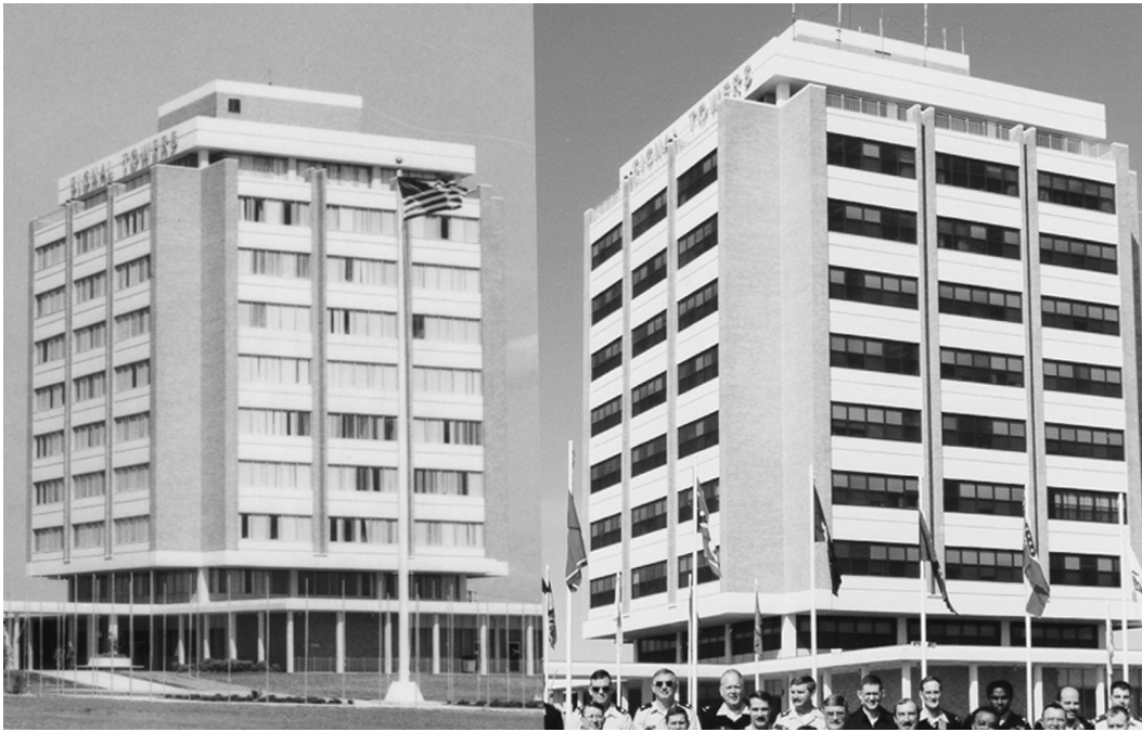
Figure 268. Building 29808, Signal Towers, comparison of the original windows [left] and the replacement windows [right] (Signal Corps Historian Office).
