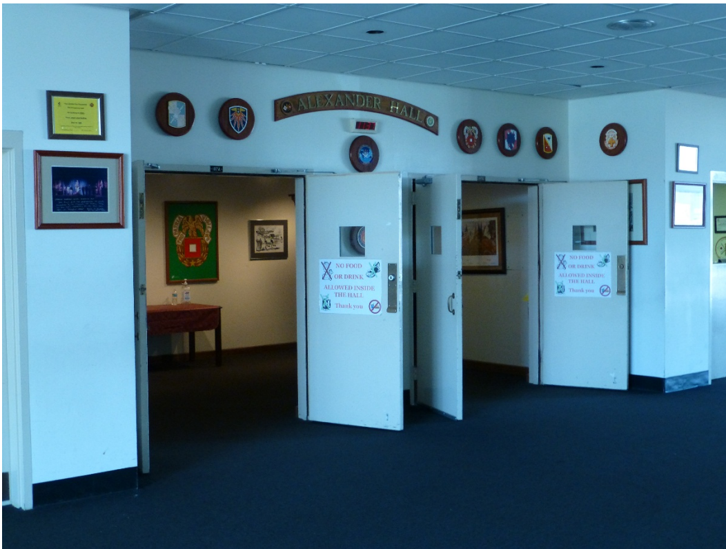
Figure 154. Doors leading from the lobby into the Alexander Hall auditorium space in Building 29805 (ERDC-CERL, 2015).
