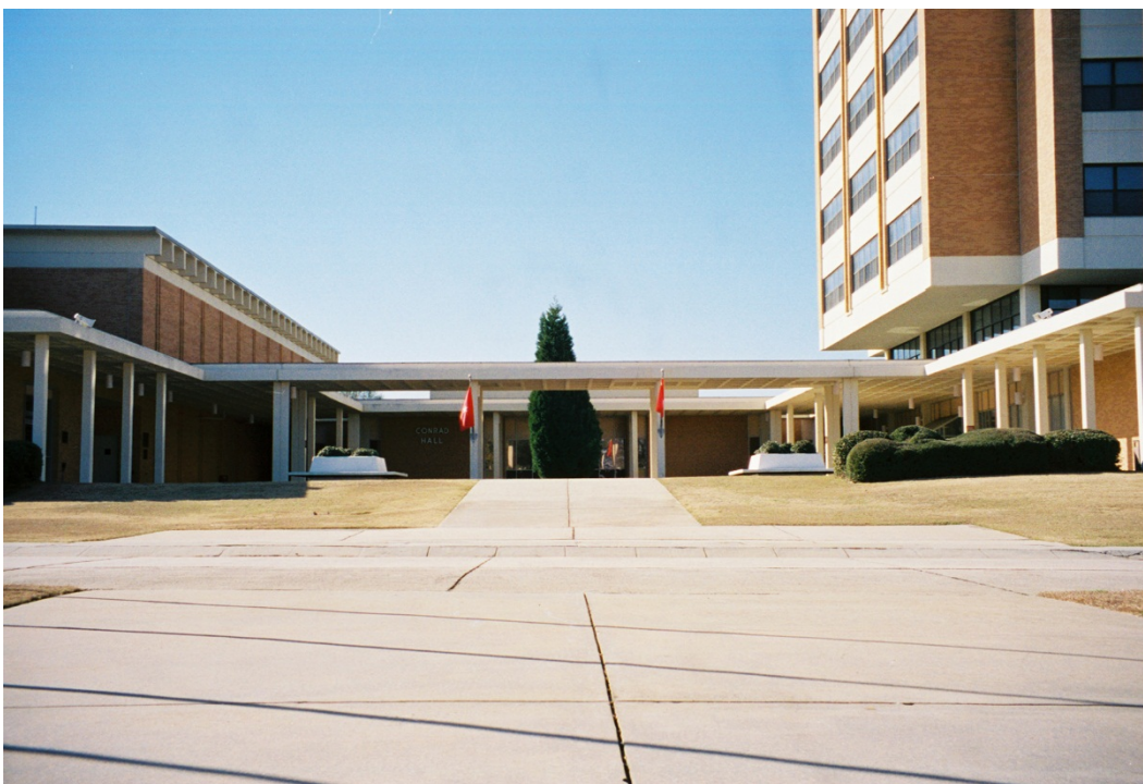
Figure 235. Overall view of the plaza connecting Building 29805 [left], Building 29807 [center], and Building 29808 [right] (ERDC-CERL, 2004).
