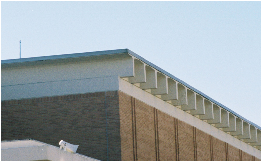
Figure 236. Roof detail of Building 29805, Alexander/Olmstead Halls (ERDC-CERL, 2004).
