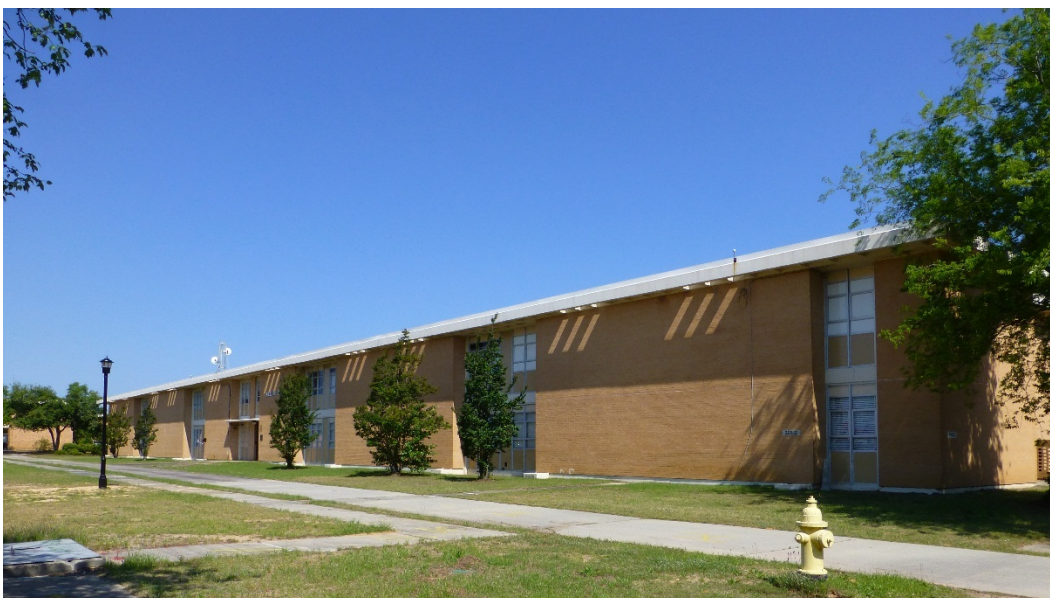
Figure 31. Two-story classroom Building 29813, Allen Hall (ERDC-CERL, 2015).
