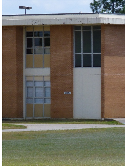
Window pattern: window bays on the left and right sides of the north elevation.
