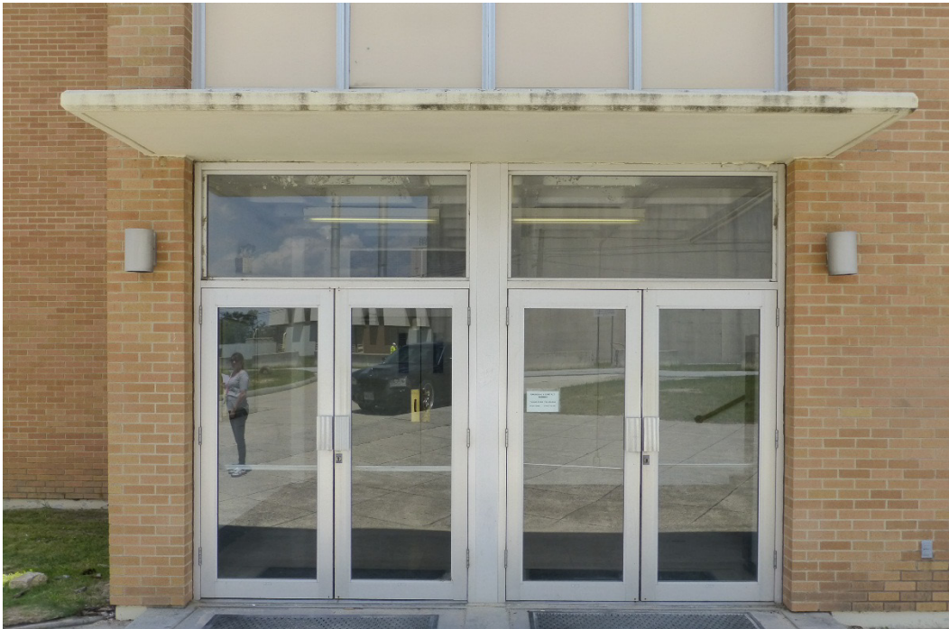
Figure 71. Wall-mounted light fixtures flanking either side of an entry, Building 25810, Brant Hall (ERDC-CERL, 2015).
