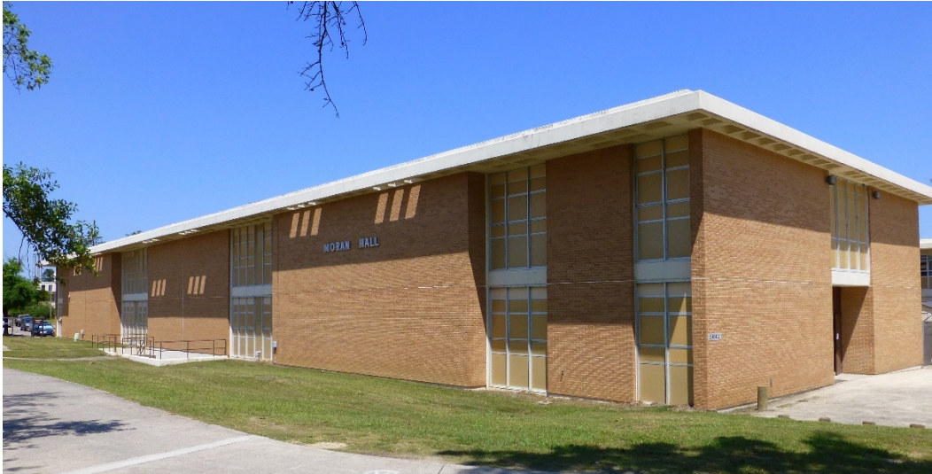
Figure 26. Rectangular massing, Building 29802, Moran Hall south (ERDC-CERL, 2015).
