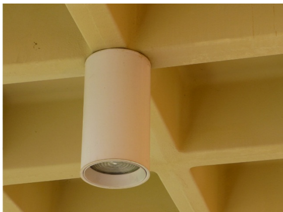
Figure 256. Ceiling-mounted light fixture – comparison of the original drawing detail from 1966 [left] to the current condition of the ceiling-mounted light fixture under the concrete waffle canopy [right] (ERDC-CERL, 2015).
