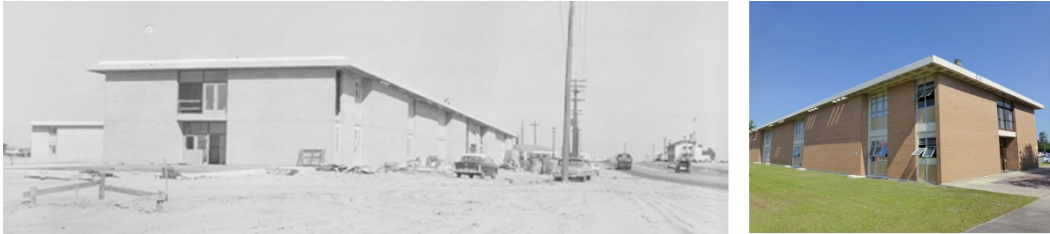
Figure 382. Southeast oblique - comparison of the original design and materials for Building 29815 construction in 1966 [left] to the current condition of the southeast oblique of Building 29815, Hazen Hall [right] (ERDC-CERL, 2015).
