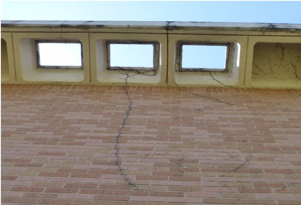
Figure 37. Perforated concrete waffle overhang, Building 29803, Moran Hall north (ERDC-CERL, 2015).
