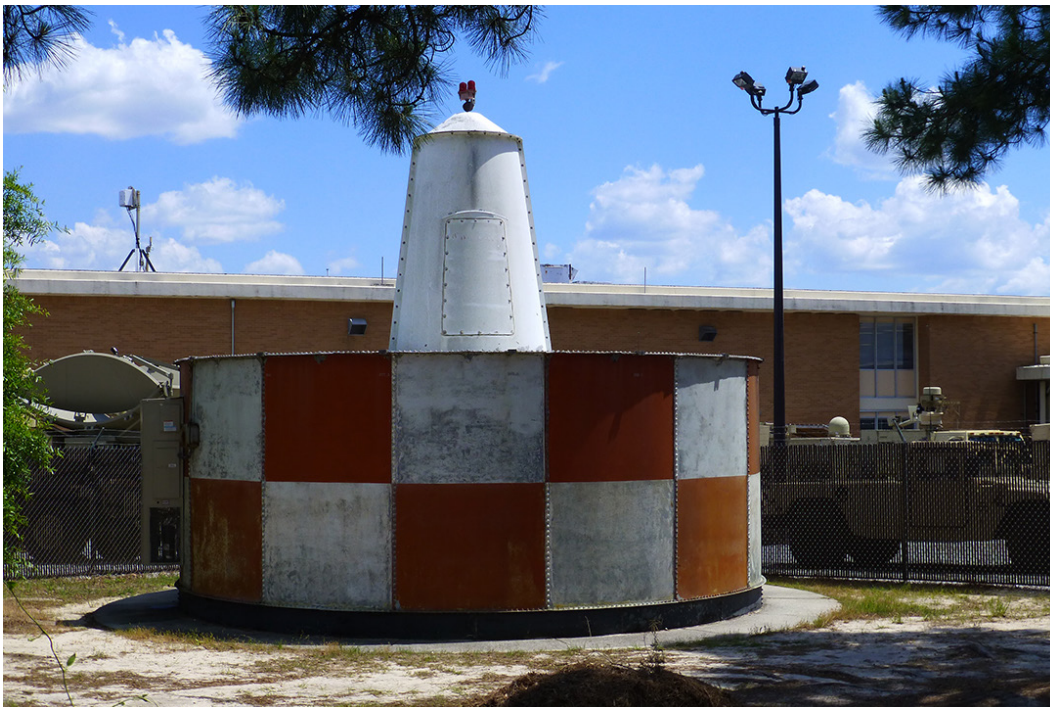
Figure 456. Building 25811 is a concrete pad supporting an IFR beacon that is not real property and was placed here in 1985 (ERDC-CERL 2015).
