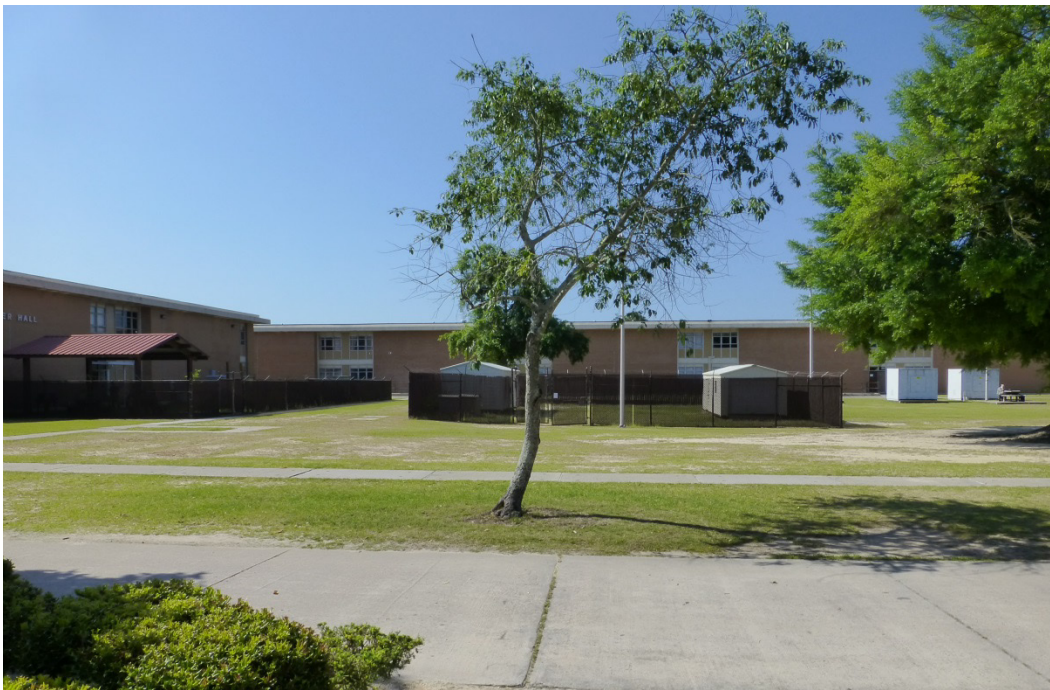
Figure 465. Covered Training Area (no number) on left, and two moveable sheds that are not real property in the center (ERDC-CERL, 2015).
