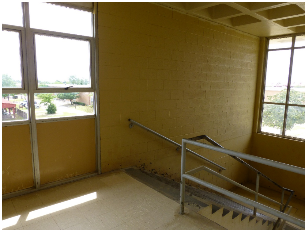
Figure 137. Typical stairwell (ERDC-CERL, 2015).
