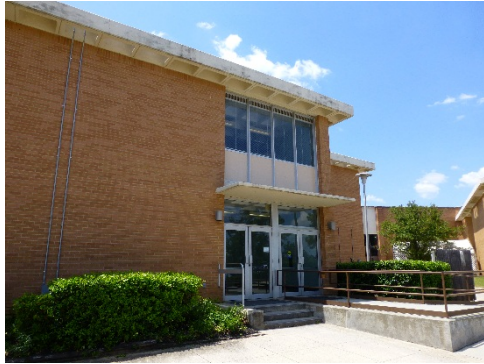
Secondary entrances at the end of the rectangular classroom wings and landscaping.
