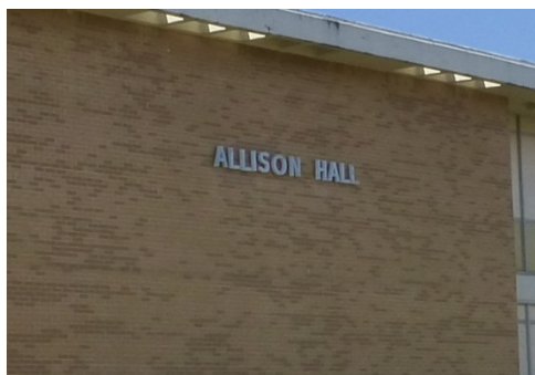
Lettering on the north and south elevations.
