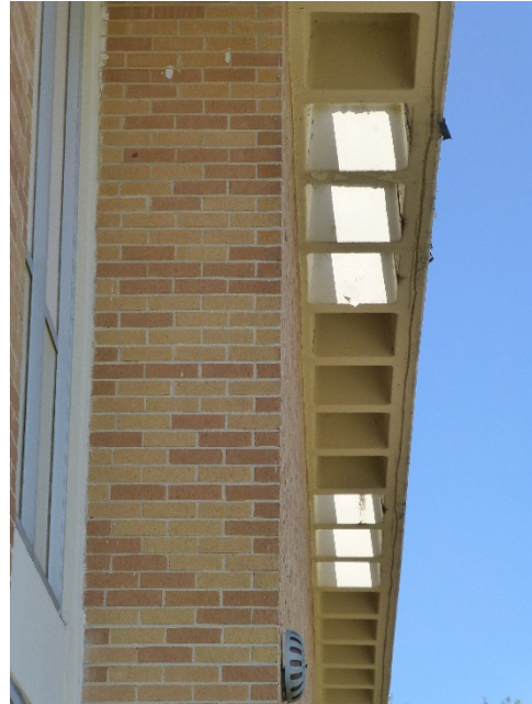
Perforated concrete waffle overhang.
