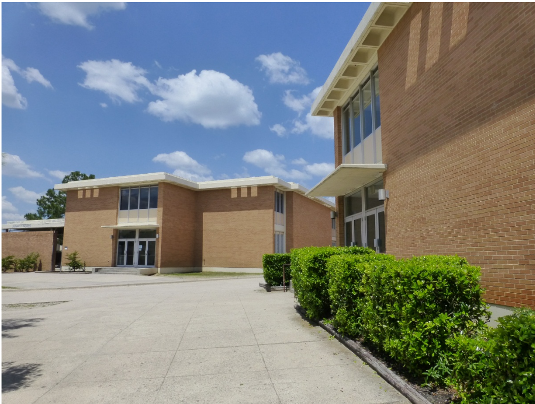
Figure 176. Building 25810, Brant Hall; left is the northwest wing and right is the west side of the south wing (ERDC-CERL, 2015).
