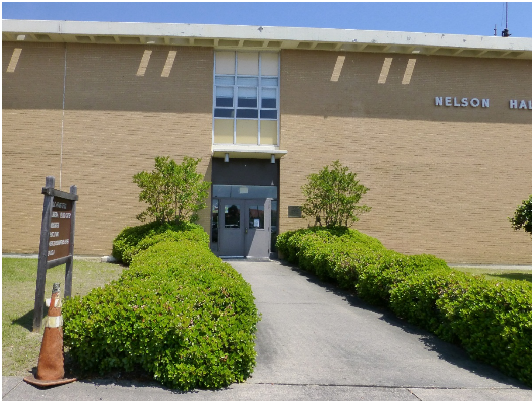
Figure 191. South elevation of Building 29801, Nelson Hall (ERDC-CERL, 2015).
