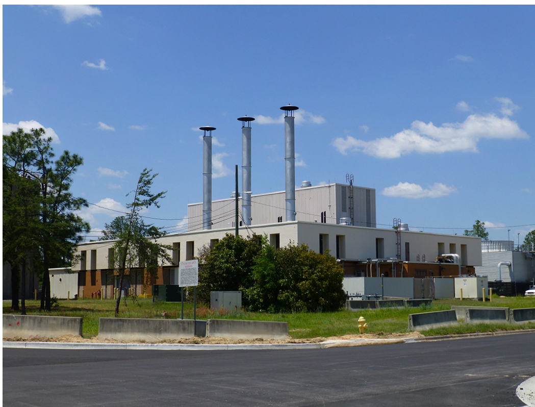
Figure 460. Building 25910 Heating/AC Plant was constructed in 1966 and designed by Sewell and Associates (ERDC-CERL 2015).
