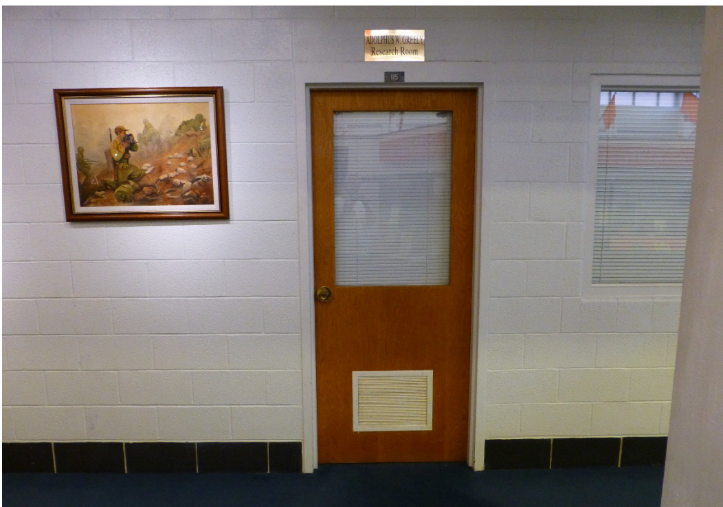
Figure 155. Interior wood door with large light in Building 29807, Museum (Conrad Hall) (ERDC-CERL, 2015).
