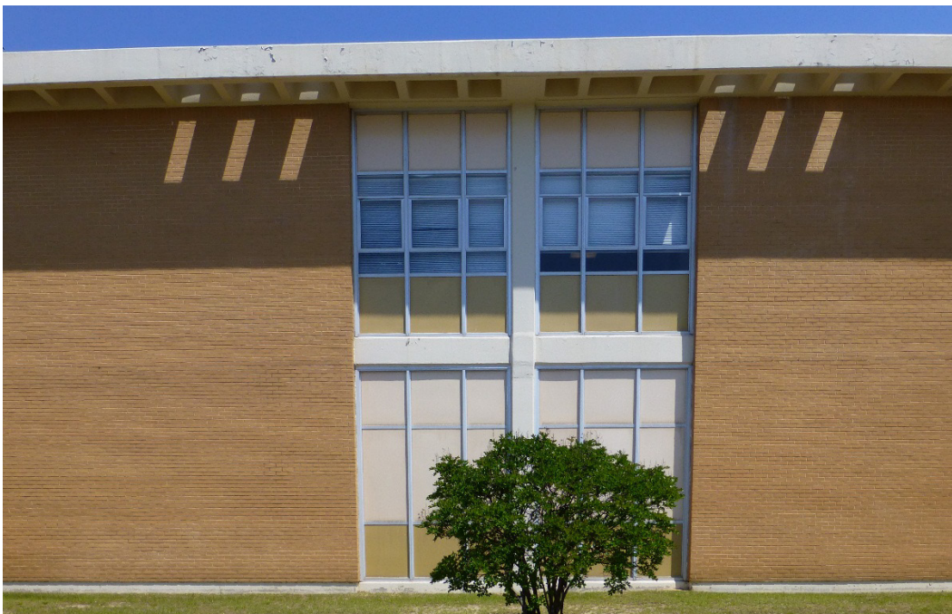
Figure 41. Example of the “light pattern” created by the perforated waffle overhang, Building 29801, Nelson Hall (ERDC-CERL, 2015).
