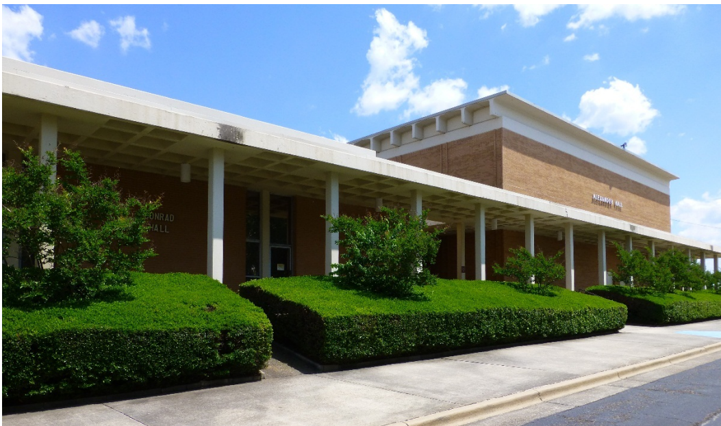
Figure 248. West side of Building 29807 with single entry doors and the concrete waffle canopy that connects to Buildings 29805 and 29808 (ERDC-CERL, 2015).
