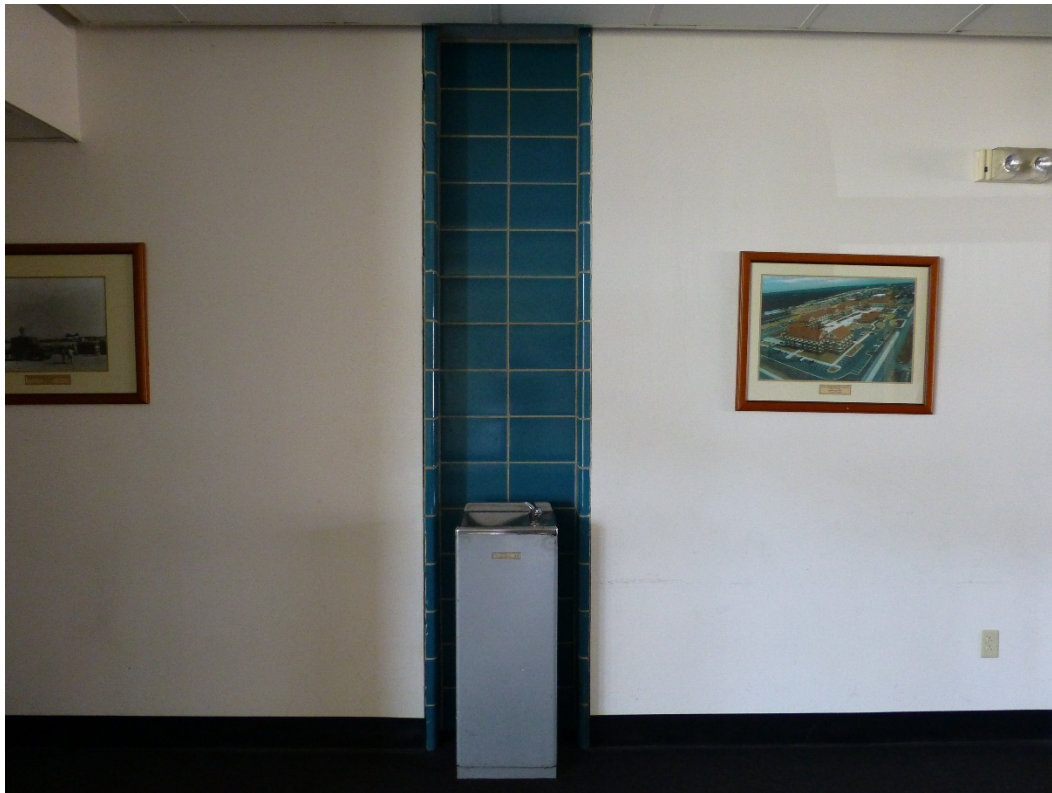
Figure 164. Water fountain alcove in Building 29805 (ERDC-CERL, 2015).
