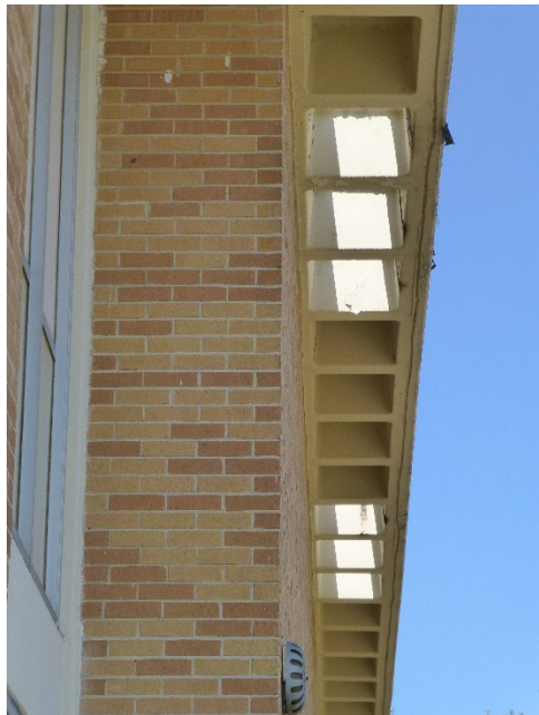
Concrete overhang with perforated waffle.
