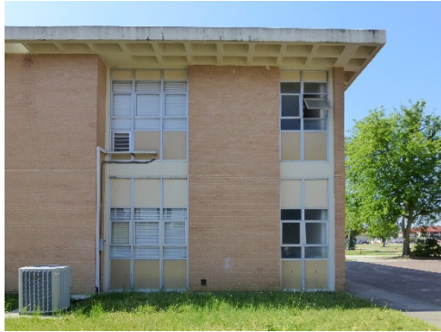
Window bays consisting of bright-aluminum three-pane awning-style windows sandwiched between insulated panels.
