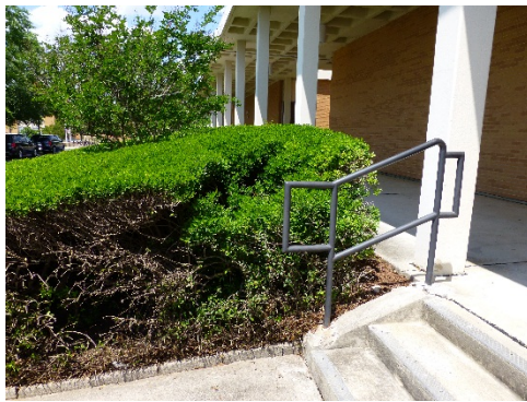
Landscaping surrounding the administration complex and handrails.
