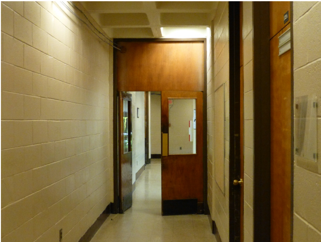
Figure 152. Typical interior wood doors with large pane and wood transom, located in the hallway [left] and typical wood door with wood transom leading into room off hallway [right] (ERDC-CERL, 2015).
