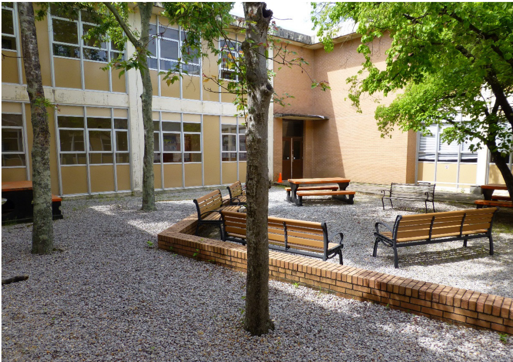
Figure 96. Interior view of the east courtyard in Building 29809, Greely Hall, showing the designed landscape plan of the trees and the brick-sitting wall (ERDC-CERL, 2015).
