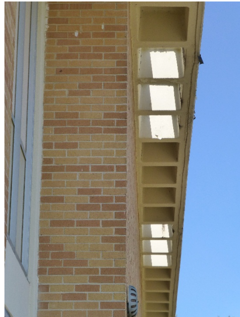
Perforated concrete waffle overhang.
