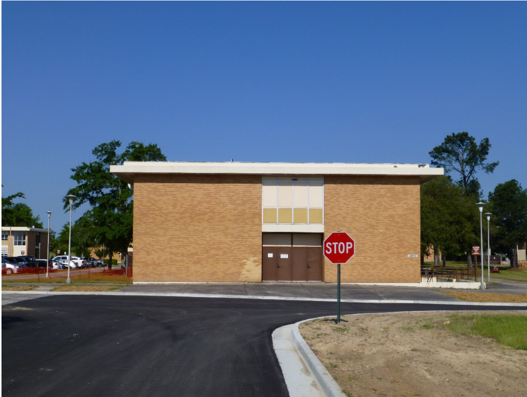
Figure 442. East elevation of Building 29819, Stansell Hall (ERDC-CERL, 2015).
