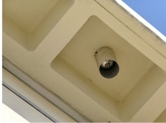
Figure 454. Ceiling-mounted exterior light fixture under waffle overhang - comparison of the original design and materials details drawing from 1966 [left] to the current condition of the light fixture [right] (ERDC-CERL, 2015).
