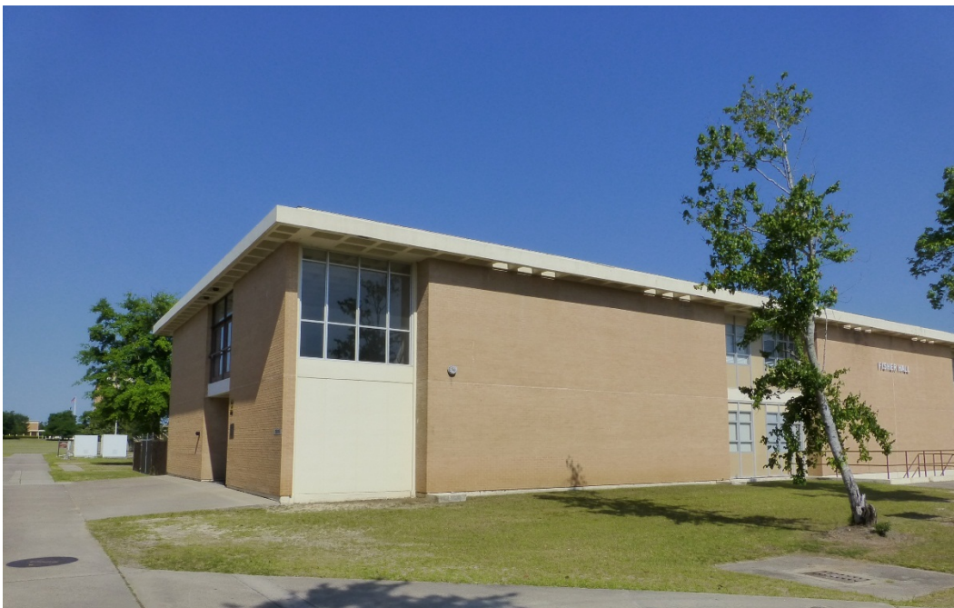
Figure 33. Flat roof construction of Building 29816, Fisher Hall (ERDC-CERL, 2015).
