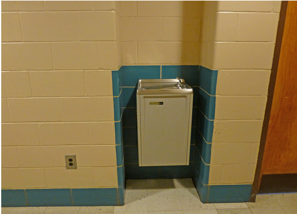
Figure 130. Example of painted, exposed concrete block wall, partial height blue glazed concrete block in drinking fountain alcove, and blue glazed concrete block baseboard in classroom buildings (ERDC-CERL, 2015).
