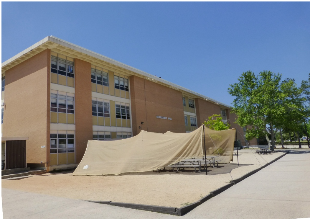
Figure 300. North elevation of Building 29810, Burkhardt Hall (ERDC-CERL, 2015).
