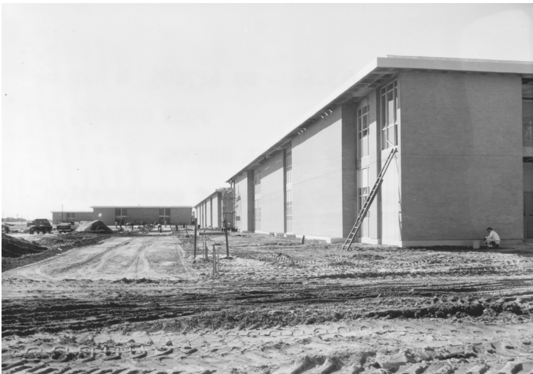
Figure 347. View of the Signal School construction, southeast corner of Building 29818 in the front and Buildings 29813, 29811, and 29809 at back left of photo, March 1966 (National Archives at College Park, MD).
