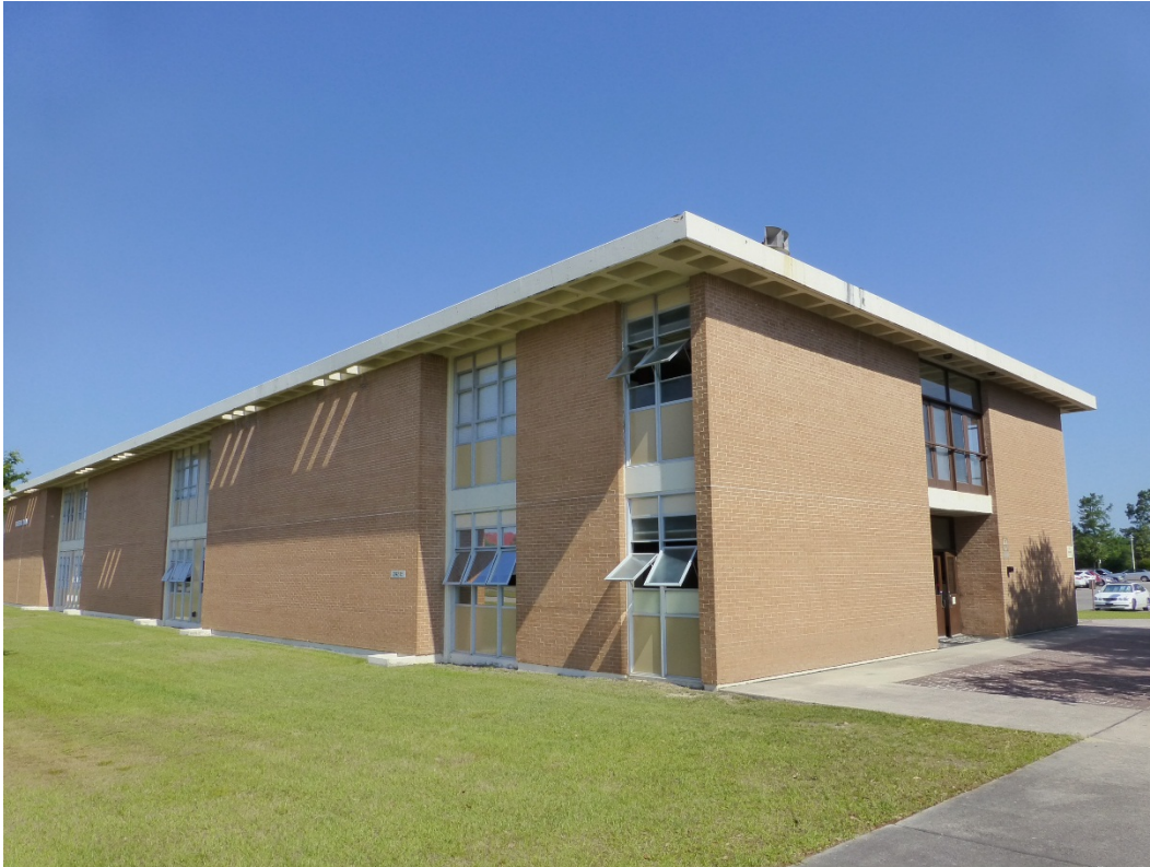
Figure 372. East elevation of Building 29815, Hazen Hall (ERDC-CERL, 2015).
