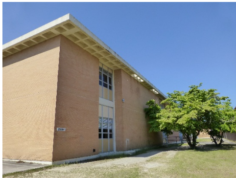
Overall massing, footprint, roof shape, brick veneer, and concrete waffle overhang.
