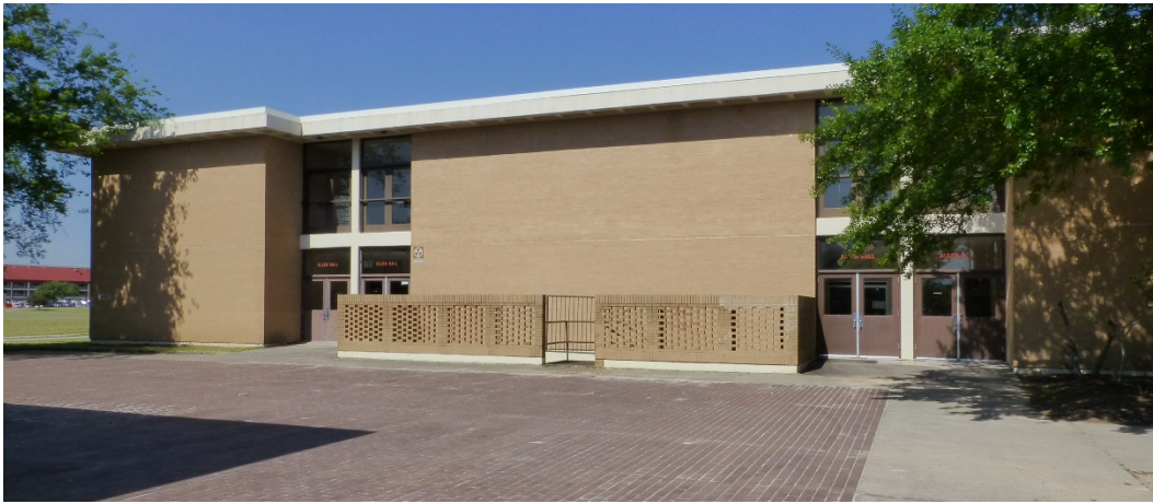
Figure 91. Close-up of the perforated brick wall showing the same type of brick used as the building's brick-veneer exterior wall, Building 29817, Allison Hall (ERDC-CERL 2015).
