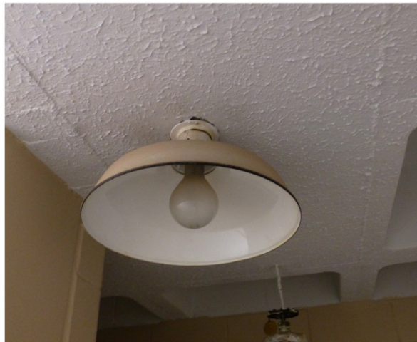
Figure 146. Ceiling-mounted pendant light fixture – comparison of the original design drawing and light fixture type from 1966 [left] to the current condition of the metal ceiling-mounted pendant light fixture [right] (ERDC-CERL, 2015).
