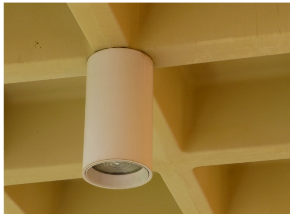
Figure 243. Ceiling-mounted light fixture – Comparison of the original drawing detail from 1966 [left] to the current condition of the ceiling-mounted light fixture under the concrete waffle canopy [right] (ERDC-CERL, 2015).
