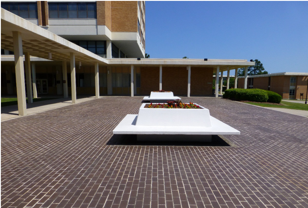
Figure 260. Brick plaza connects Buildings 29805, 29807, and 29808 (ERDC-CERL, 2015).
