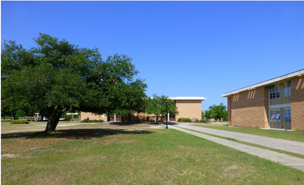
Figure 113. View looking west across the campus plan with Building 29811, Saltzman Hall, on the right and Building 29809, Greely Hall, in the background (ERDC-CERL, 2015).
