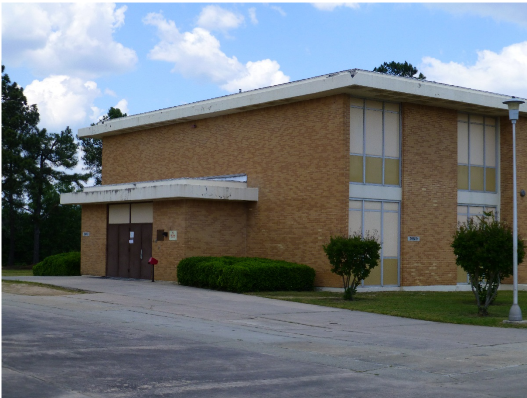
Figure 443. Southwest oblique of Building 29819, Stansell Hall (ERDC-CERL, 2015).
