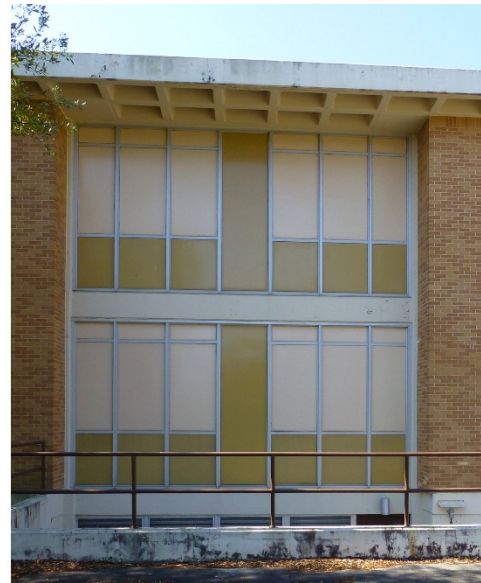
Figure 453. Large window bay on the north elevation – comparison of the original design and materials detail drawing from 1966 [left] to the current condition of the bright-aluminum framed insulated panels separated by exposed concrete structural system [right] (ERDC-CERL, 2015).
