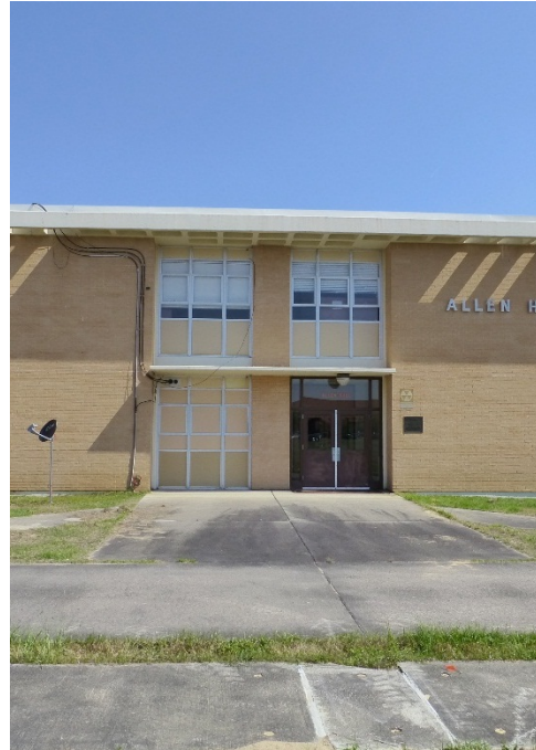
Main entry on the south elevation with groups of three windows, flat concrete canopy, and metal entry doors.
