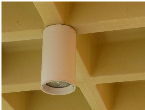
Ceiling-mounted light fixtures.
