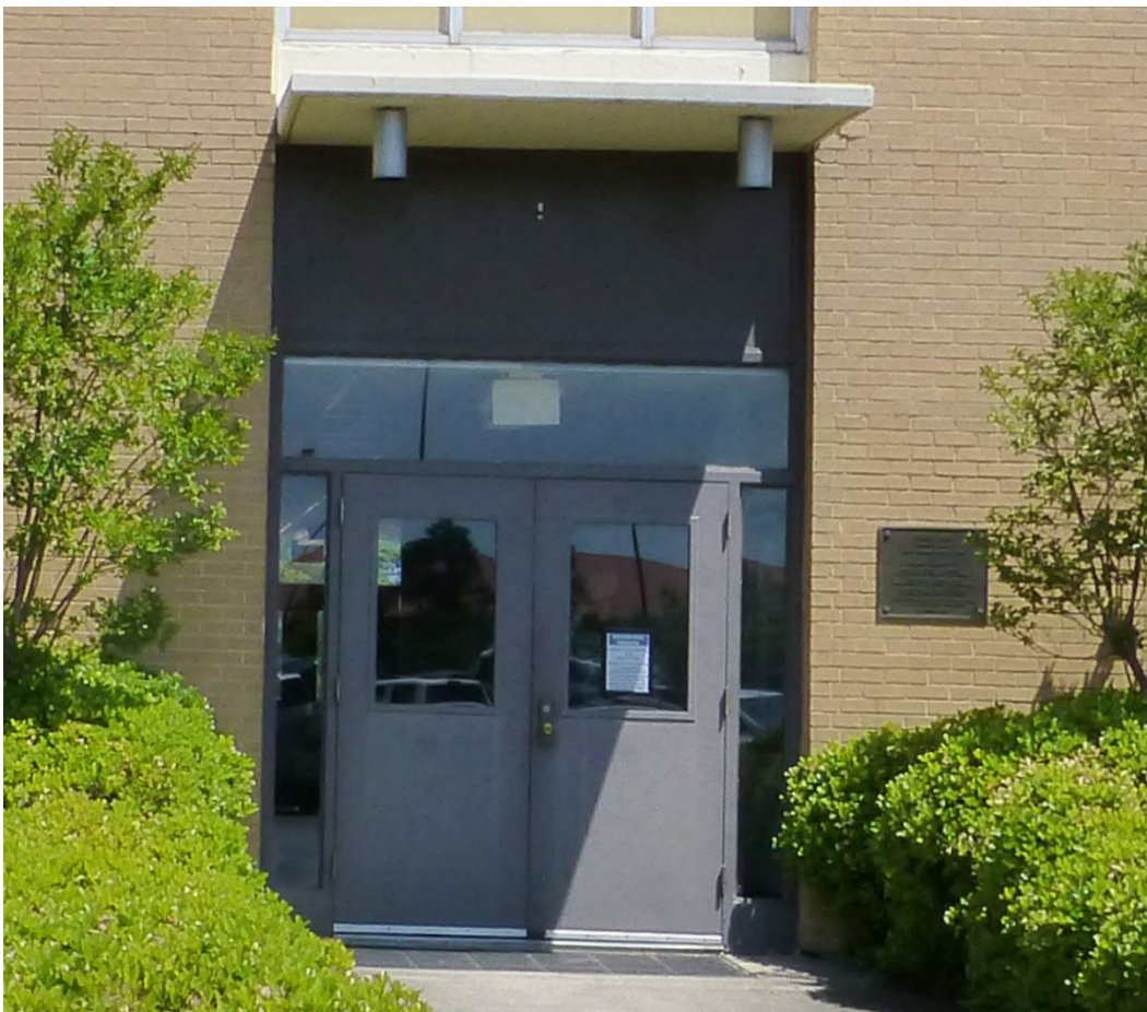
Figure 56. A set of metal doors with pane, sidelights, glass transom, and insulated panel above, Building 29801, Nelson Hall (ERDC-CERL, 2015).
