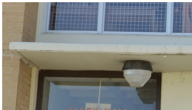
Figure 369. Ceiling-mounted light fixture under flat concrete canopy – comparison of the original design and material from 1966 [left] to the current condition of the replacement ceiling-mounted light fixture [right] (ERDC-CERL, 2015).
