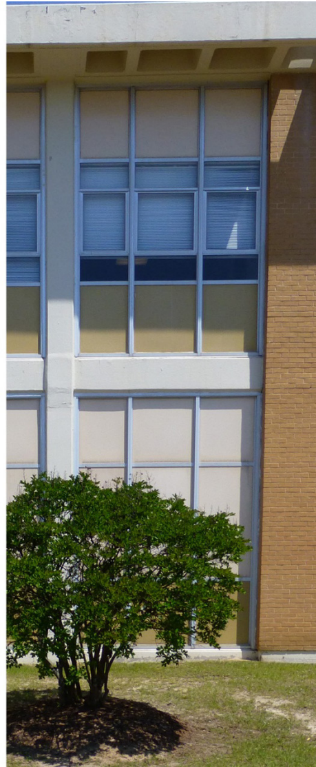
Figure 201. South elevation window bay - comparison of the original drawing detail from 1966 [left] to the current condition of the bright-aluminum awning windows with panel inserts separated by the concrete structure [right] (ERDC-CERL, 2015).
