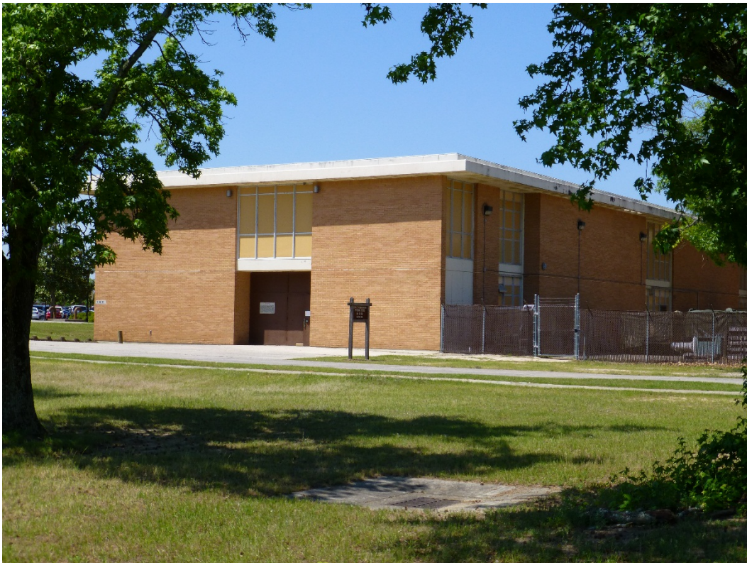
Figure 206. Northeast oblique of Building 29802, Moran Hall south (ERDC-CERL, 2015).
