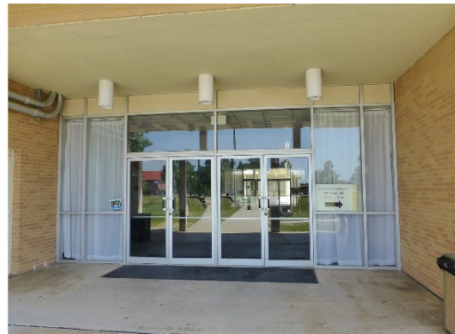
Figure 242. Main entry on the north elevation – comparison of the original drawing detail from 1966 [left] to the current condition of the bright-aluminum and plate-glass doors, sidelights, and transoms [right] (ERDC-CERL, 2015).
