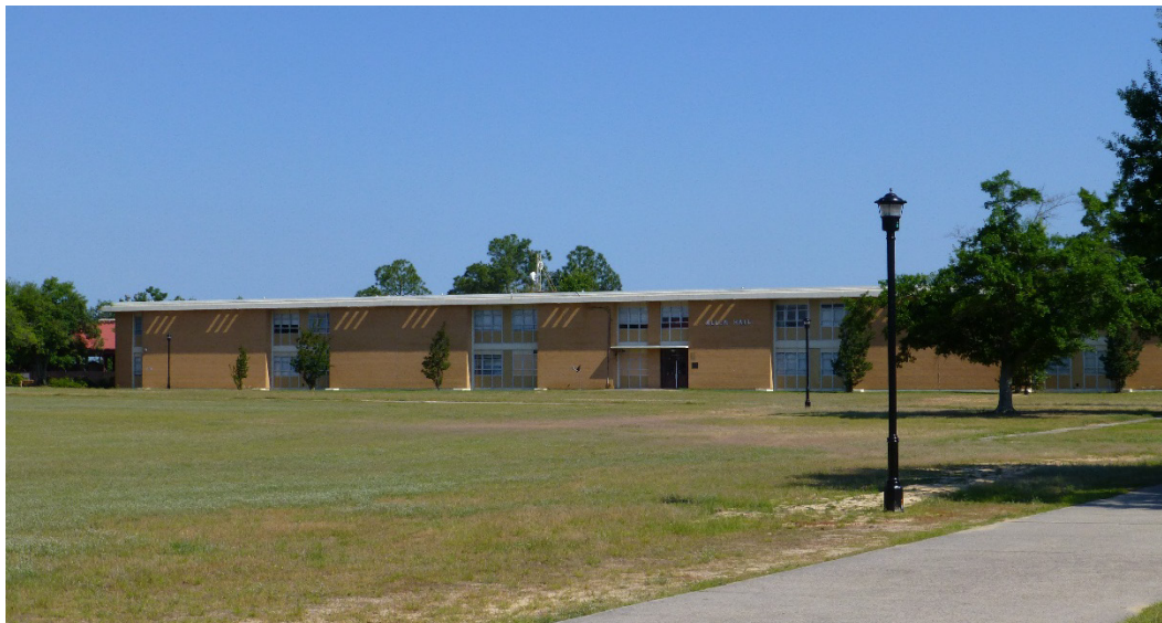
Figure 343. South elevation of Building 29813, Allen Hall (ERDC-CERL, 2015).
