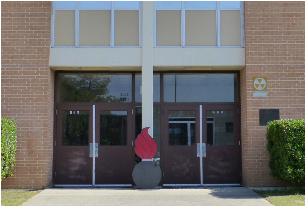
Figure 57. Two sets of metal doors with pane and transoms above separated by exposed concrete structure, Building 29815, Hazen Hall (ERDC-CERL, 2015).
