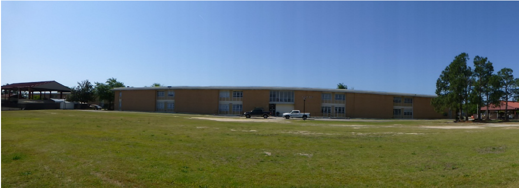
Figure 344. North elevation of Building 29813, Allen Hall (ERDC-CERL, 2015).
