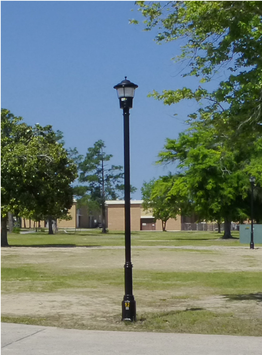
Figure 120. An example of one type of the replacement sidewalk lights (ERDC-CERL, 2015).
