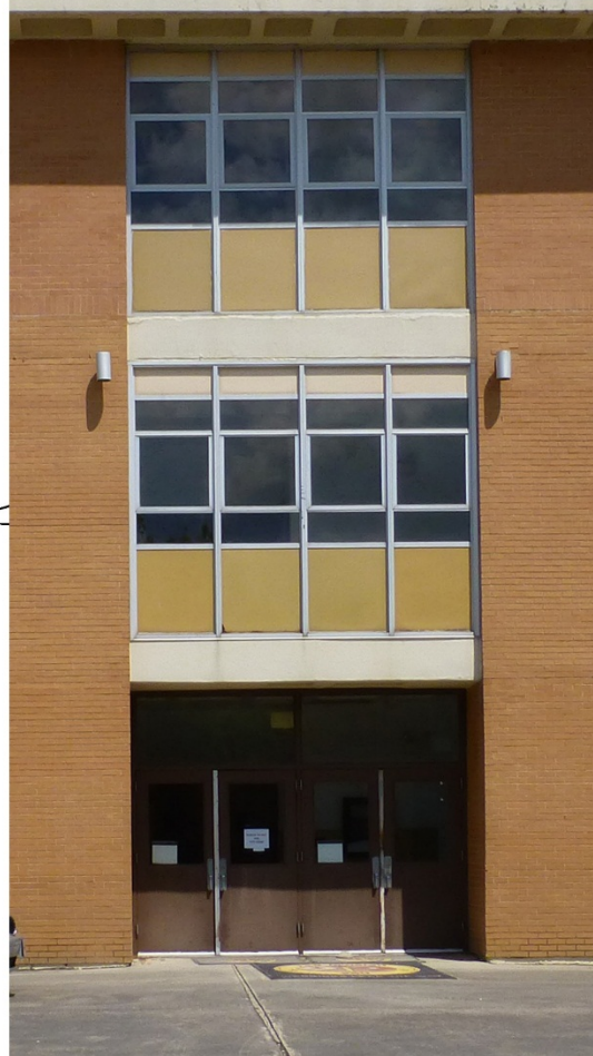
Figure 309. Entry bays on the east and west elevations – comparison of the original design 5 and materials from 1966 [left.] to the current condition of the three-story entry bay with metal doors with pane and transom above and groups of four bright-aluminum framed three-pane awning-style windows sandwiched between insulated panels [right] (ERDC-CERL, 2015).
