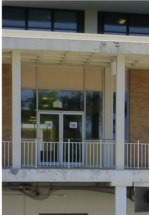
Bright aluminium and plate-glass entry doors.
