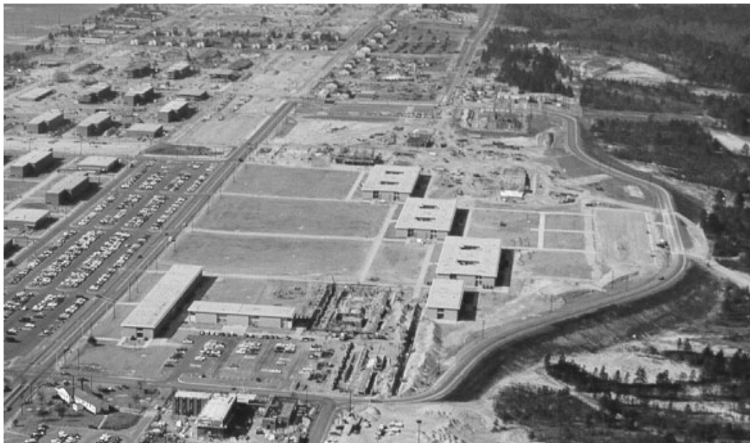
Figure 7. Aerial view of the Signal School Campus, with the completion of the six Phase I classroom buildings (light rectangular roofs in photo's center), the beginning construction of Phase II, 1968 (barracks buildings at center left of photo) and the construction of Building 33800 (bottom center) (Signal Corps Historian Office).
