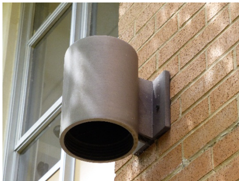
Wall-mounted bronze light fixtures located near secondary entries at the end of the rectangular classroom wings.
