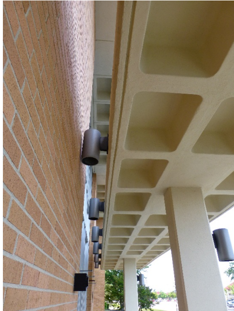
Concrete waffle canopy near main entry.
