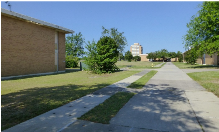
Figure 118. Looking west toward Building 29808, Signal Towers, at some of the connecting sidewalks (ERDC-CERL, 2015).
