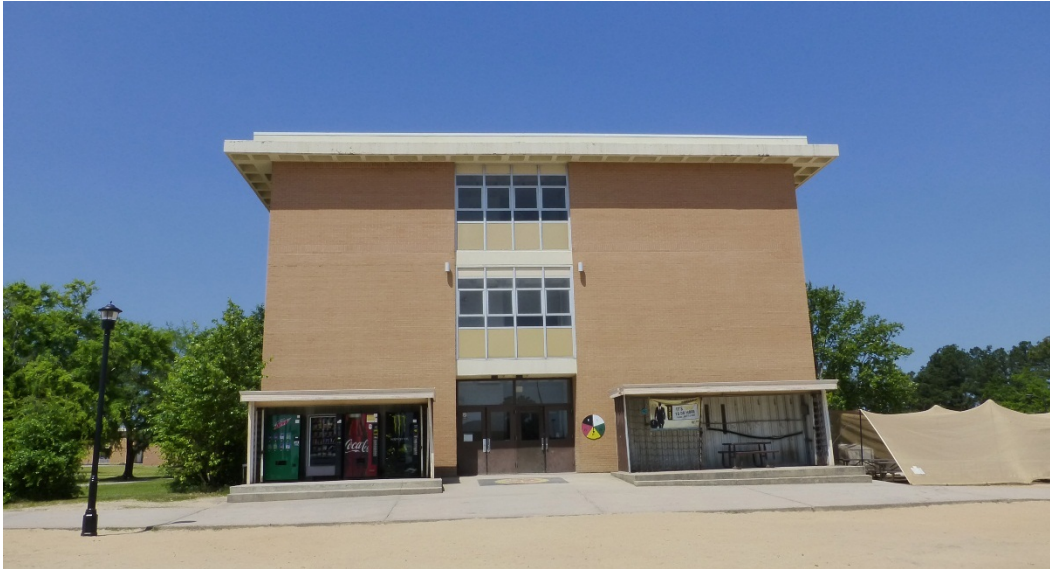
Figure 32. Flat roof construction of Building 29810, Burkhardt Hall (ERDC-CERL, 2015).
