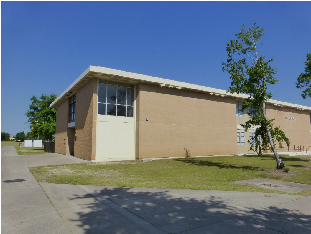
Figure 387. Southeast oblique of Building 29816, Fisher Hall (ERDC-CERL, 2015).
