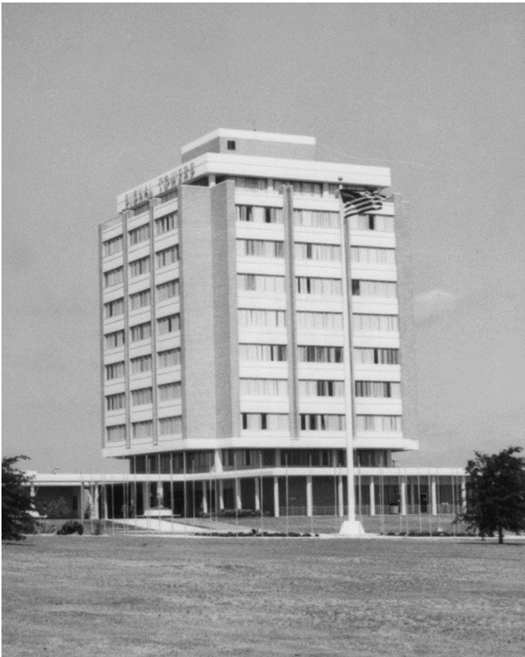
Figure 263. Building 29808, Signal Towers, April 1978 (National Archives at College Park, MD).
