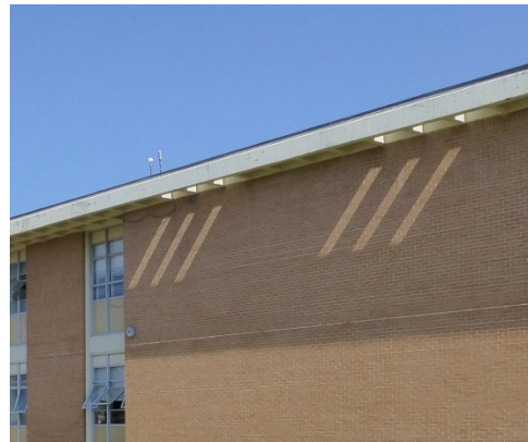
"Light pattern" created by the perforated concrete waffle overhang.
