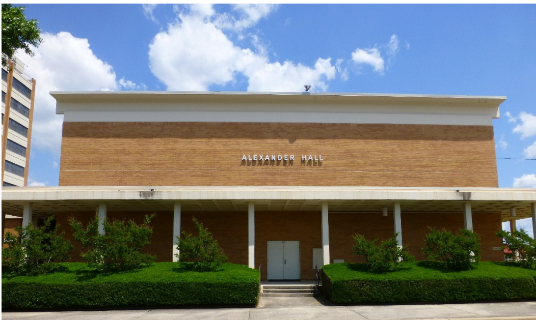
Figure 27. Rectangular massing, Building 29805, Alexander/Olmsted Halls (ERDC-CERL, 2015).
