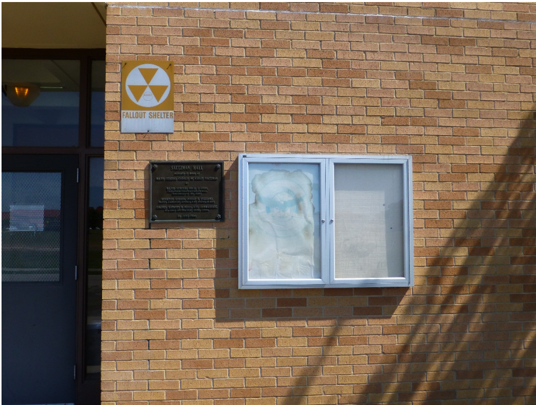
Figure 84. Bright-aluminum exterior display case, Building 29811, Saltzman Hall (ERDC-CERL, 2015).
