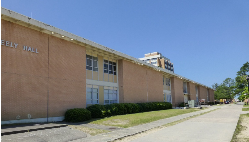
Figure 274. North elevation of Building 29809, Greely Hall (ERDC-CERL, 2015).
