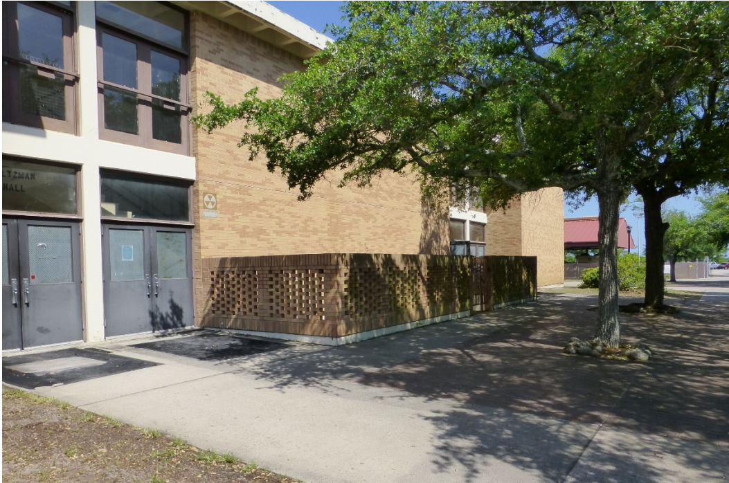
Figure 315. East elevation of Building 29811, Saltzman Hall (ERDC-CERL, 2015).
