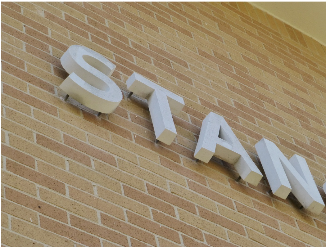
Figure 82. Close-up of the uniform lettering, Building 29819, Stansell Hall (ERDC-CERL, 2015).
