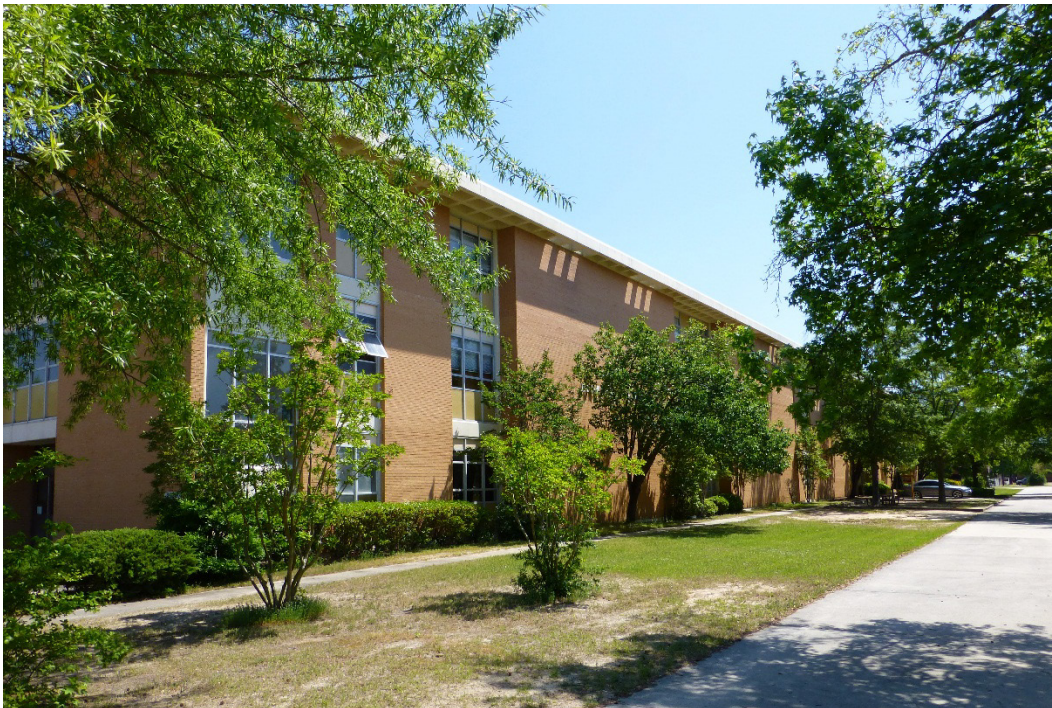
Figure 101. Landscaping between Building 29810, Burkhardt Hall, and the sidewalk (ERDC-CERL, 2015).
