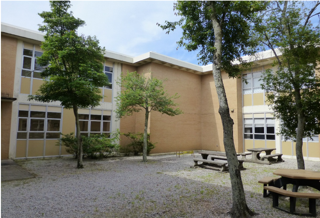
Figure 93. Interior view of the east courtyard in Building 29813, Allen Hall, showing the designed landscape of the four trees placed within the courtyard (ERDC-CERL 2015).
