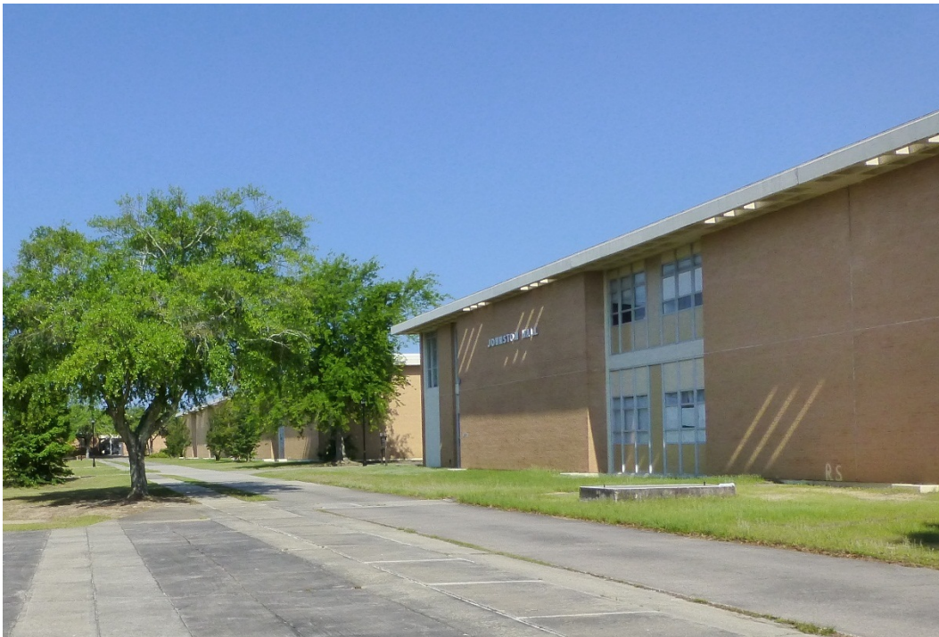
Figure 426. Left side of the south elevation of Building 29818, Johnston Hall (ERDC-CERL, 2015).
