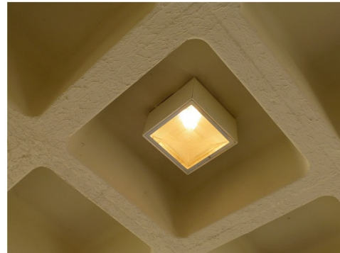
Figure 148. Ceiling-mounted pendant light fixture – comparison of the original design drawing and light fixture type from 1966 [left] to the current condition of the replacement ceiling-mounted light fixture [right] (ERDC-CERL, 2015).
