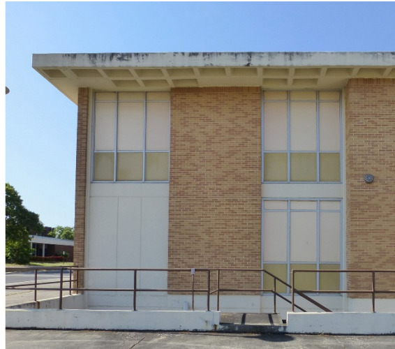
Figure 452. Northeast window bays – comparison of the original design and materials detail drawing from 1966 [left] to the current condition of the concrete panels and bright-aluminum framed insulated panels [right] (ERDC-CERL, 2015).
