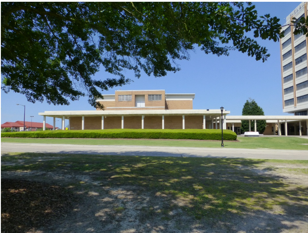
Figure 227. East elevation of Building 29805, Alexander/Olmstead Halls (ERDC-CERL, 2015).
