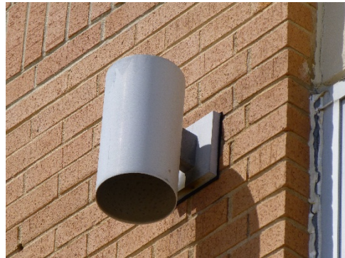
Wall-mounted light fixtures on the east and west elevations.
