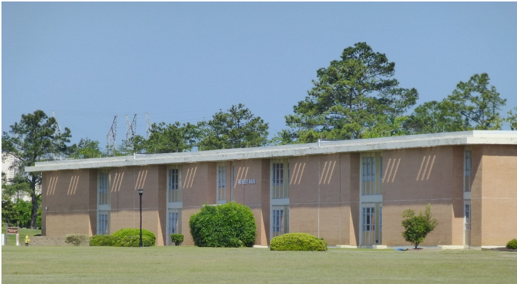
Figure 28. Rectangular massing, Building 29809, Greely Hall (ERDC-CERL, 2015).
