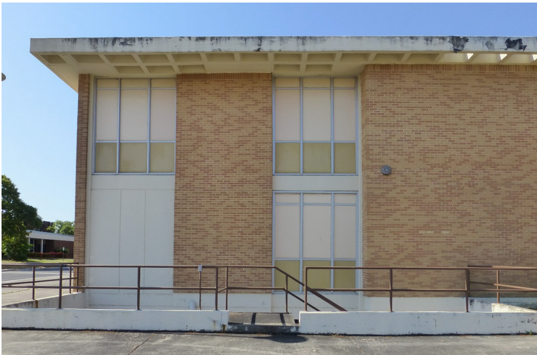
Figure 51. Some of the Signal School buildings were designed with bays of insulated panel inserts, for example Building 29819, Stansell Hall (ERDC-CERL, 2015).
