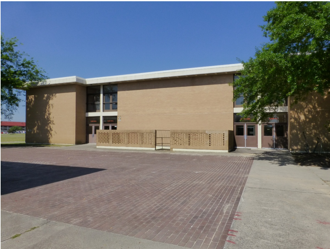
Figure 345. East elevation of Building 29813, Allen Hall (ERDC-CERL, 2015).
