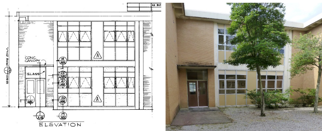
Figure 366. North wall of the right courtyard comparison of the original design and materials from 1964 [left] to the present-day [right] (ERDC-CERL, 2015).
