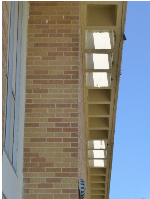
Perforated concrete waffle overhang.
