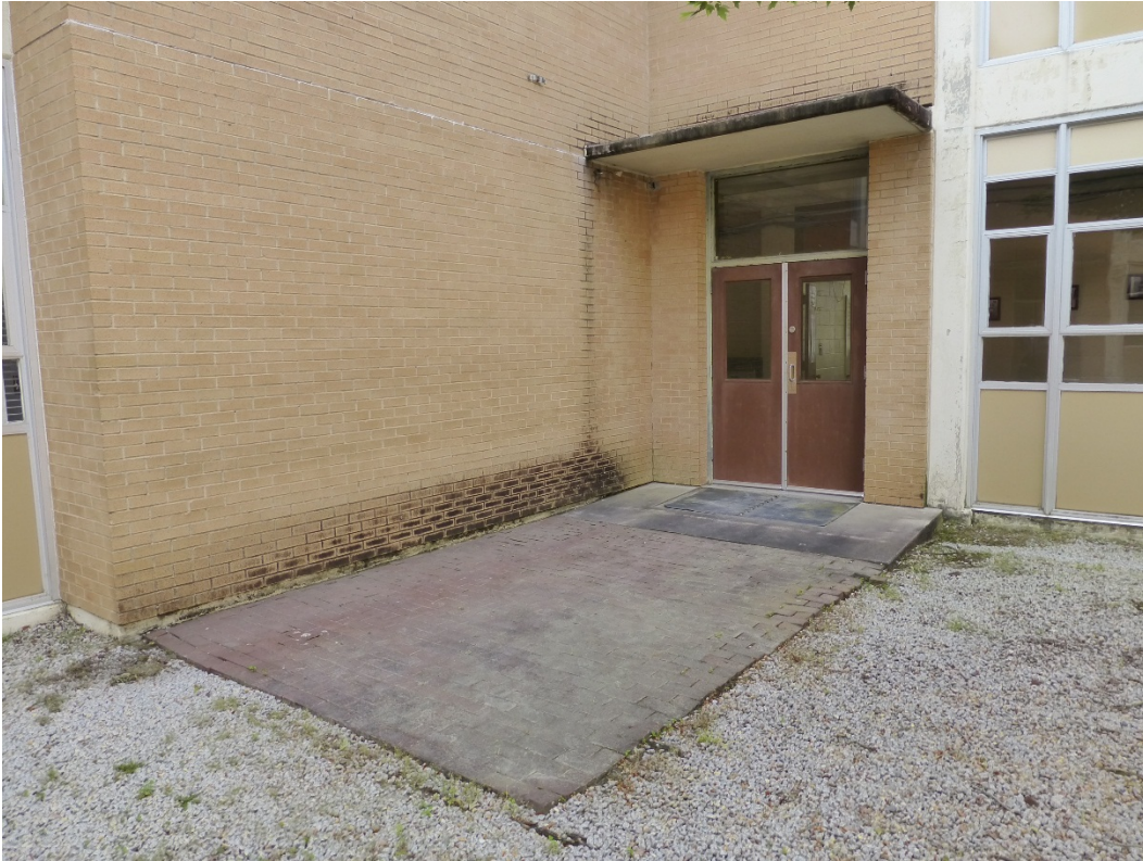
Figure 97. Brick paved area located in front of a courtyard entry (ERDC-CERL, 2015).
