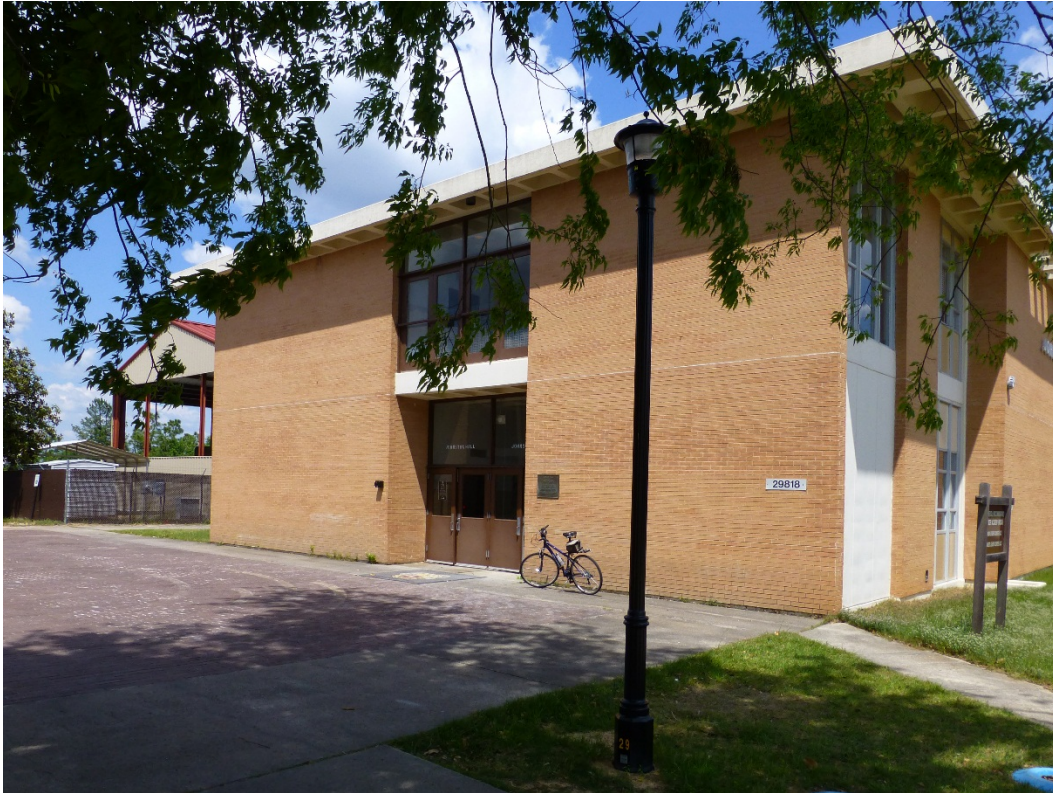
Figure 425. Southwest oblique, Johnston Hall (ERDC-CERL, 2015).
