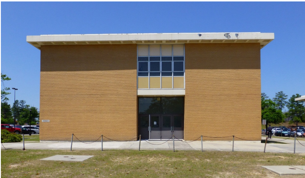
Figure 192. East elevation of Building 29801, Nelson Hall (ERDC-CERL, 2015).
