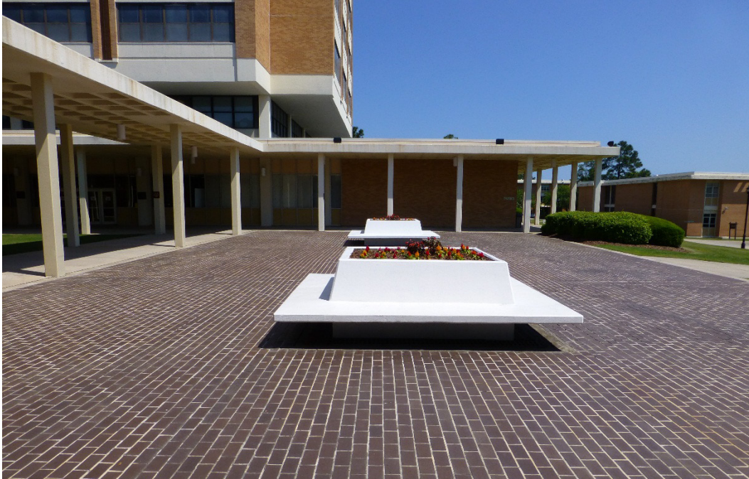
Figure 107. Designed brick plaza that connects the main administration buildings together, Buildings 29805, Alexander Hall/Olmsted Hall; 29807, Conrad Hall; and 29808, Signal Towers; and the concrete planter bench located in the middle of the plaza (ERDC-CERL, 2015).
