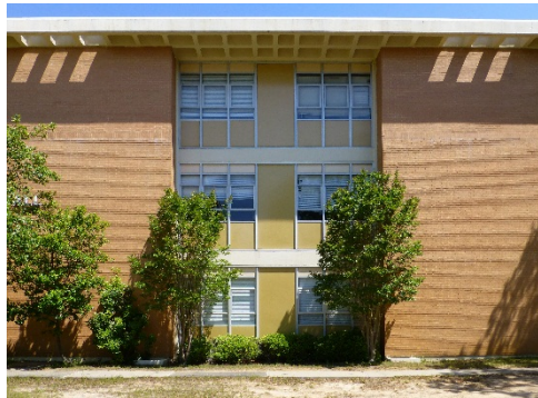
“Light pattern” created on the third-floor brick wall from the perforated waffle overhang.
