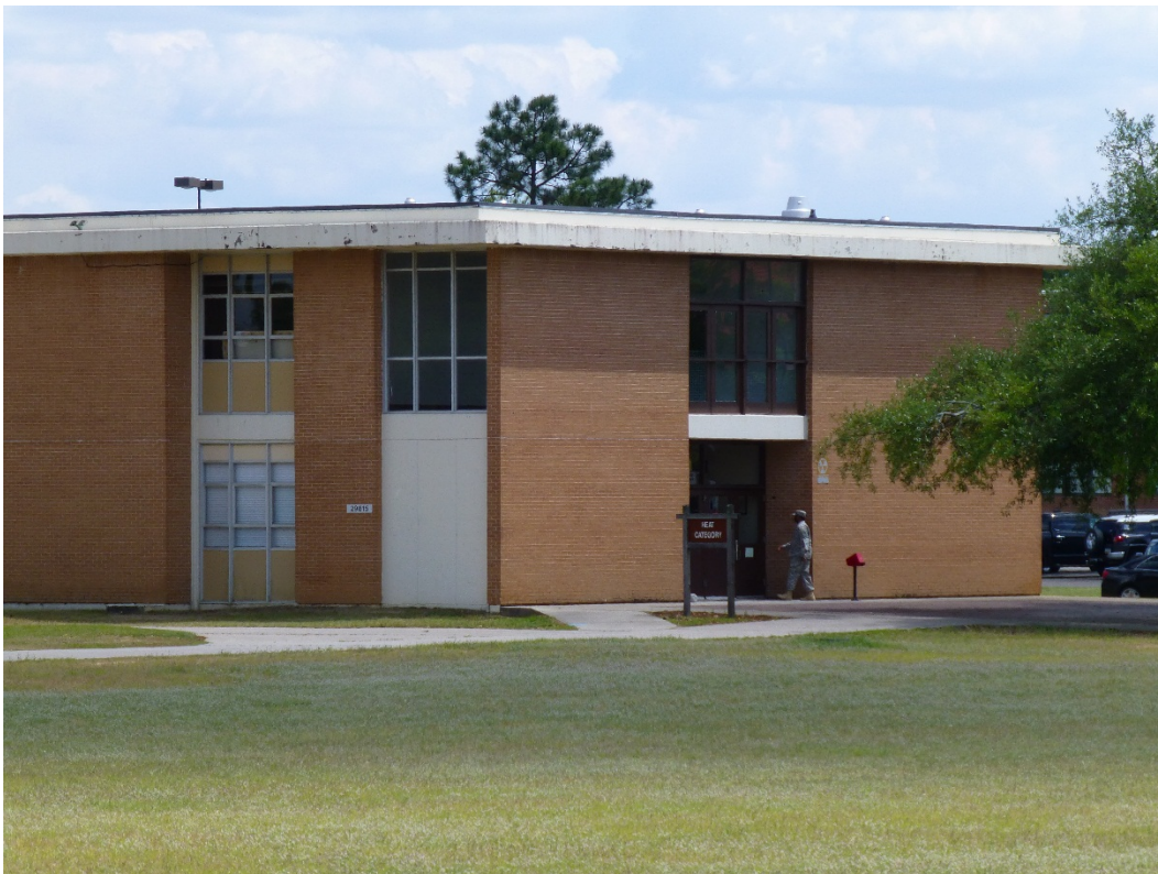
Figure 373. West elevation of Building 29815, Hazen Hall (ERDC-CERL, 2015).
