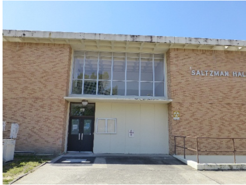
Entry bay on north elevation with concrete panels, metal doors, flat concrete canopy, and fixed windows framed with bright-aluminum sashes.
