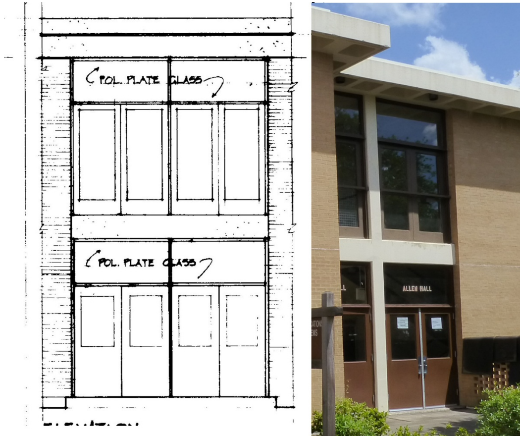
Figure 365. Doors on the east and west elevations – comparison of the original design and materials from 1964 [left] to the current condition of the metal doors with pane and transoms on the first floor and the metal and plate-glass doors with security bars on the second floor [right] (ERDC-CERL, 2015).
