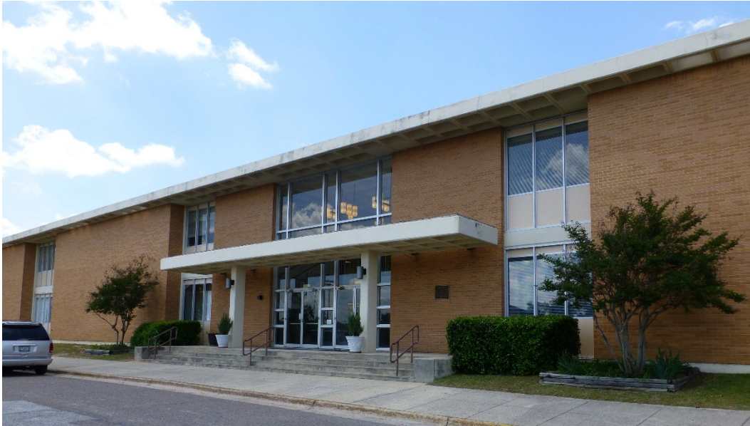
Figure 175. Building 25810, Brant Hall, south [front] elevation (ERDC-CERL, 2015).
