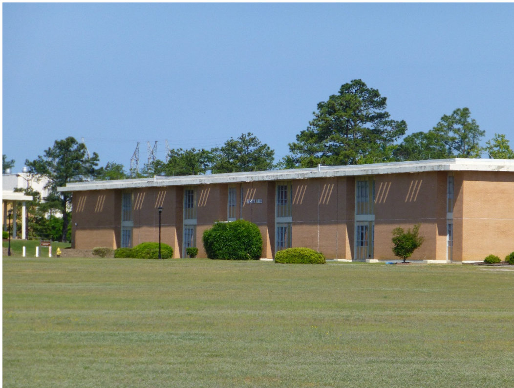
Figure 273. South elevation of Building 29809, Greely Hall (ERDC-CERL, 2015).
