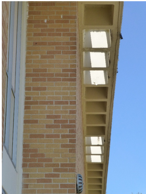
Perforated concrete waffle overhang.
