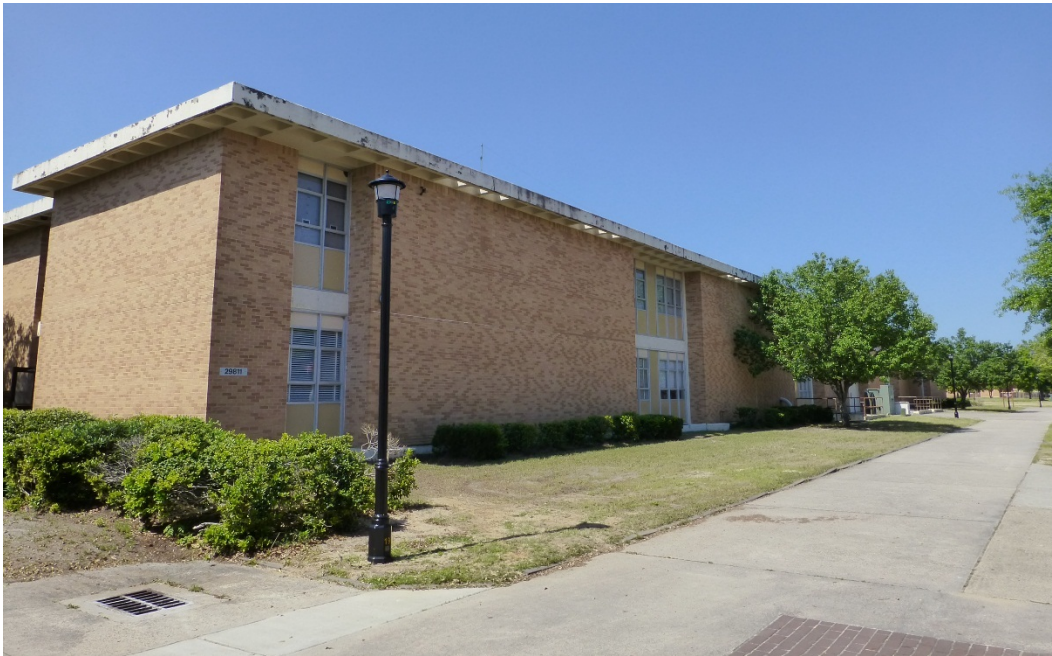
Figure 313. Left side of the south elevation of Building 29811, Saltzman Hall (ERDC-CERL, 2015).
