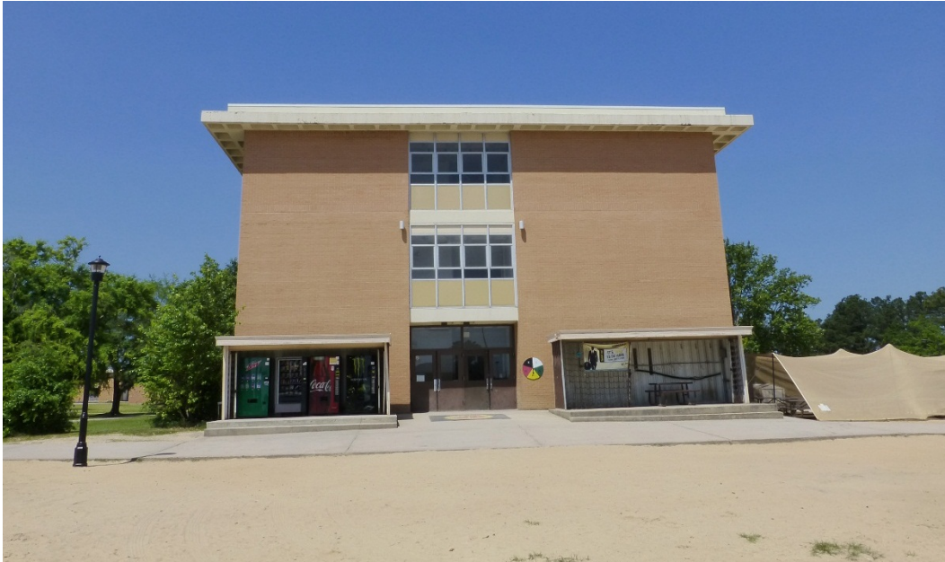
Figure 301. East elevation of Building 29810, Burkhardt Hall (ERDC-CERL, 2015).
