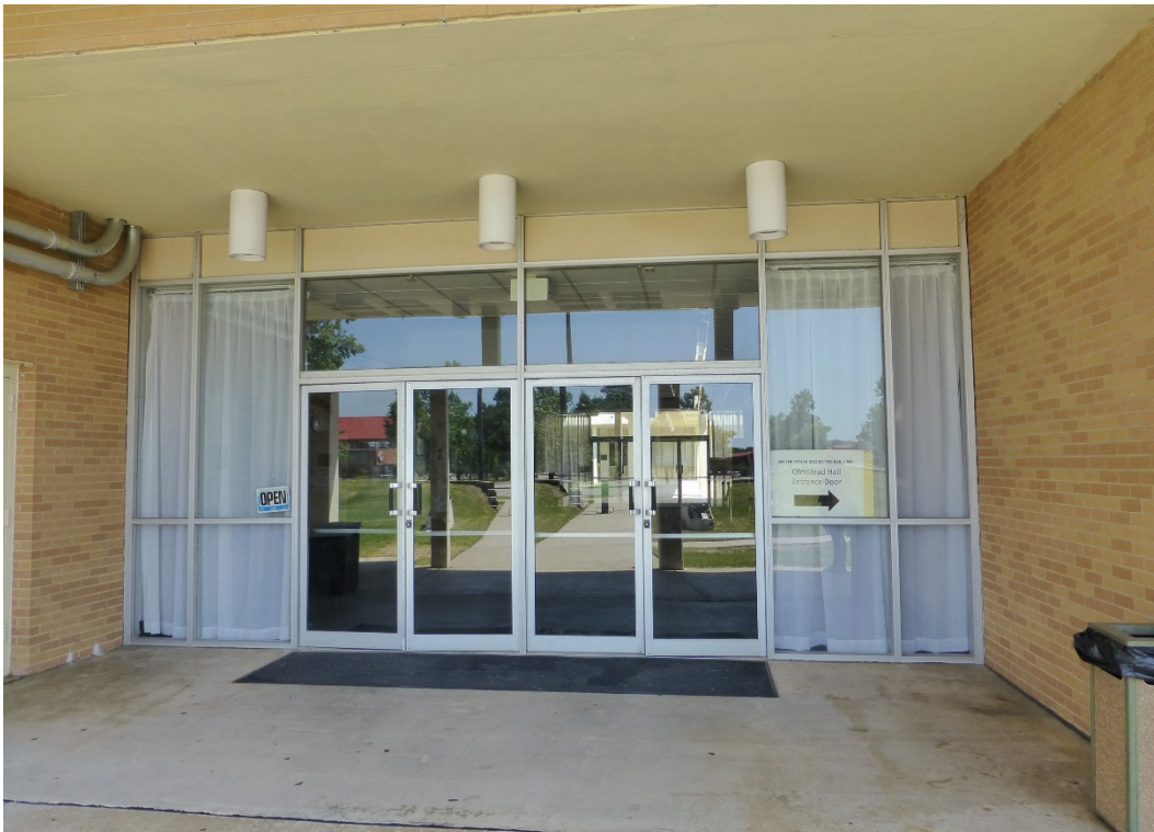
Figure 229. Bright-aluminum and plate-glass doors, sidelights, and transoms on the north elevation leading into the lobby of Building 29805 (ERDC-CERL, 2015).
