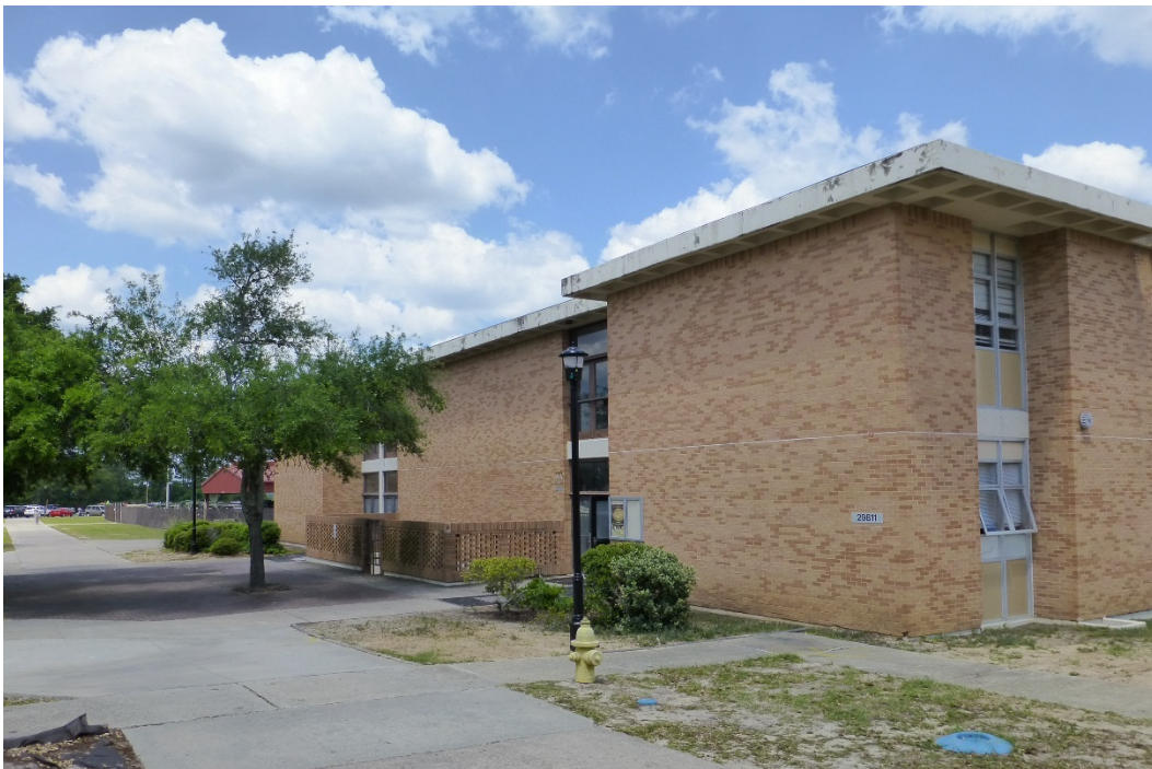
Figure 316. West elevation of Building 29811, Saltzman Hall (ERDC-CERL, 2015).
