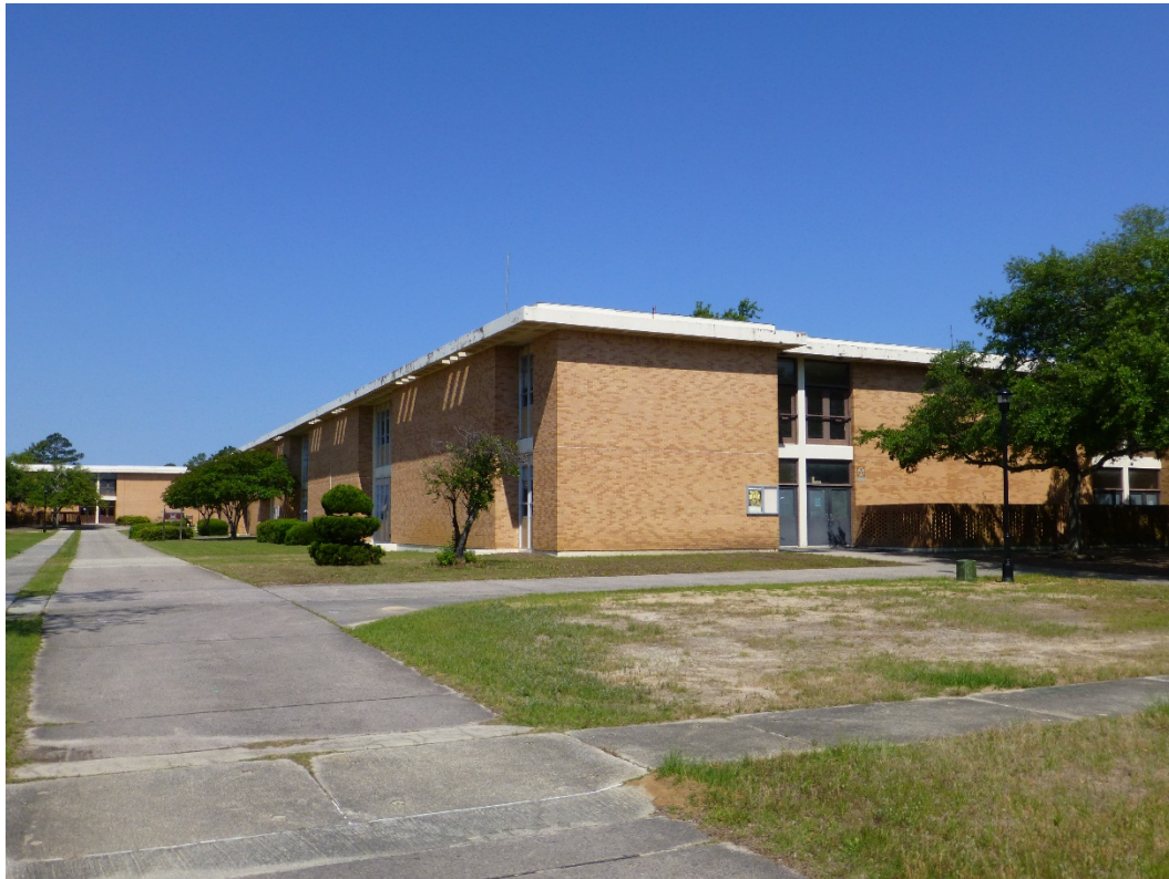
Figure 312. Southeast corner of Building 29811, Saltzman Hall, (ERDC-CERL, 2015).
