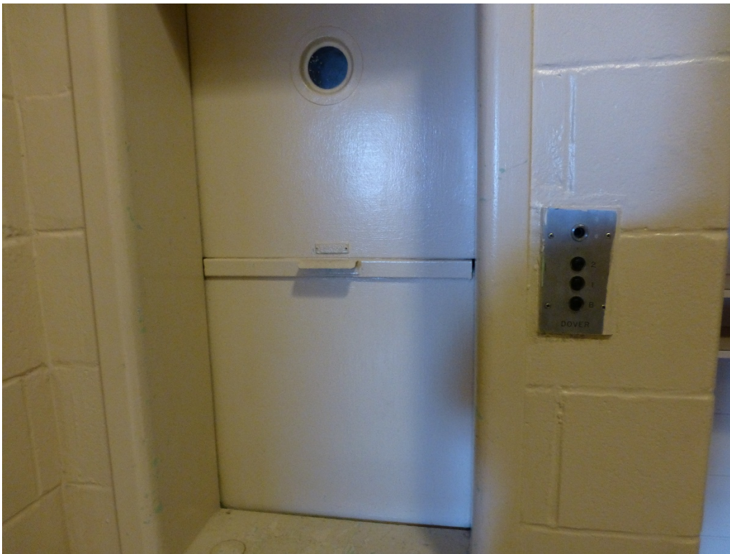
Figure 166. Example of an original dumbwaiter in the classroom buildings (ERDC-CERL, 2015).
