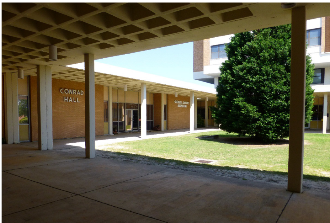
Figure 246. Looking at the main entry into Building 29807, Conrad Hall on the east elevation (ERDC-CERL, 2015).
