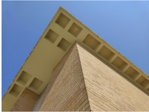
Concrete waffle overhang.
