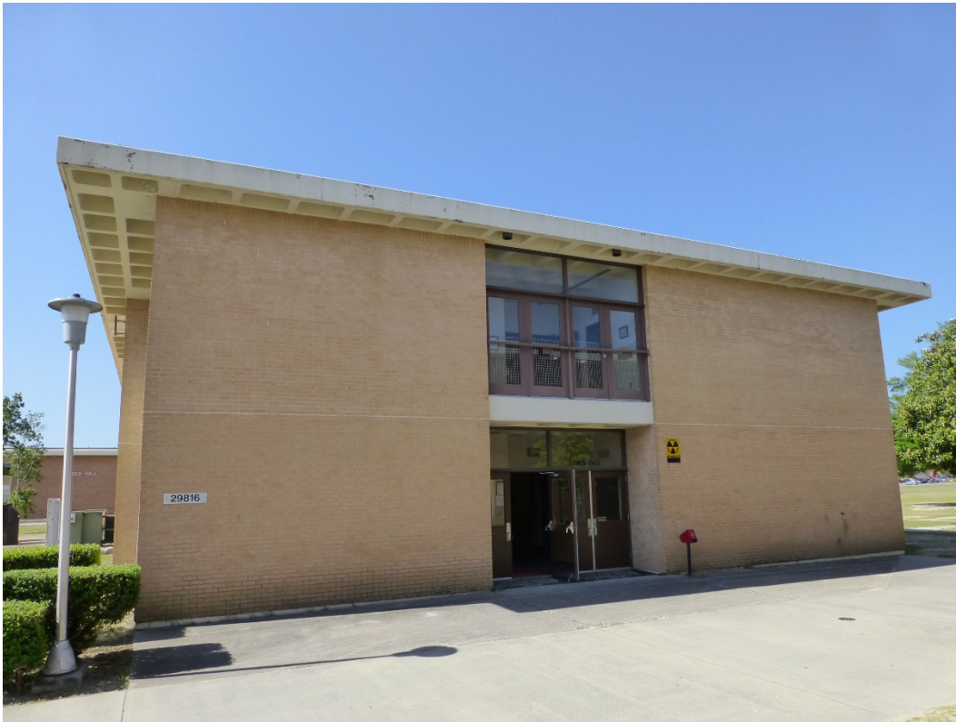
Figure 390. North elevation of Building 29816, Fisher Hall (ERDC-CERL, 2015).
