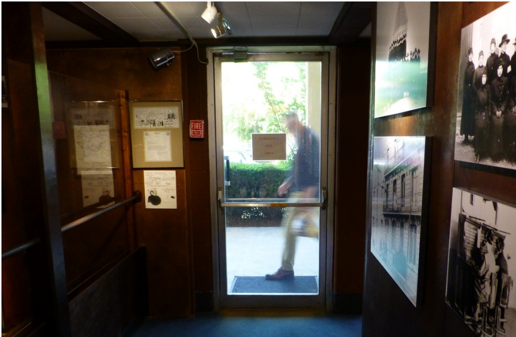
Figure 251. Building 29807, single-entry bright-aluminum and plate-glass door (ERDC-CERL, 2015).
