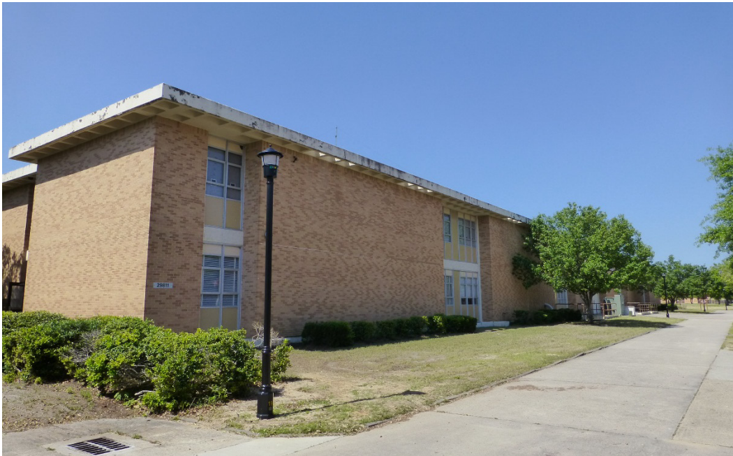
Figure 30. Two-story classroom building, Building 29811, Saltzman Hall (ERDC-CERL, 2015).
