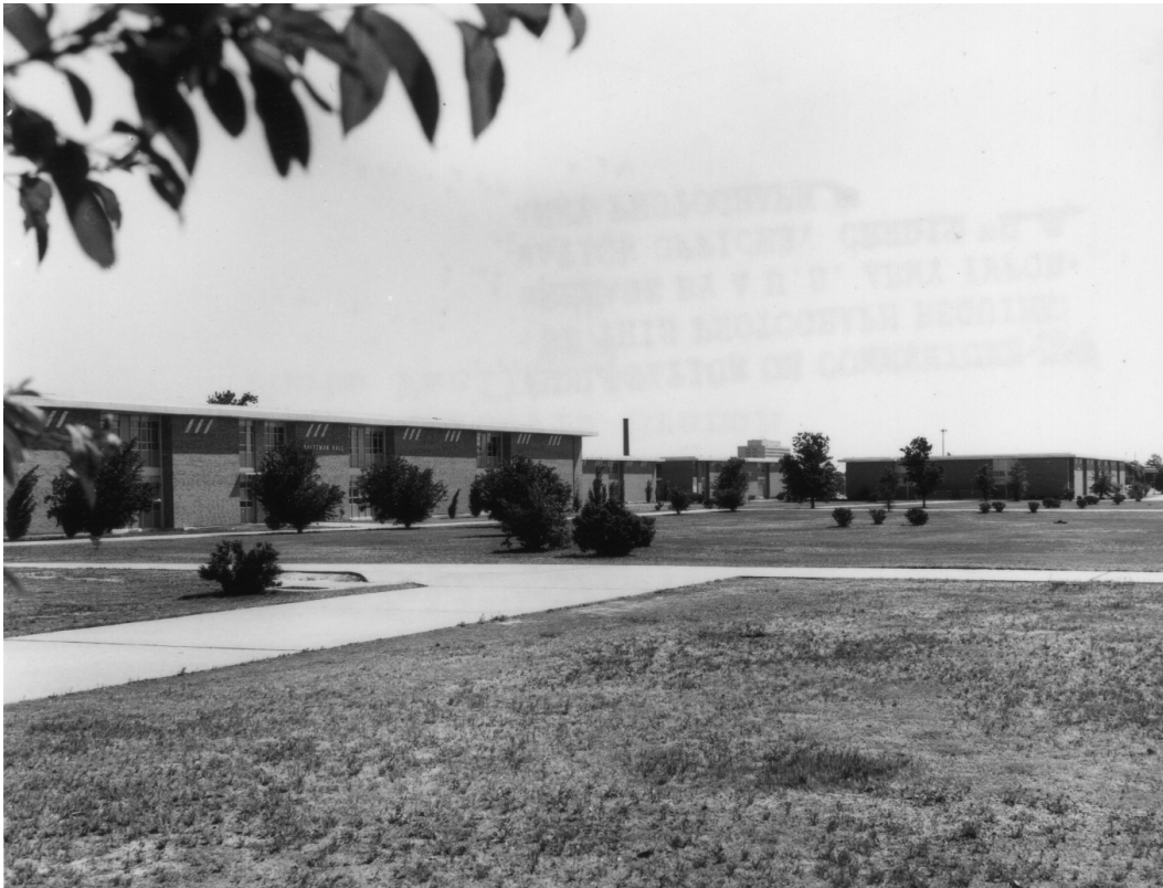
Figure 319. View looking northeast, Building 29811 is on the left and Building 29817 is on distant right, April 1978 (National Archives at College Park, MD).
