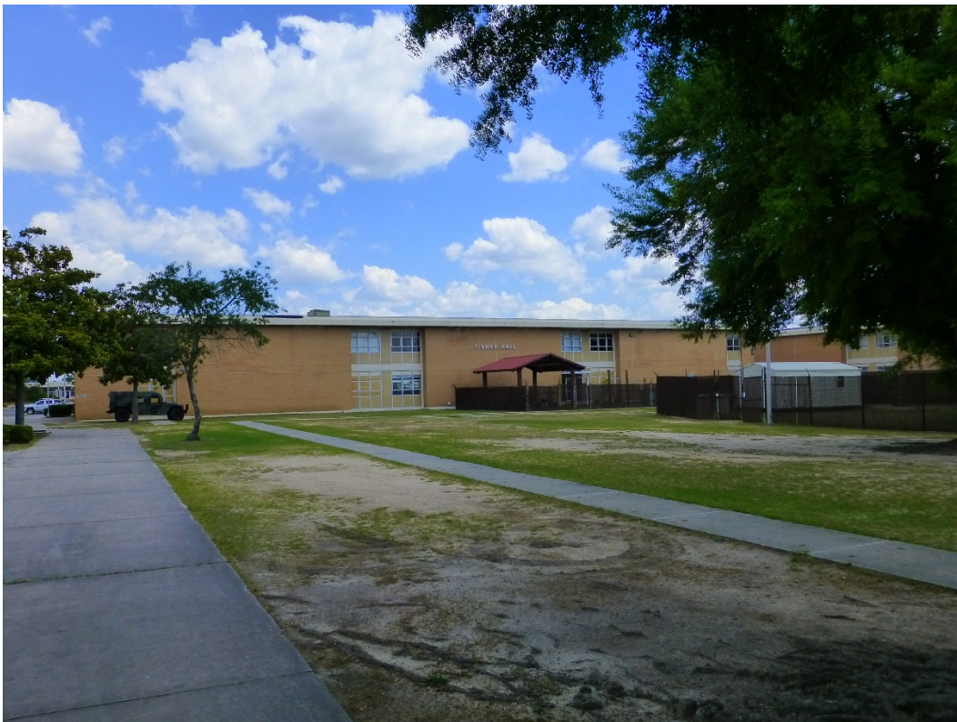
Figure 391. West elevation of Building 29816, Fisher Hall (ERDC-CERL, 2015).
