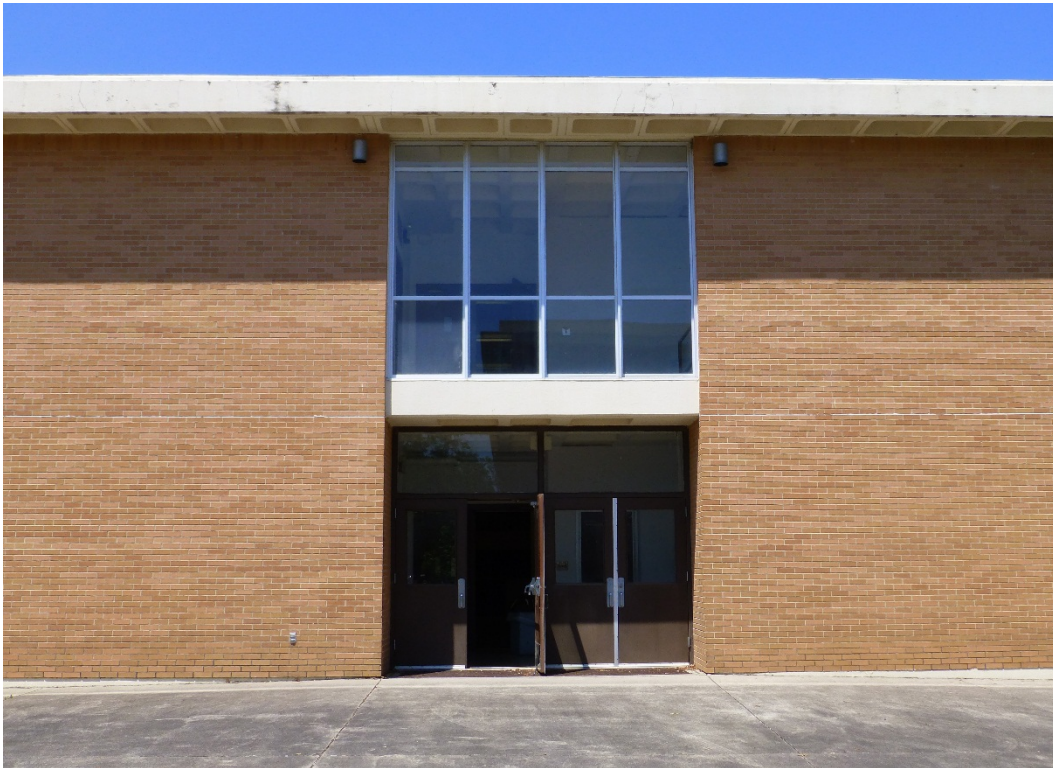
Figure 215. East entry for Building 29803, Moran Hall north (ERDC-CERL, 2015).
