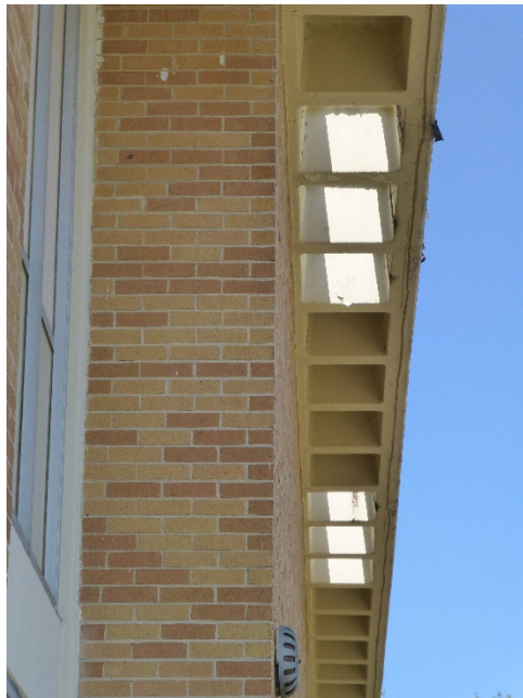
Perforated concrete waffle overhang.
