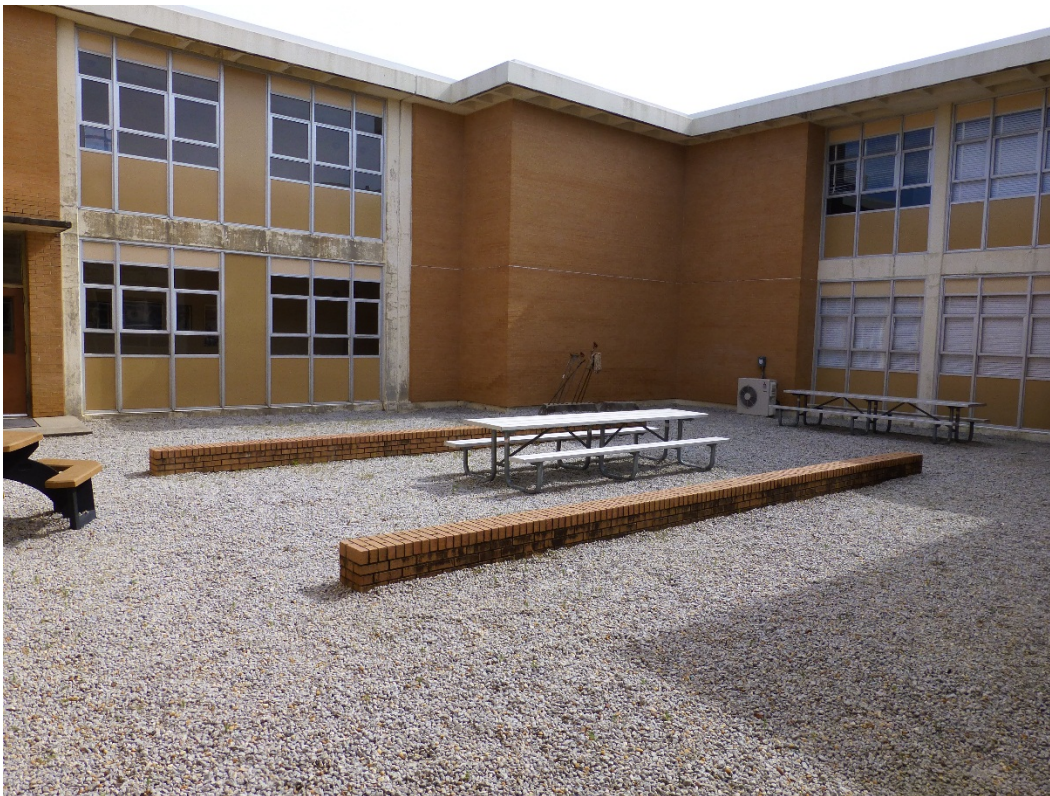
Figure 92. Interior view of the west courtyard in Building 29813, Allen Hall, showing the window bays and parallel brick sitting walls. Note the absence of vegetation that has been removed and replaced with gravel infill (ERDC-CERL, 2015).
