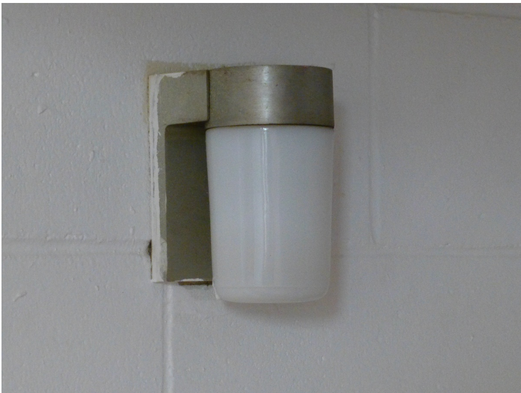
Figure 144. Typical original wall-mounted light fixture (ERDC-CERL, 2015).
