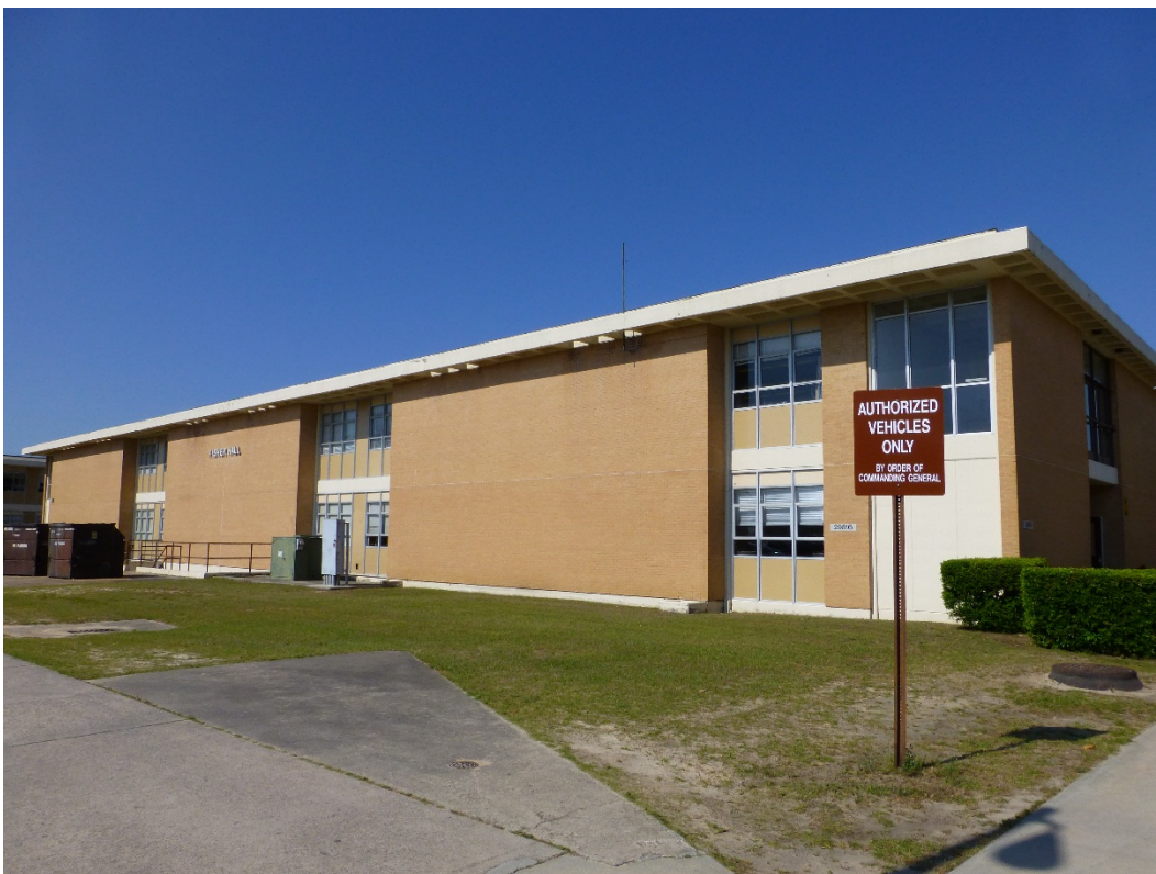
Figure 389. East elevation of Building 29816, Fisher Hall (ERDC-CERL, 2015).
