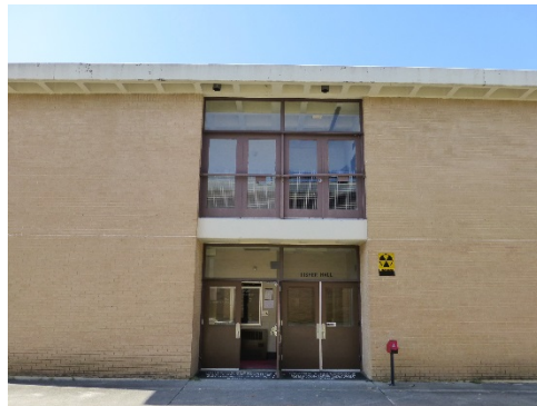
Metal doors with pane and transom on first floor and metal and plate glass doors on second floor, separated by exposed concrete structural system.
