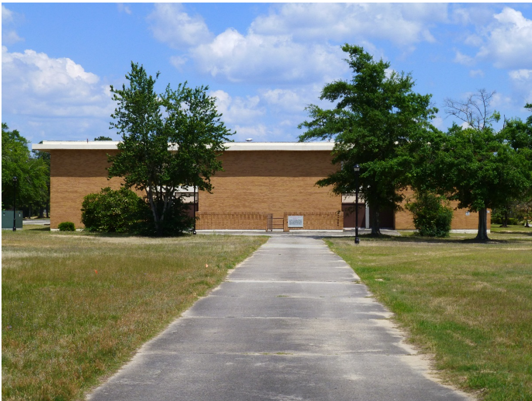
Figure 406. West elevation of Building 29817, Allison Hall (ERDC-CERL, 2015).
