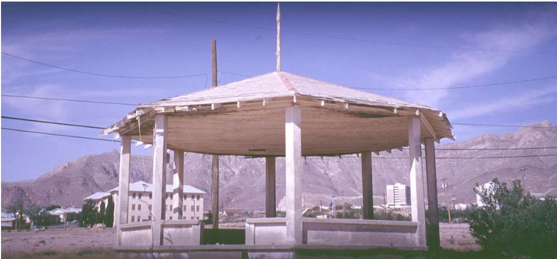
Photograph 1. Exterior photograph of Building 7122 (bandstand).
