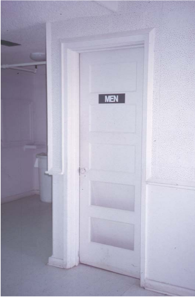
Photograph 18. Theater washroom door vent detail.
