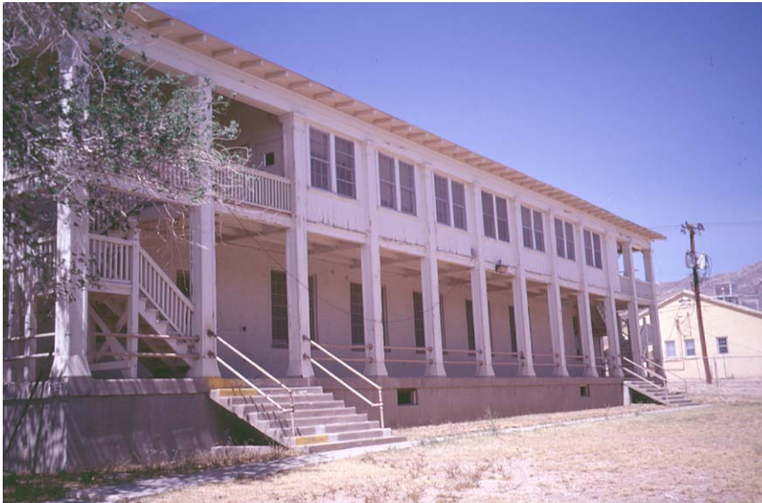
Photograph 41. Non-historic second-story barracks porch enclosure.
