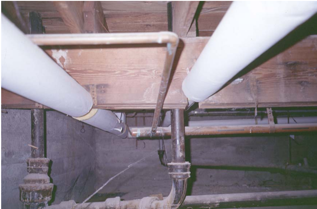
Photograph 75. Notched floor beam in Conference Center crawlspace.
