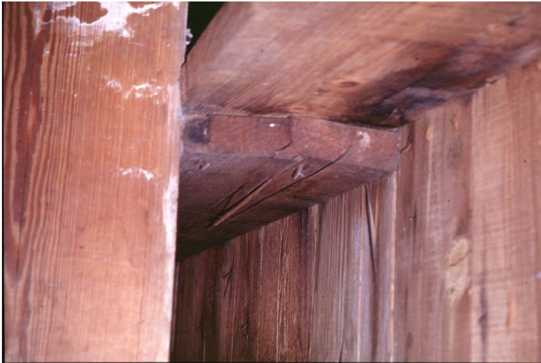
Photograph 55. Detail of Building 7159 floor joists.
