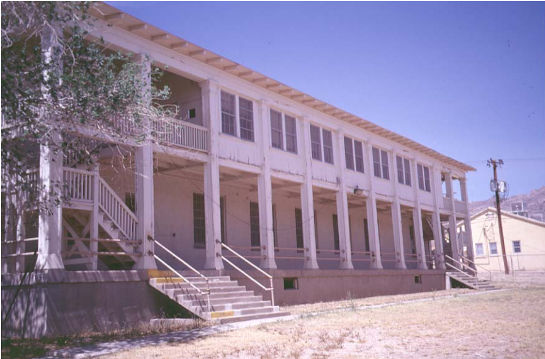
Photograph 32. Exterior photograph of Building 7157 (barracks).
