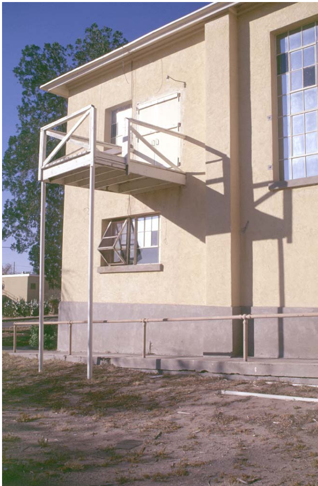
Photograph 23. Unused gymnasium fire escape tower.
