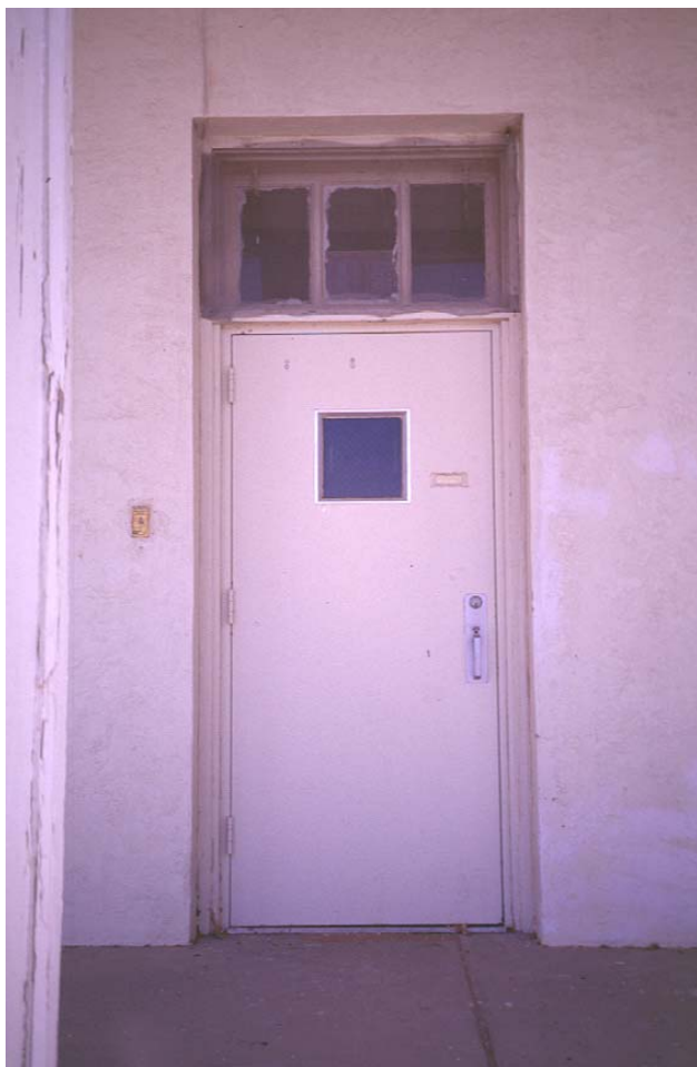
Photograph 44. Non-historic barracks replacement door.
