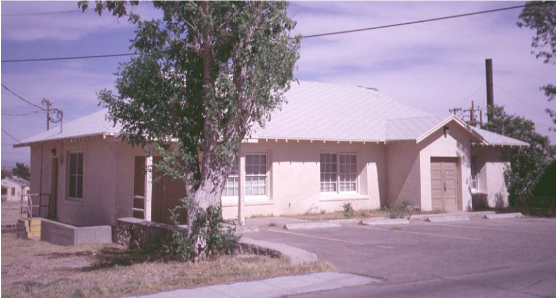
Photograph 68. Exterior slab and parking area at BOQ.
