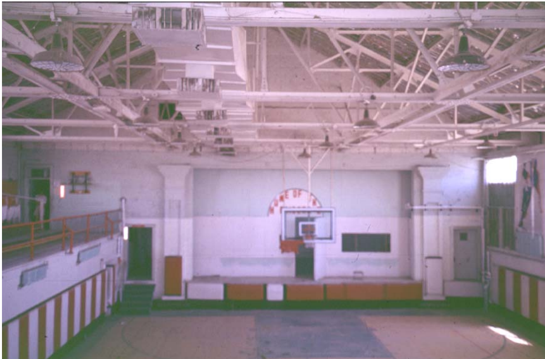
Photograph 29. Ornamental pilasters inside gymnasium.
