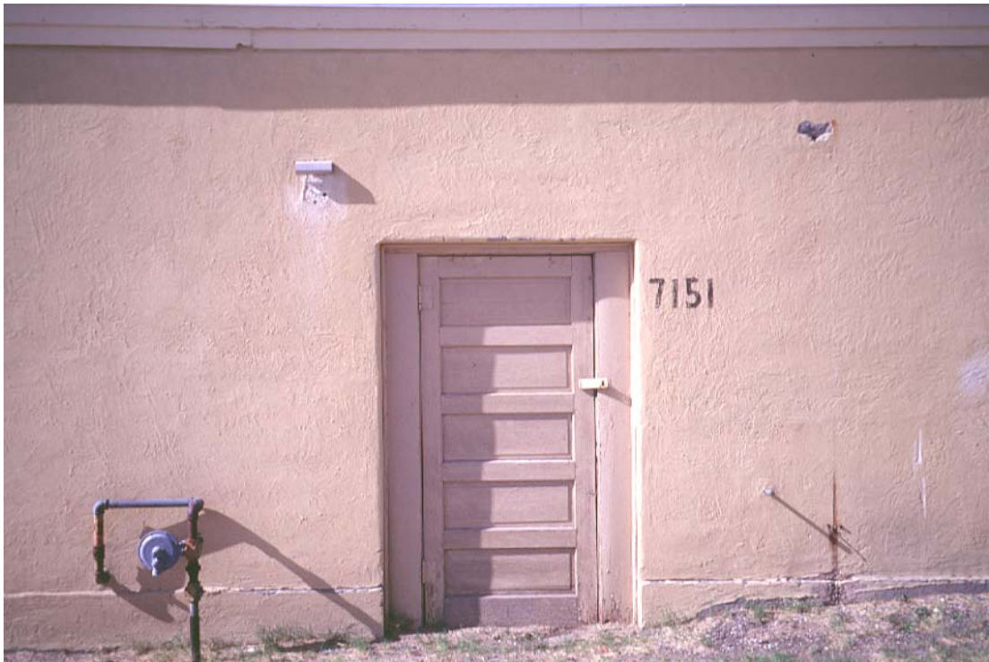
Photograph 14. Chapel site drainage detail.
