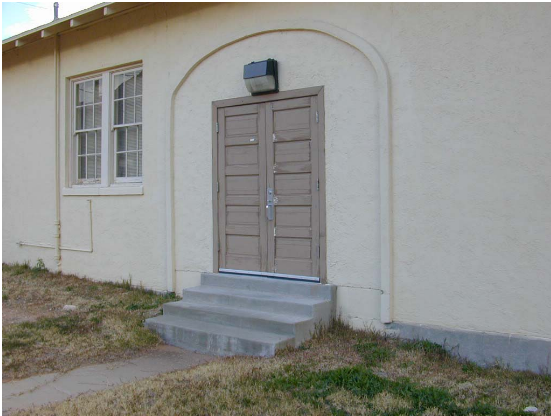
Photograph 79. Original arch opening in Conference Center.
