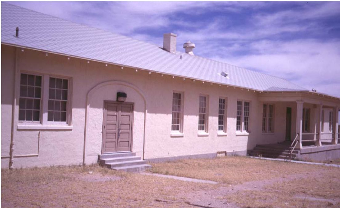
Photograph 70. Exterior photograph of Building 7167 (conference center).
