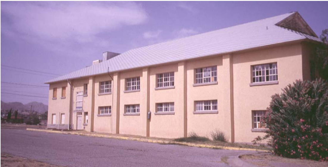
Photograph 19. Exterior photograph of Building 7155 (gymnasium).
