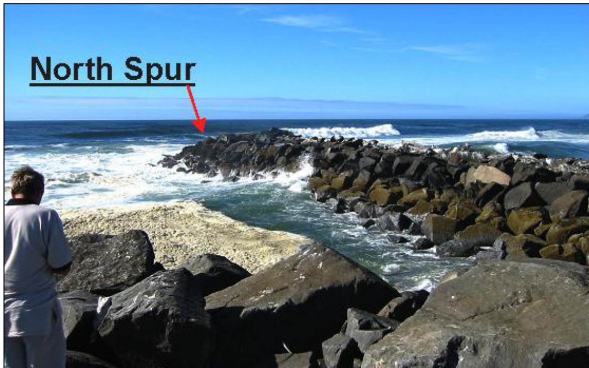
Figure 2. Example of spur construction at Siuslaw River, OR
