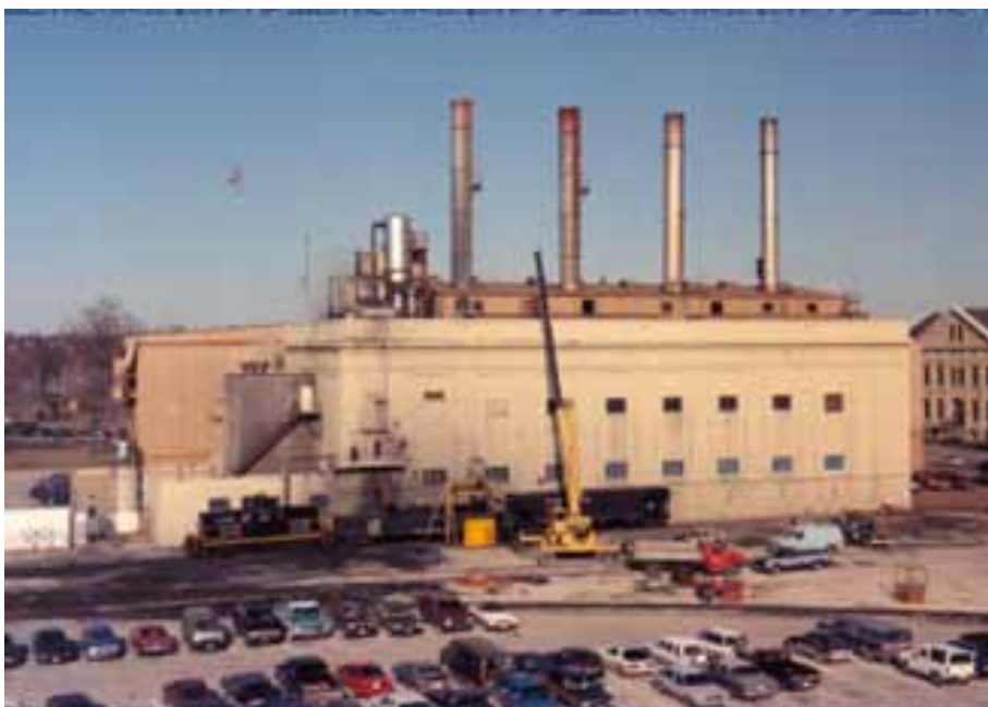
Figure 21. General view of the coal-fired central boiler plant.
