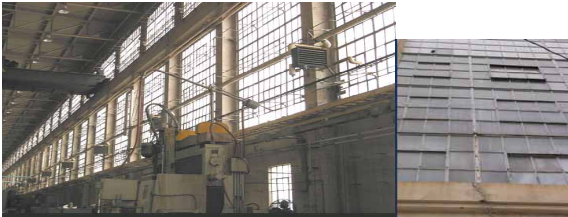
Figure 15. Building envelope of the Building 220.
