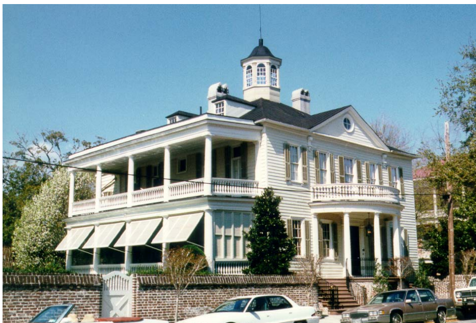
Figure 8. Returning a building to its original color may be helpful from a sustainable point of view (source, R. Young).
