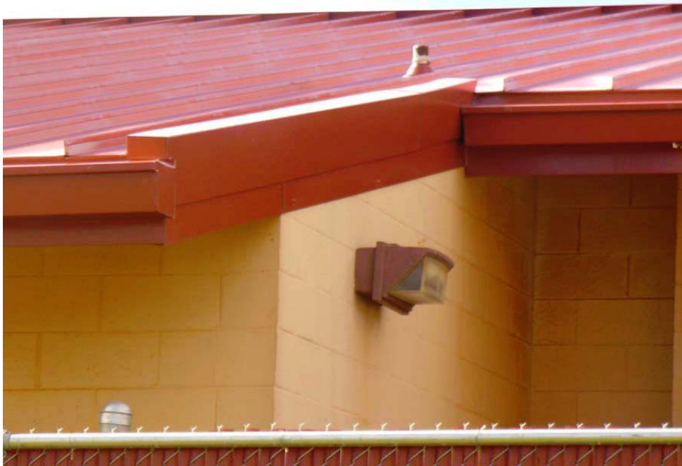
Figure 23. Finished detail work of fascia and gutter.
