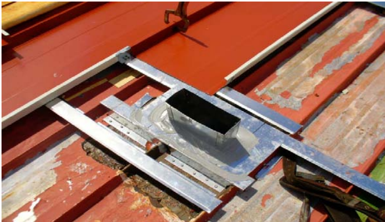
Figure 19. Installation of vent flashing support purlins.
