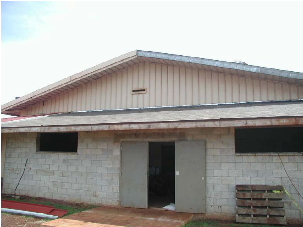
Figure 24. Building addition with asphalt shingles prior to metal roof installation.
