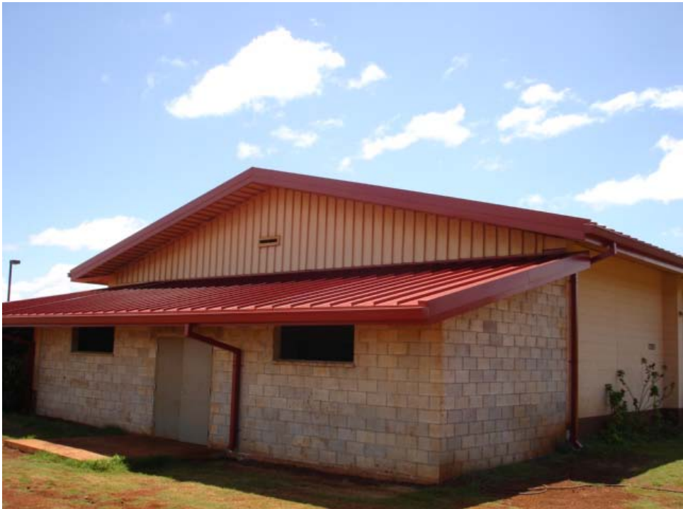
Figure 25. Building addition with finished standing seam roof.
