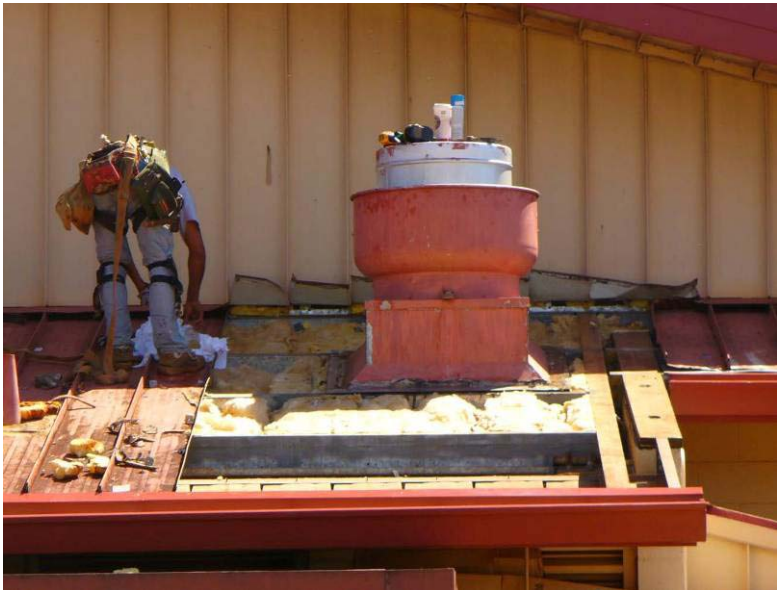
Figure 21. Demolition of lower roof above kitchen area.
