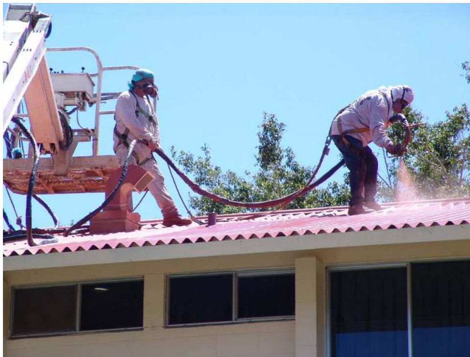
Figure 27. Topcoat being applied with overspray evident.
