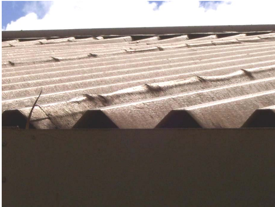
Figure 2. Existing roof on Building 118 prior to demonstration.
