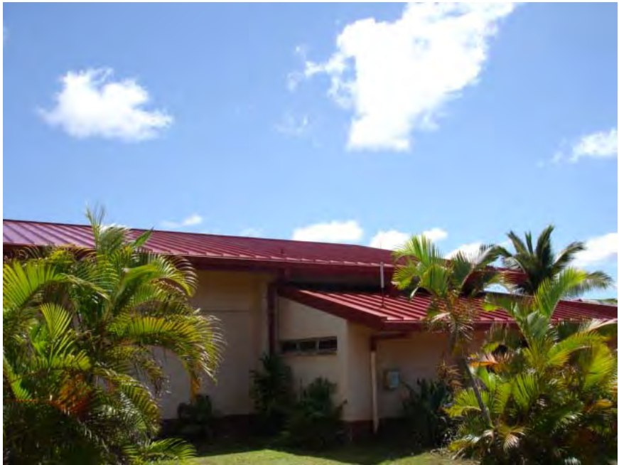
ROOF AFTER - 17 SEPT 08
