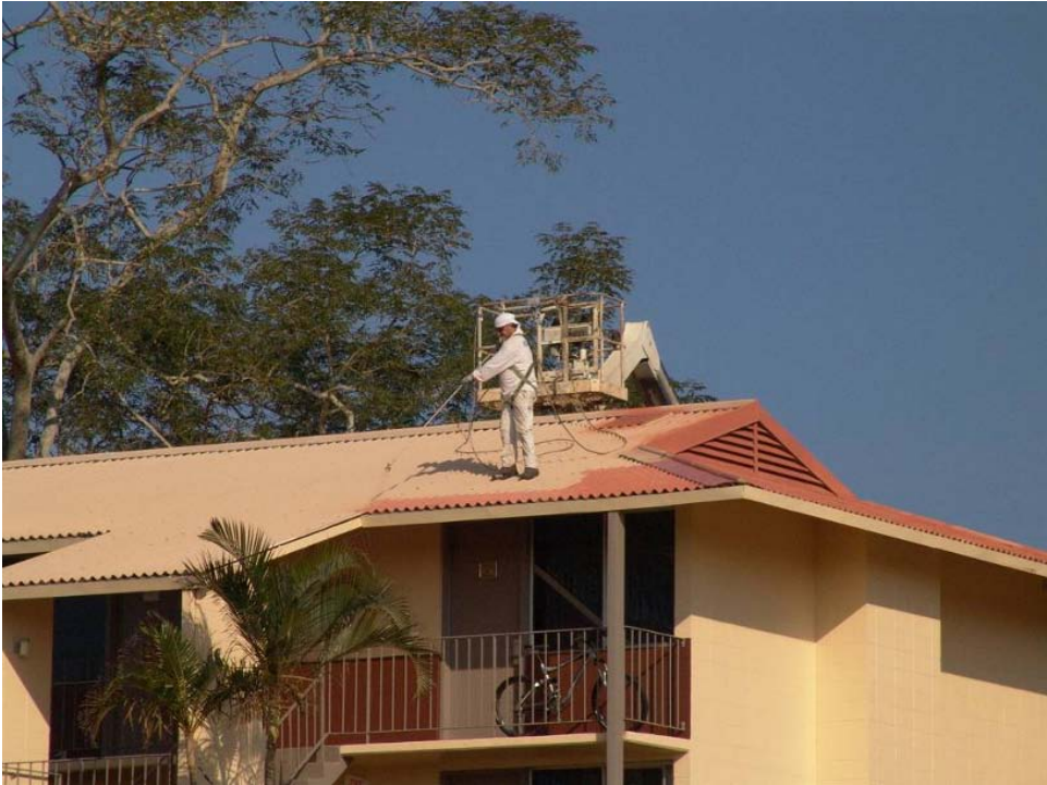
Figure 6. Spraying primer coat.
