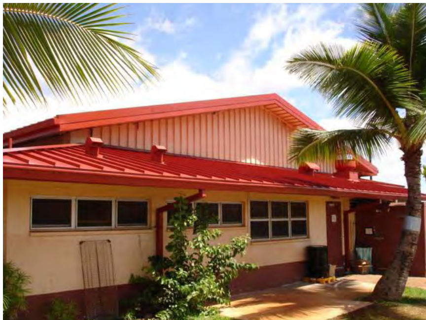
ROOF AFTER - 17 SEPT 08
