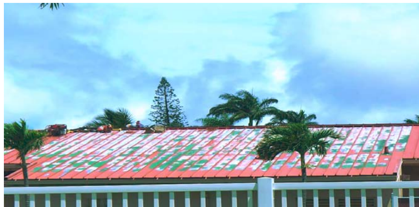
Figure 11. Pressure washed and rust-treated roof areas.
