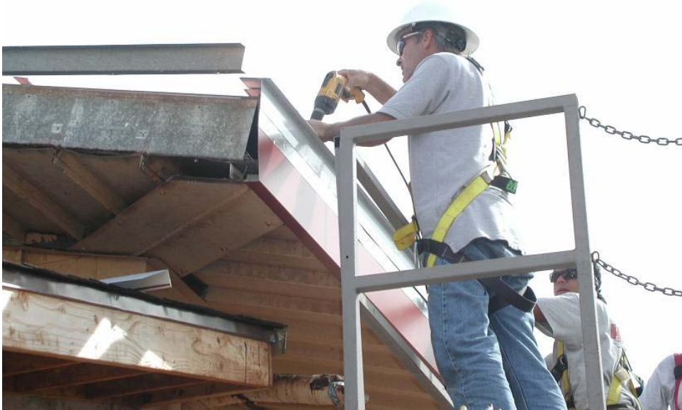
Figure 14. Installation of fascia flashing.
