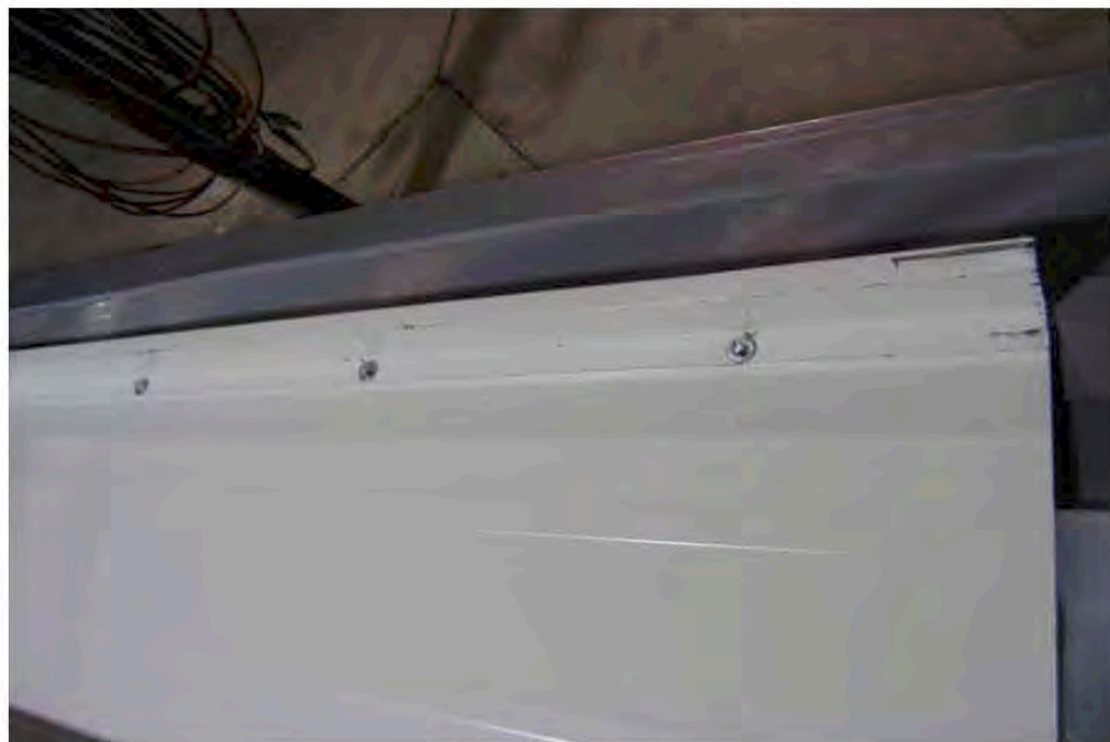
PHOTOGRAPH 4 FIRST PANEL INSTALL
