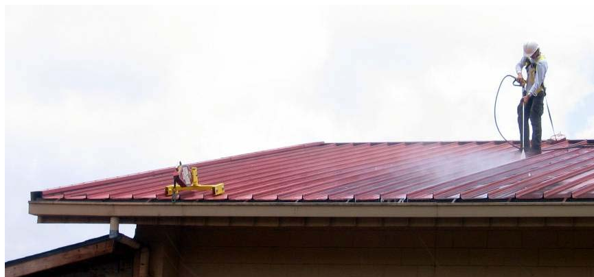
Figure 12. Pressure washing upper roof
