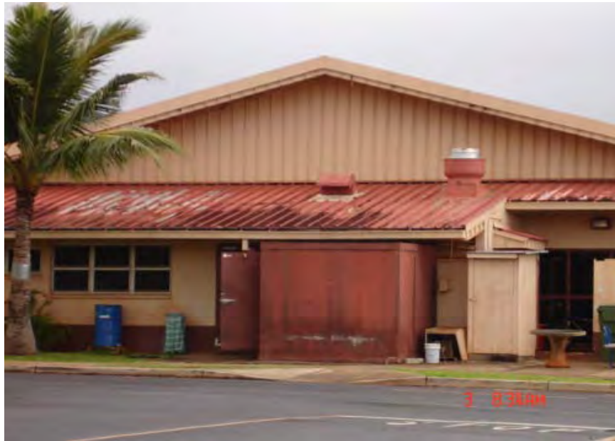
ROOF BEFORE - 03 AUG 08
