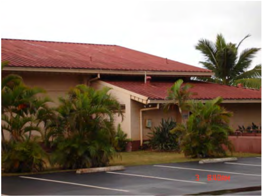
Roof Before - 03 Aug 08
