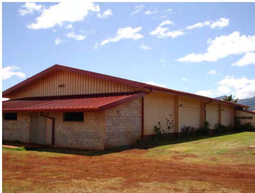
ROOF AFTER - 17 SEPT 08
