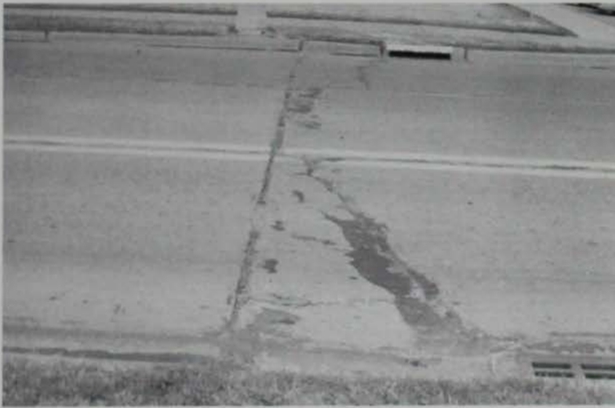
Figure 34b. Medium-Severity Punchout.
