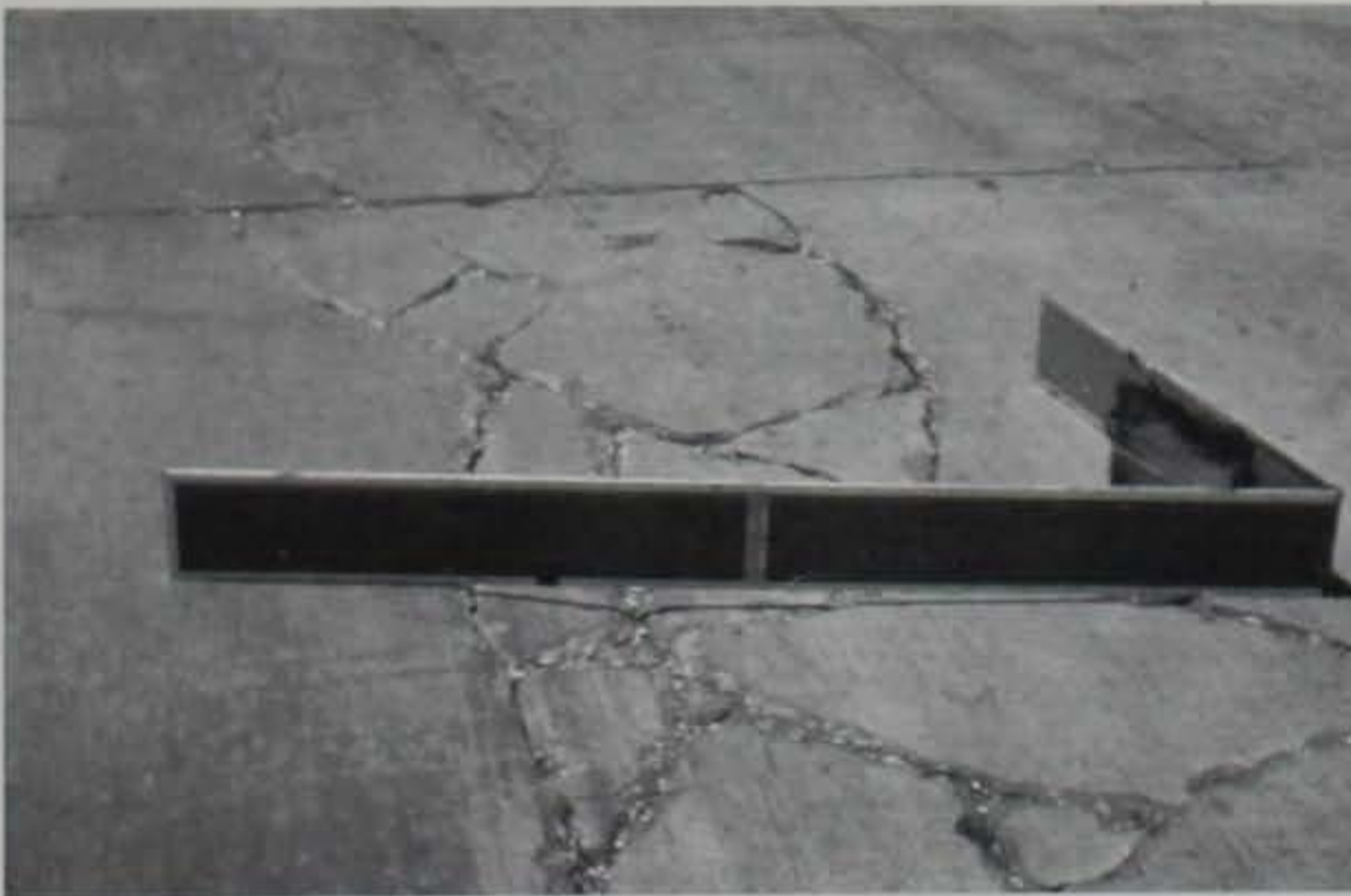
Figure 34c. High-Severity Punchout.
