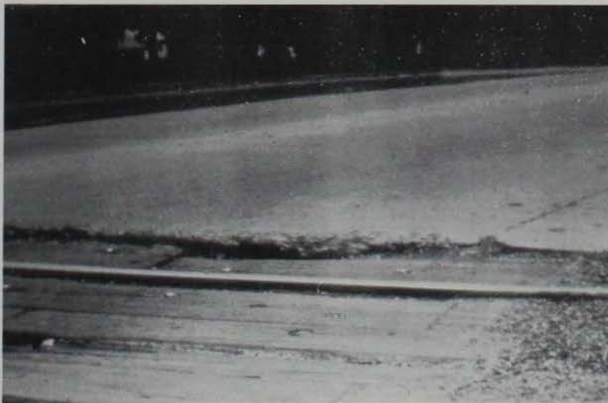
Figure 35c. High-Severity Railroad Crossing.
