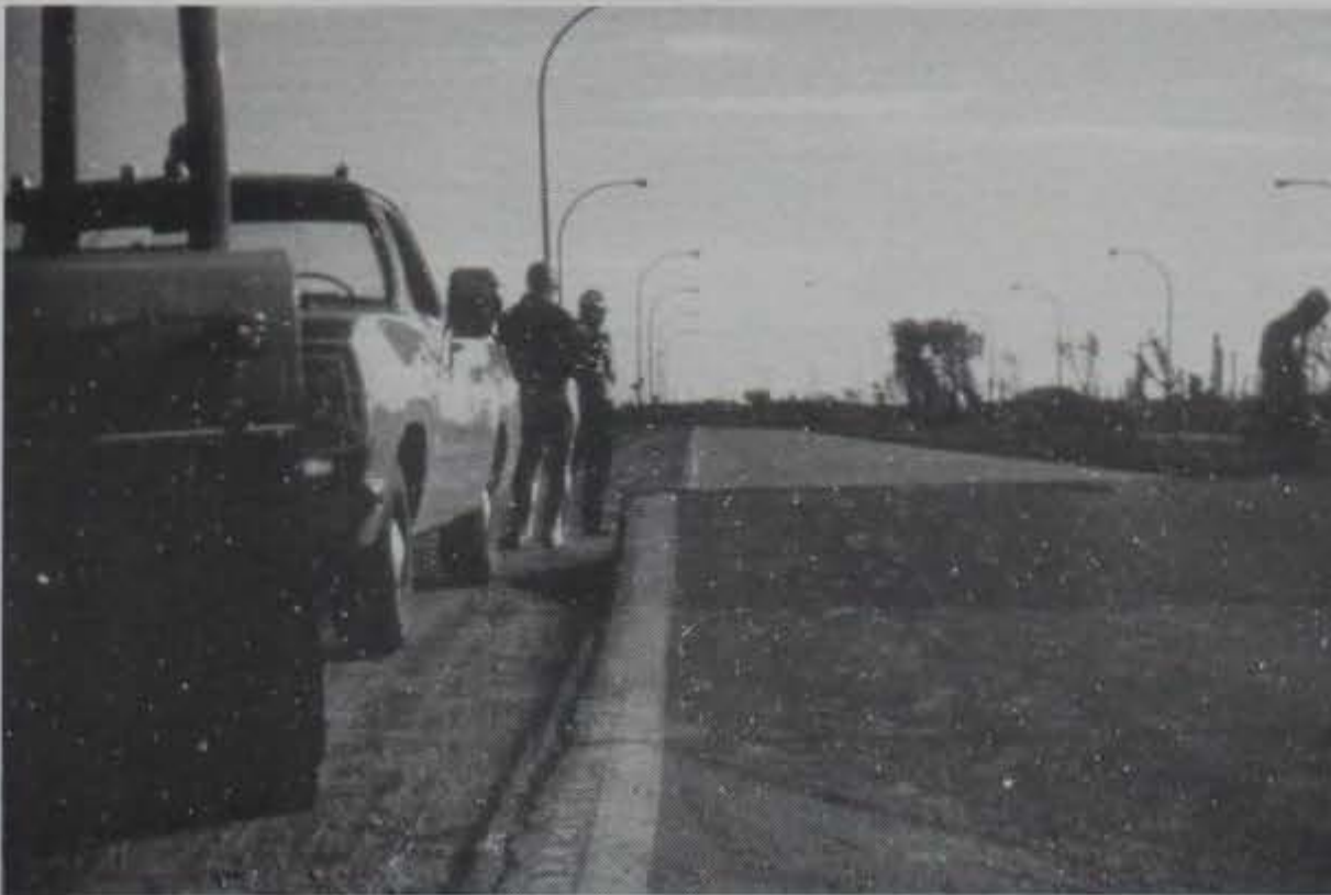
Figure 21c. High-Severity Blowup/Buckling.
