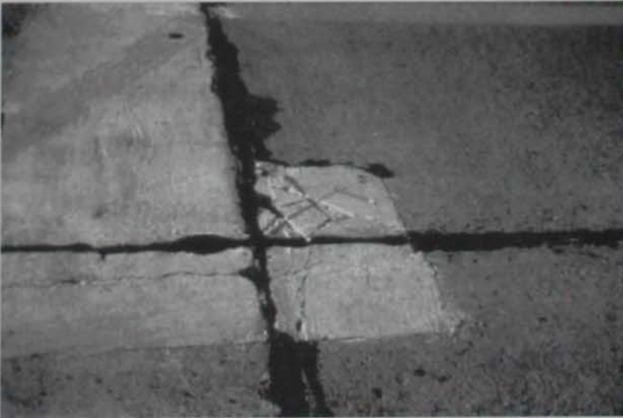
Figure 30b. Medium-Severity Patching, Small.
