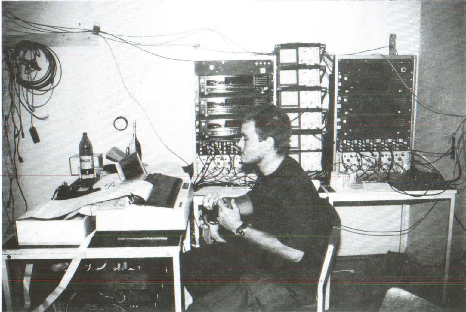
Figure 13. The instrument control room—data collection station.
