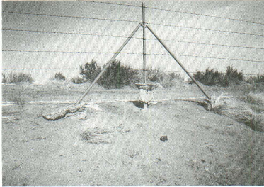
Figure 10. Typical eroded site along a fence line.
