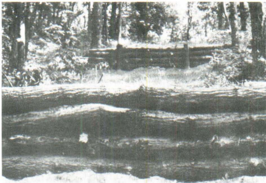
Figure 4. Substitution of log timbers for railroad ties on a steep slope.
