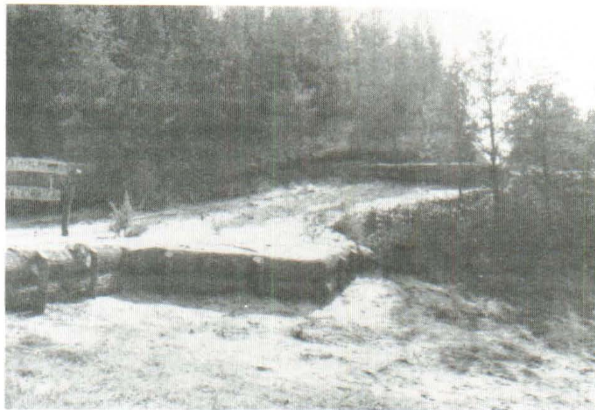
Figure 6. Slope stabilization at varying elevations.
