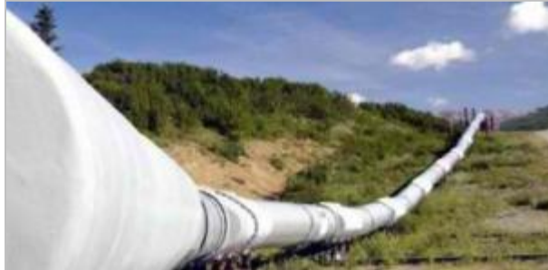
Figure 26. Seventy-two-in. pipe.
