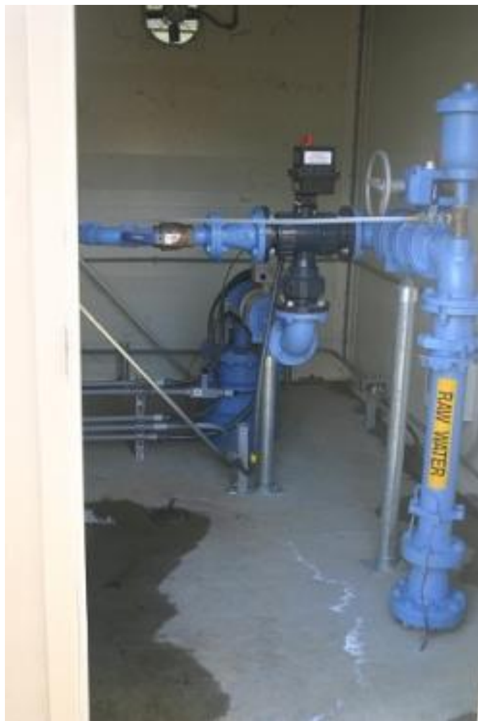
Figure 45. New well construction at Camp Rilea.
