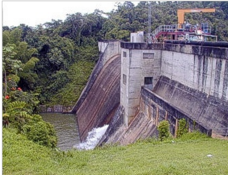
Figure 29. Spillway at Lago de Cidra Reservoir.
