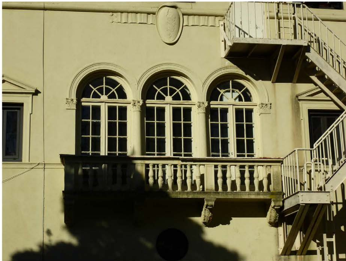
Photo 16. View to west of the French doors on the east facade that lead out from the second floor lounge.
