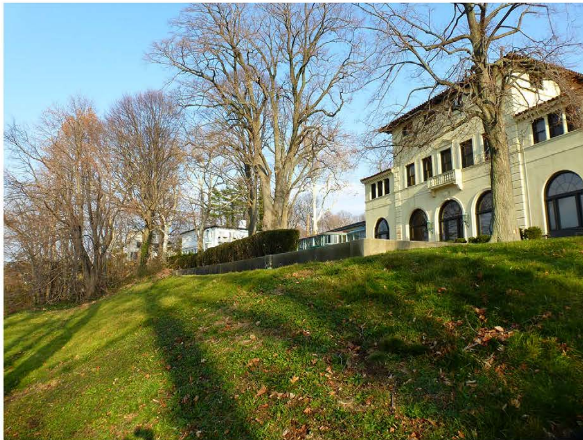
Photo 4. View to north showing the slope from the mansion down to the Long Island shore.
