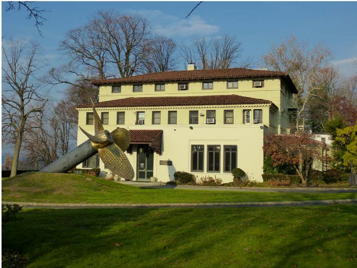
Photo 1. View to the north of the south facade.
