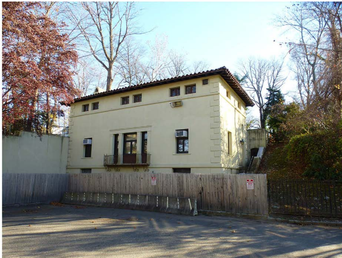
Photo 53. View to the northeast of the garage building.
