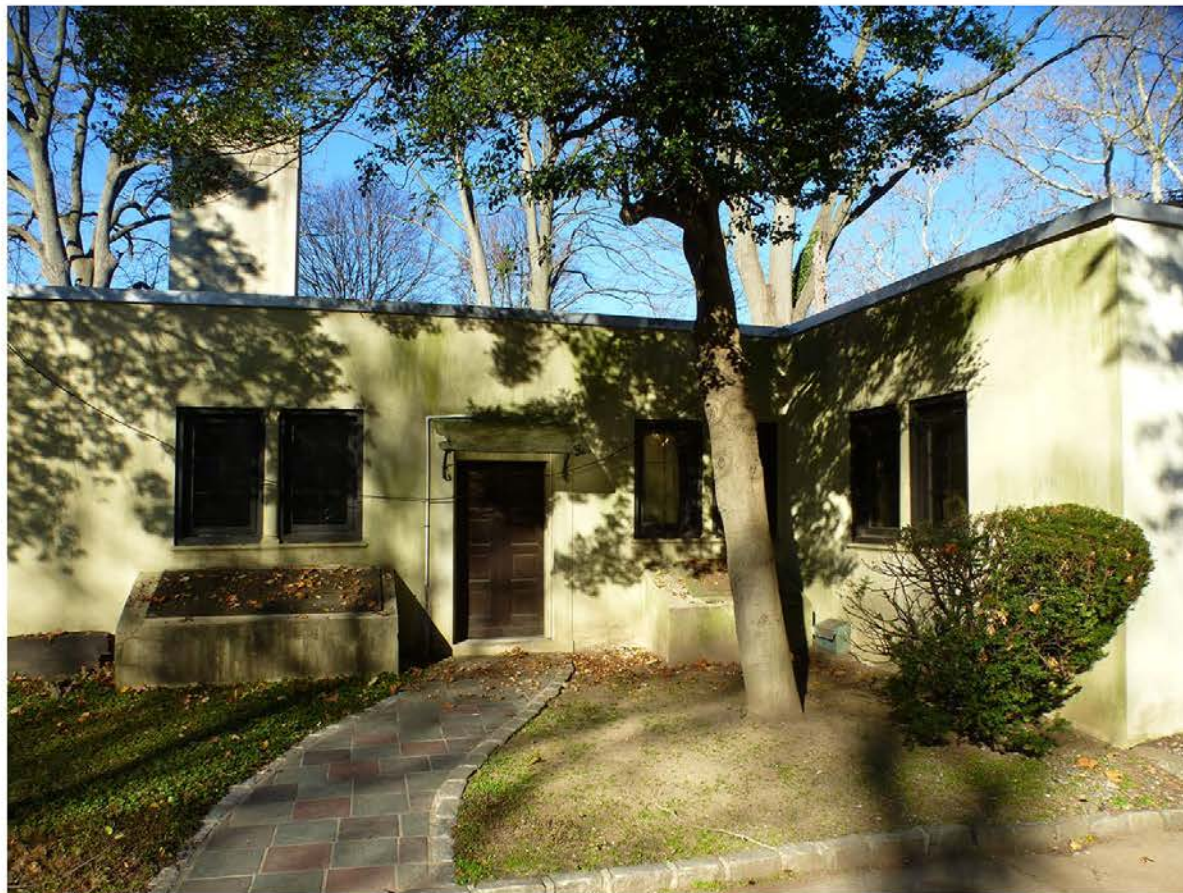
Photo 13. View to the west of the north entrance door into the music room addition.
