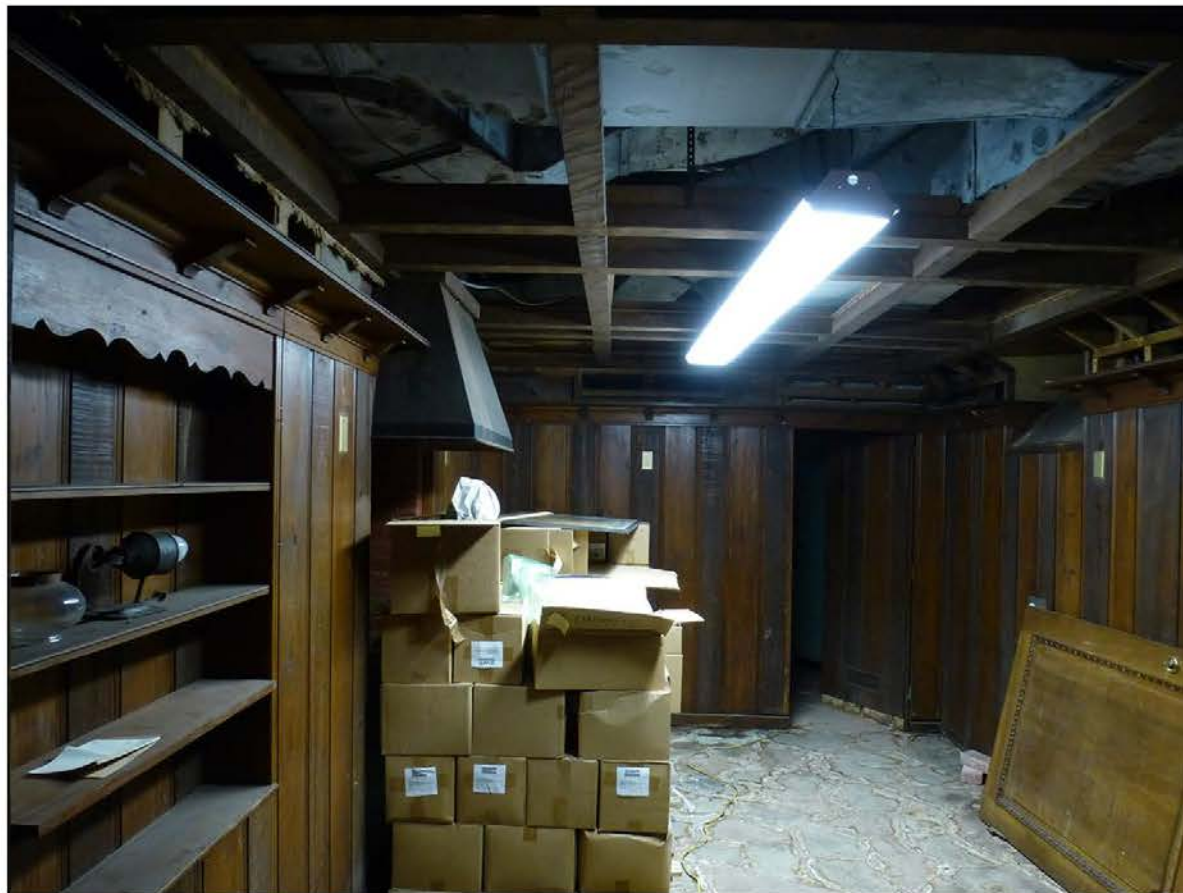
Photo 51. View to the north of the tap room in the basement of the music room addition.
