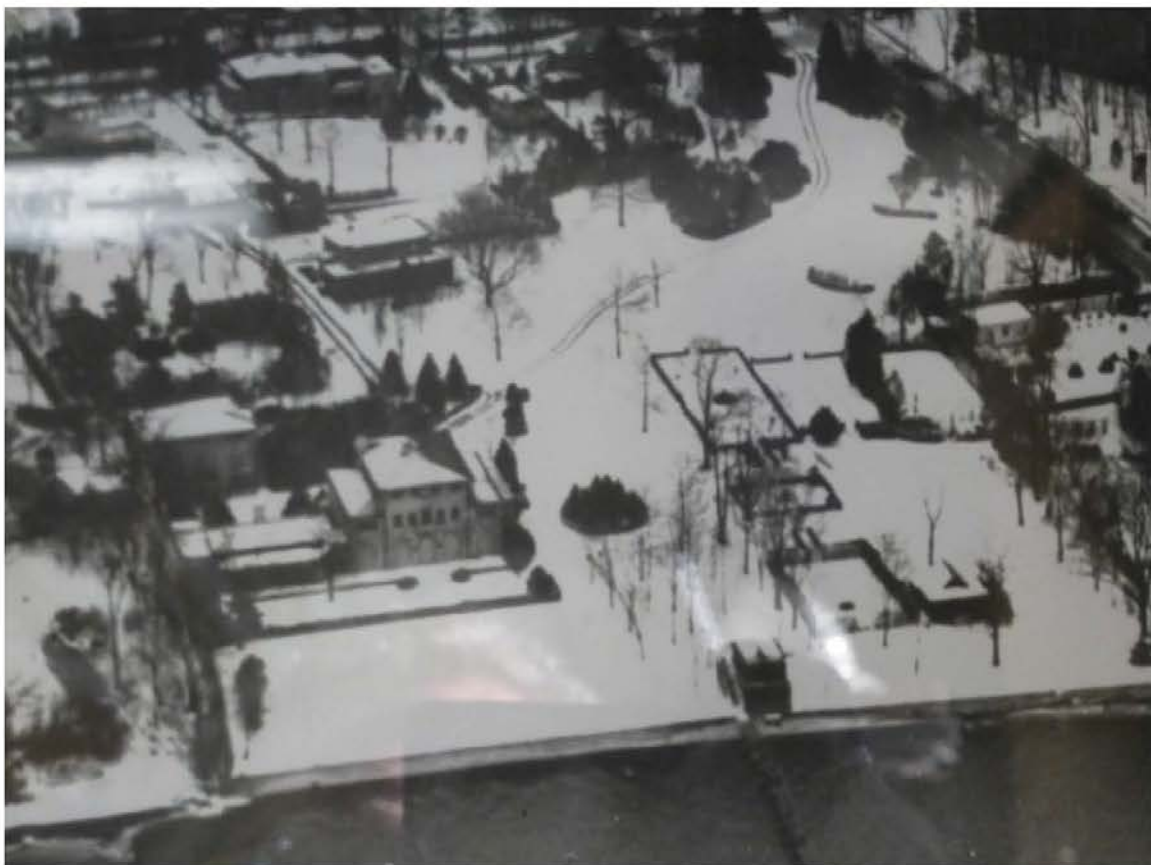
Figure 13. Aerial of post-1931 Barstow Estate, (Bland Library, USMMA). Visible in the photograph are the mansion (bottom left), the garage behind it, the guest house, the Superintendent's house (upper right), the parterre gardens, pier, boat house, and tea/summer house (next to the lowest garden). The folly is located in the bend of the driveway.
