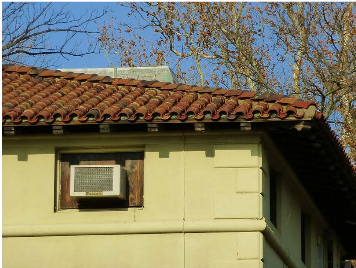
Photo 7. View to the north of the third floor showing a window opening, belt course, and quoins.
