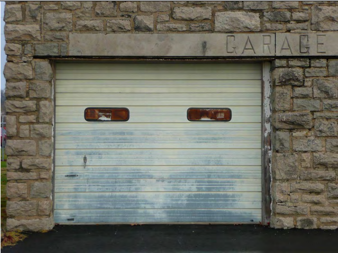
Photo 17 – replacement metal garage door on south elevation
