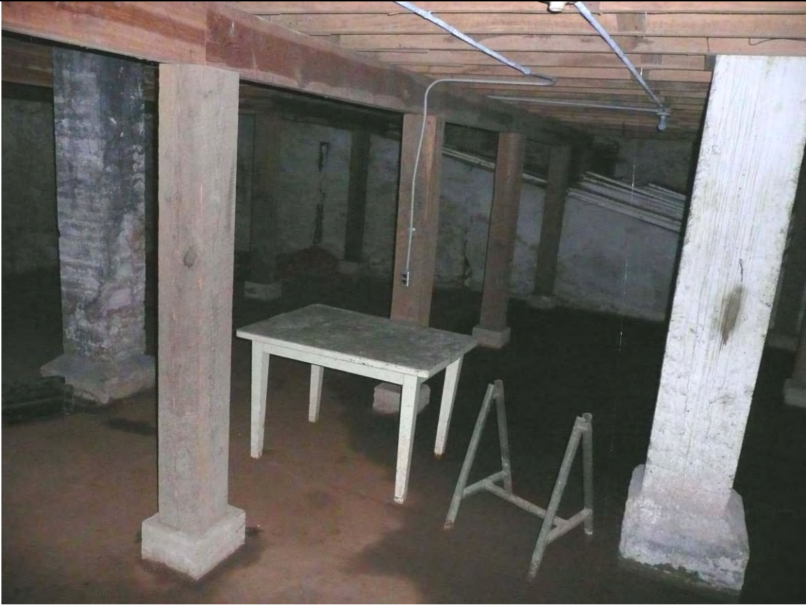
Photo 15 – view of added wood columns used to support first floor
