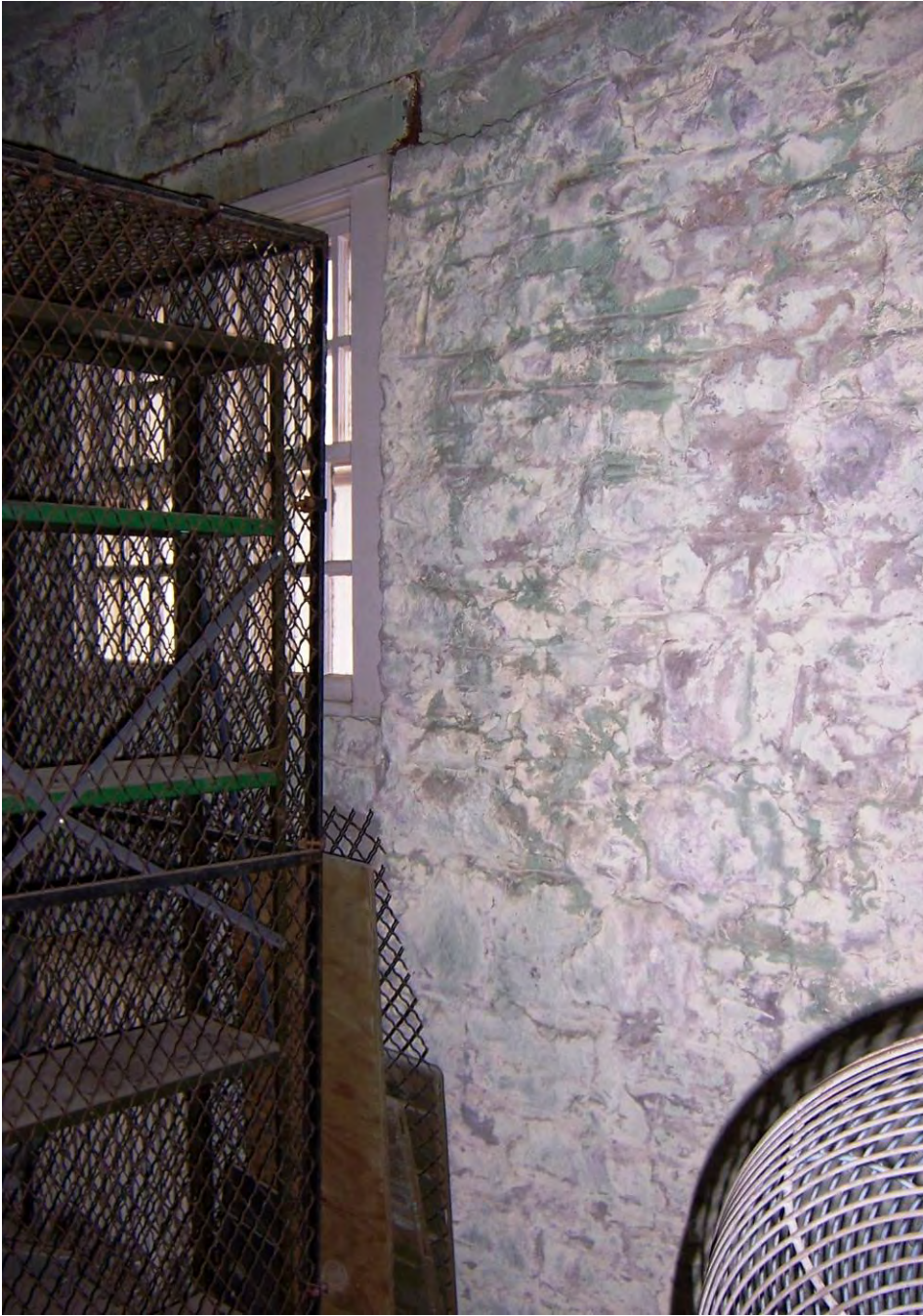
Photo 38 – interior view of cut limestone wall
