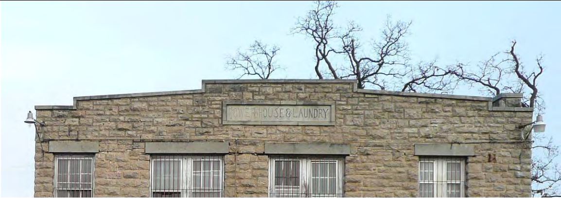
Photo 28 – stepped parapet detail on south elevation
