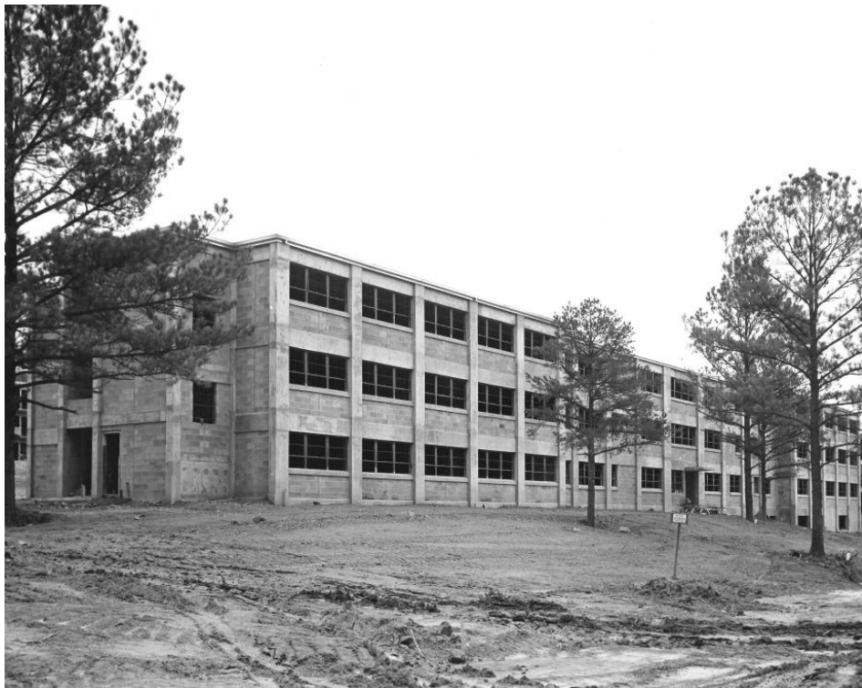
Figure 62. Typical Enlisted Women's barracks under construction at WAC Training Center, Fort McClellan, 1953 (WAC Museum, Vertical Files, File: Construction VI-A-13).
